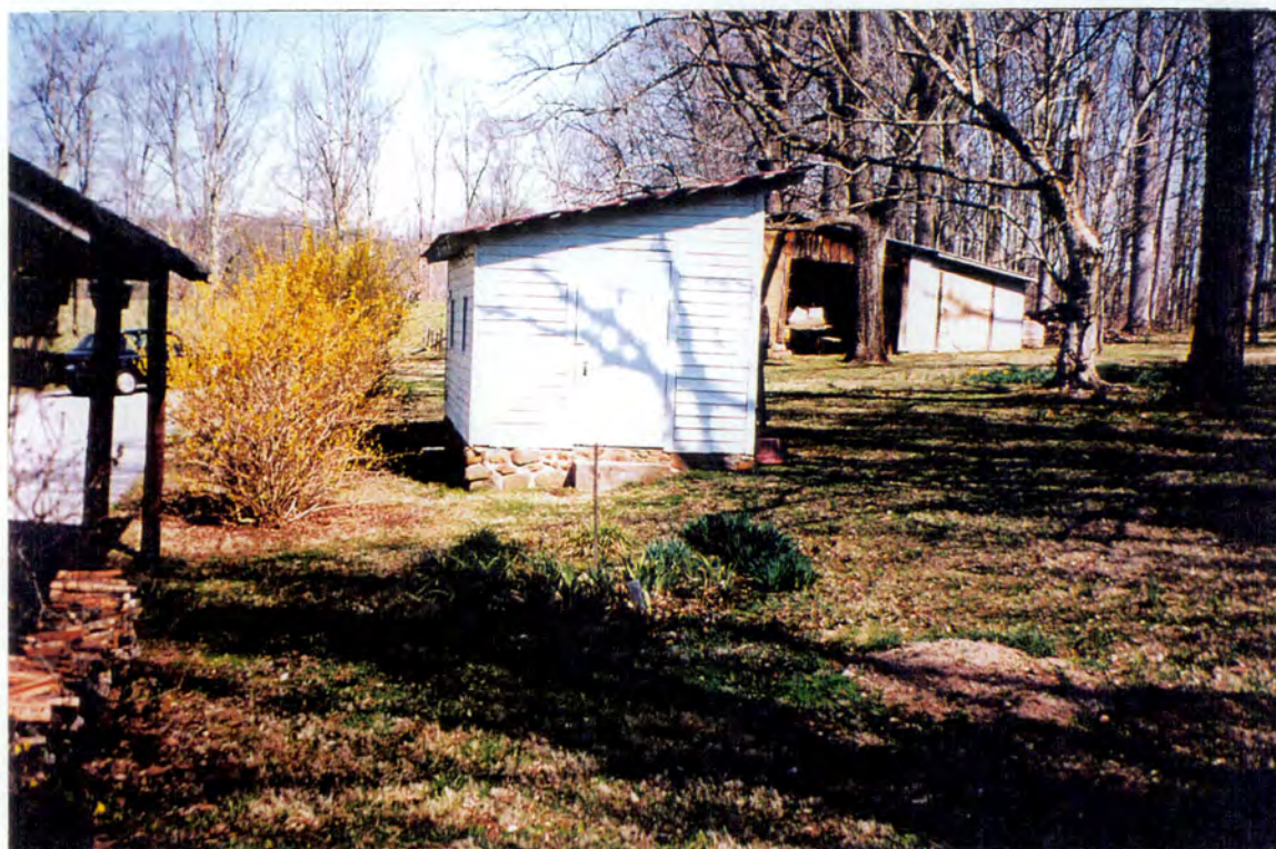
Relocated Milkhouse Herman A. Hauser House
