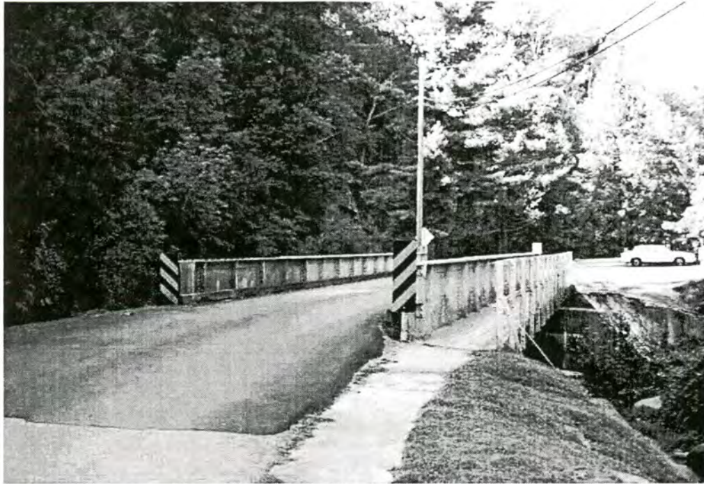
Figure 23: Bridge No. 175 over Big Creek
