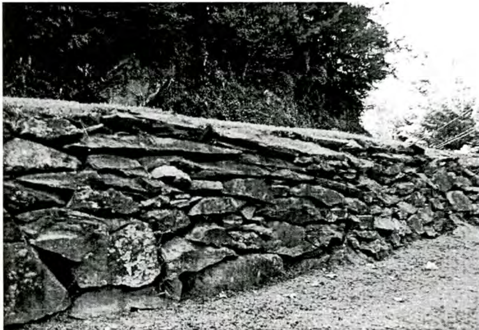
Figure 20: Waterville Village, wall
