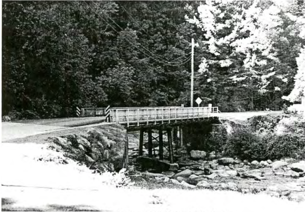
Figure 21: Bridge No. 175 over Big Creek
