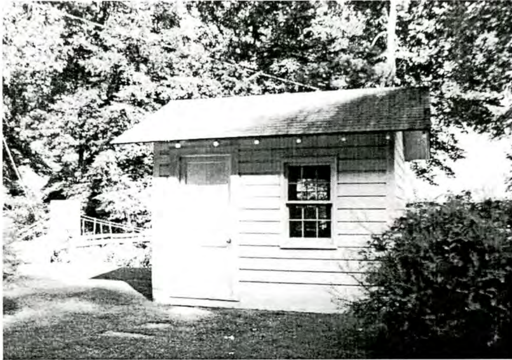
Figure 15: Waterville Village, pump house
