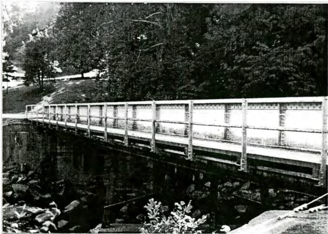
Figure 22: Bridge No. 175 over Big Creek
