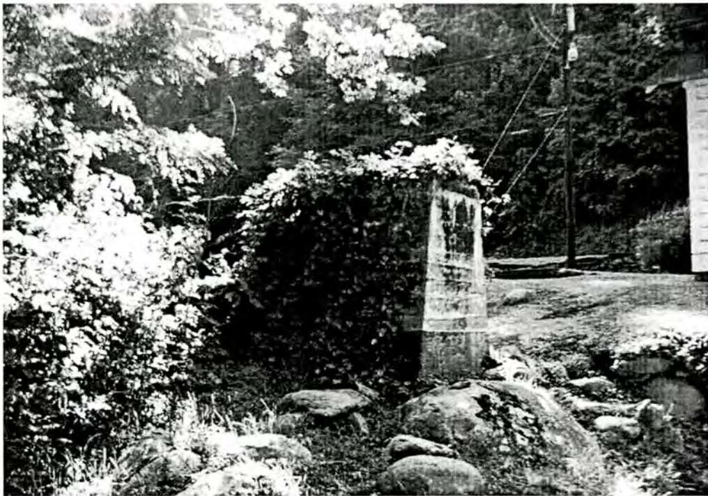
Figure 18: Waterville Village, footing of former pedestrian bridge
