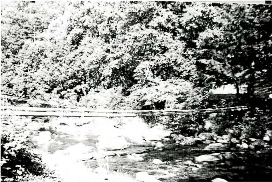
Figure 17: Waterville Village, waterline across Big Creek
