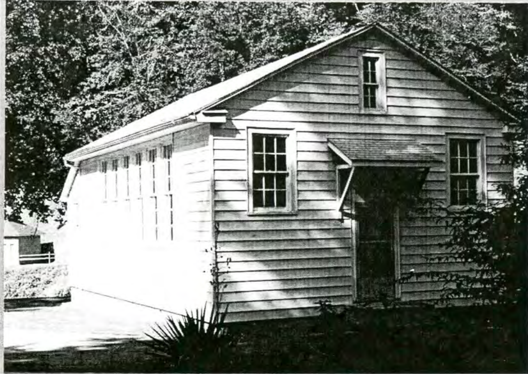
Figure 13: Waterville Village, former school
