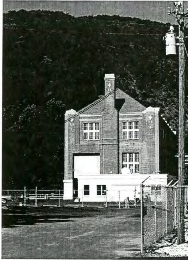
Figure 5: Walters Power Plant
