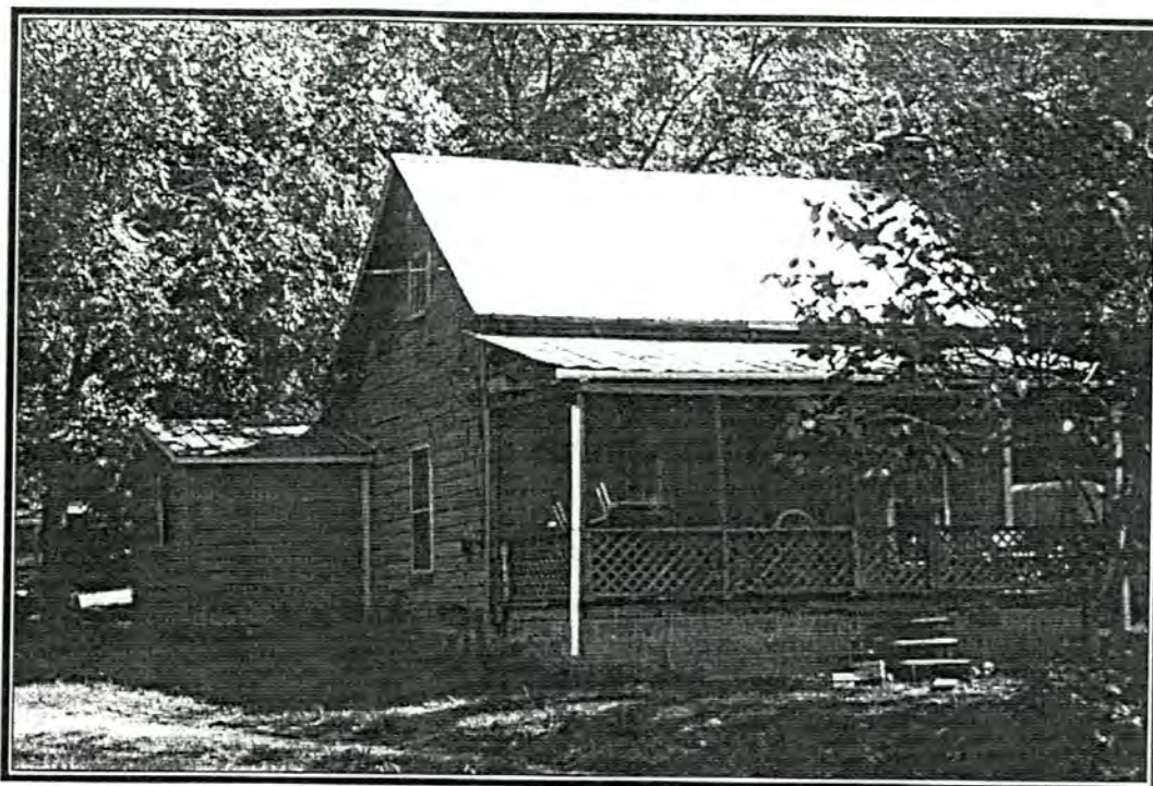
Photograph 1: Nineteenth-Century Log House, facing northeast
