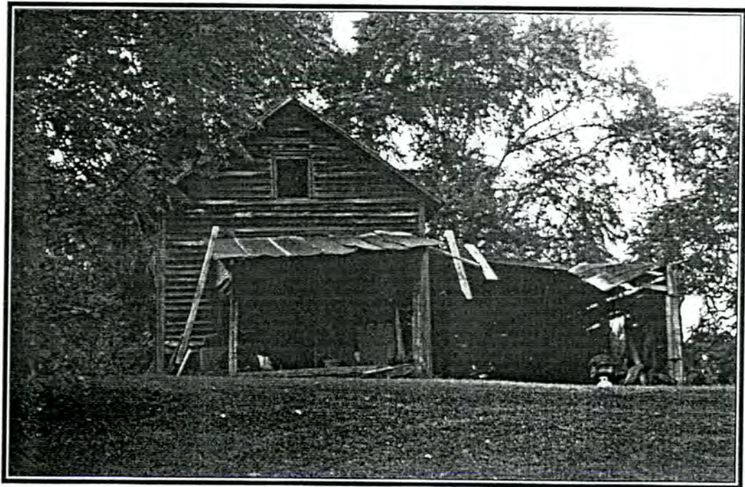
Photograph 4: Granary, view facing north
