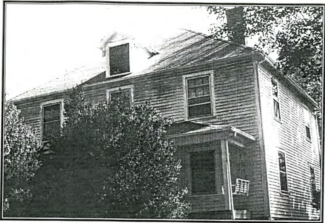
Photograph 1: Early Twentieth-Century Frame House, facing northeast
