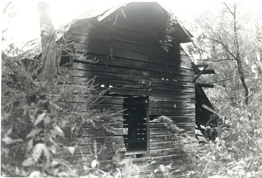
Plate 5. O. H. Winchester Farm, Ruinous Well House, Looking North.
