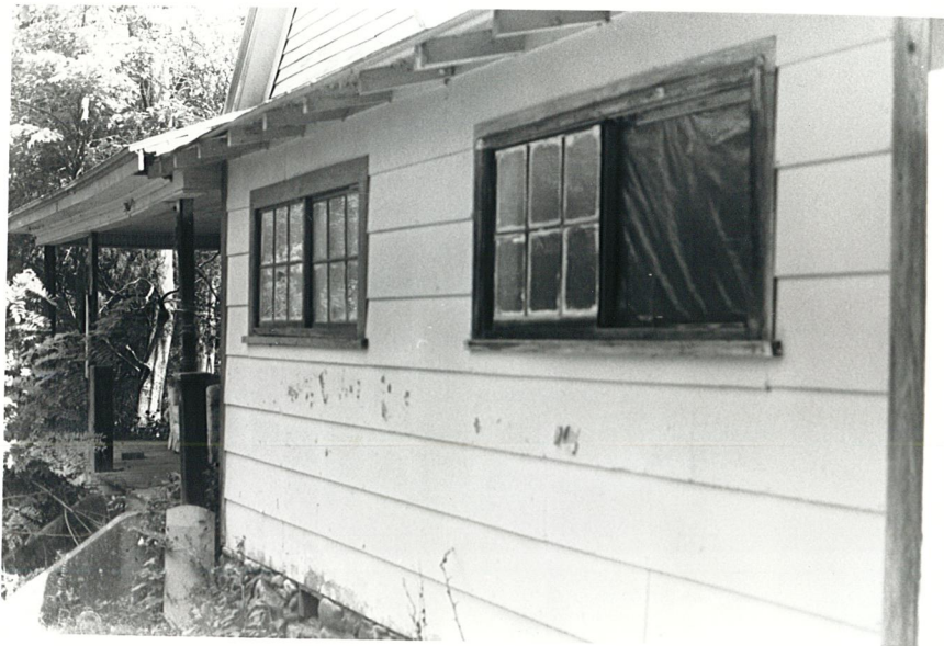
Plate 3. O. H. Winchester Farm, Winchester House, West Elevation, Looking East.
