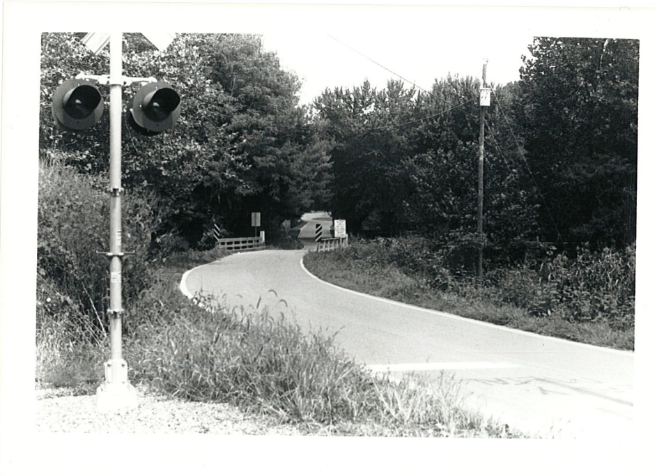
Plate 10. O. H. Winchester Farm, Looking North Towards Bridge No. 300.
