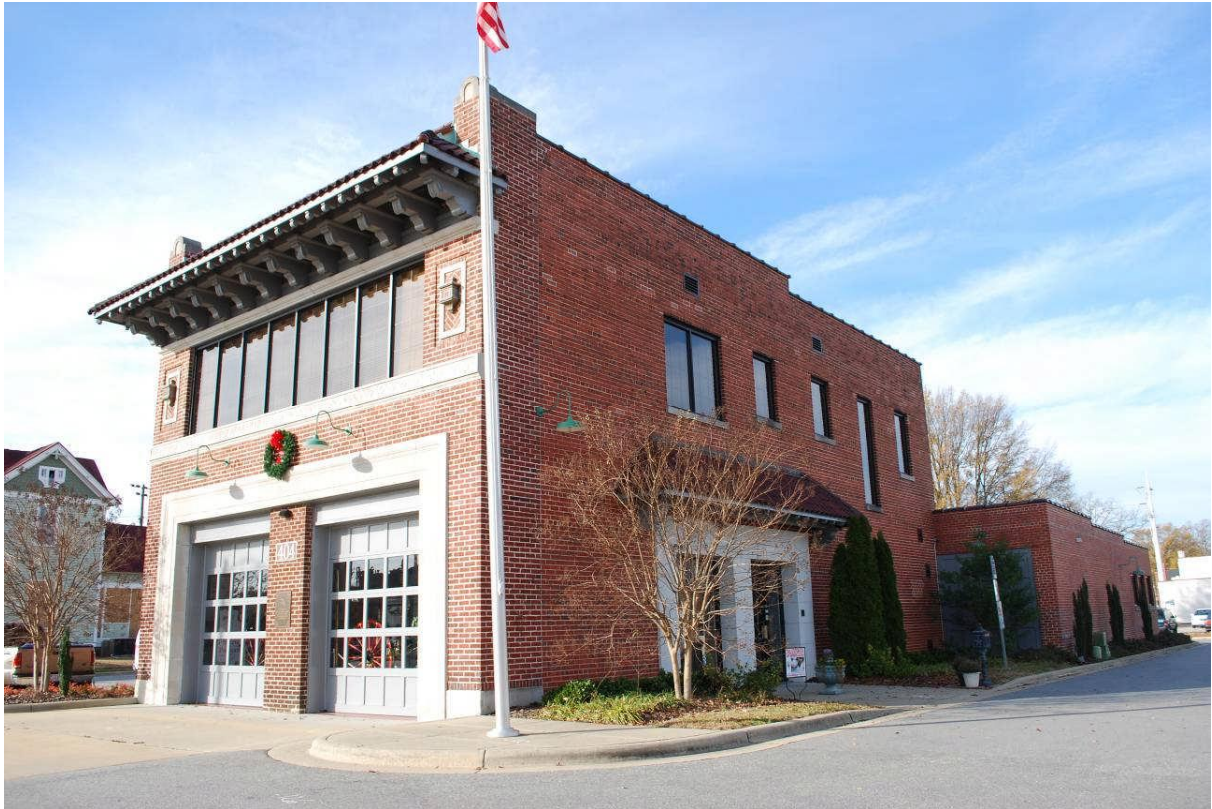
Fire Engine Company No. 2, 404 South Church Street, boundary increase
