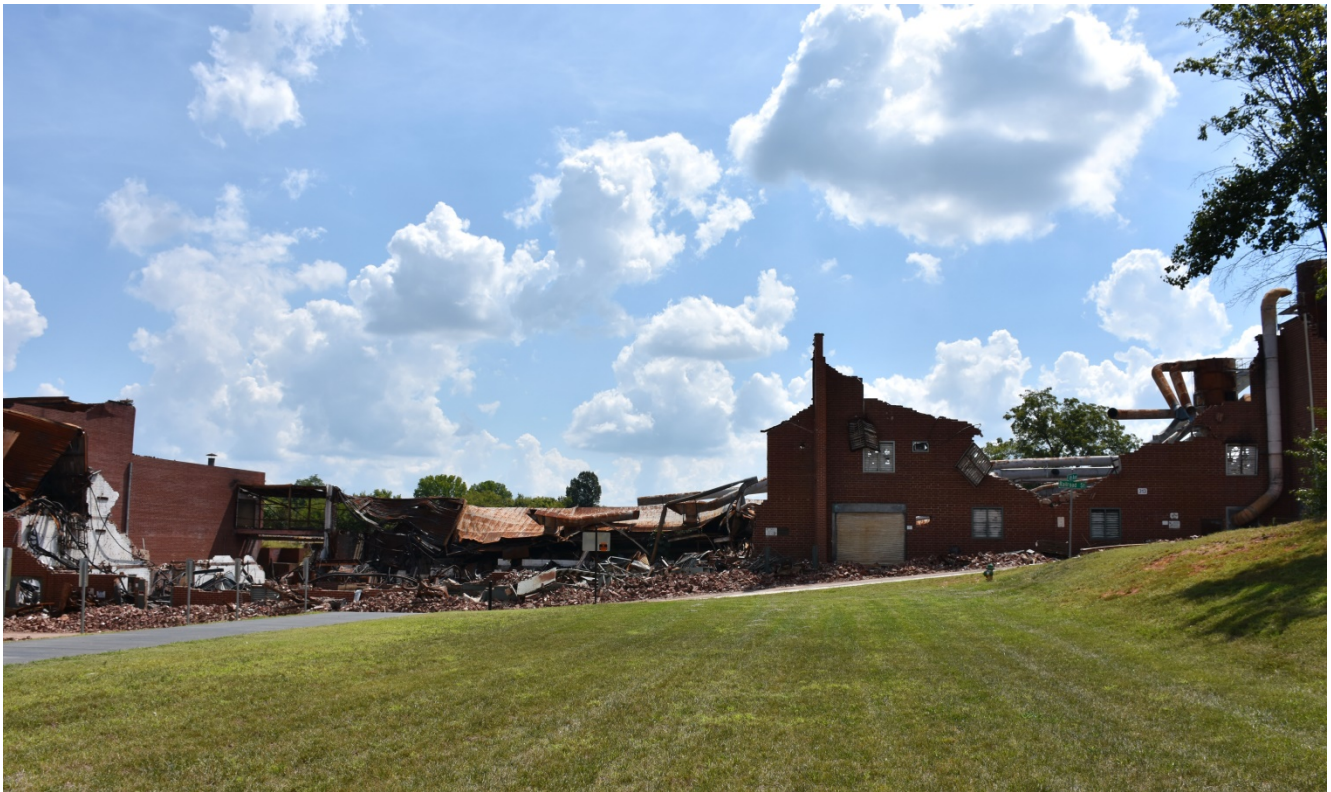
12. Dixie Furniture Company - Lexington Furniture Industries, Ruins of Building Nos. 25-14 to 25-16, South Railroad Street, looking south, September 7, 2018 Demolition commenced in November 2018
