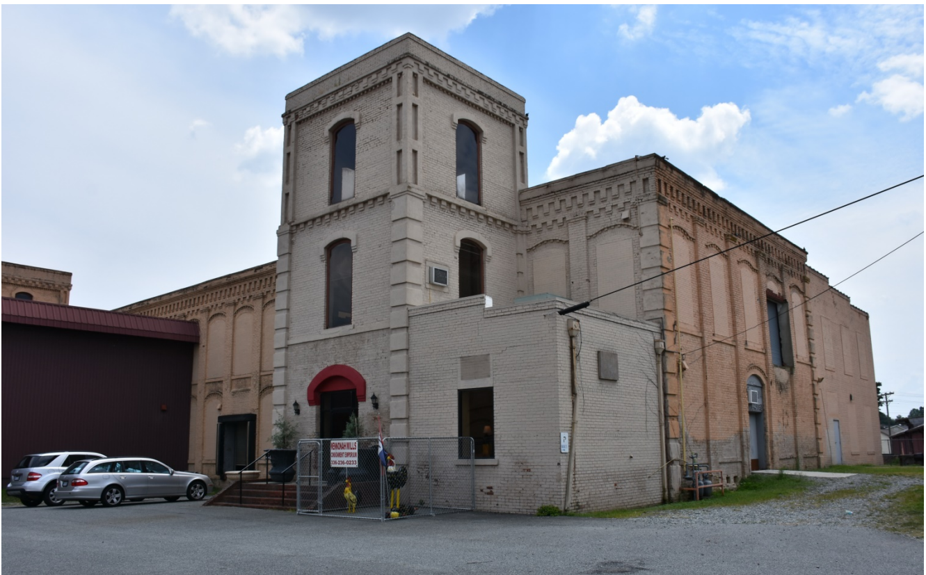
1. Wenonah Cotton Mill No. 1, 800 South Salisbury Street, looking southwest
