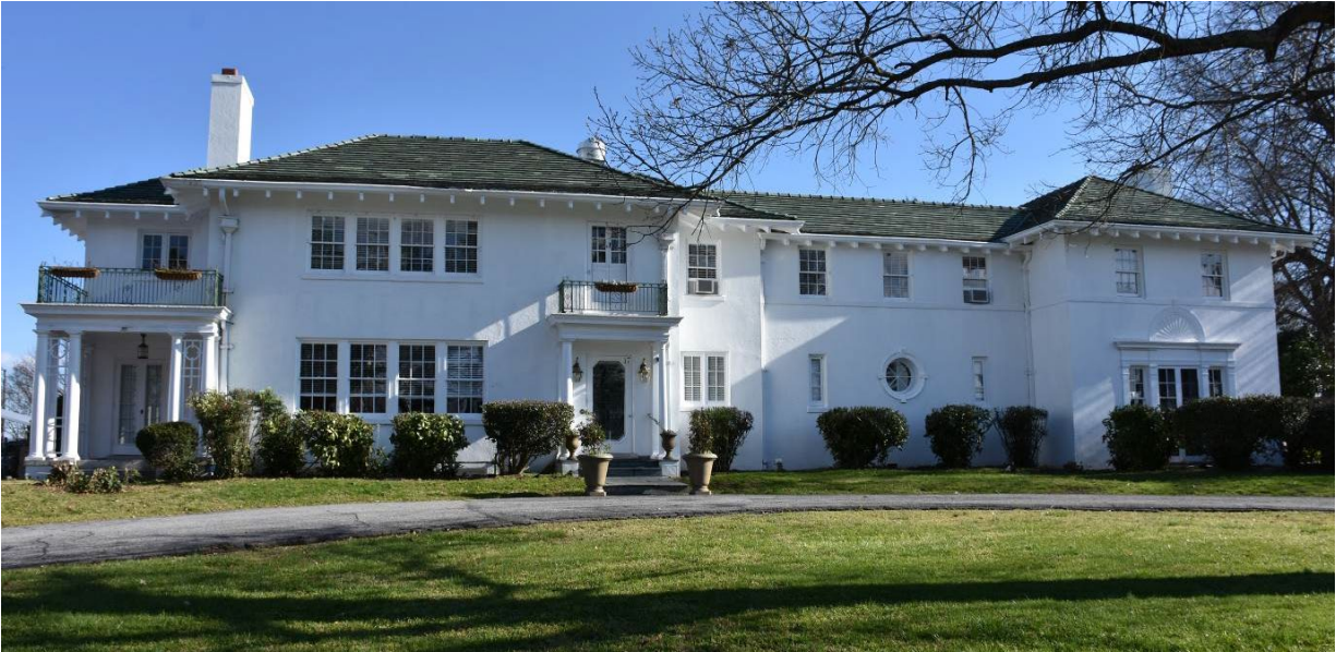
North elevation, looking south
