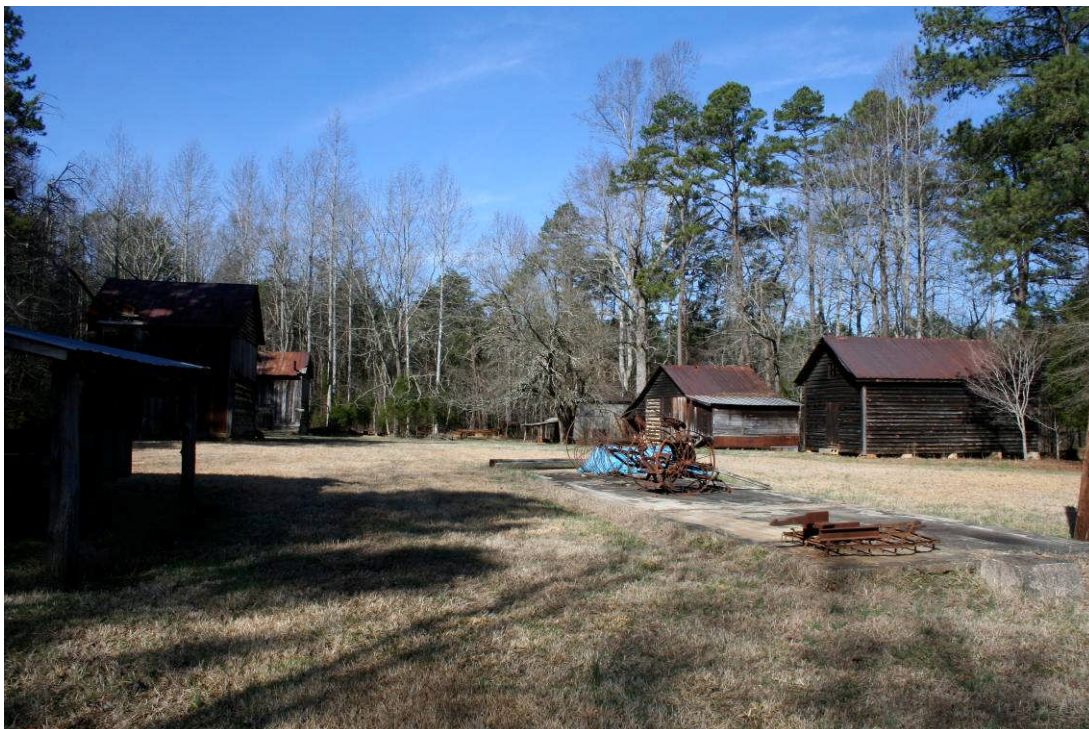
Farm outbuildings – general view
