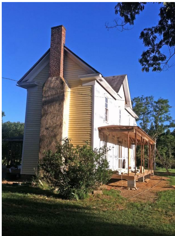
D. C. Umstead House – overall view
