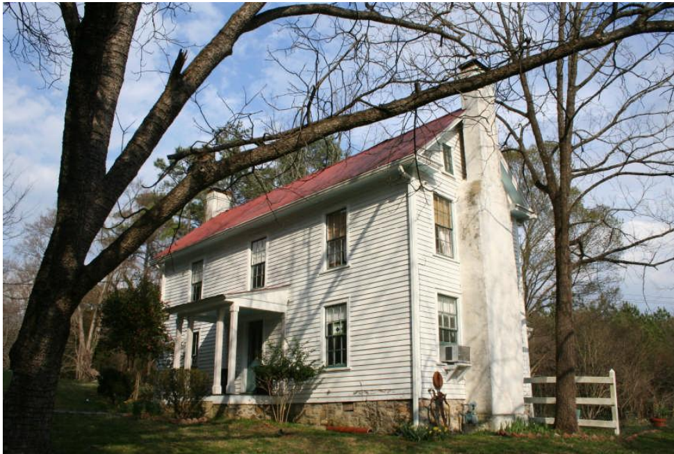
Overall front view
