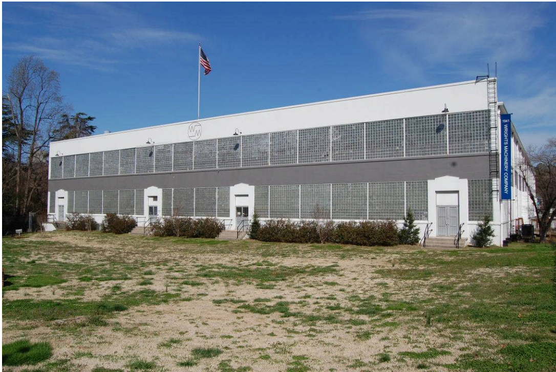
Façade and side view
