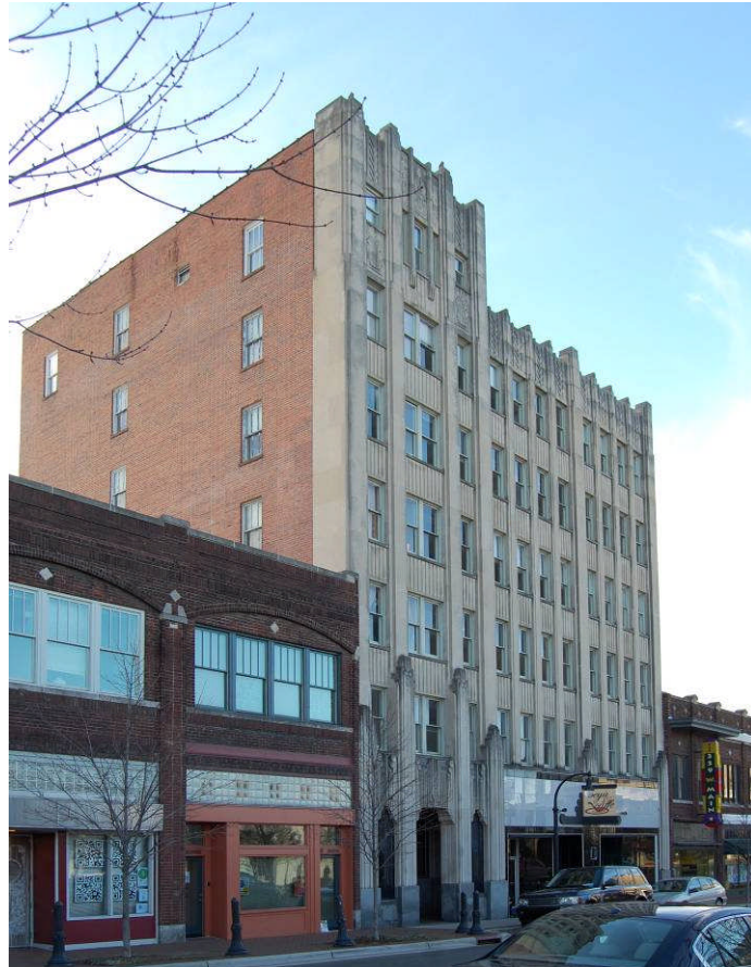
Snow Building, 331-335 West Main Street
