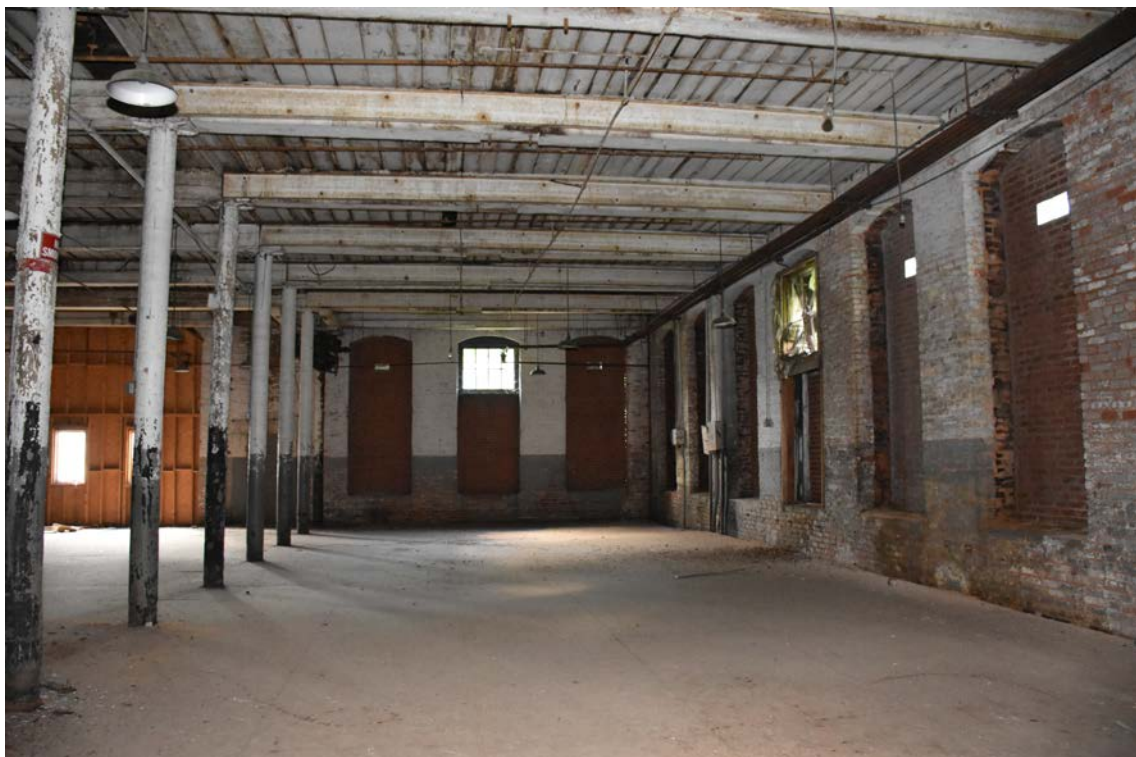
1896/1903 factory, first floor, southwest section, looking south
