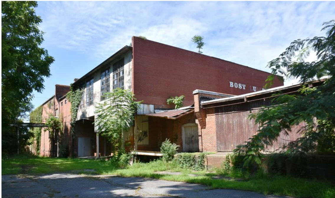
East elevation, north section, looking southwest
