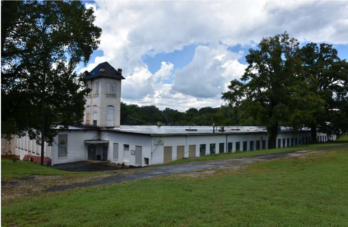
Southeast corner, view northwest
