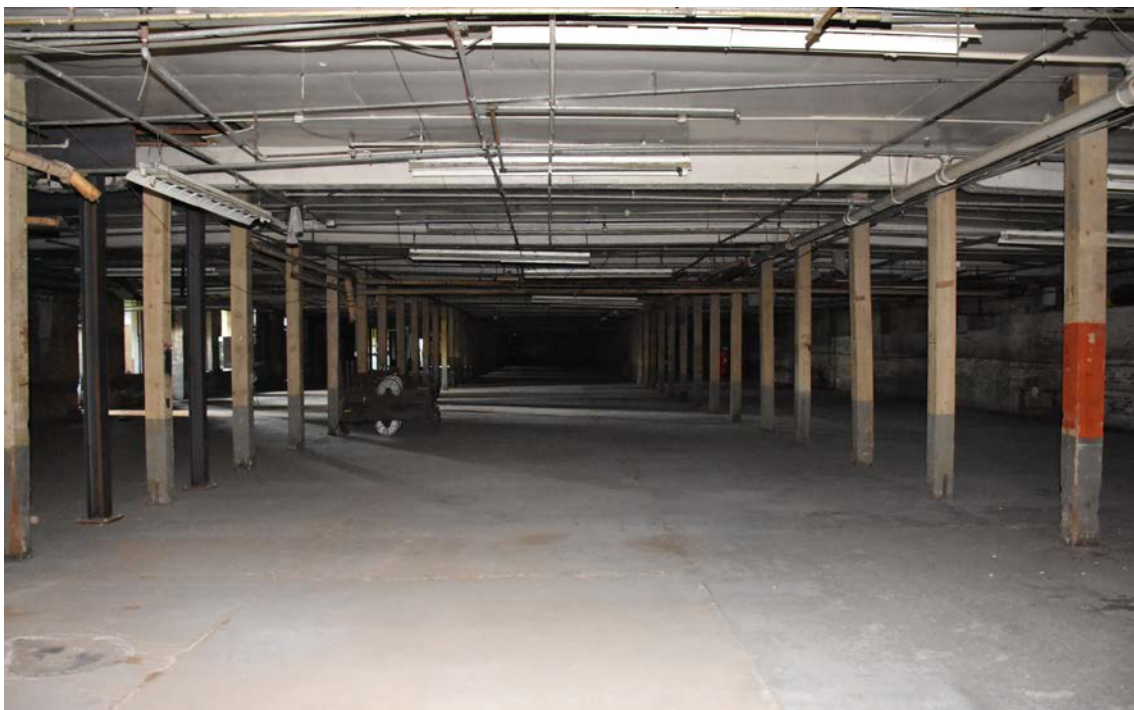
1902-1903 mill, basement, looking southwest
