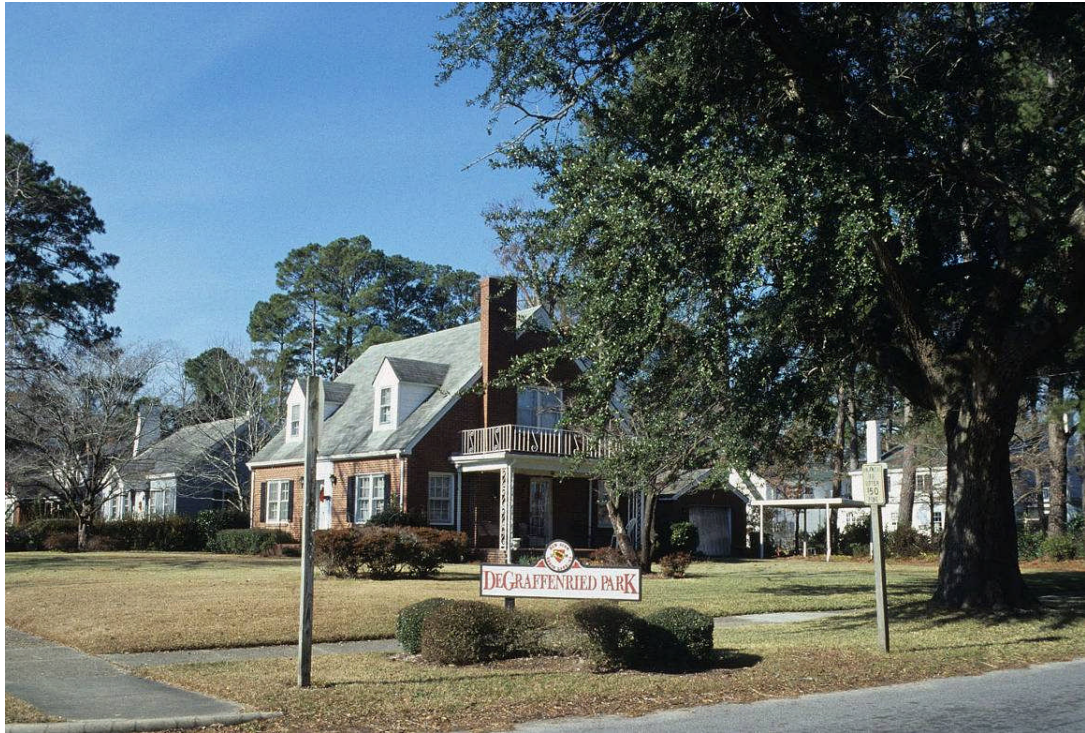
Trent Boulevard, north side, looking northwest
