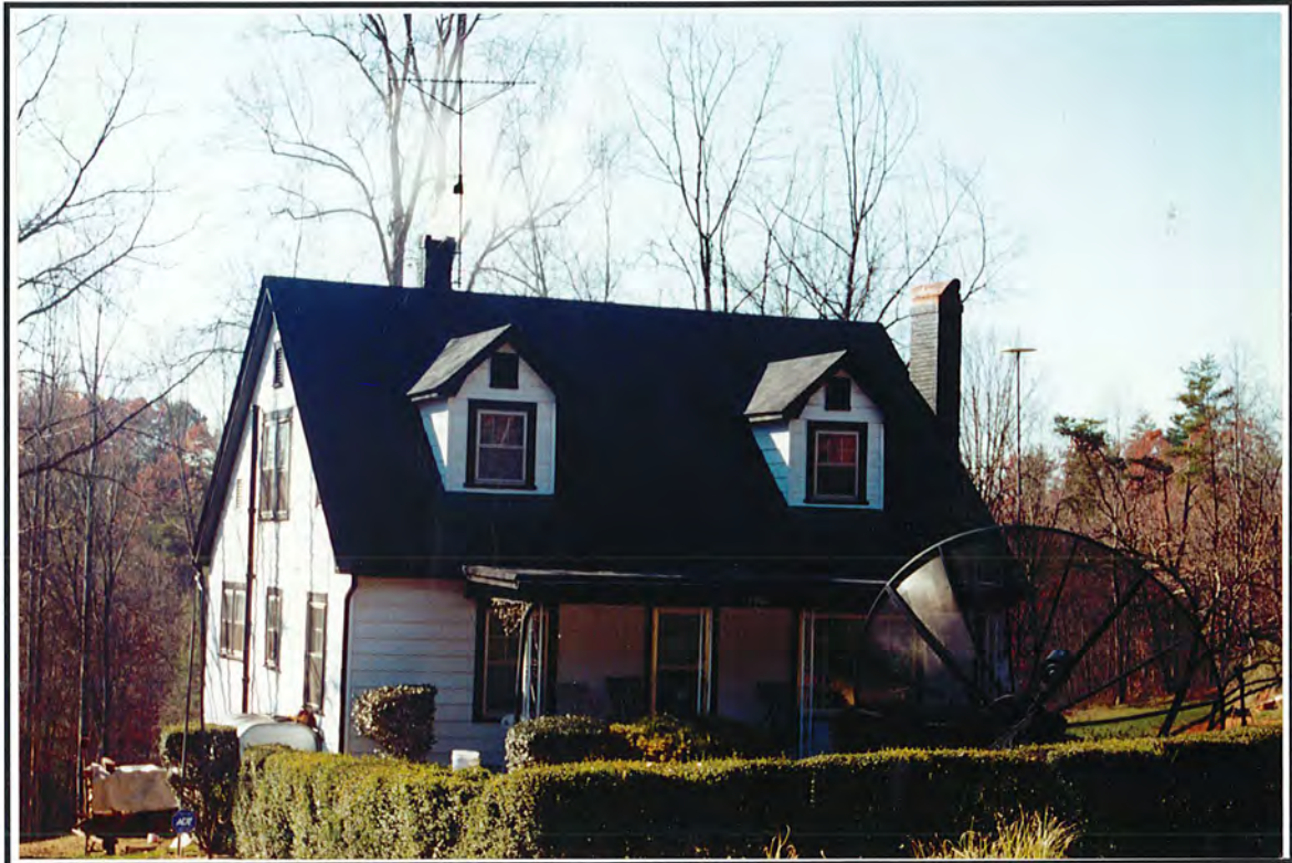
Photograph 138. View of Structure 76, facing southwest.
