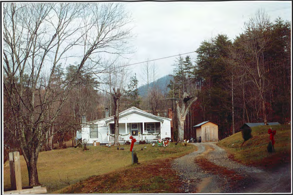
Photograph 91. View of Structure 48, facing northeast.
