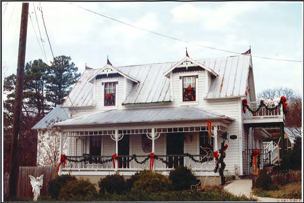
Photograph 49. View of Structure 23, facing northwest.
