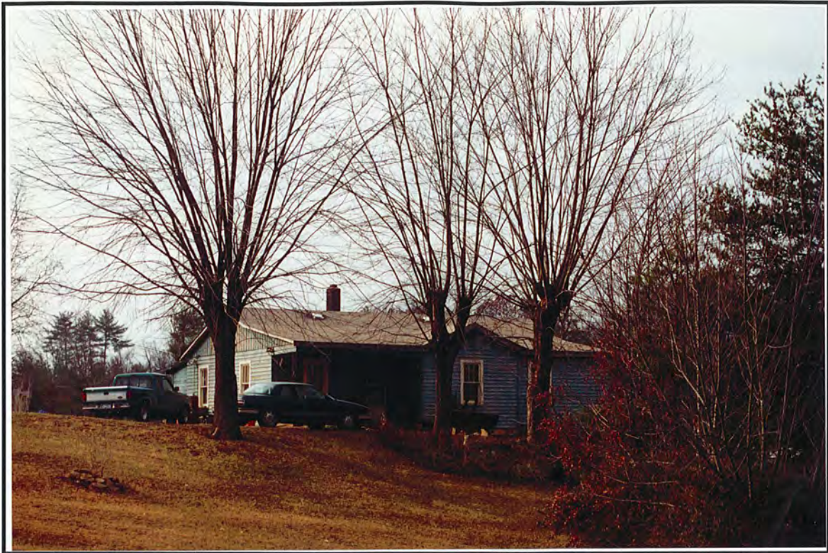
Photograph 89. View of Structure 47, facing northwest.
