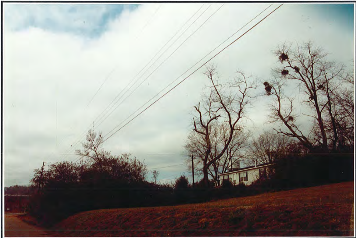
Photograph 44. View from Structure 20, towards proposed tower site, facing northwest.
