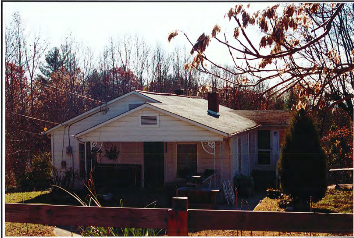
Photograph 146. View of Structure 81, facing south.
