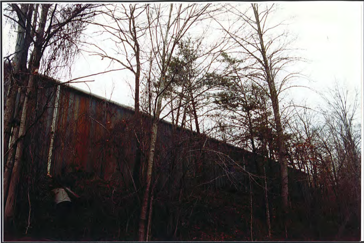
Photograph 111. View from Structure 60, towards proposed tower site, facing west-northwest.
