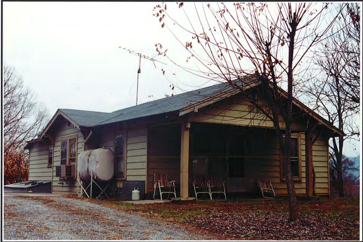
Photograph 30. View of Structure 14, representative of historic structures on Nuway Circle, facing east.
