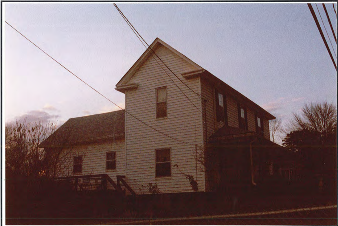
Photograph 96. View of Structure 51, facing northwest.
