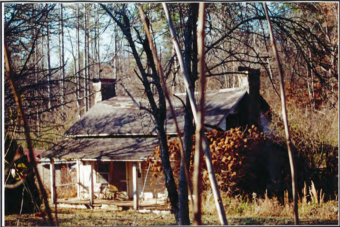
Photograph 125. View of Structure 68, facing southwest.
