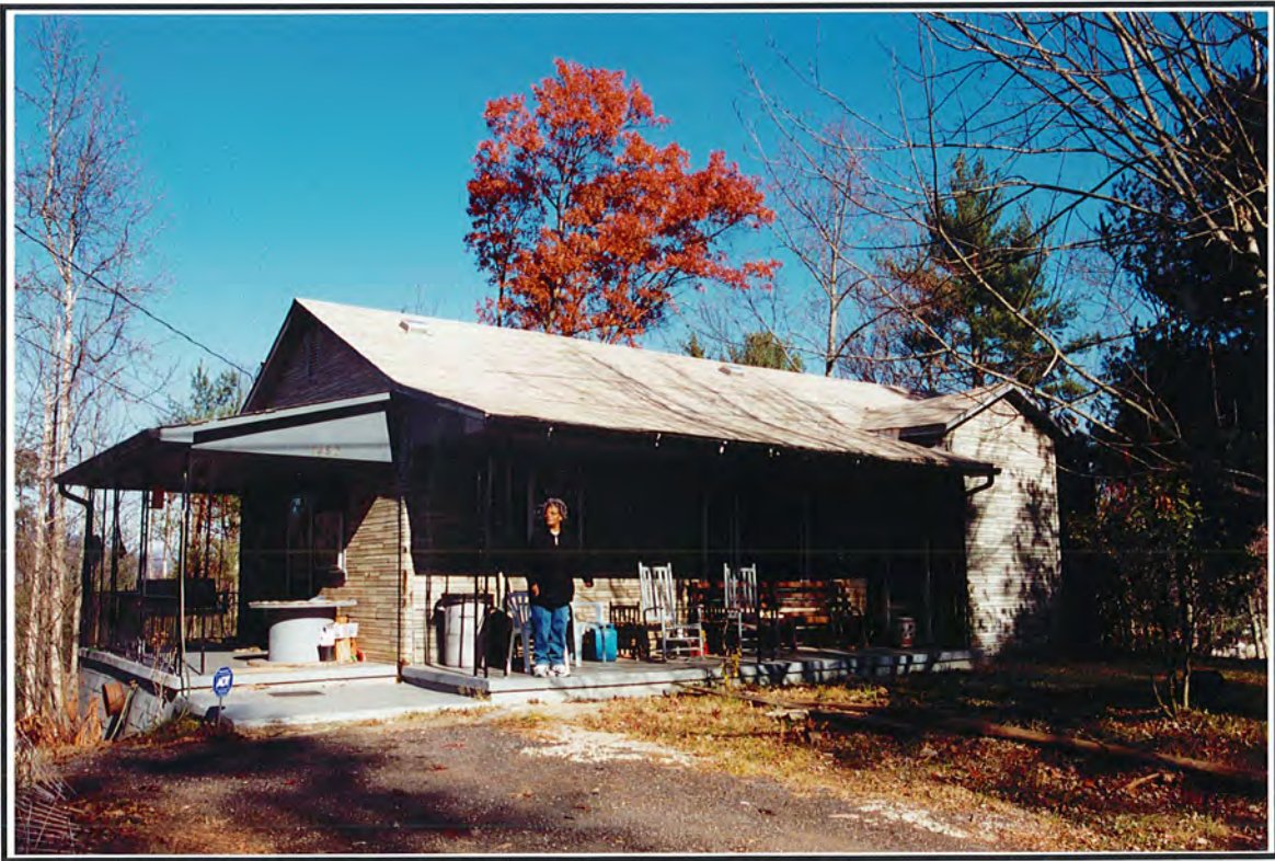
Photograph 140. View of Structure 77, facing north.
