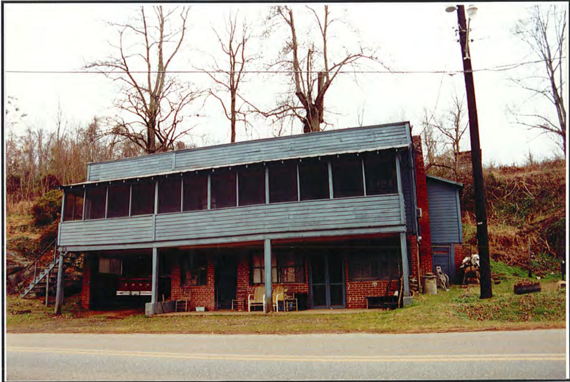
Photograph 92. View of Structure 49, facing southwest.
