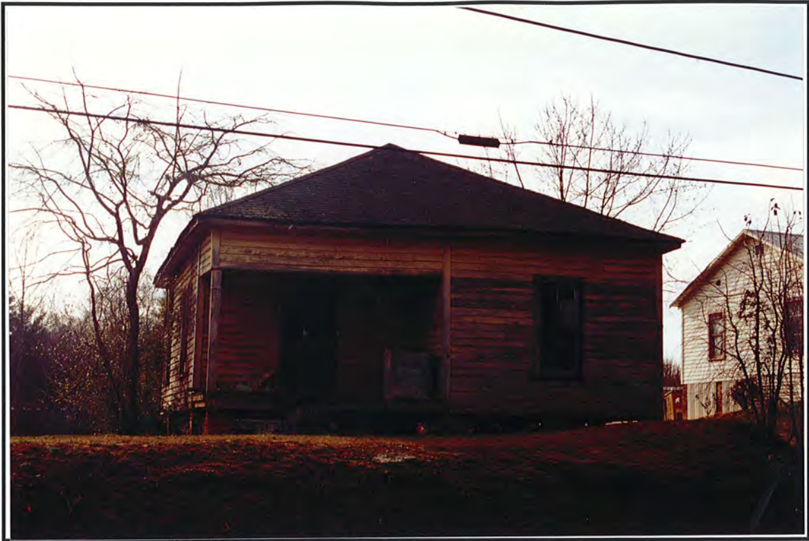
Photograph 99. View of Structure 53, facing southwest.
