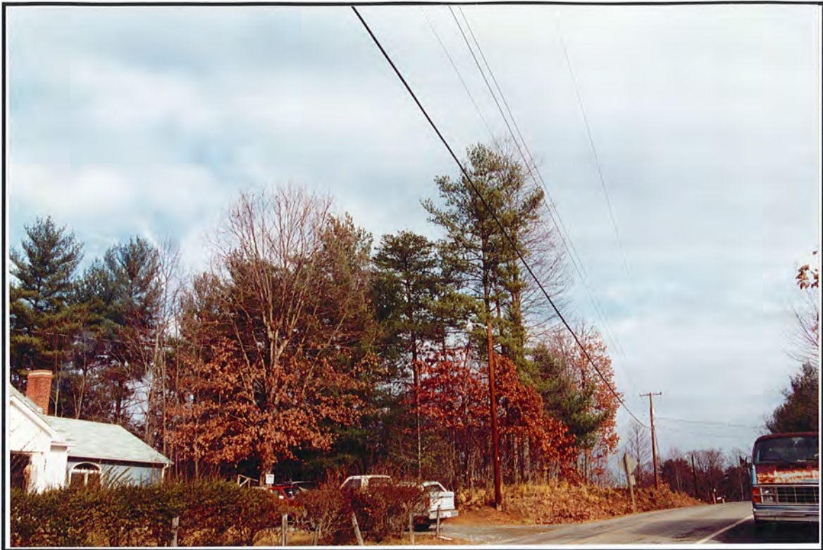
Photograph 145. View from Structures 80 and 81, towards proposed tower site, facing east-northeast.
