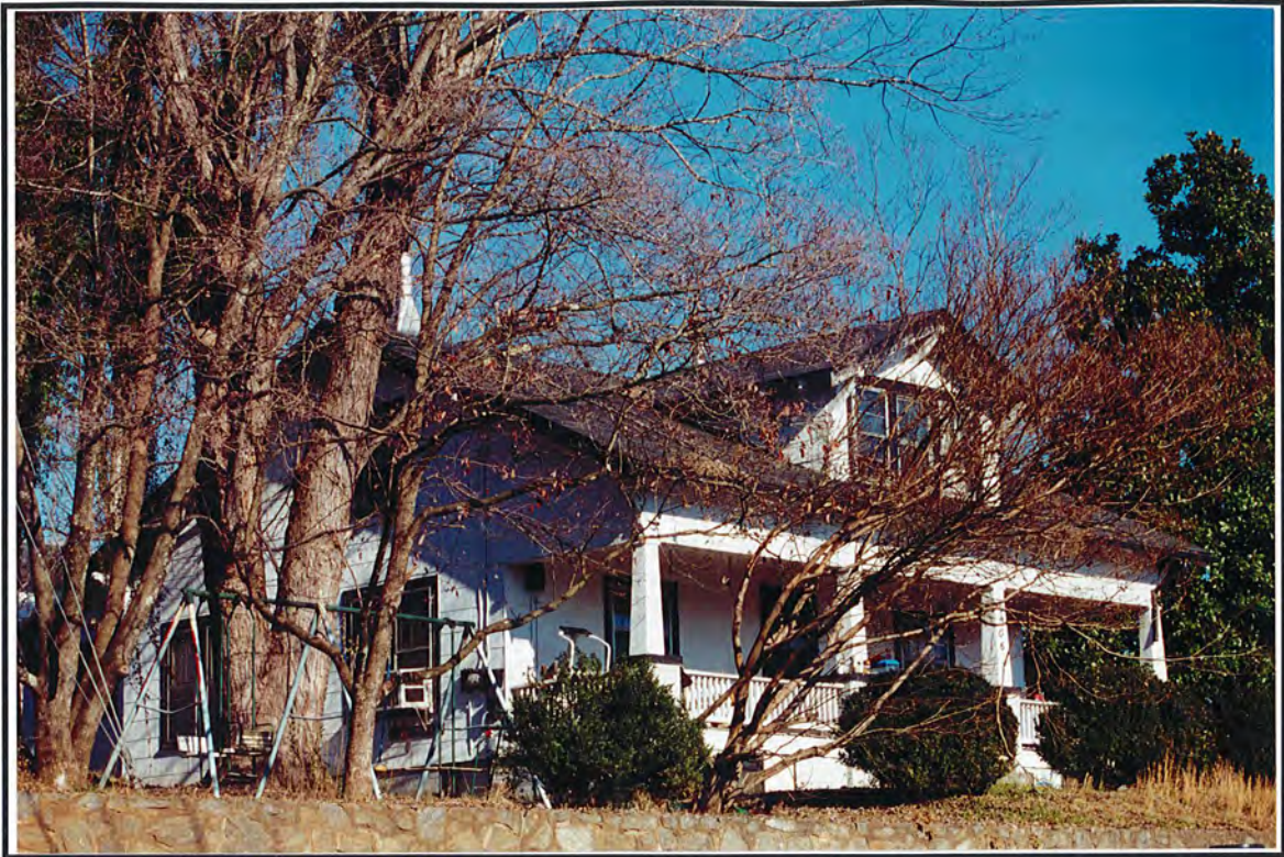
Photograph 131. View of Structure 71, facing north.
