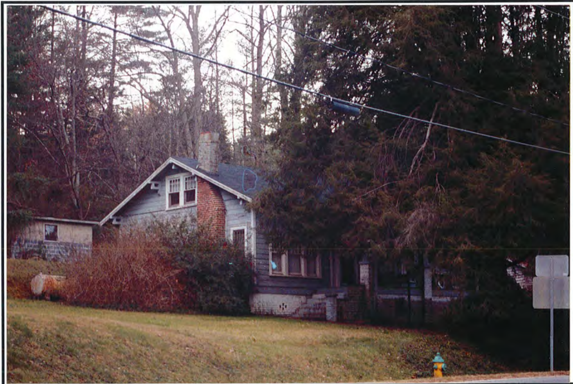
Photograph 84. View of Structure 44, facing northwest.
