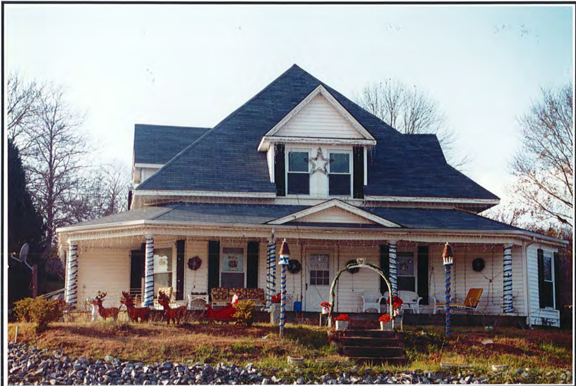
Photograph 54. View of Structure 25, facing west-northwest.
