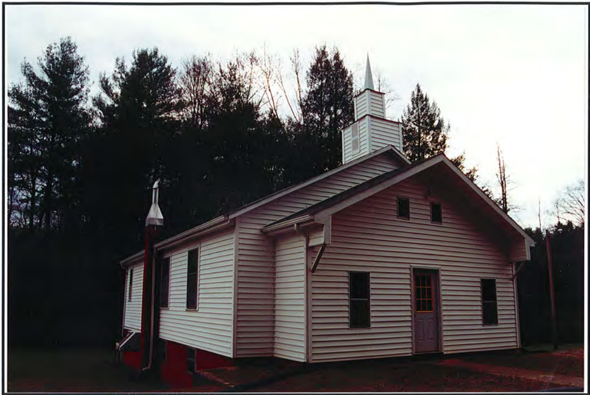
Photograph 9. View of Structure 2, Morning Star Baptist Church, facing southeast.
