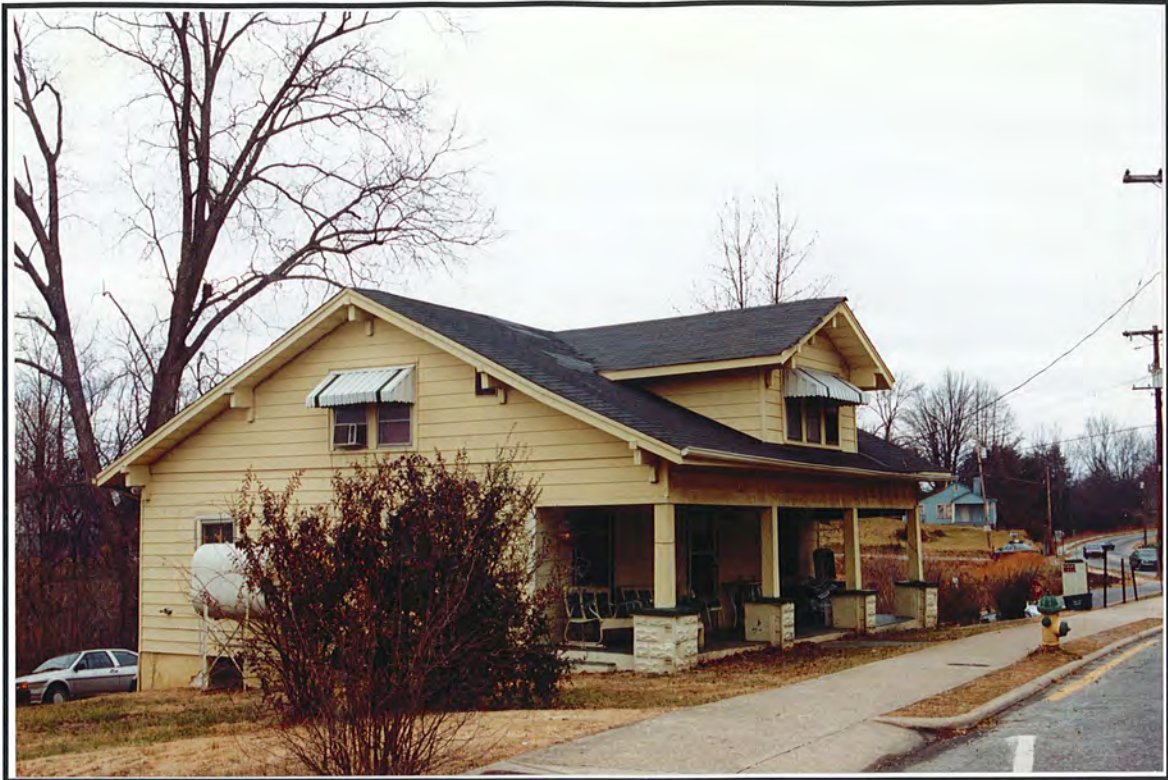
Photograph 119. View of Structure 65, representative of historic structures on Finley Avenue, facing northeast.
