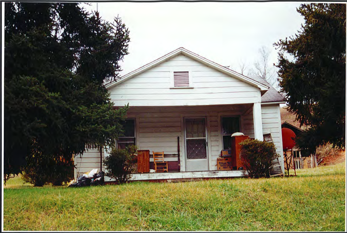
Photograph 11. View of Structure 4, facing west-southwest.
