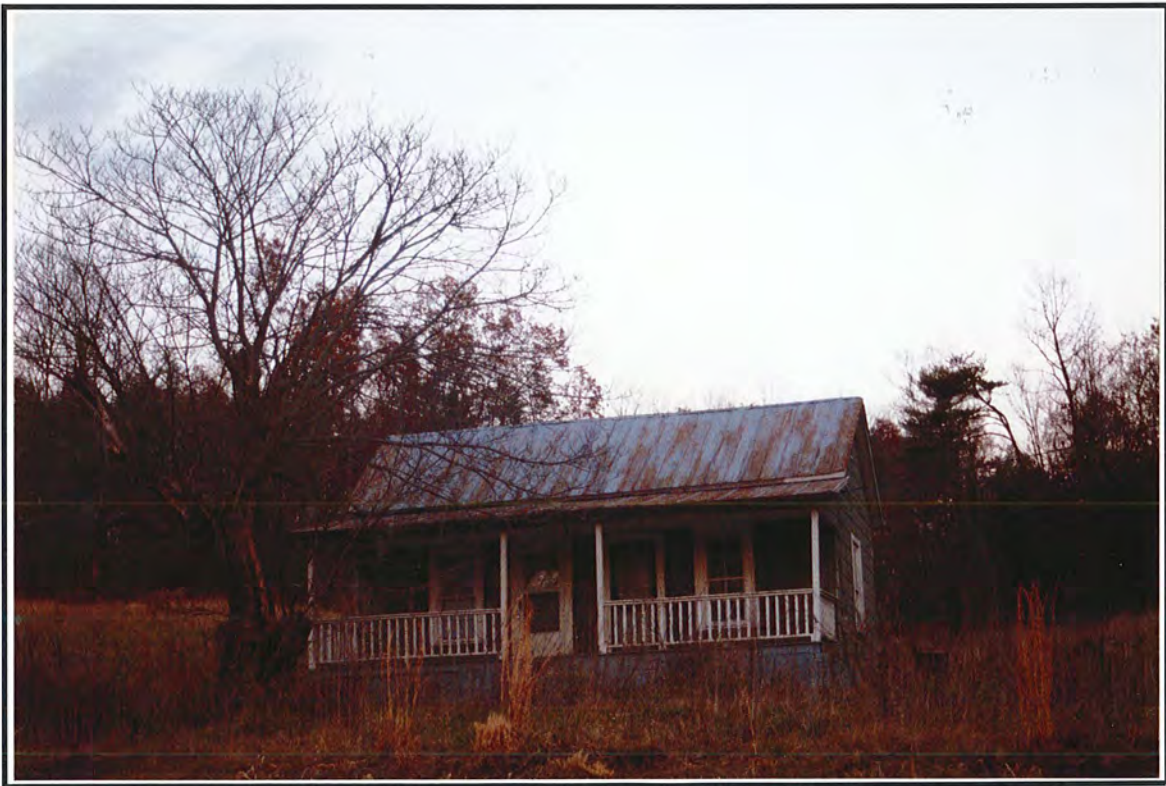
Photograph 104. View of Structure 56, facing northeast.
