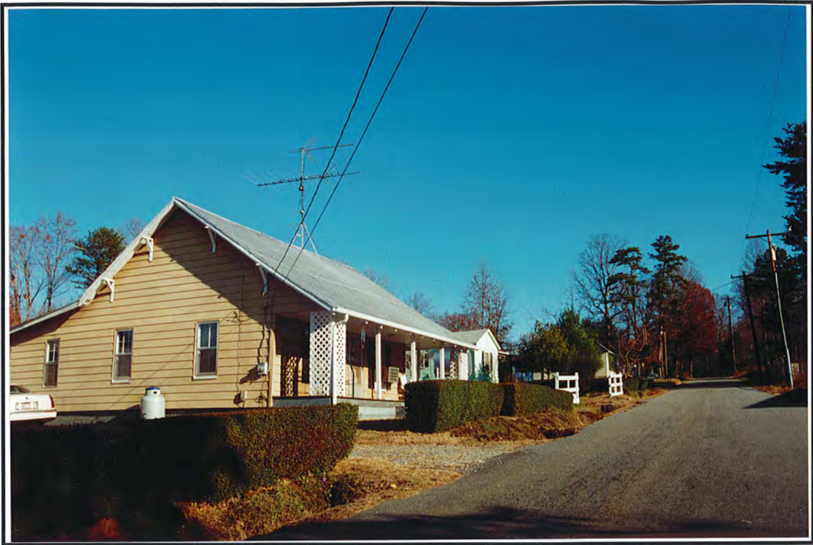
Photograph 121. View of Streetscape 66, representative of historic structures on Merriman Street, facing northwest.
