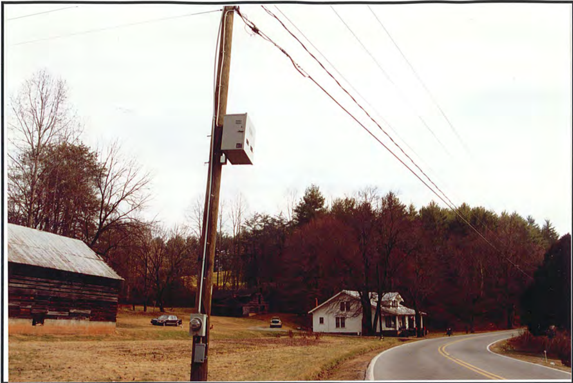
Photograph 87. View from Structures 45 and 46, towards proposed tower site, facing southeast.
