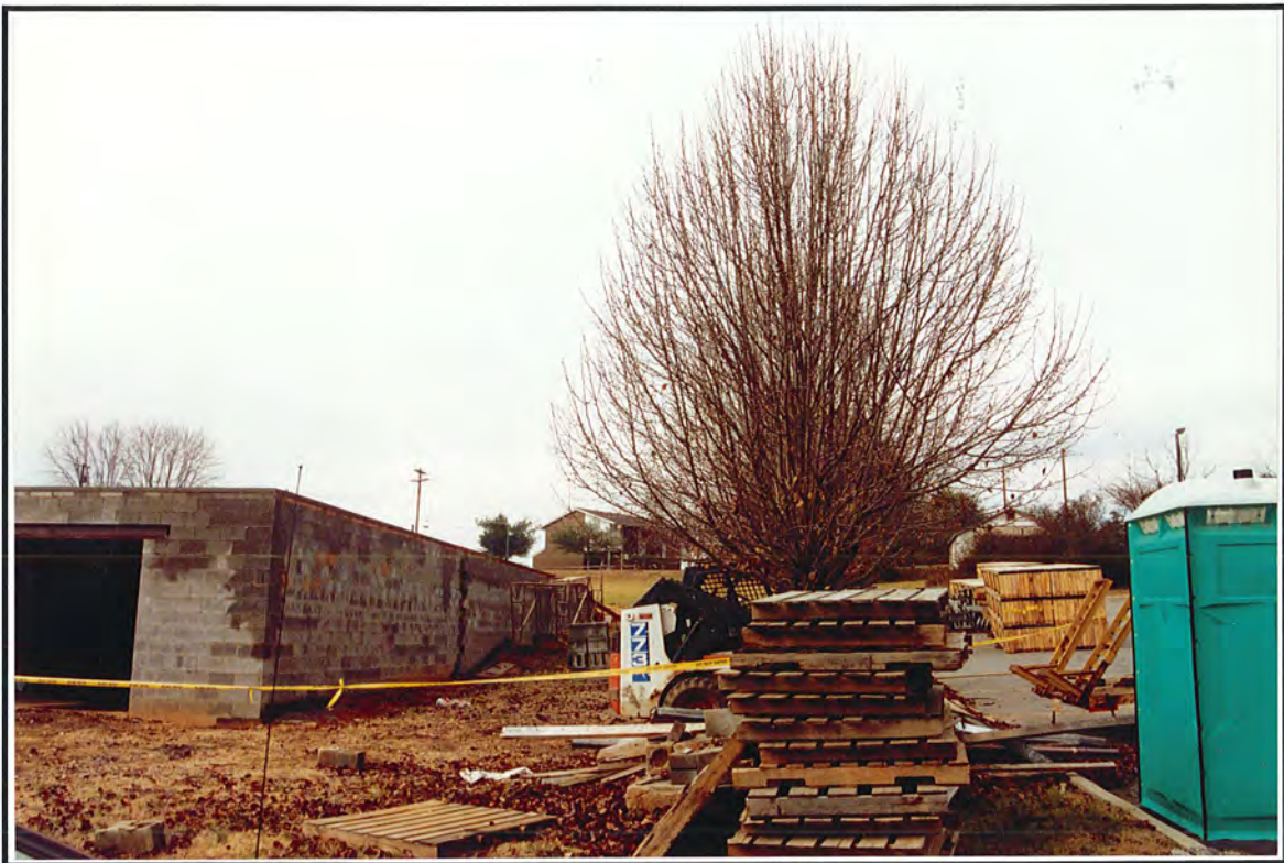
Photograph 40. View from Structure 18, towards proposed tower site, facing northwest.
