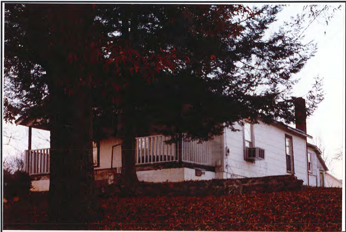
Photograph 98. View of Structure 52, facing northeast.
