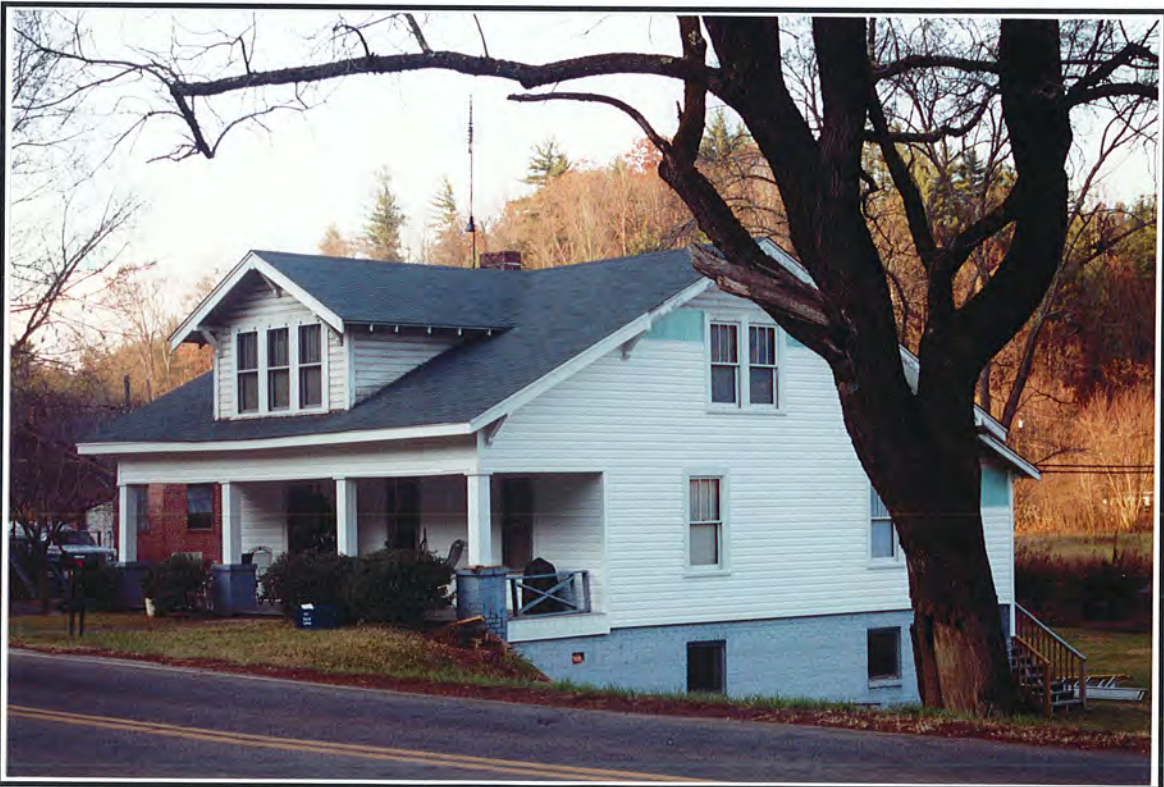
Photograph 80. View of Structure 41, representative of historic structures on Highway 90, facing north.
