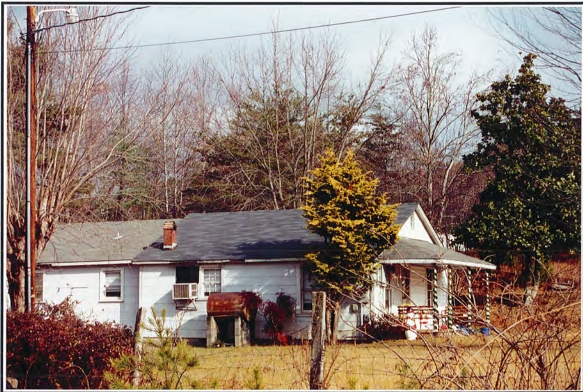
Photograph 76. View of Structure 39, facing northeast.
