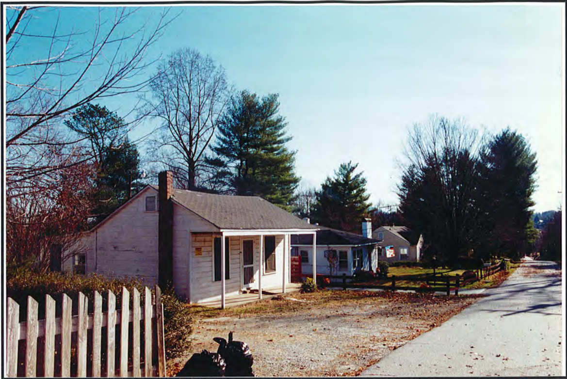
Photograph 137. View of Streetscape 75, representative of historic structures on Plaza Street, facing east.
