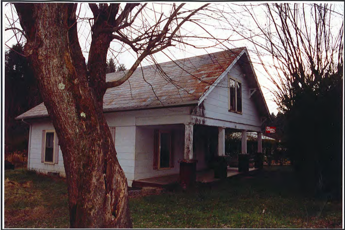
Photograph 15. View of Structure 6, facing south.
