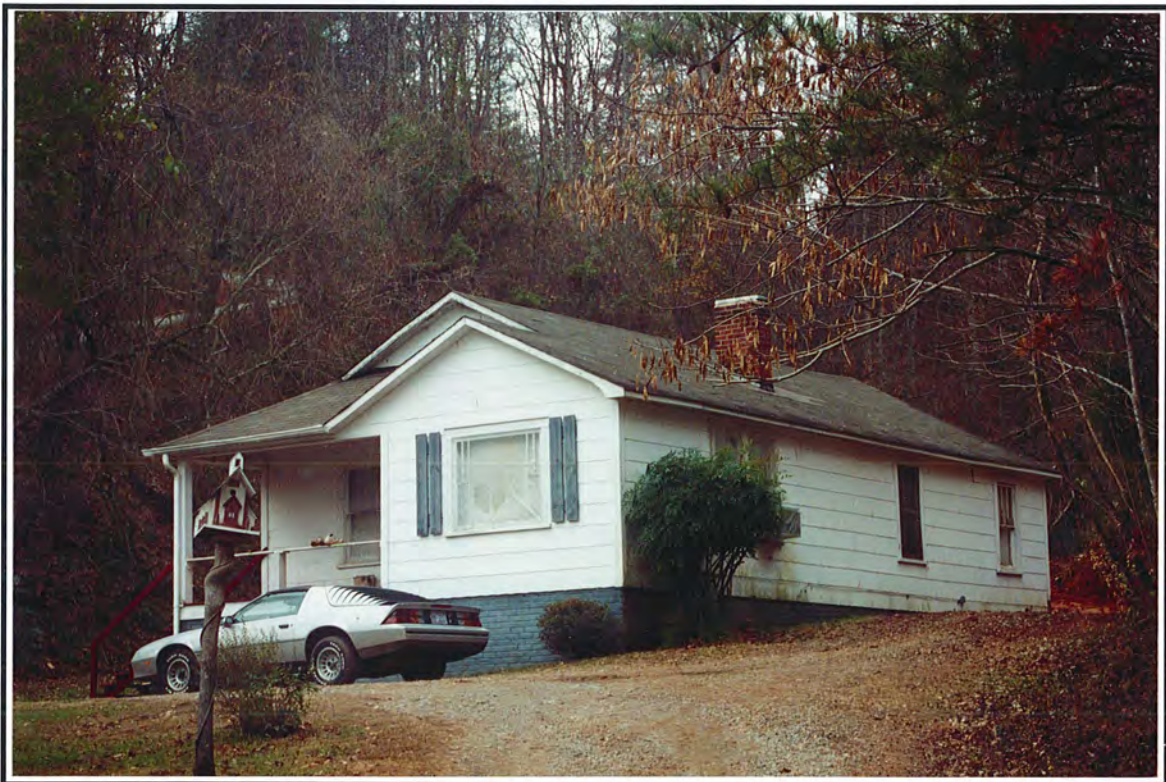
Photograph 10. View of Structure 3, facing south-southwest.
