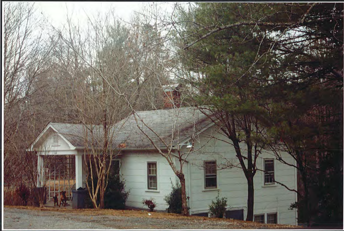
Photograph 110. View of Structure 60, facing northeast.
