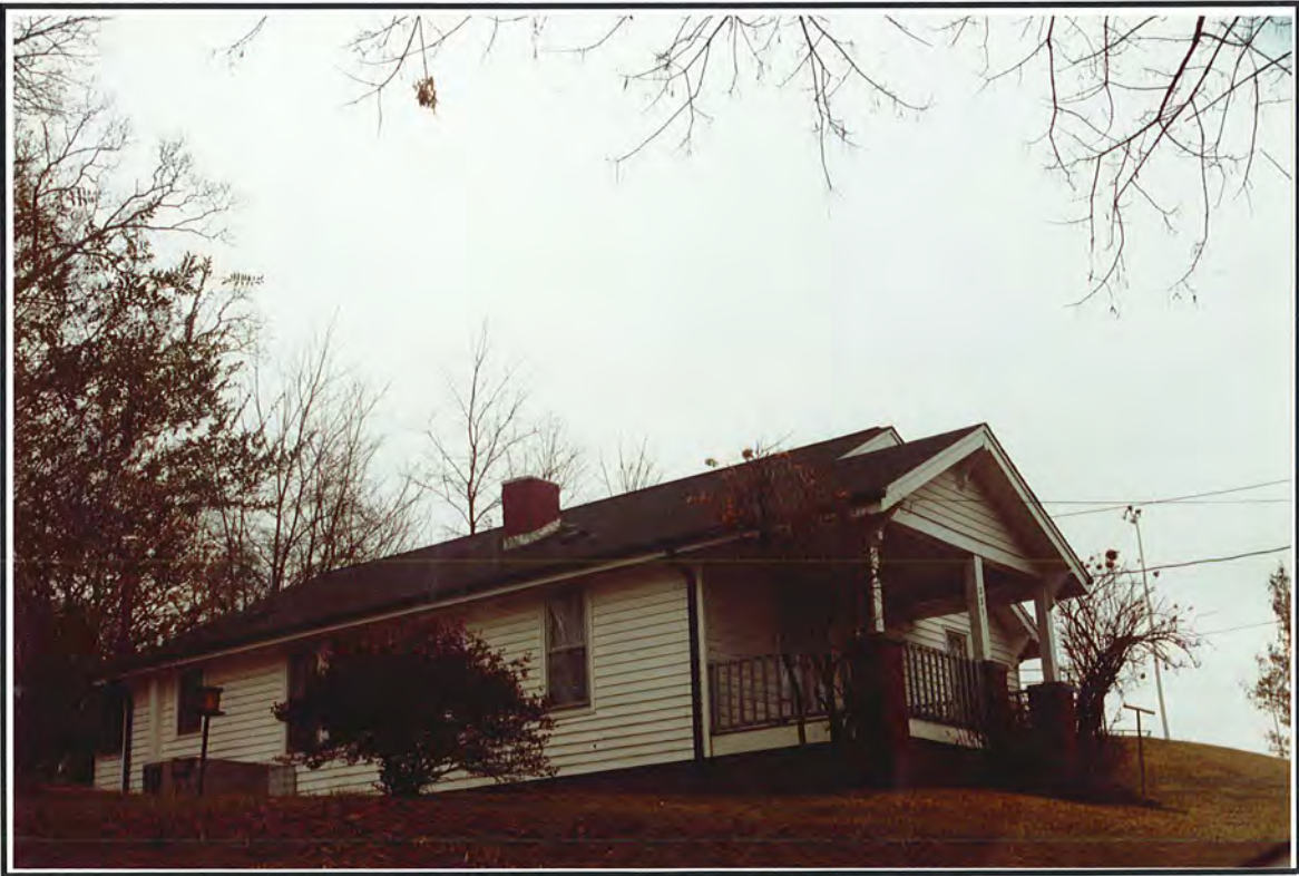
Photograph 116. View of Structure 63, representative of historic structures on Greenhaven Drive, facing southeast.
