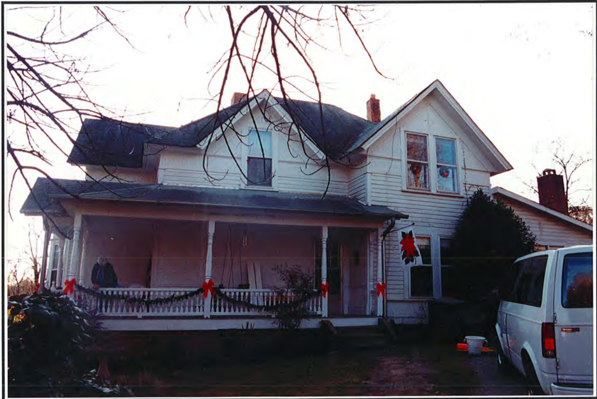
Photograph 64. View of Structure 31, facing southwest.
