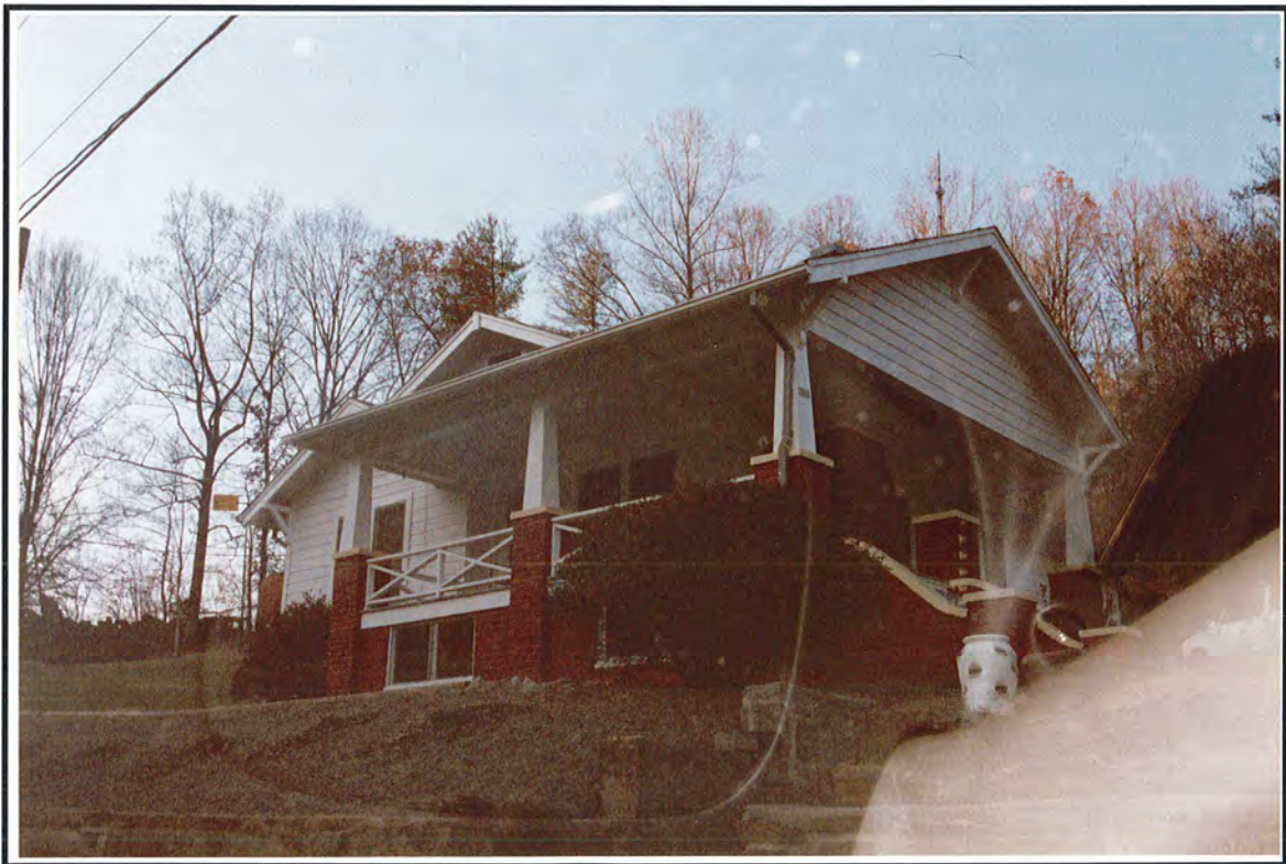
Photograph 88. View of Structure 46, facing north.
