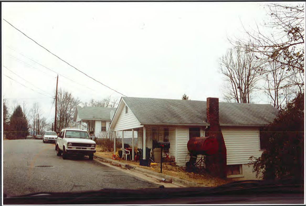
Photograph 112. View of Streetscape 61, representative of structures on Holloway Road, facing northeast.
