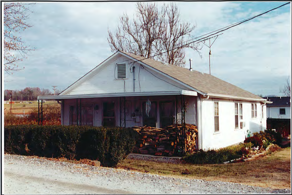
Photograph 39. View of Structure 18, representative of historic structures on Calvary Place, facing east.
