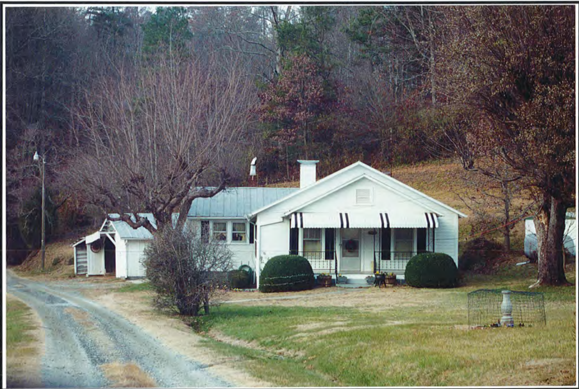
Photograph 22. View of Structure 10, facing north-northwest.
