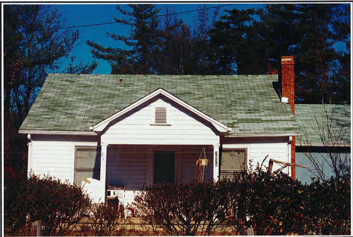
Photograph 144. View of Structure 80, facing north.
