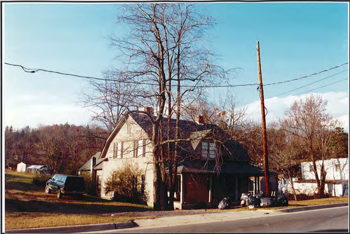
Photograph 59. View of Structure 28, facing north.
