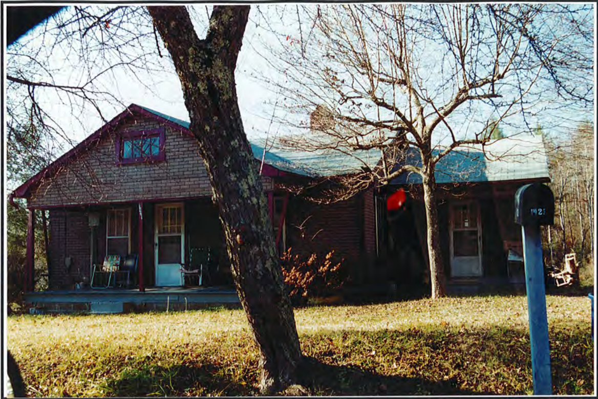
Photograph 127. View of Structure 69, facing southwest.
