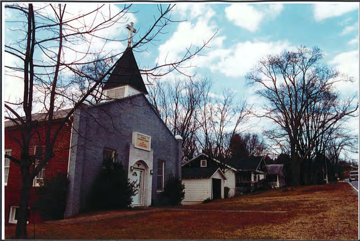
Photograph 47. View of Streetscape 22, representative of structures on Elizabeth Street, facing north.
