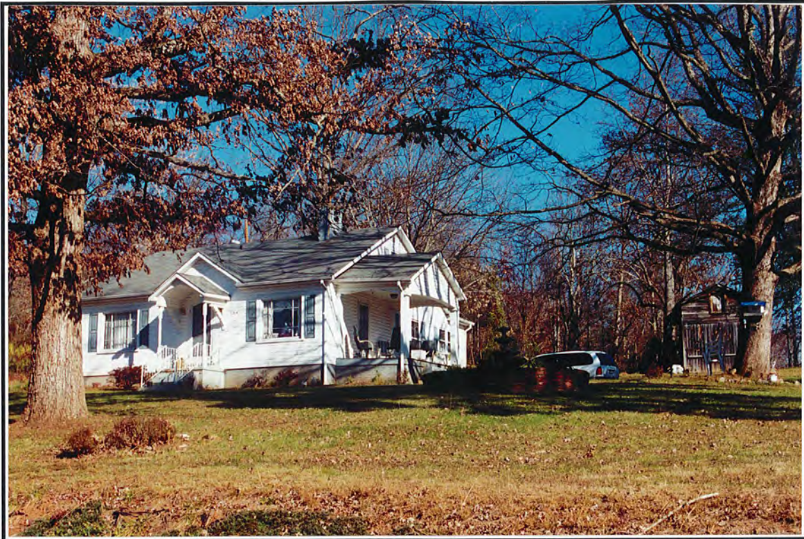
Photograph 105. View of Structure 57, facing north.
