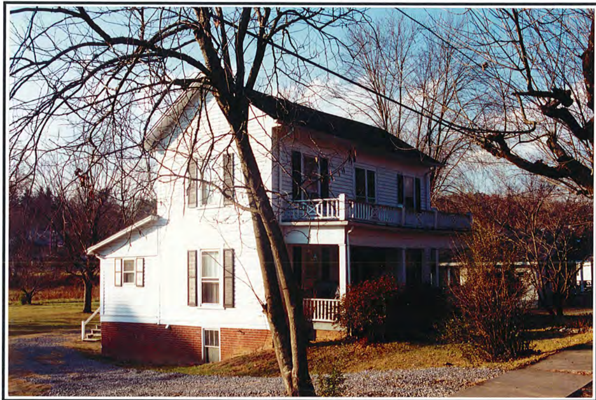
Photograph 66. View of Structure 32, facing northwest.
