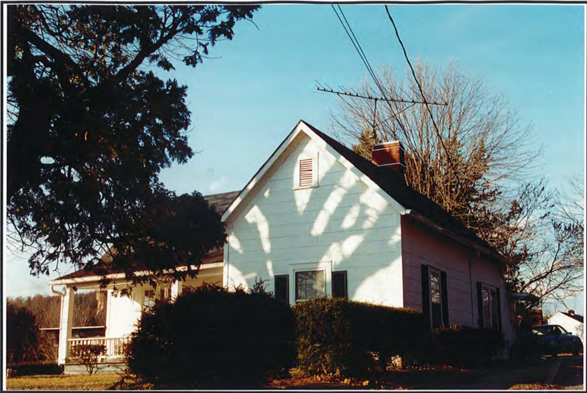
Photograph 69. View of Structure 34, facing north.
