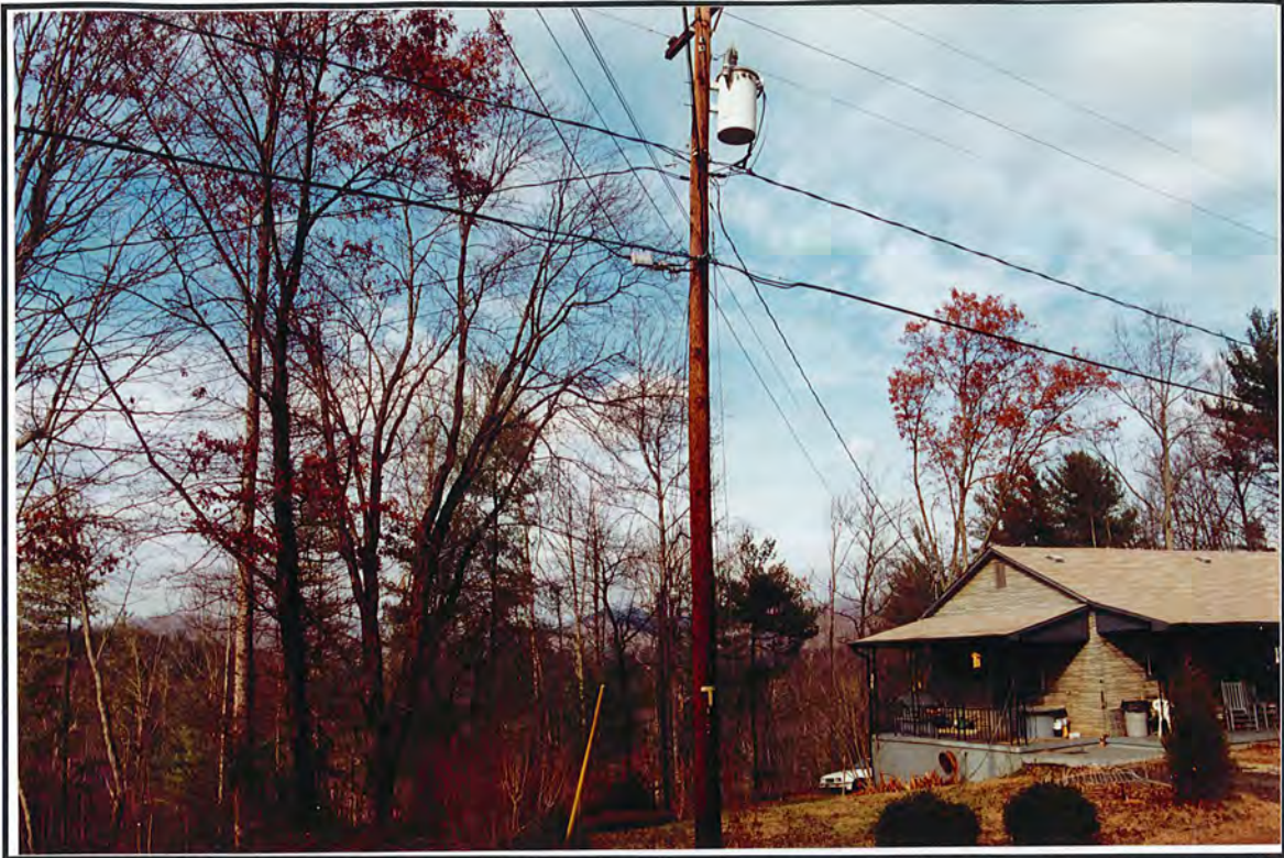
Photograph 141. View from Structures 77, 78, and 79, towards proposed tower site, facing east-northeast.
