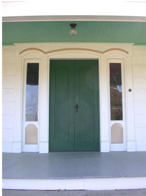
Front entrance detail
