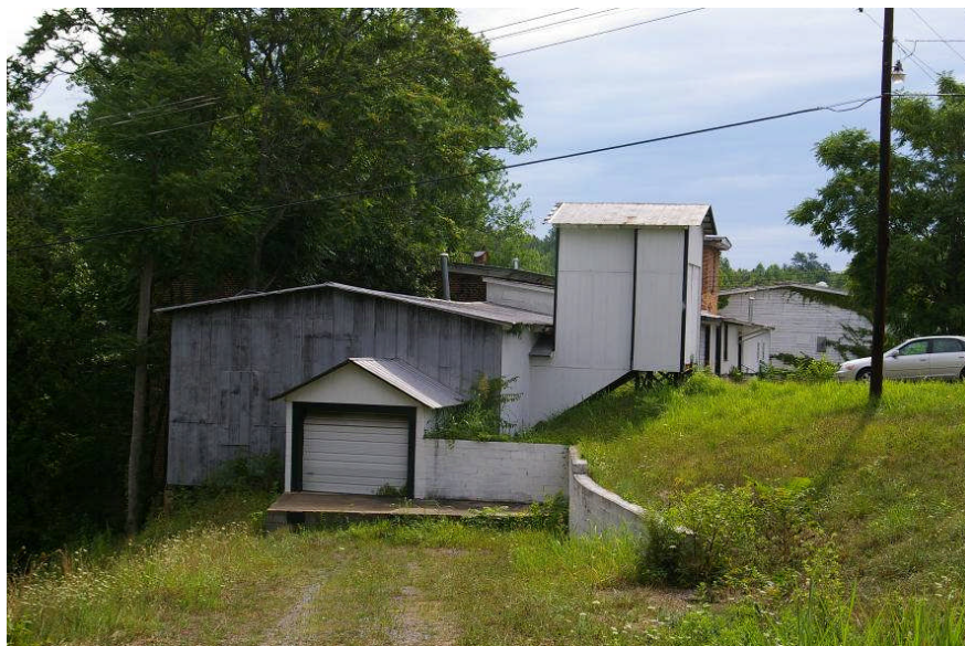
Overall view from the west
