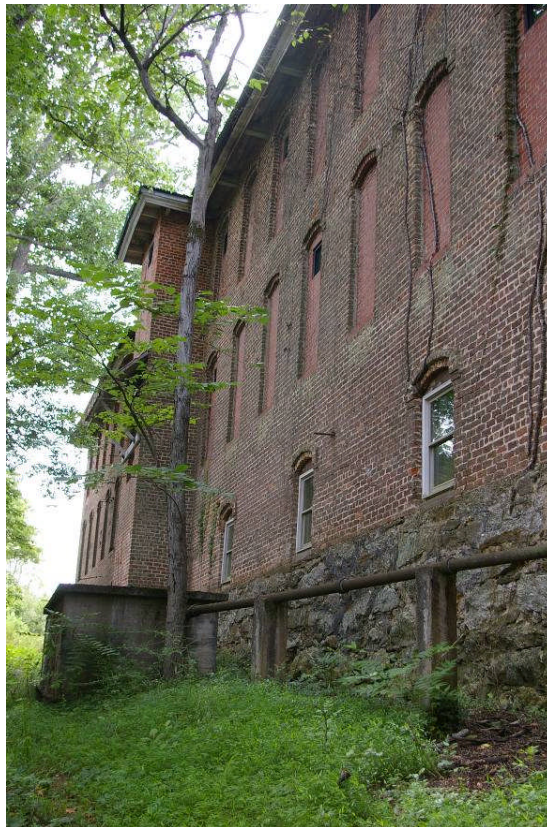
North elevation, facing the river
