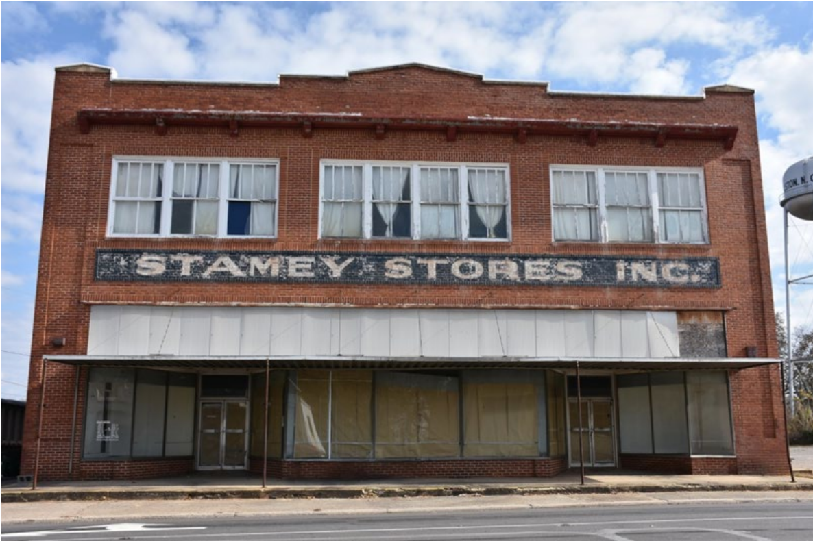
Front façade (west elevation), facing east
