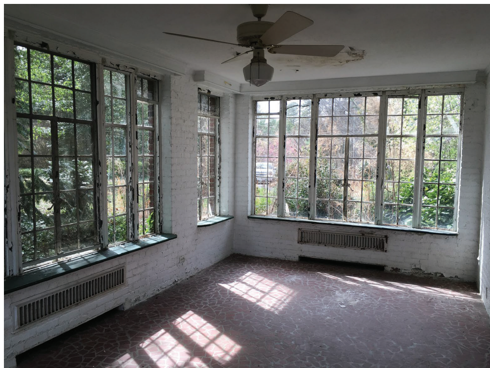
Sun parlor interior, looking West
