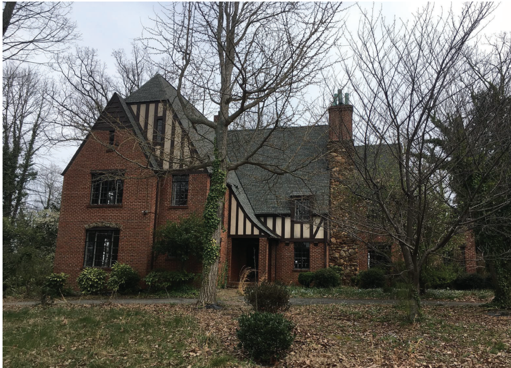
Front Façade (West elevation), looking East
