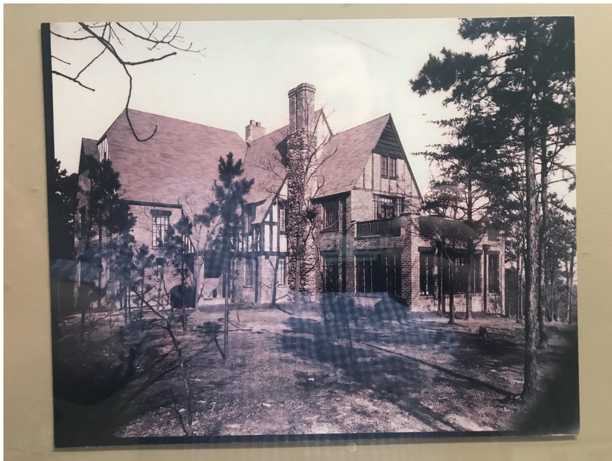
Figure 1. Circa 1928 View of House Looking Northeast 3
