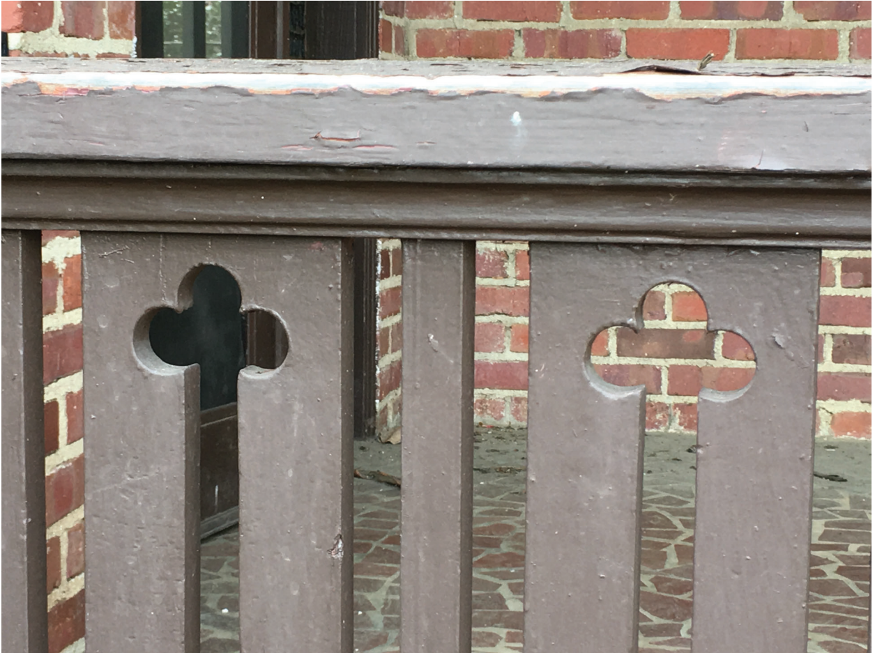
#9. Wood Trefoil Cutouts on Terrace Railing
