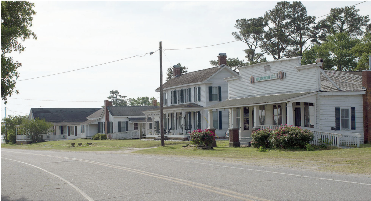
Wilson Walker House and Walker-Snowden Store, looking southwest
