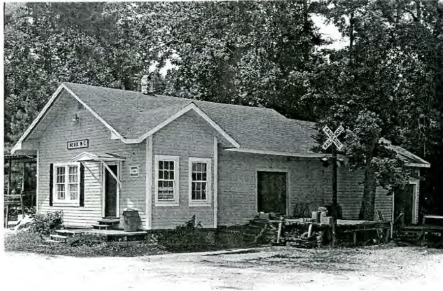
Plate 75. Neuse Railroad Station, Looking North.
