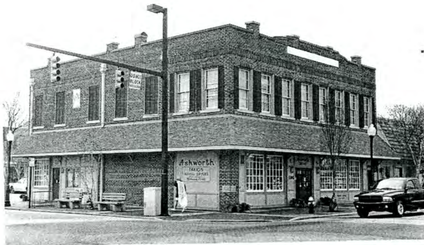
Plate 40. Masonic Hall/Ashworth Drug Store, Front and East Elevations.
