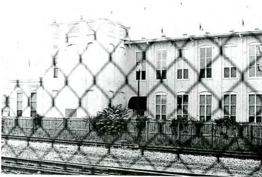
Plate 66. Raleigh Cotton Mill, Looking West.
