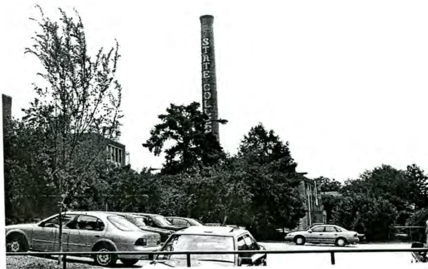
Plate 50. N.C. State University Campus Historic District, Yarborough Heating Plant.
