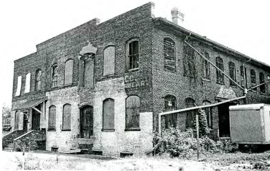
Plate 63. Melrose Knitting Mill, Front Facade.
