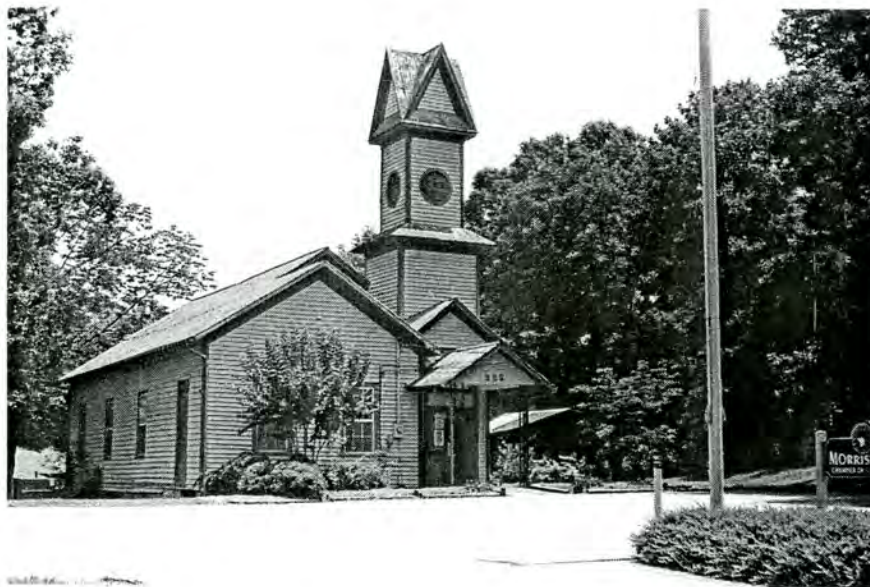
Plate 27. (Former) Morrisville Christian Church, Front Facade.
