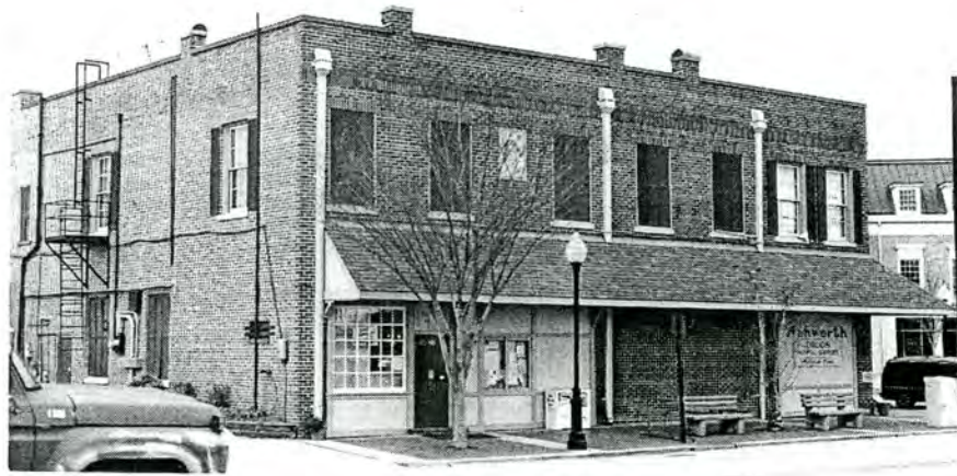
Plate 41. Masonic Hall/Ashworth Drug Store, East and Rear Elevations.
