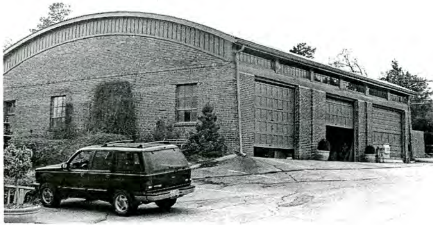
Plate 69. Gulf Petroleum Products Warehouse, Looking South.
