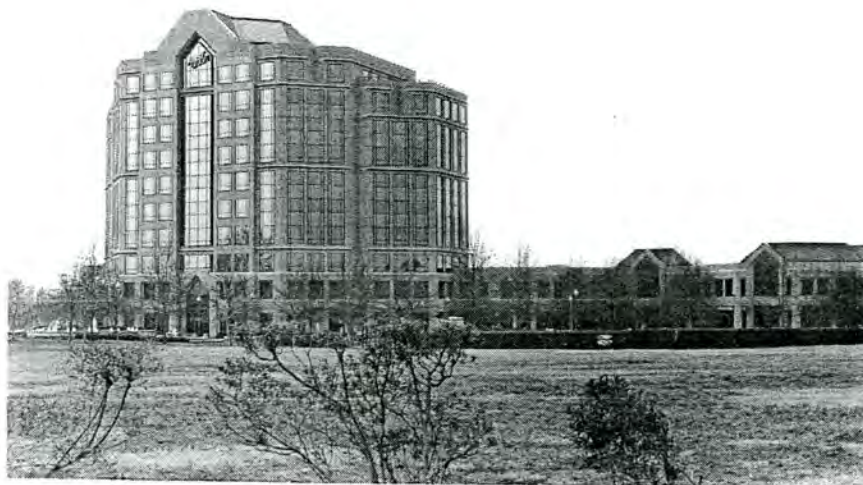
Plate 2. West Durham Historic District, Erwin Square Complex.
