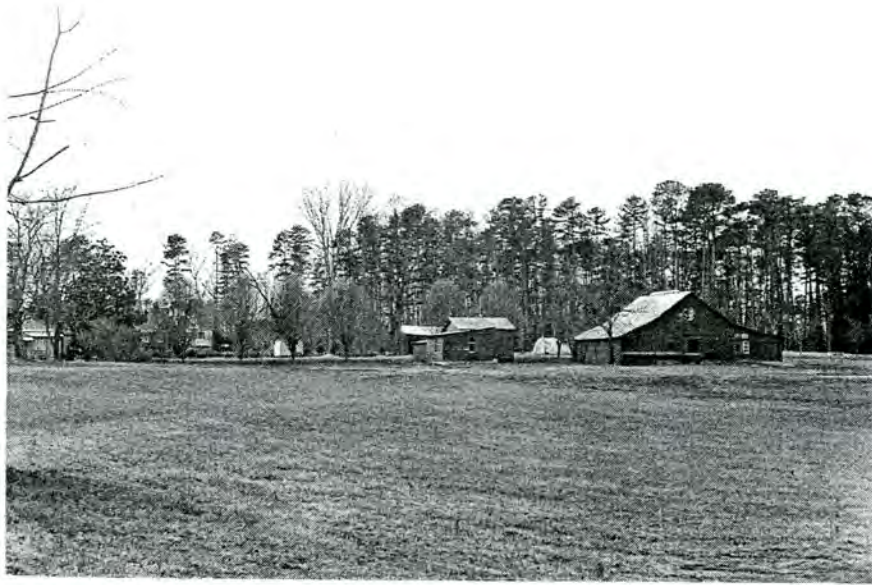
Plate 73. Norwood House Tract, Outbuildings Looking North.
