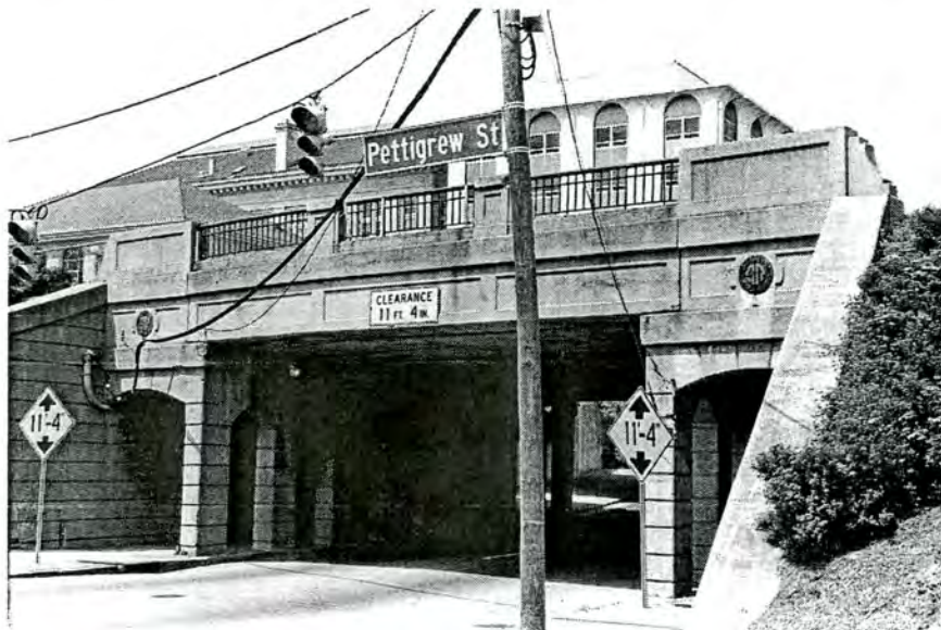
Plate 18. Southern Railway Bridge, Looking South.
