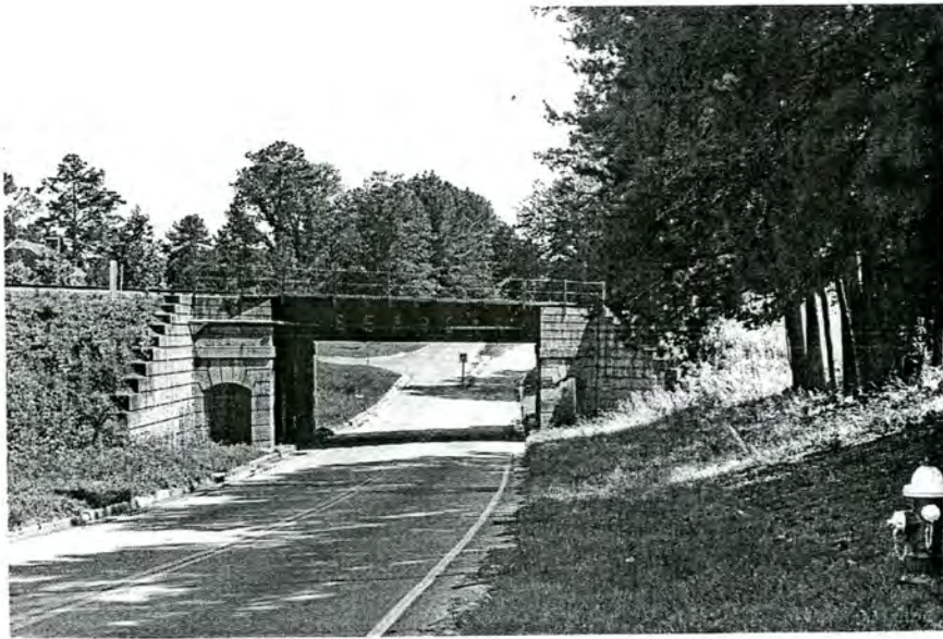
Plate 46. Seaboard Airline Railway Bridge, Looking West.
