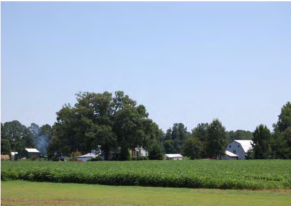
Plate 52. Bell-Pierce Farm, Eastern Tract, Overall View of Farm Complex, Looking Southeast from Ten Ten Road.
