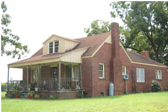
No. 69 House (No PIN), 3908 Benson Road, Garner Vicinity, Wake County
