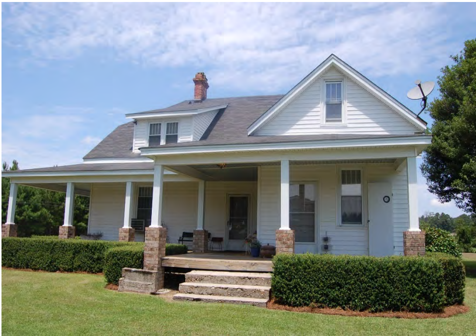
Plate 462. Bryan Farms Historic District, George W. and Julia Bryan Farm (No. 247), House, Side (South) Elevation, Looking North.
