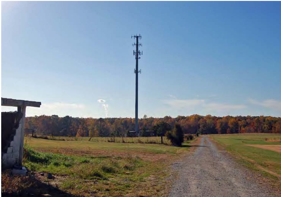
Plate 36. Pierce Farm, Cell Tower and Farmland West of Farm Complex, Looking West.
