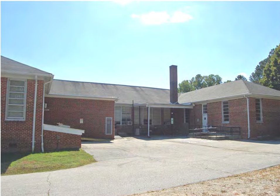
Plate 289. Mount Auburn School, Rear (North) Elevation, Looking South.
