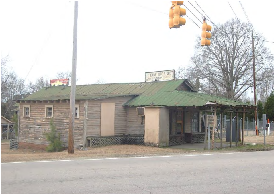
Plate 571. Thomas Store, Front (Northeast) and Side (Southeast) Elevations, Looking West.
