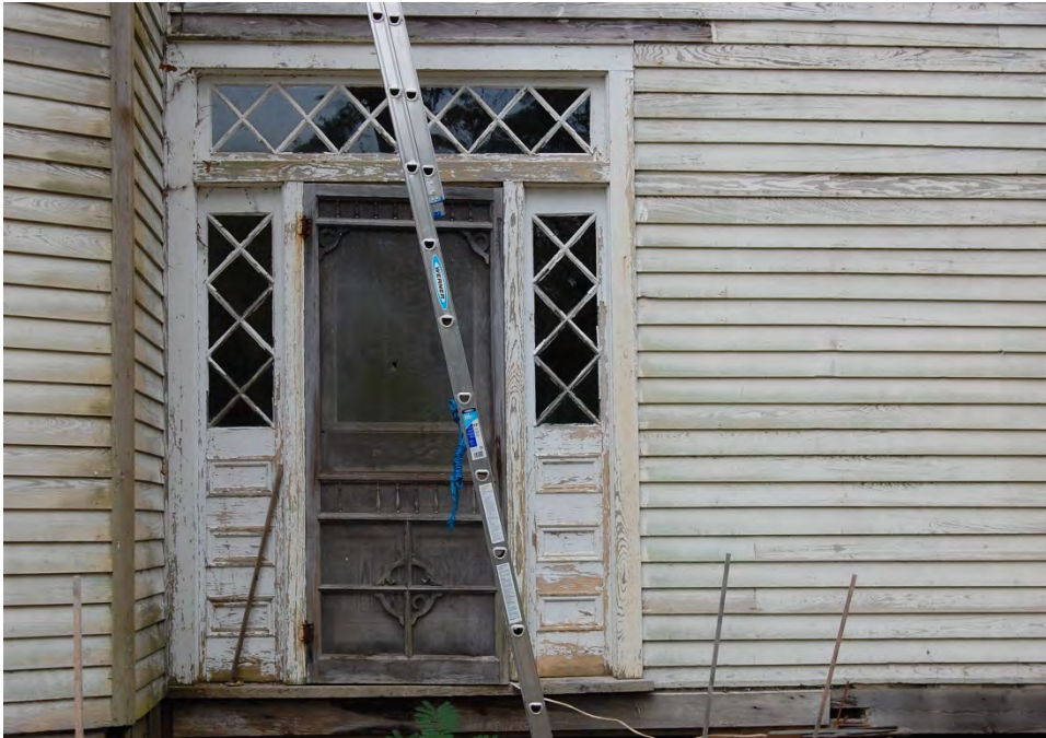
Plate 596. Atkinson-Whitted House, Main Entrance, Looking West.
