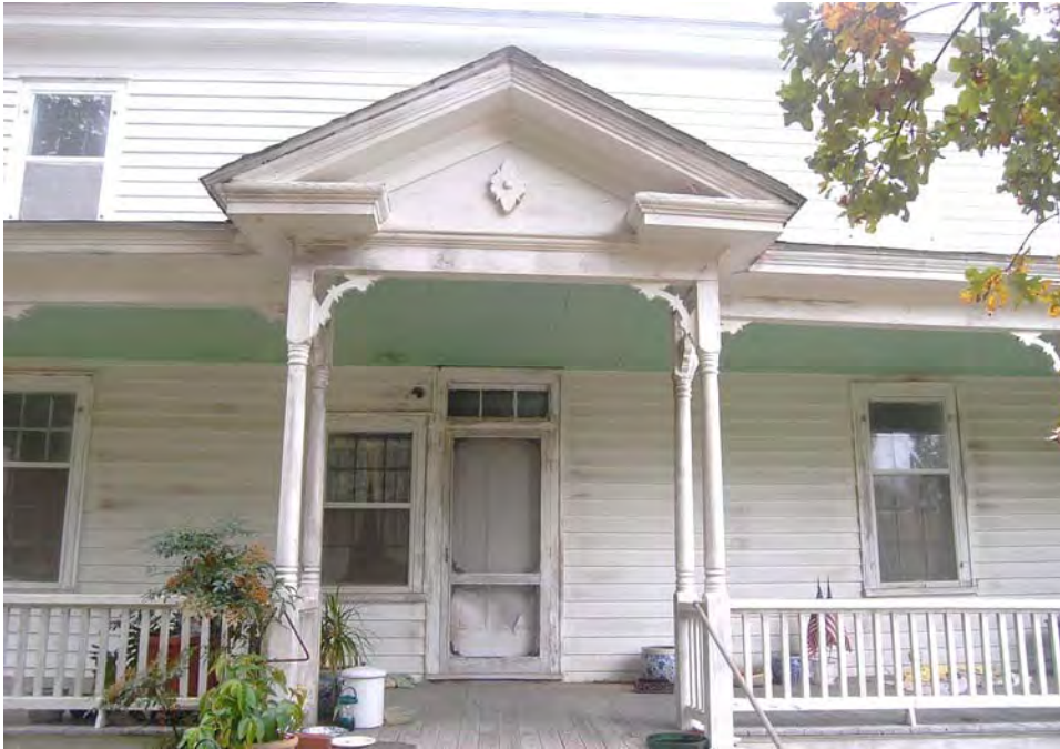
Plate 337. Baucom-Stallings House, Main Entrance, Looking North.
