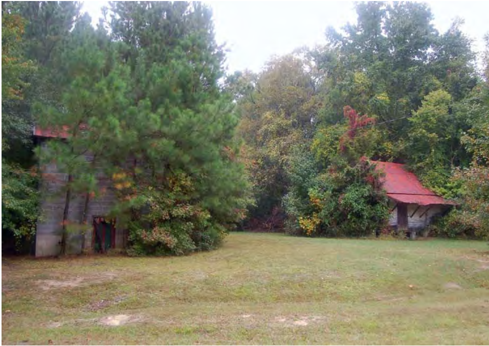
Plate 352. The Oaks, Tobacco Barn and Former Tenant House/Grading Room, Looking North.
