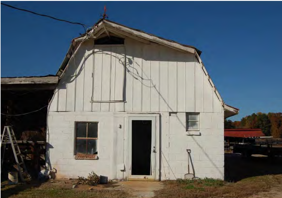
Plate 30. Pierce Farm, Dairy Barn, Looking North.
