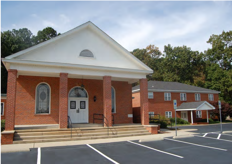
Plate 436. New Bethel Baptist Church, 1931 Church and 1954 Classroom and Fellowship Hall Building, Looking West.
