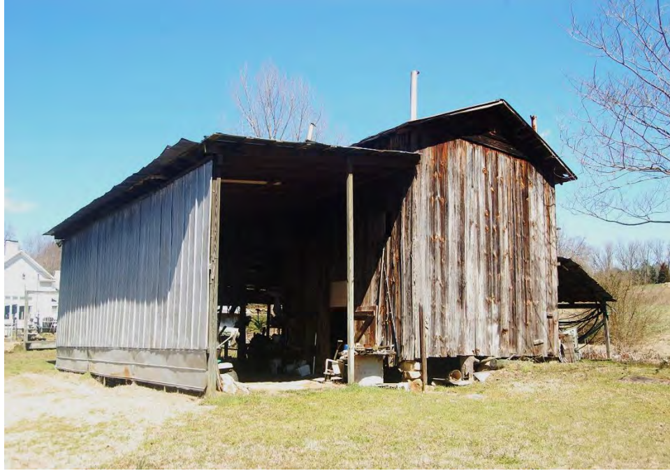
Plate 666. Jim Jordan Farm Complex, Tobacco Barn/Equipment Shed, Looking North.
