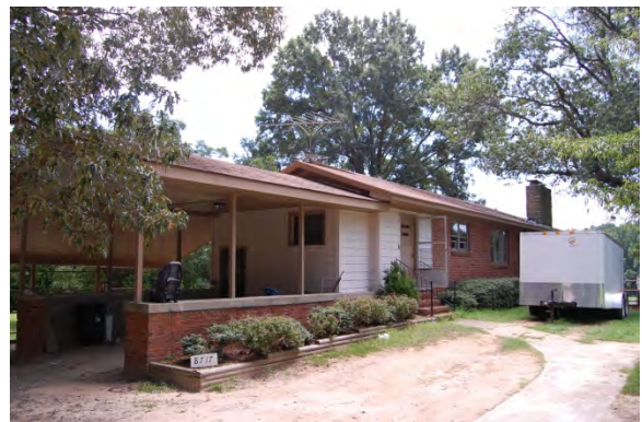
No. 11 House (PIN 0760524264), 8717 Pierce Olive Road, Holly Springs Vicinity, Wake County
