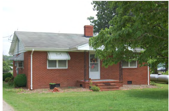
Nos. 39-40 Russell-McGee Complex (WA2450) (PINs 0699805778 and 0699804698), 9317-9321 Old Stage Road, Williams Crossroads Vicinity, Wake County
