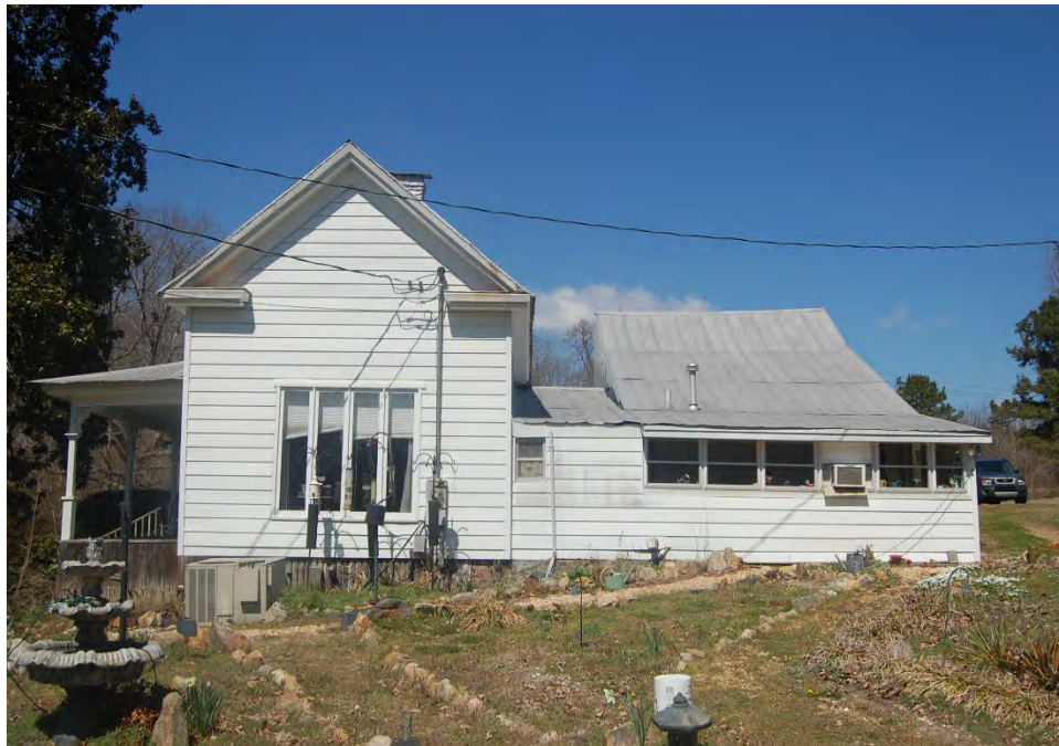
Plate 663. Jim Jordan Farm Complex, House, Side (South) Elevation, Looking North.
