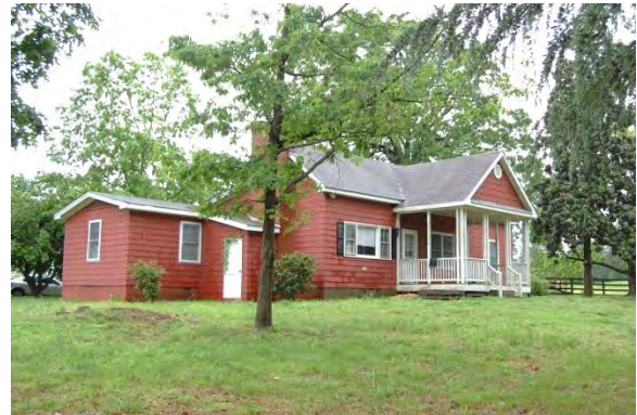
No. 138 House (PIN 1741315557), 2609 Branch Road, Garner Vicinity, Wake County
