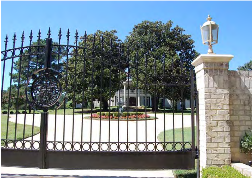
Plate 224. Ransom Penny House, Front Gate, Looking West.
