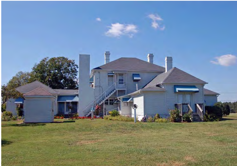
Plate 245. Richard Burnette House, Rear (East) Elevation, Looking West.
