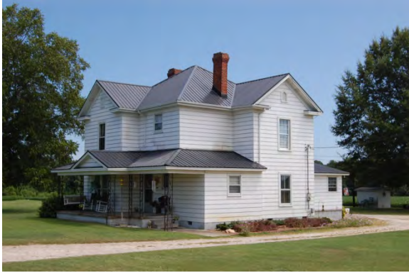
No. 20 Lee-Ennis House (WA1244) (PIN 0689187150), 3901 Johnson Pond Road, Apex Vicinity, Wake County
