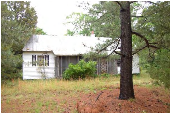
No. 145 House (PIN 1740596158), 7728 Old Baucom Road, Garner Vicinity, Wake County
