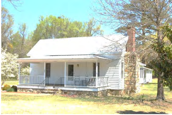
No. 100 William Henry Coats House (WA0291), (PIN 1649289640), 4420 Guy Road, Garner Vicinity, Wake County
