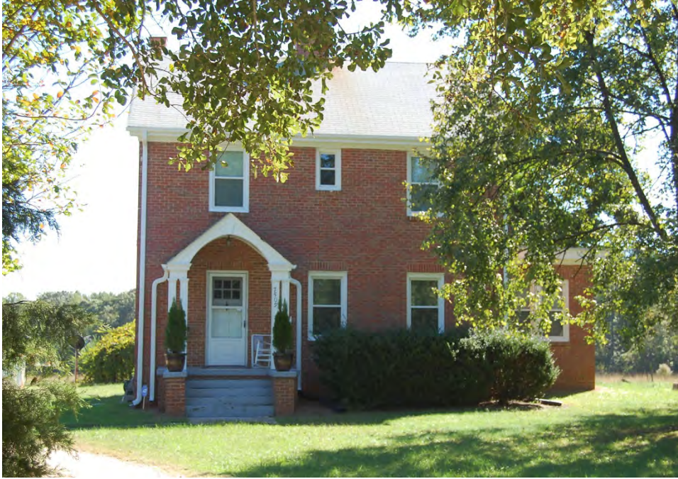
Plate 401. Dr. L. J. Faulhaber Farm, House, Façade, Looking East.
