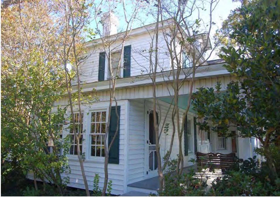
Plate 301. Icana Poole House, Enclosed Porch, West Elevation, Looking East.
