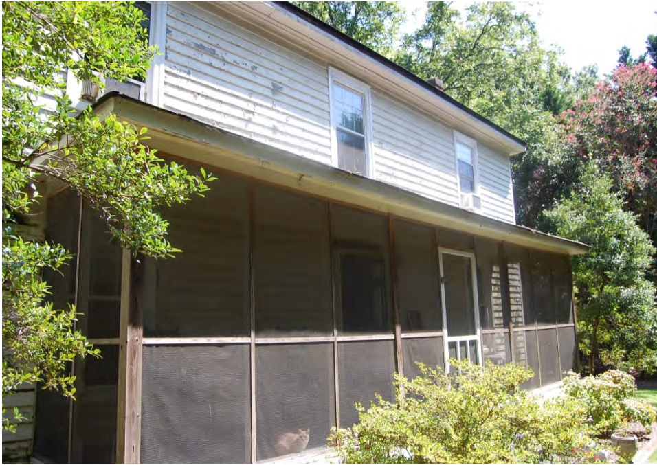
Plate 486. David Lewis House, Façade, Looking Northeast.
