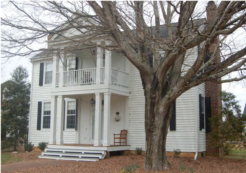
Plate 685. Burt-Utley House, Façade (South Elevation), Looking North.
