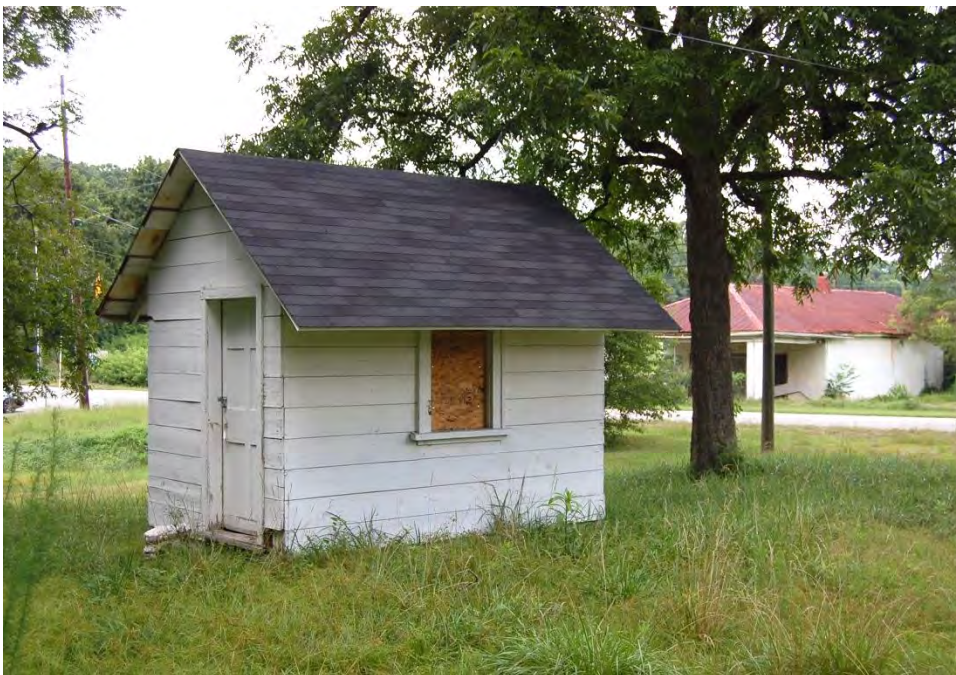
Plate 514. Johns-Lane-Poole House, Shed (circa 1925), Looking Northwest (Holland Smith Store in Background).
