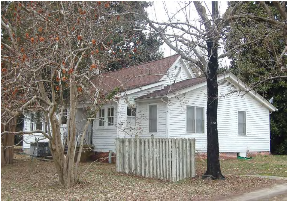
Plate 611. Jones-Johnson Farm, Ethelred Jones House, Rear (South) Elevation, Looking Northwest.
