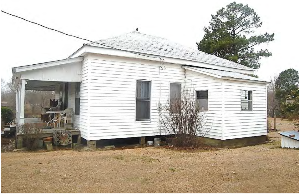
Plate 623. Grady Rowland House, Rear (North) Elevation, Looking South,
