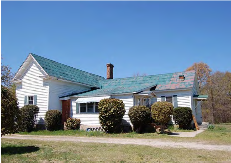
Plate 280. Gower-Johnson House, Side (South) Elevation and Rear Ell, Looking North.
