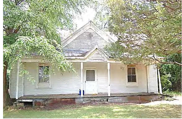
No. 181 House (WA1216) (PIN 0699739024), 9000 Old Stage Road, Williams Crossroads, Wake County
