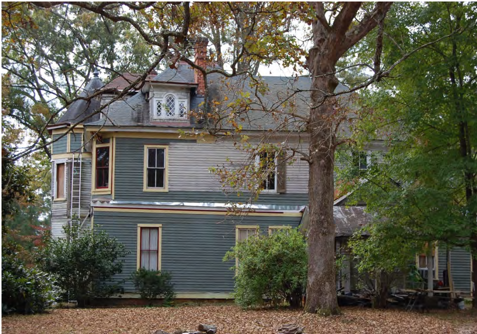
Plate 597. Atkinson-Whitted House, Side (North) Elevation, Looking East.
