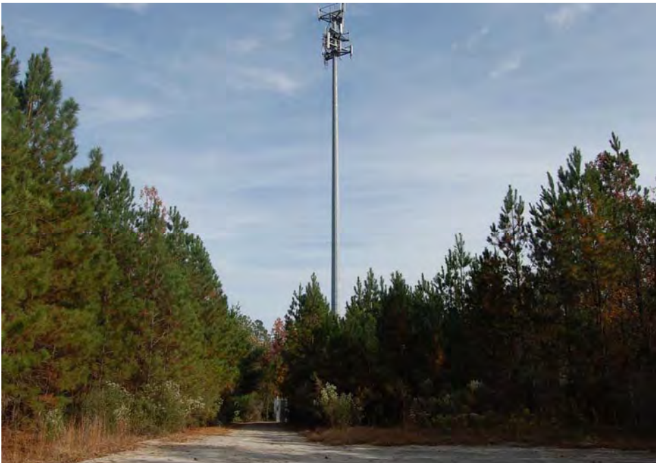
Plate 86. Bell-Pierce Farm, Western Tract, Cell Tower and Woodland, Looking East.
