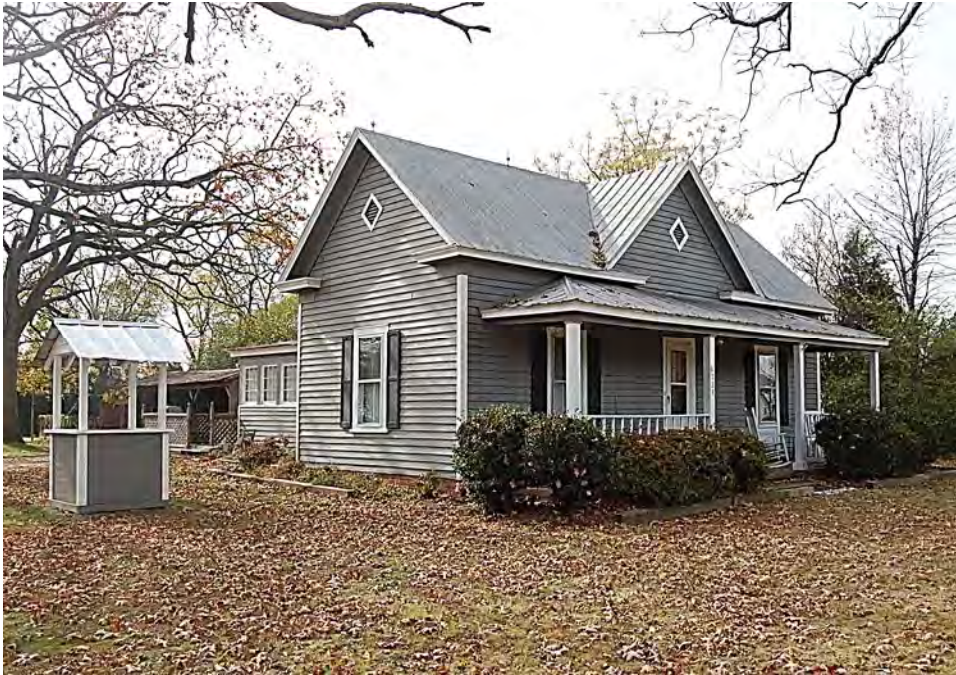
Plate 384. Arthur Atkins House, House and Setting, Looking South.
