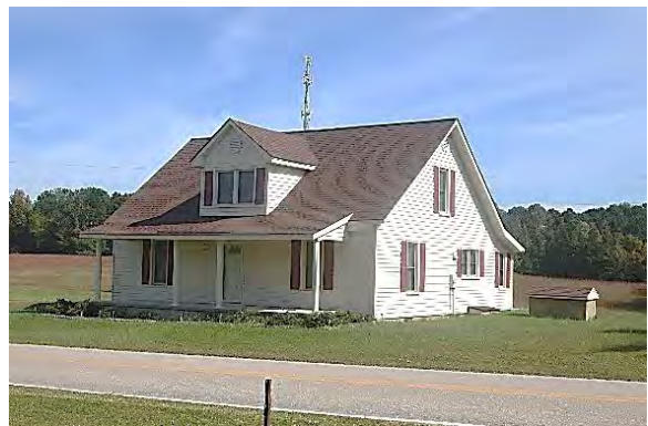
No. 235 House (PIN 1700856190), 802 Thompson Road, Garner Vicinity, Wake County
