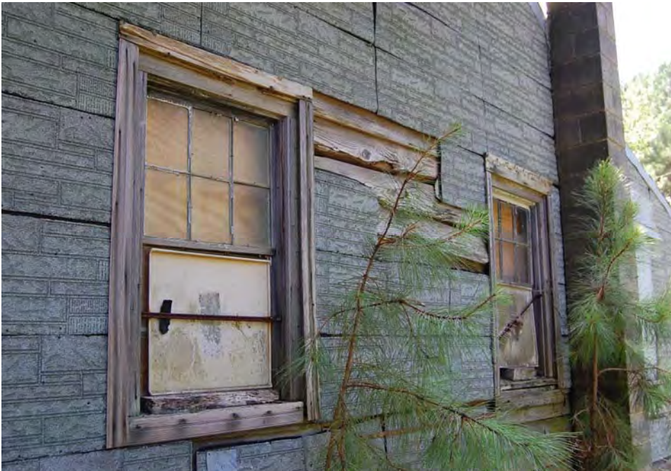
Plate 14. Wes Jones Farm, House, Side (North) Elevation, Looking Southwest.
