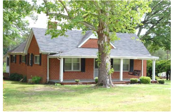
No. 162 House (PIN 1742480304), 2709 Hodge Road, Garner Vicinity, Wake County
