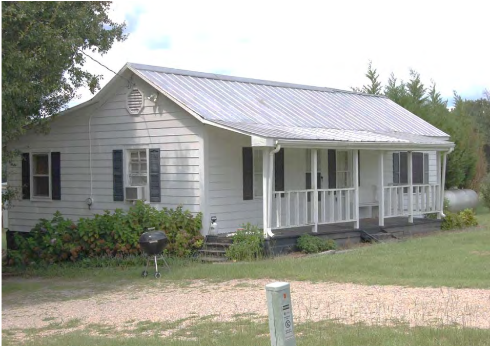
Plate 218. Jones Family Farm, Second House (No. 59) on West Side of Jordan Road, Looking West.
