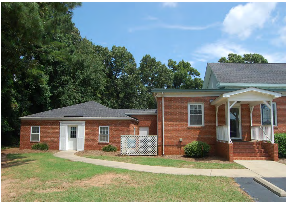
Plate 437. New Bethel Baptist Church, Rear Additions (1930s-1947), Looking North.
