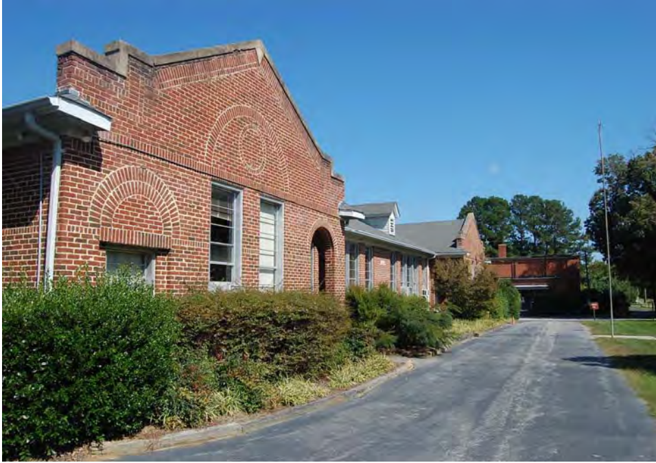
Plate 286. Mount Auburn School, Façade, Looking East Along Drive towards Gymnasium.
