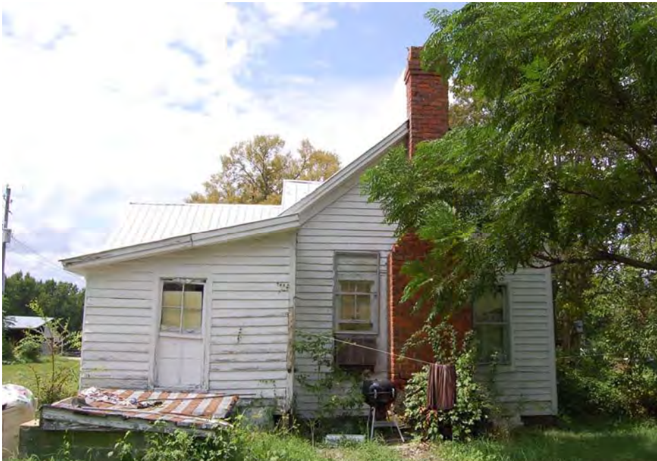
Plate 209. Jones Family Farm, House, Rear Elevation of Rear Ell, Looking West.
