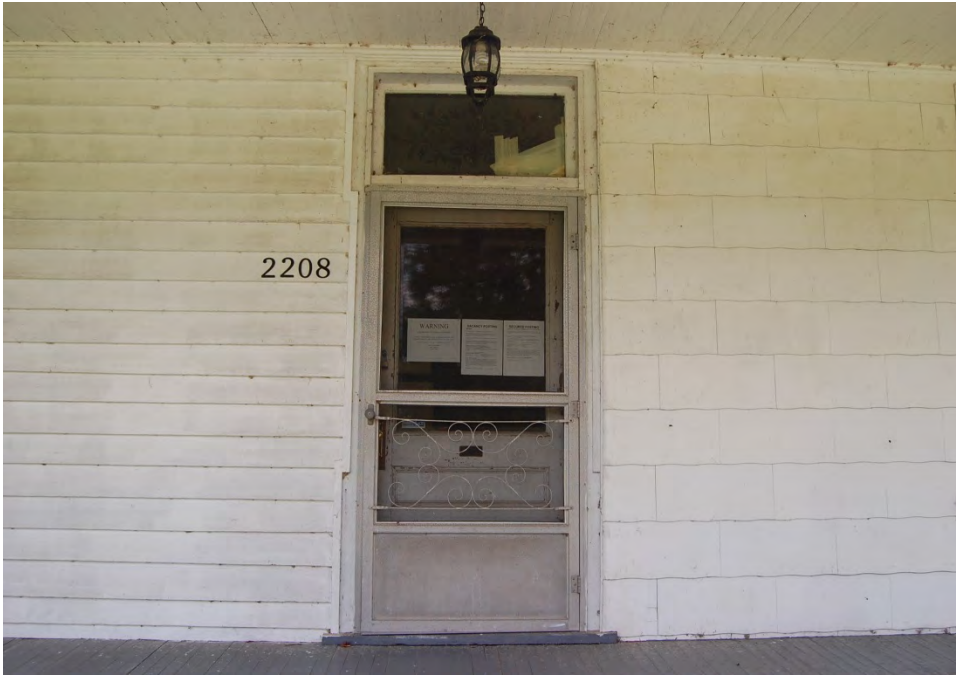
Plate 509. Johns-Lane-Poole House, Detail of Front Entrance.
