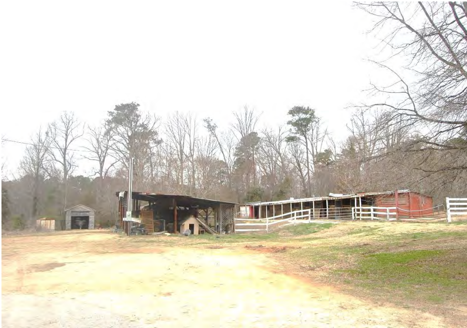
Plate 619. Ballentine Farm, Sheds and Garage, Looking West.
