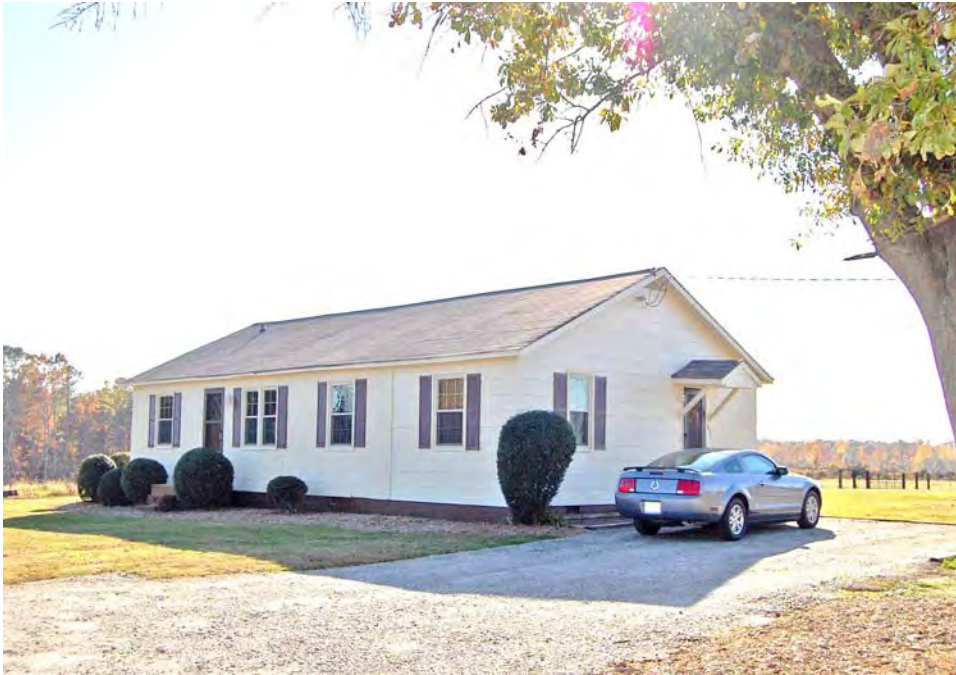
Plate 35. Pierce Farm, Modern House, Looking Southwest.
