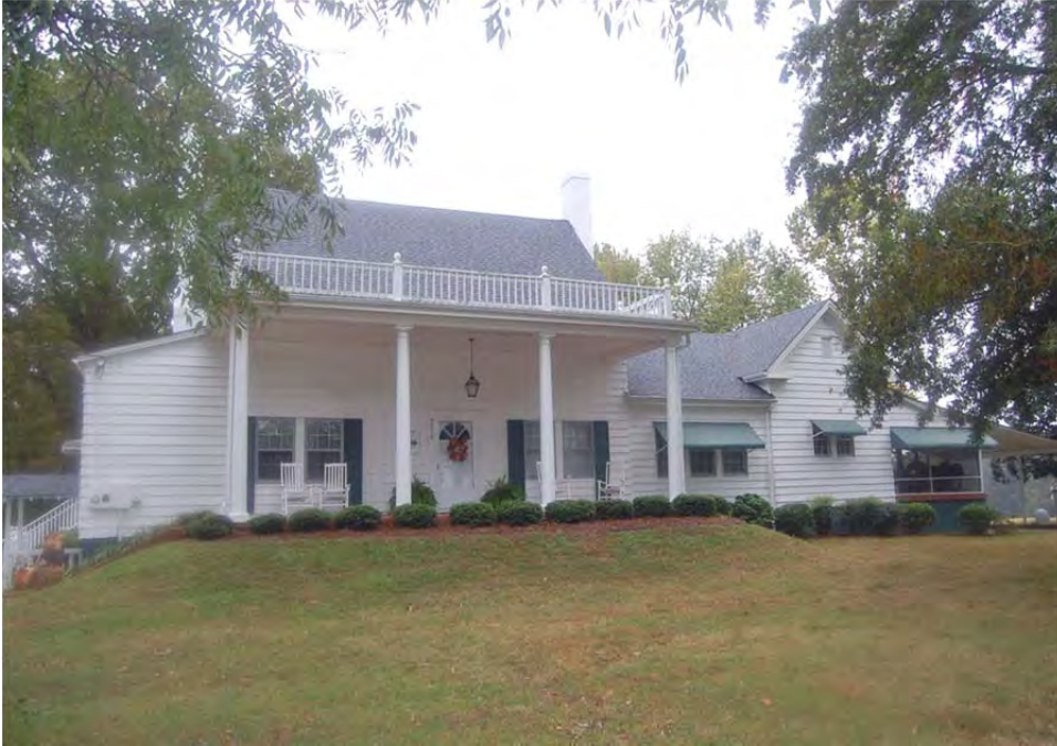
Plate 346. The Oaks, House Facade, Looking West.
