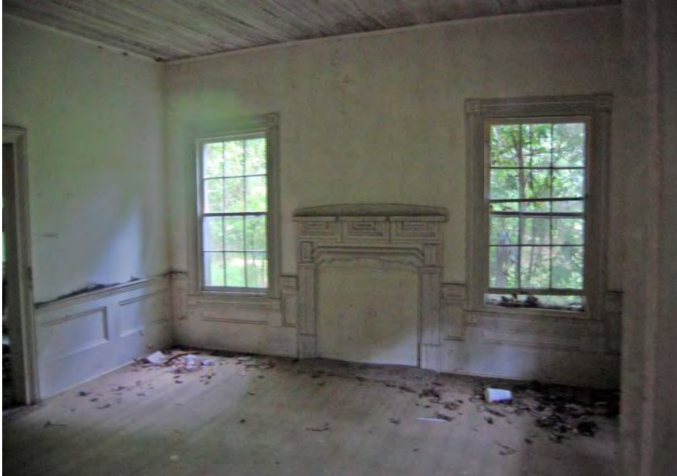
Plate 326. Penny House, Interior, South Room, Mantel, Wainscoting, and Window Surrounds.
