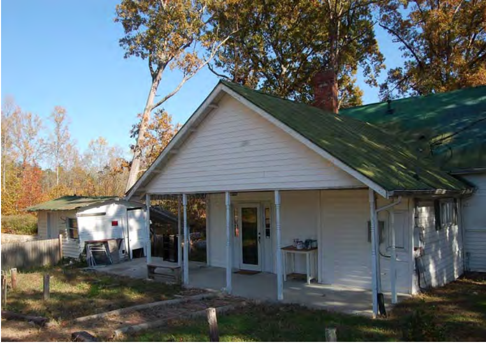
Plate 5. G. L. Pierce House, Rear (West) Elevation and Shed, Looking Northeast.
