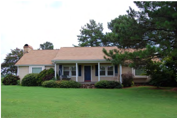
No. 47 House (PIN 0698778963), 9901 Old Stage Road, Williams Crossroads Vicinity, Wake County
