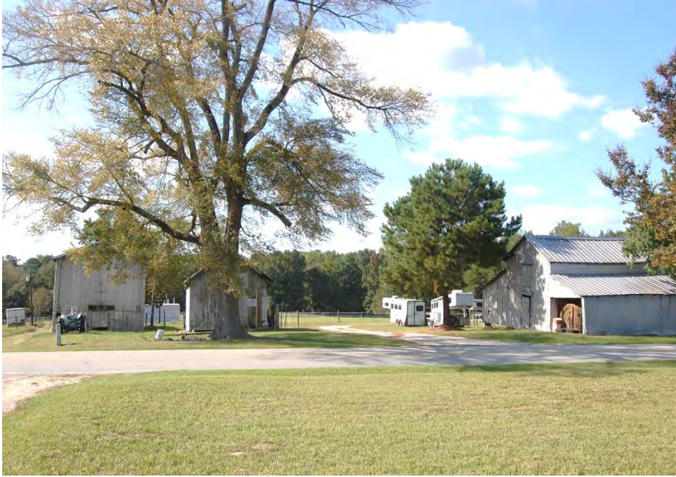
Plate 214. Jones Family Farm, Outbuildings on West Side of Jordan Road, Looking West from House.
