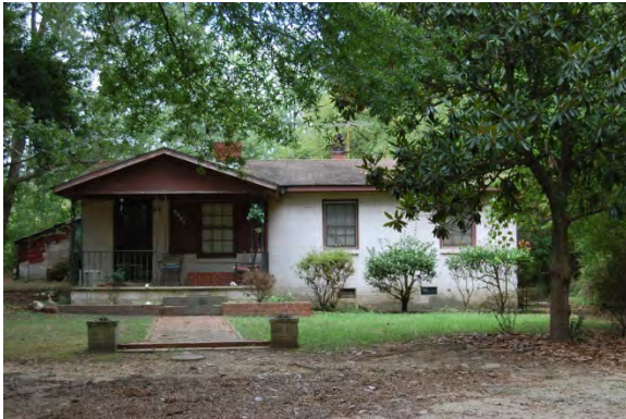
No. 1 House (PIN 0740940641), 2208 East Williams Street, Apex, Wake County
