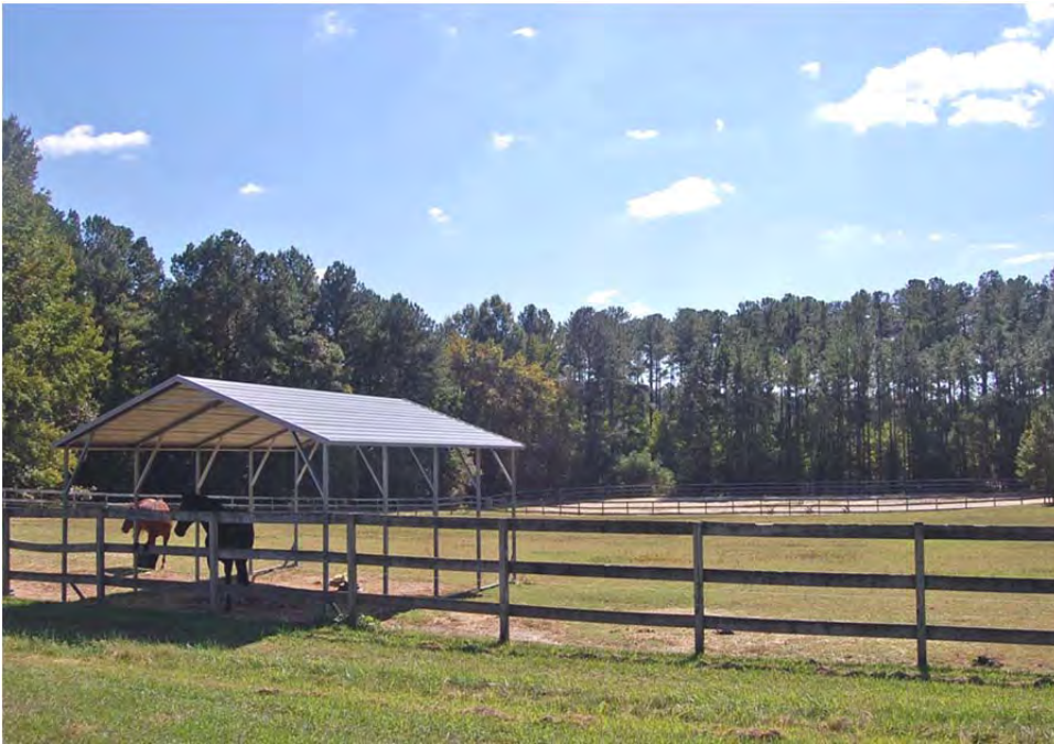
Plate 259. John Williams Farm, Pasture and Run-In Shed, Looking South.
