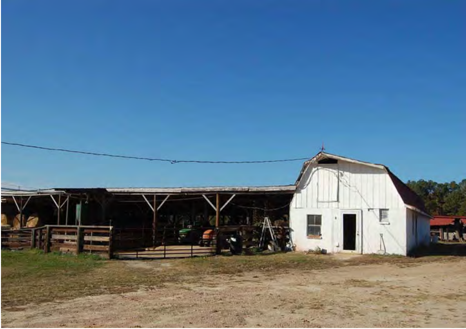
Plate 29. Pierce Farm, Dairy Barn, Looking North.
