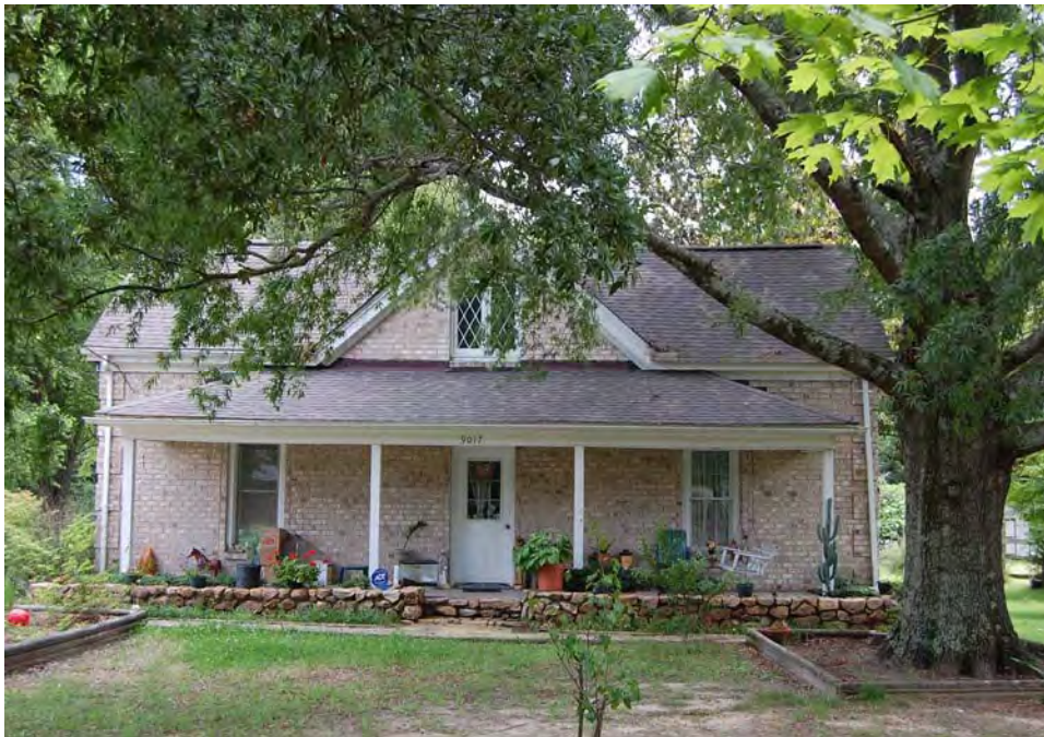
Plate 176. Juniper Level, House, 9017 Sauls Road, Looking East.
