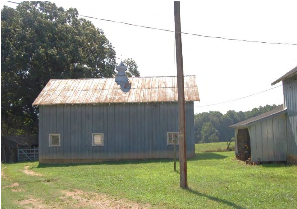
Plate 406. Dr. L. J. Faulhaber Farm, Dairy Barn, East Side of Complex, Looking East.
