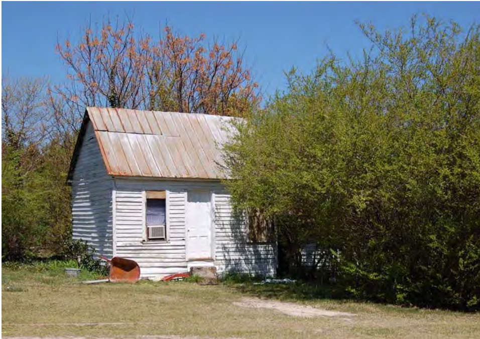
Plate 282. Gower-Johnson House, Original Kitchen, Looking North.
