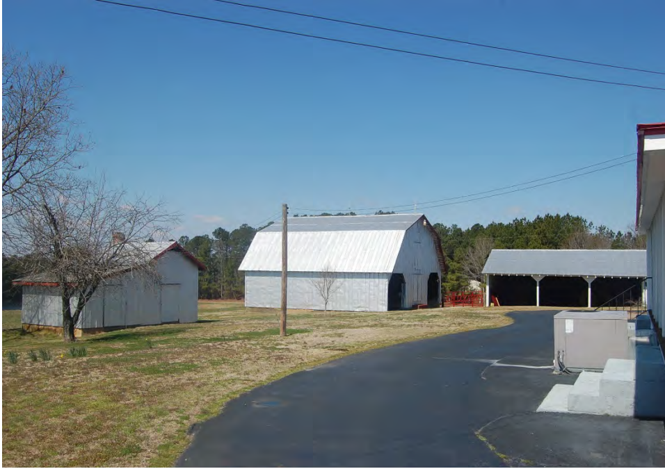
Plate 633. Joseph M. Blalock Farm, Potato House, Packhouse, Looking North.
