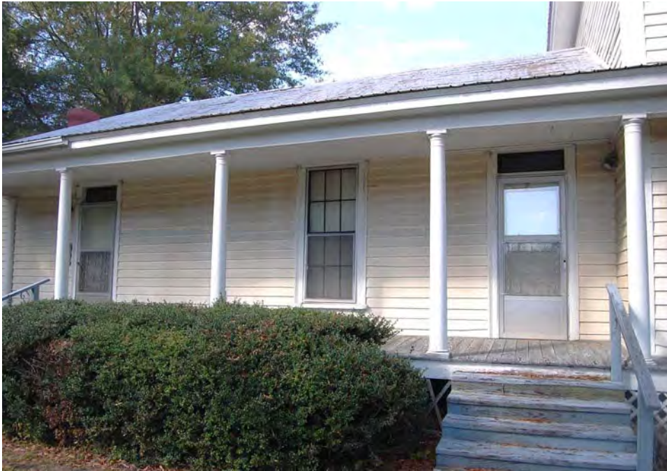
Plate 93. John B. Strain House, Rear Porch, South Elevation, Looking North.
