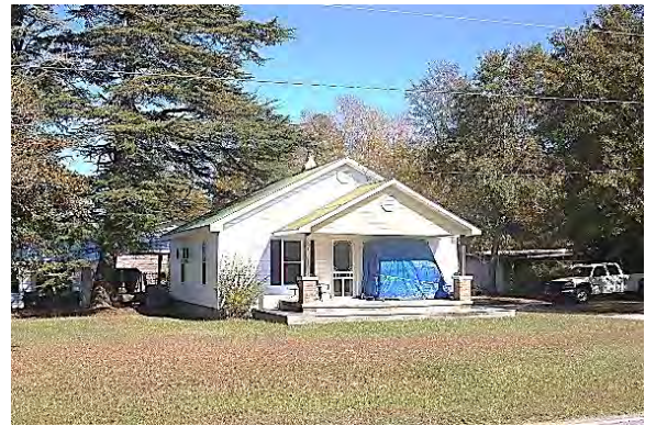
No. 308 House (PIN 162700-37-5793), 13456 Cleveland School Road, Garner Vicinity, Johnston County
