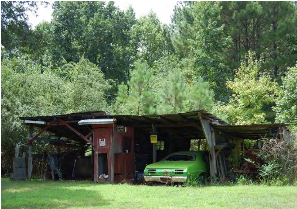
Plate 18. Wes Jones Farm, Equipment Storage Shed, East Side of Pierce Olive Road, Looking East.
