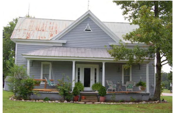
No. 31 House (WA1223) (PIN 0699422621), 9013 Fanny Brown Road, McCullers Crossroads Vicinity, Wake County
