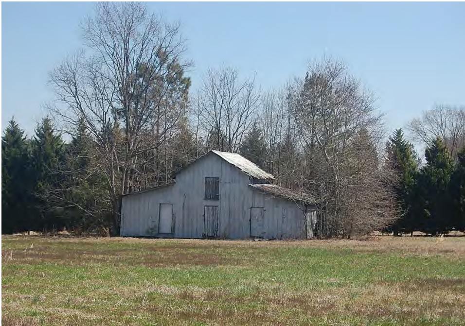
Plate 681. Thomas Woolard Farm, Packhouse, Looking East.
