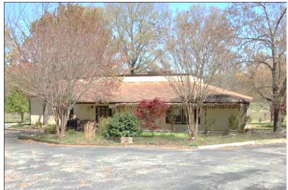
No. 95 House (PIN 1639765023) 2917 Escondido Farm Road, Garner Vicinity, Wake County
