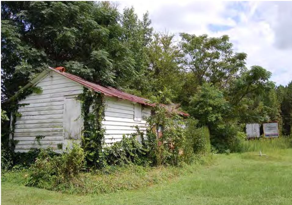
Plate 213. Jones Family Farm, Tobacco Grading Room behind House, Looking East.
