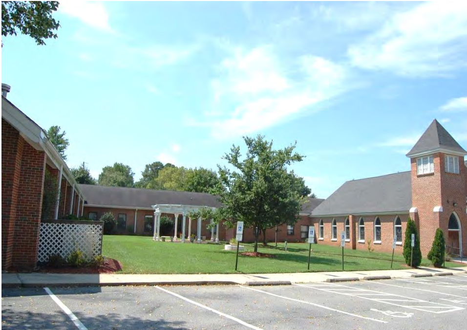
Plate 430. Popular Springs Christian Church, 1932 Church, Side (East) Elevation, and 1996 Wing, Looking Southwest.
