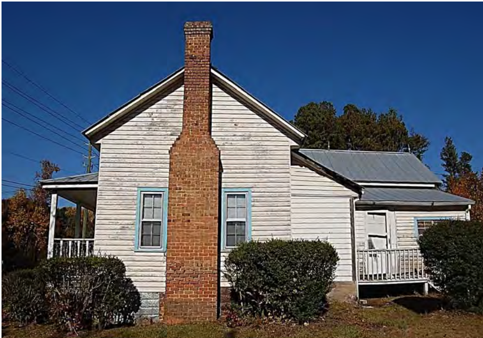
Plate 380. William Pierce House, Side (South) Elevation, Looking North.
