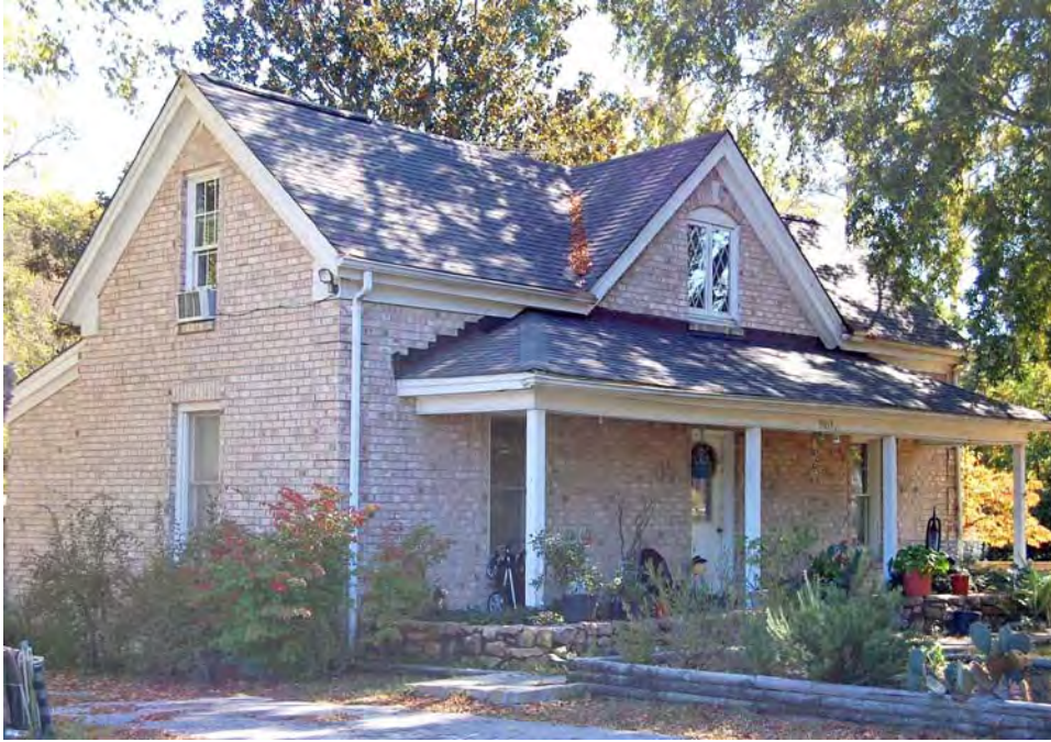
Plate 177. Juniper Level, House, 9017 Sauls Road, Looking Southeast.
