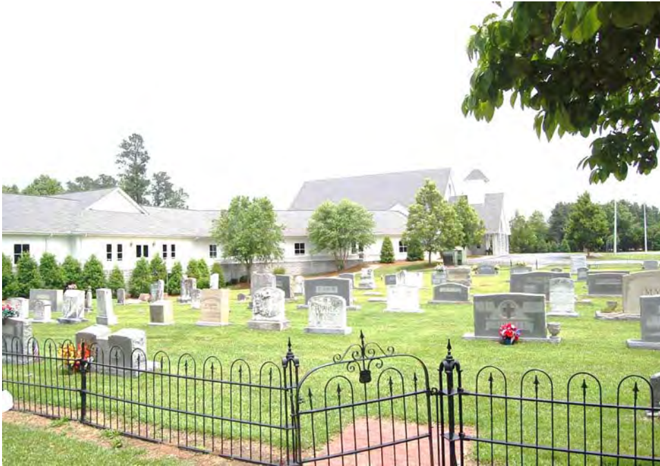
Plate 139. Williams Crossroads, Hollands Methodist Church, Cemetery, Looking East towards Modern Additions.
