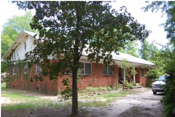
No. 23 House (PIN 0689455964), 8537 Lake Wheeler Road, McCullers Crossroads Vicinity, Wake County
