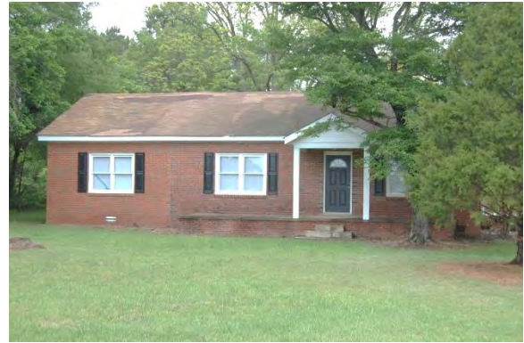
No. 160 House (PIN 1742369880), 2905 Hodge Road, Garner Vicinity, Wake County
