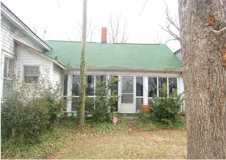
Plate 583. James Sugg House, Rear Bathroom Addition and Rear Ell, Looking East.
