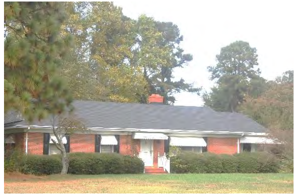
No. 251 House (PIN 1720446107), 7400 Bryan Road, Garner Vicinity, Wake County
