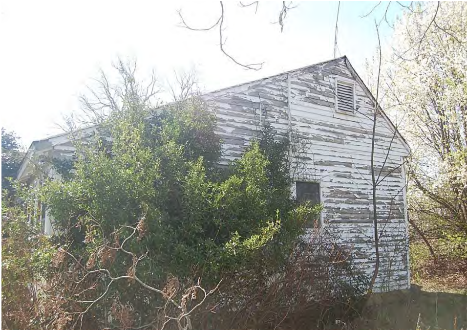
Plate 680. Thomas Woolard Farm, House, Rear Ell, Rear (North) Elevation, Looking South.
