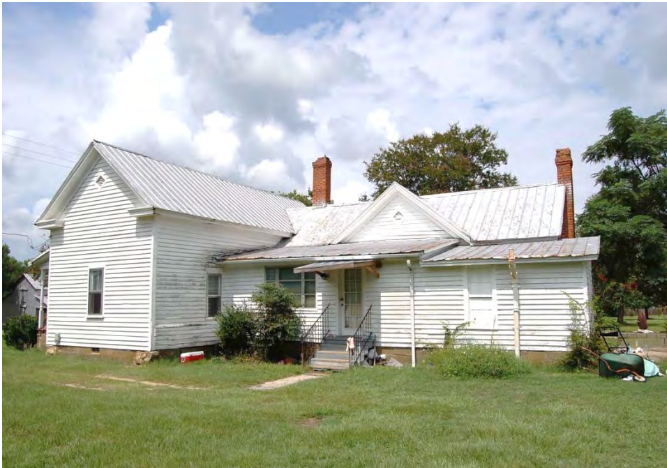
Plate 207. Jones Family Farm, House, Side (South) Elevation and Rear Ell, Looking North.
