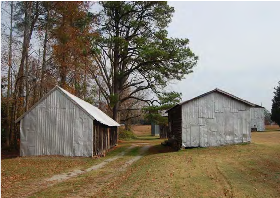
Plate 155. George Williams Farm, Packhouses, Looking East.
