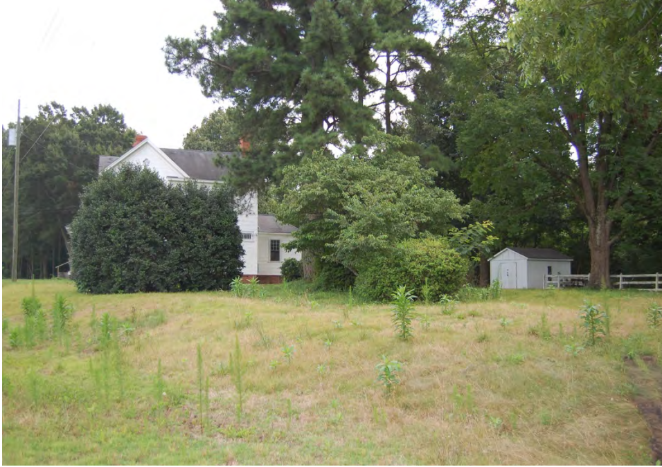
Plate 515. Johns-Lane-Poole House, House, Modern Shed, and Setting, Looking East.
