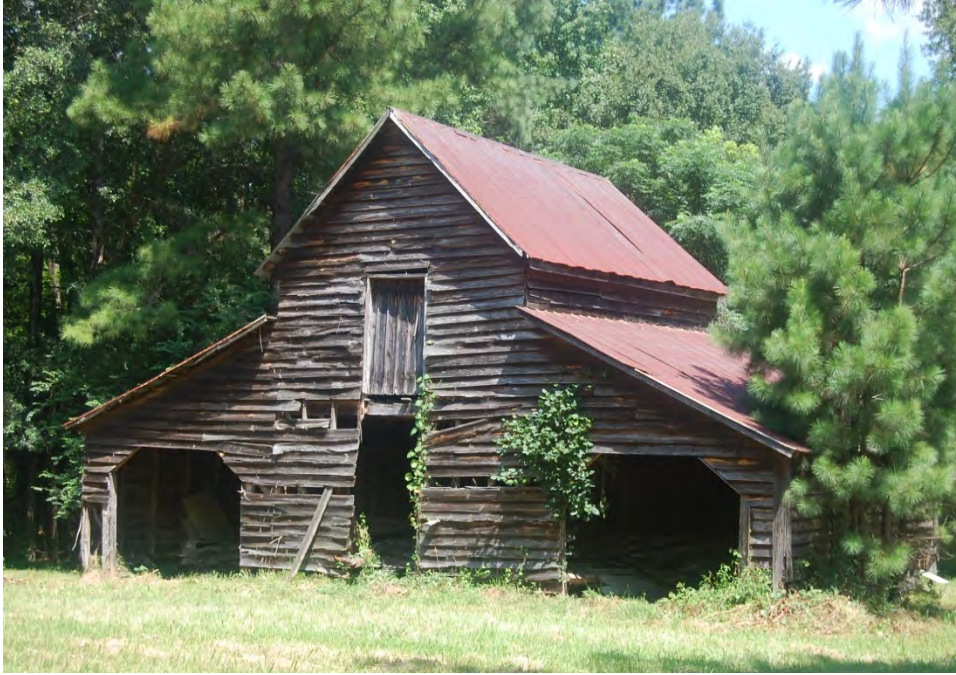
Plate 483. Yeargan House, Hay Barn, Looking North.
