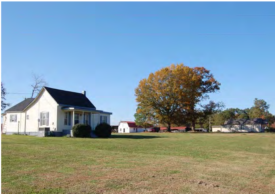
Plate 20. Pierce Farm, Relocated Nineteenth-Century House (Foreground), Looking North towards Dairy Barn and Pierce House.
