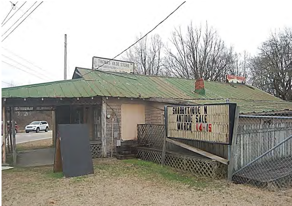
Plate 573. Thomas Store, Side (Northwest) Elevation, Looking Southeast.
