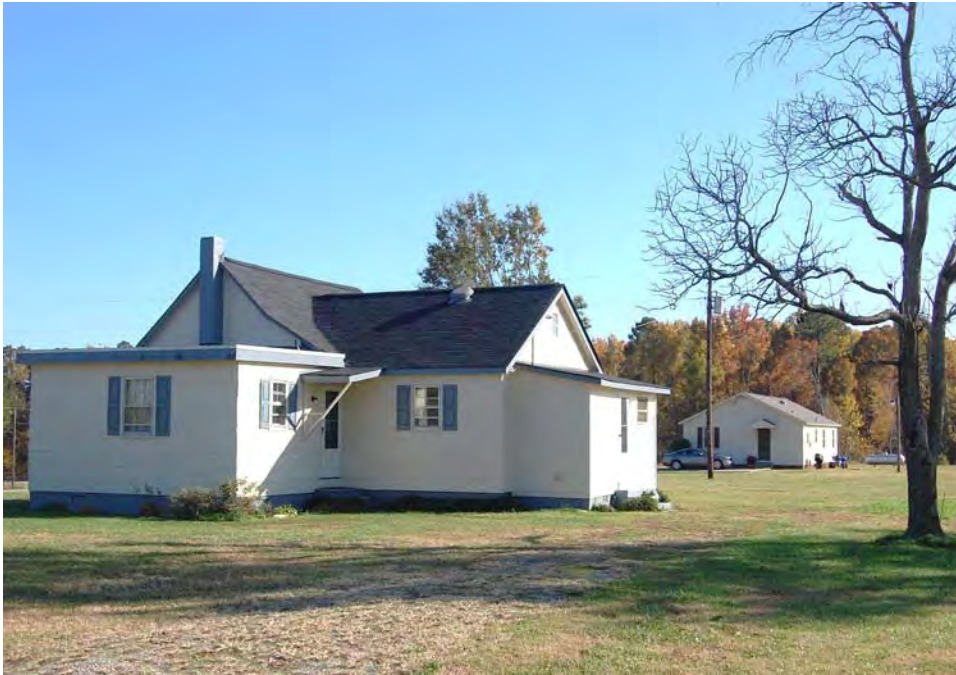
Plate 25. Pierce Farm, Relocated Nineteenth-Century House, Rear (East) Elevation, Looking South.
