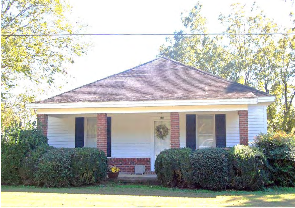
Plate 547. Auburn, House (No. 278), Looking South.
