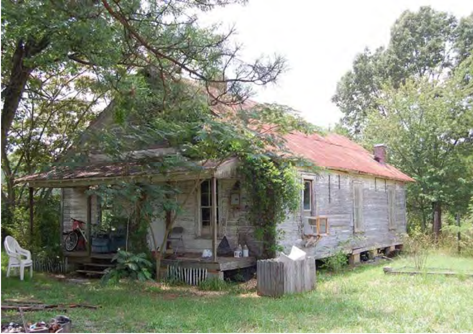
Plate 143. Williams Crossroads, House on West Side Old Stage Road, Looking West.
