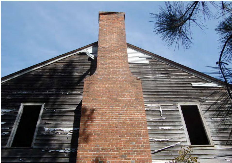
Plate 413. David and Sarah Stephenson House, South Elevation Chimney, Looking North.
