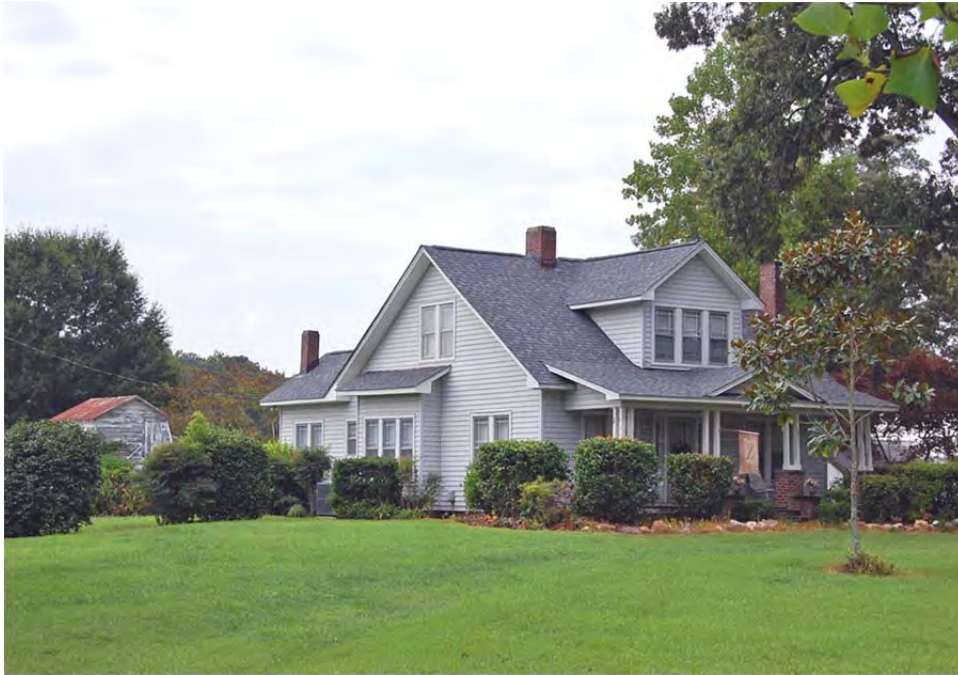
Plate 114. Percy and Mynette Strother House, House and Setting, Looking Southwest.
