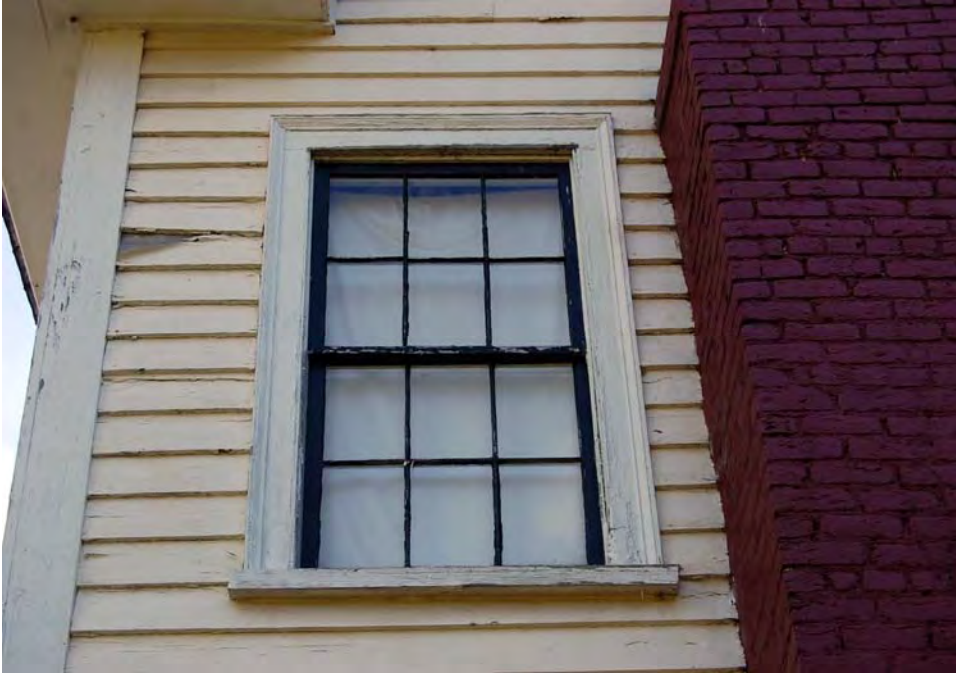
Plate 95. John B. Strain House, Window Detail, South Elevation.
