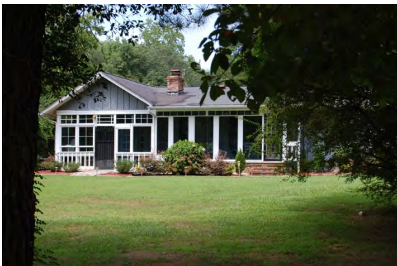
No. 6 House (PIN 0669096690), 9640 Holly Springs Road, Holly Springs, Wake County
