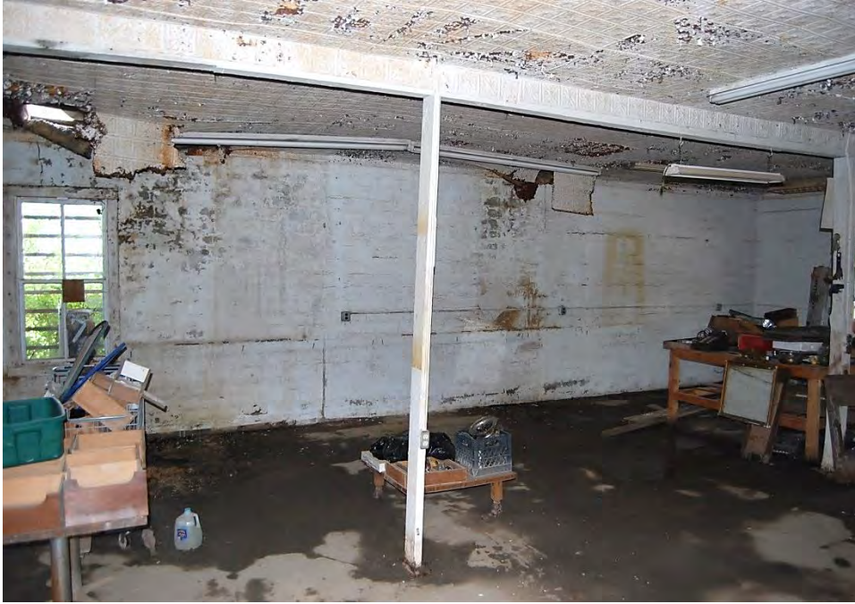
Plate 541. Auburn, Holland Smith Store (No. 272), Interior, Showing Added Supports and Water Damage.
