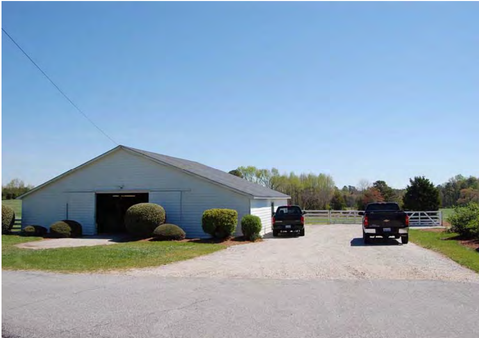
Plate 252. Richard Burnette House, Modern Equipment Storage Building, Looking East.
