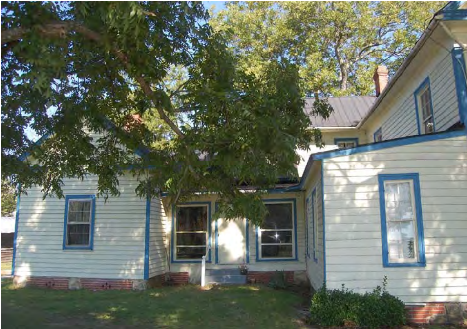
Plate 264. W. A. Gowers Farm, House, Side (South) Elevation, Looking North.
