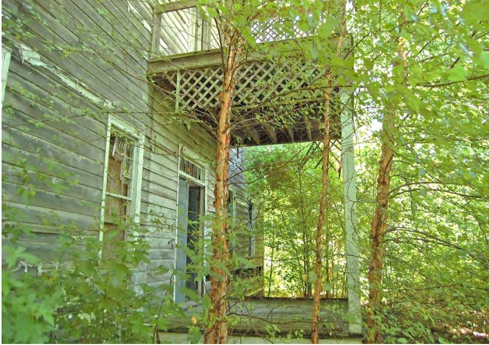
Plate 410. David and Sarah Stephenson House, Façade (West Elevation), Looking South.
