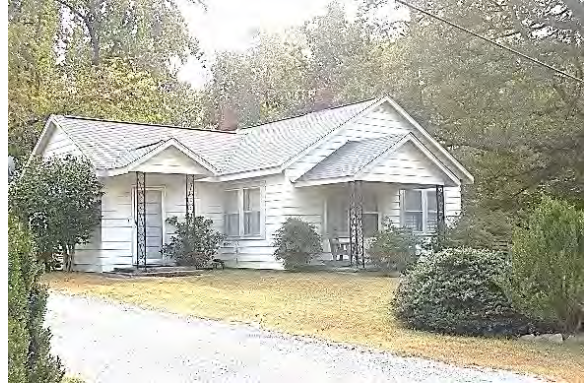
No. 244 House (PIN 1629192837), 7981 Bryan Road, Garner Vicinity, Wake County
