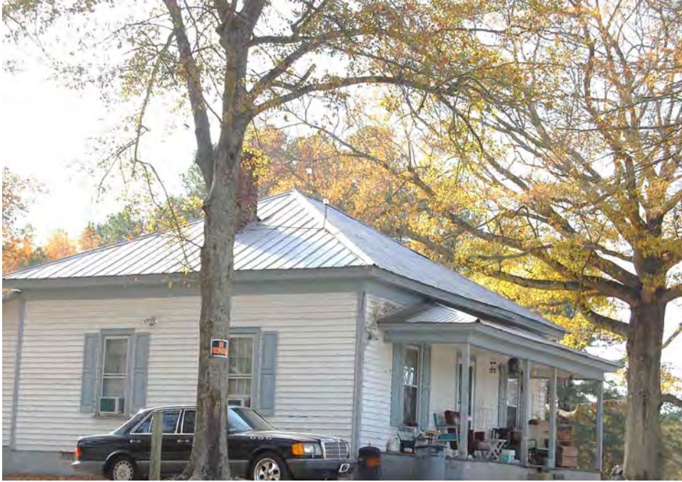
Plate 141. Williams Crossroads, Hip-Roofed Dwelling (Outside APE) on South Side of Ten Ten Road, Looking West.
