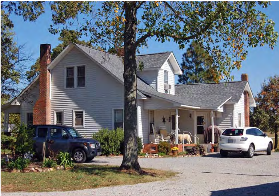
Plate 119. Percy and Mynette Strother House, Side (West) and Rear (South) Elevations, Looking East.
