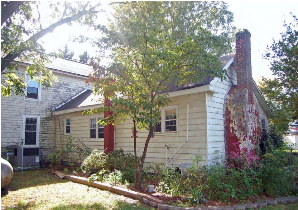
Plate 489. David Lewis House, Rear Ell, East Elevation and Chimney, Looking Southwest.
