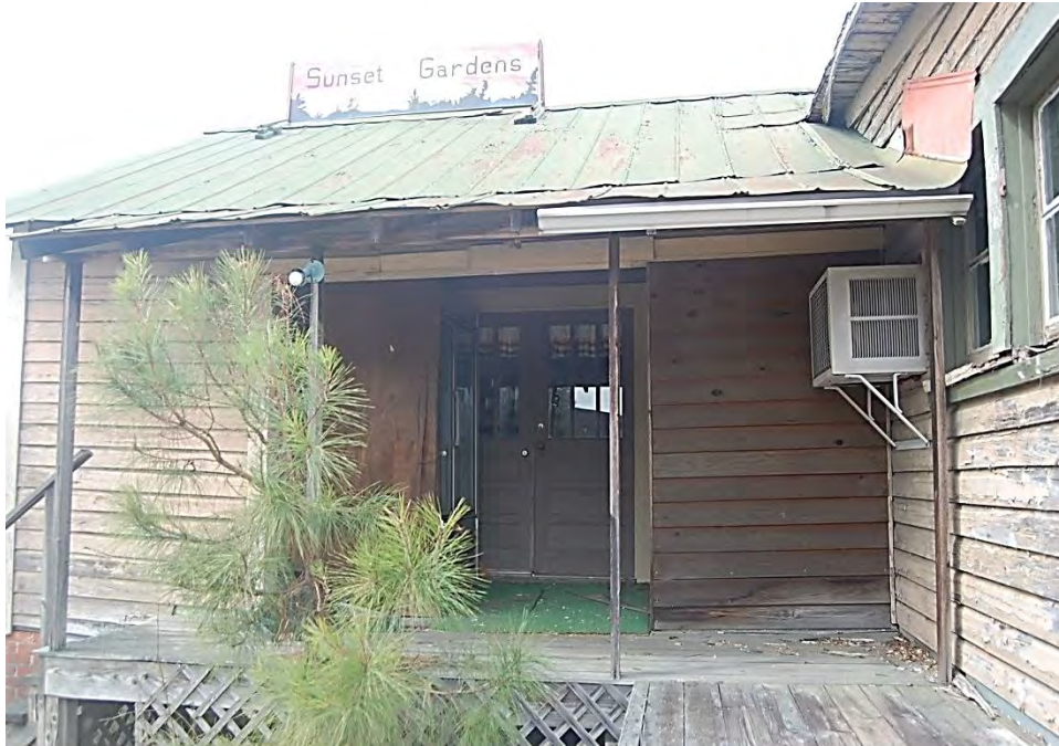
Plate 575. Thomas Store, Rear Ell, Porch and Entrance, Looking Northwest.
