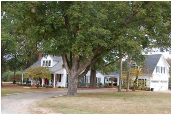
No. 319 House and Outbuildings (WA R-164) (PIN0677474471) 2321 North Main Street, Fuquay-Varina Vicinity, Wake County
