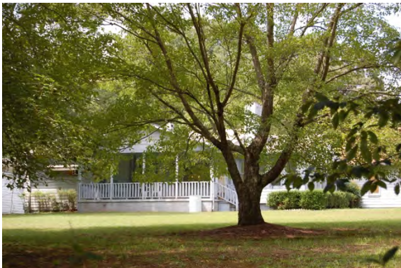
No. 4 House (PIN 0760100641), 4512 Kildaire Farm Road, Holly Springs, Wake County
