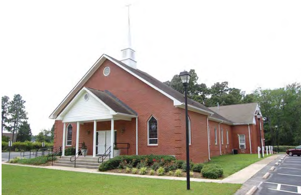
Plate 174. Juniper Level, Juniper Level Baptist Church, West Side of Sauls Road, Looking West.
