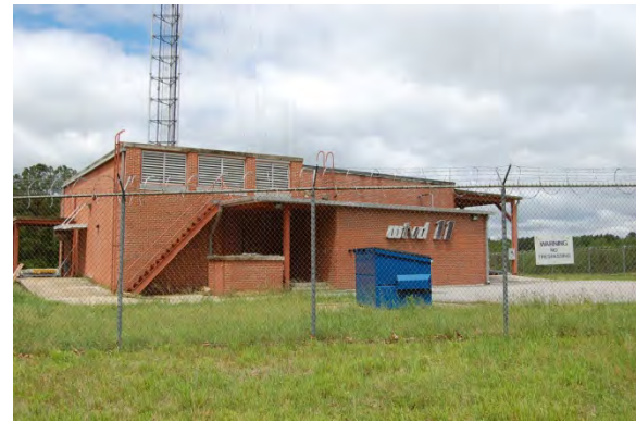
No. 154 Office and Transmitter Building (PIN 1639888459), 2901 Transmitter Road, Garner Vicinity, Wake County
