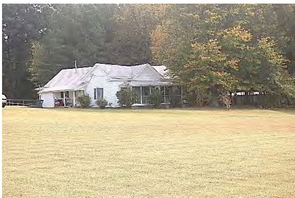
No. 252 House (PIN 1720533317), 2200 Salt Hill Road, Garner Vicinity, Wake County
