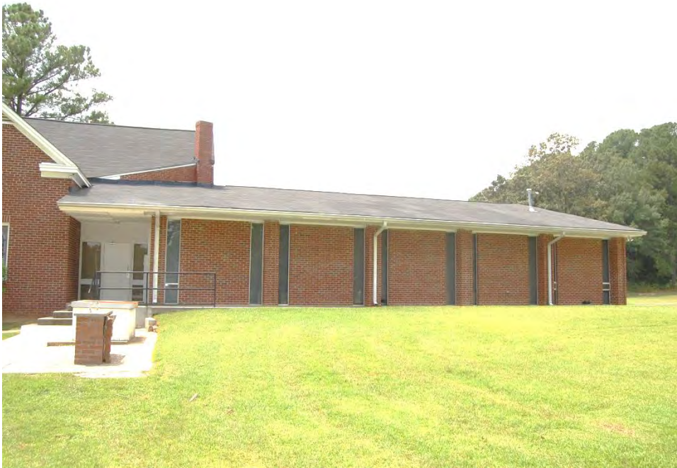
Plate 520. Springfield Baptist Church, Rear Addition, Side (East) Elevation, Looking West.
