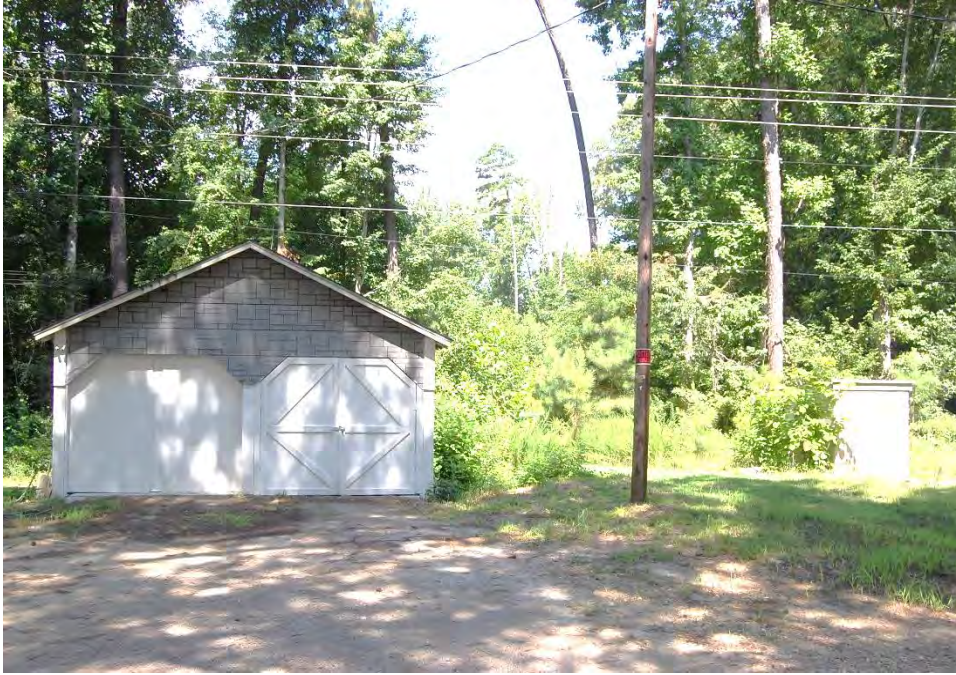
Plate 425. Willis House and Store, Garage and Pump House, Looking West.
