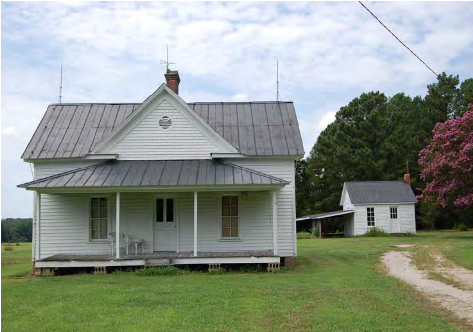
Plate 42. C. B. Sorrell House, House and Storage Building, Looking West.
