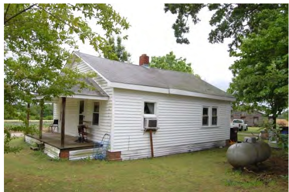
No. 156 House (PIN 1742437356), 3137 Hodge Road, Garner Vicinity, Wake County
