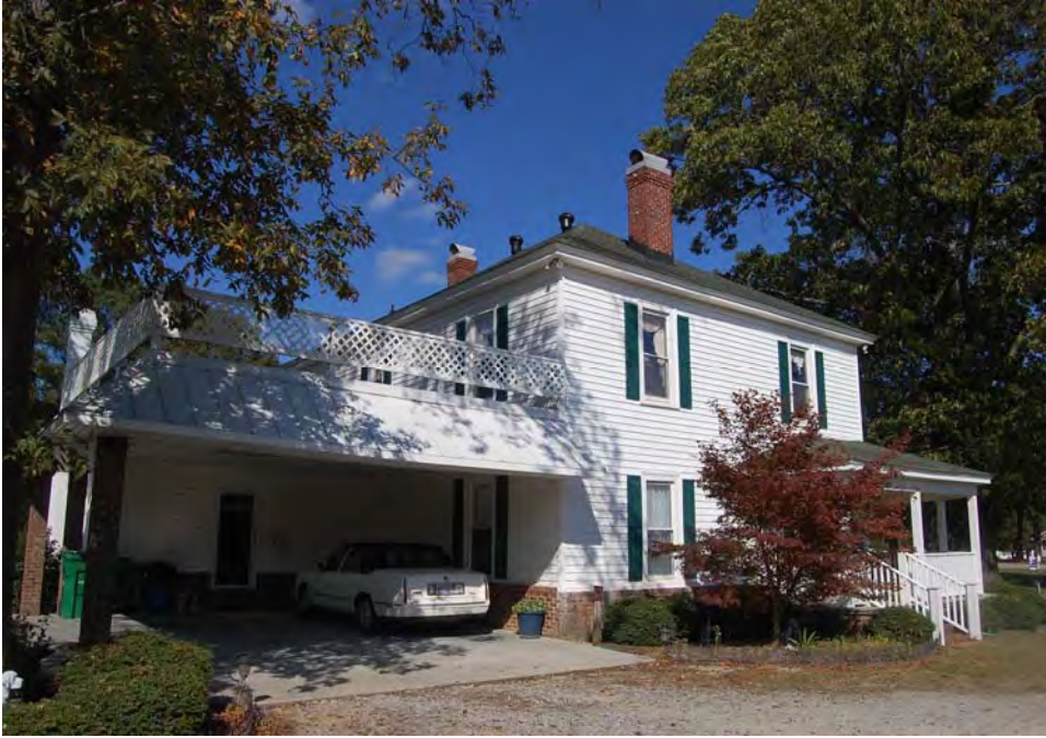
Plate 170. Samuel Jefferson Rhodes House, Side (South) Elevation and Carport, Looking Northeast.
