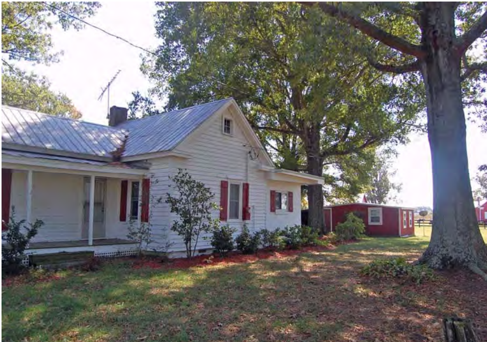
Plate 231. Umstead Farm, House, Looking South towards Office.
