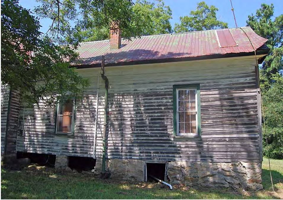
Plate 479. Yeargan House, Rear Ell, Side (East) Elevation, Looking West.
