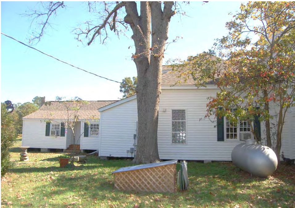
Plate 304. Icana Poole House, Side (West) Elevation, Looking East.
