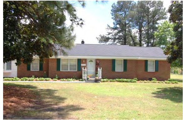
No. 172 House (PIN 1743246207), 5125 Faison Ridge Lane, Garner Vicinity, Wake County
