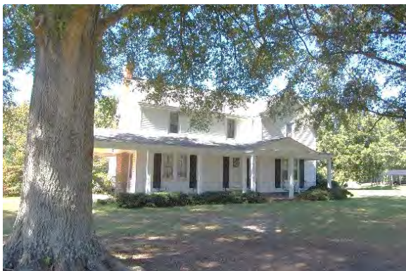
No. 213 House (WA1272) (PIN 0699193653), 7414 Fayetteville Road, Garner Vicinity, Wake County
