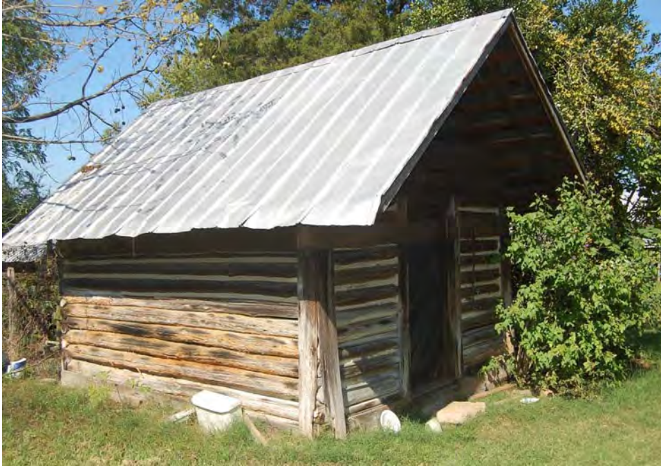
Plate 270. W. A. Gowers Farm, Log Smokehouse, Looking Northwest.
