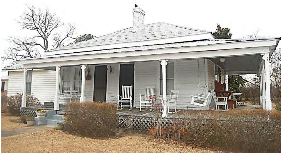
Plate 622. Grady Rowland House, Front (South) and Side (East) Elevations, Looking Northwest.
