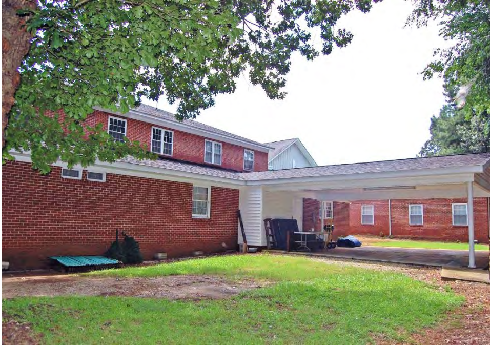
Plate 440. New Bethel Baptist Church, 1954 Classroom and Fellowship Hall Building, Rear Elevation with 1995 Additions, Looking Southeast.
