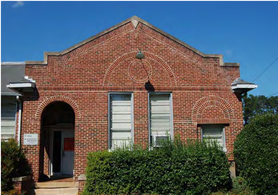
Plate 287. Mount Auburn School, Façade, Detail of East Entrance, Looking North.
