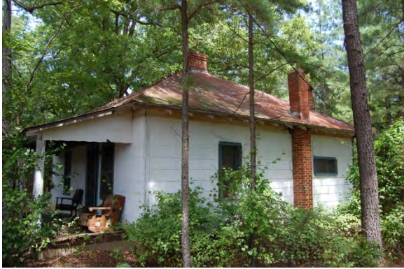
No. 12 House (PIN 0770217795), 3909 West Lake Road, Holly Springs Vicinity, Wake County
