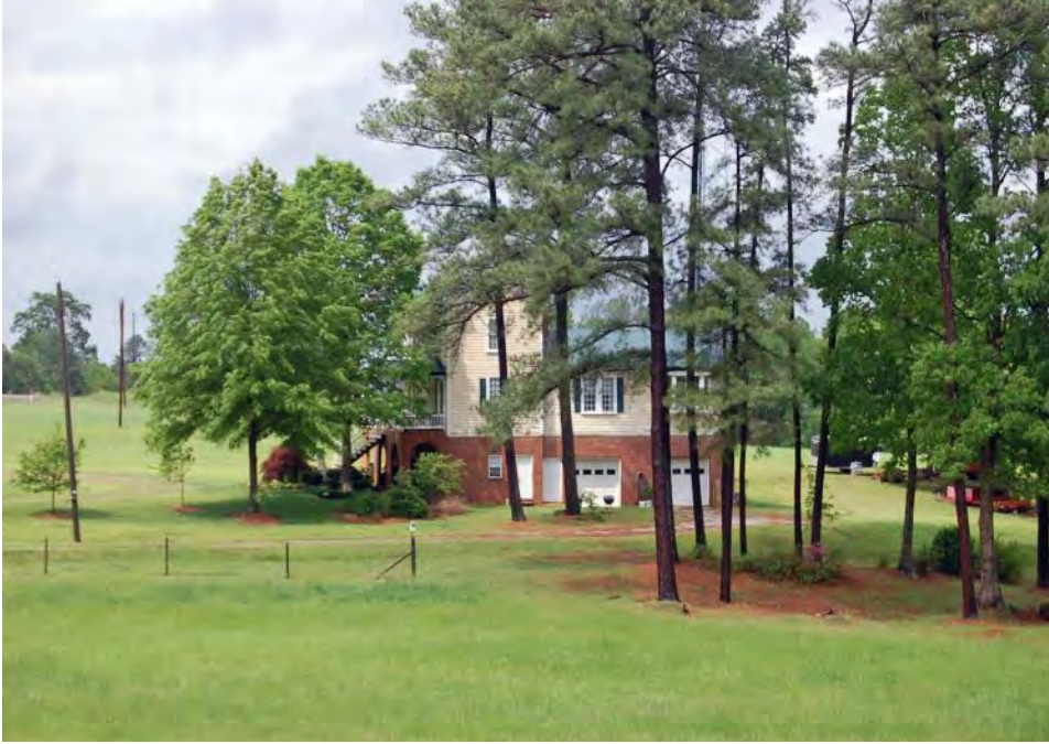
Plate 333. Walter Stallings House, Side (South) Elevation and Setting, Looking North.
