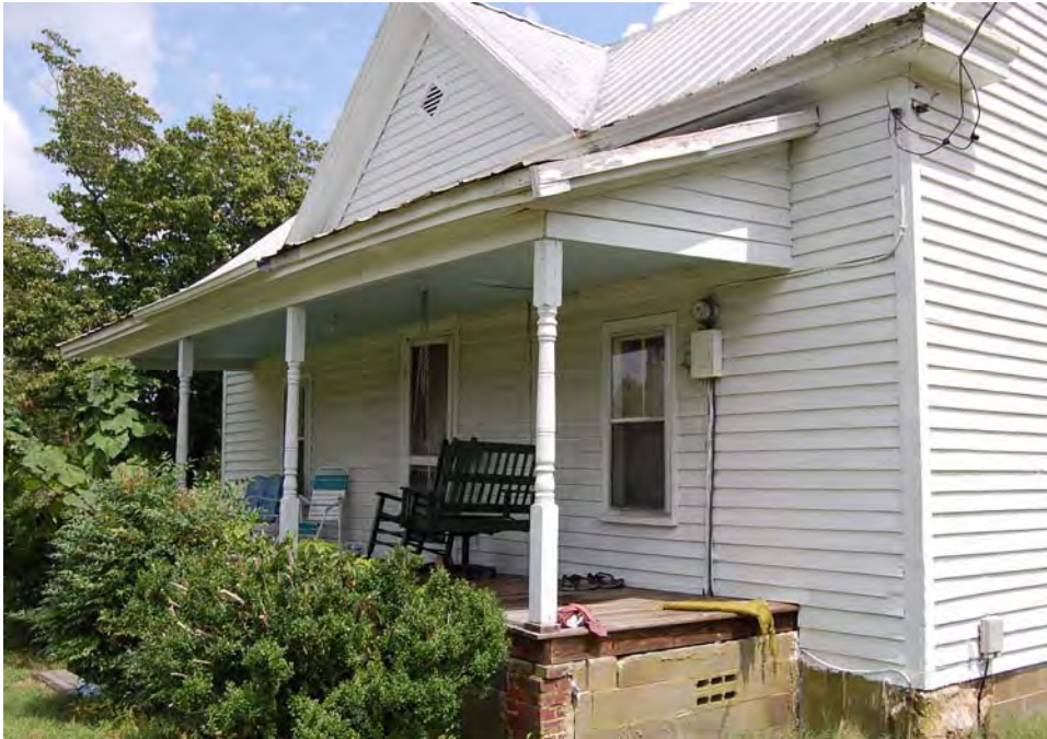
Plate 206. Jones Family Farm, House, Looking Northeast.
