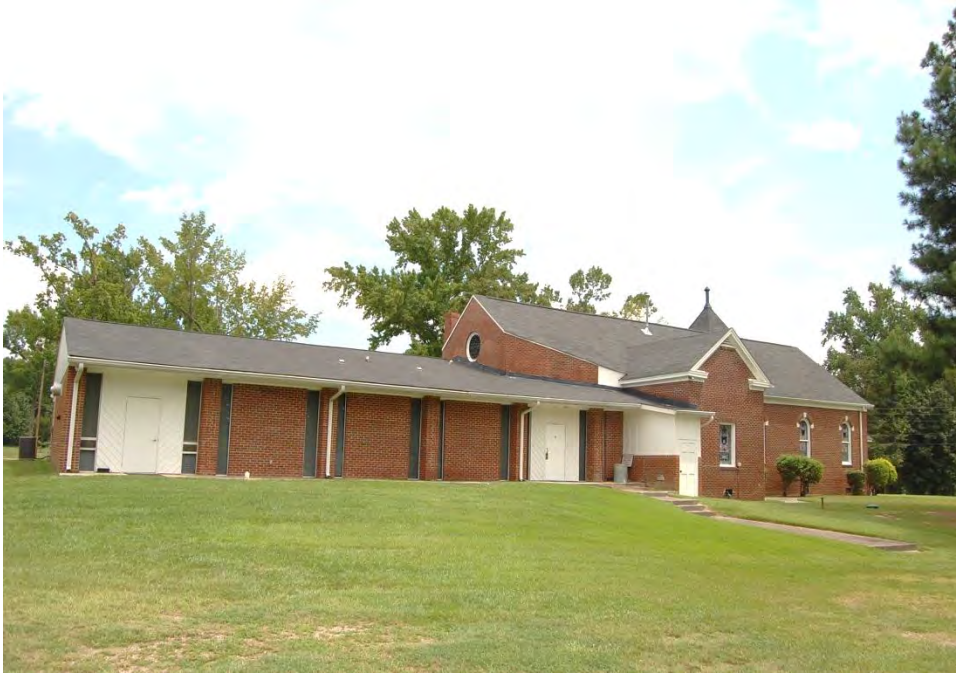
Plate 518. Springfield Baptist Church, Side (West) Elevation and Rear Addition, Looking East.
