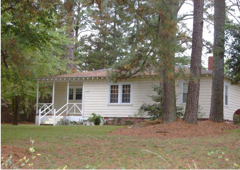
Plate 531. Auburn, House (No. 268), Looking West.
