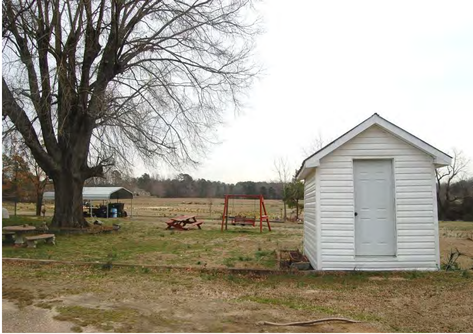
Plate 570. W. C. Thomas House, Smokehouse, Looking East.
