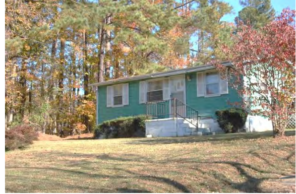
No.190 House (PIN 0669097185), 9713 Holly Springs Road, Garner Vicinity, Wake County
