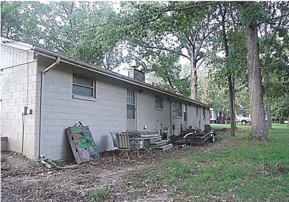
Plate 368. Gerald Cochran House, Rear (East) Elevation, Looking Northwest.
