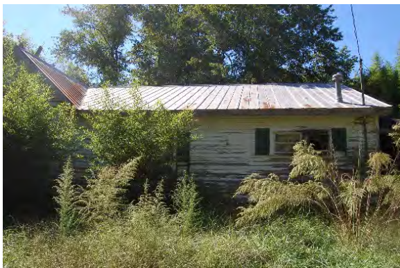
No. 202 House (PIN 0689598036), 8216 Lake Wheeler Road, Garner Vicinity, Wake County
