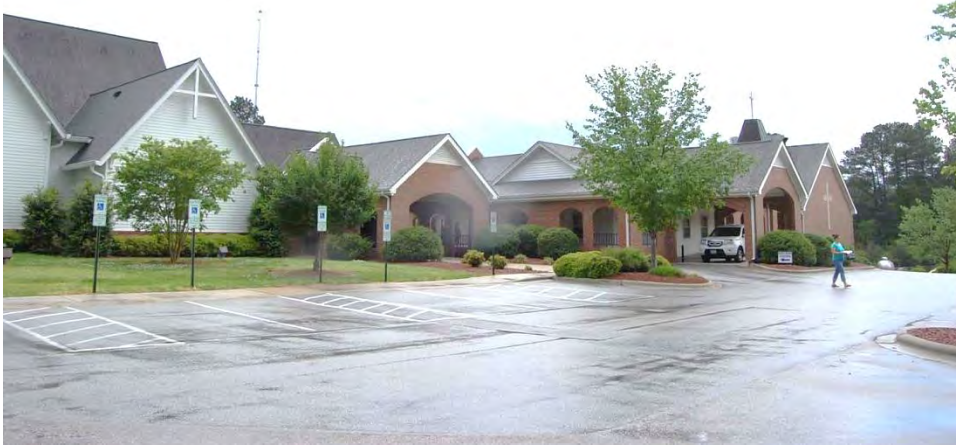
Plate 310. Mount Moriah Baptist Church, 1994-1999 Educational Building, Looking Southwest.
