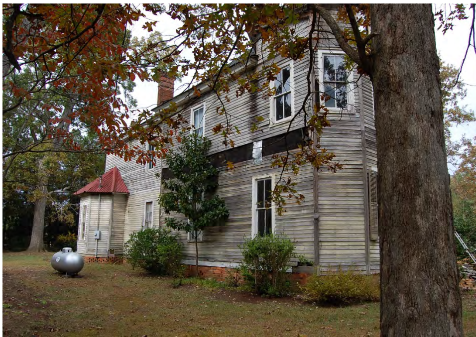
Plate 598. Atkinson-Whitted House, Side (South) Elevation, Looking West.
