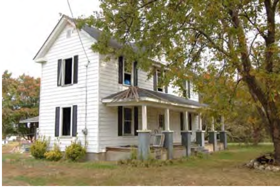
No. 323 Charles Rowland House (WA 1127) (PIN 0687027391), 6910 Kennebec Road, Fuquay-Varina Vicinity, Wake County
