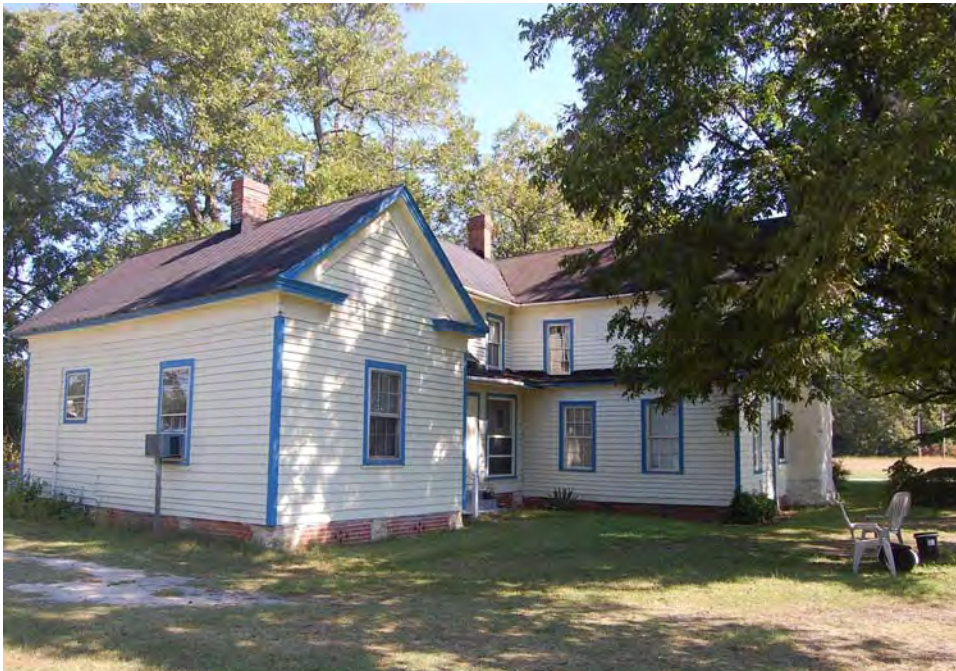
Plate 263. W. A. Gowers Farm, House, Rear (West) Elevations and Kitchen, Looking Northeast.
