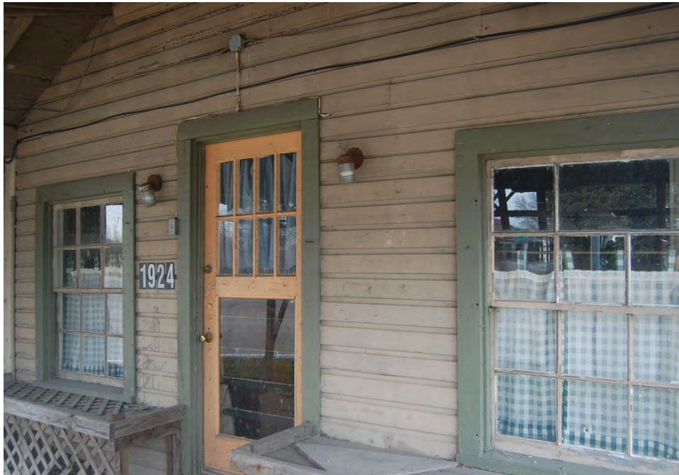
Plate 574. Thomas Store, Front Entrance.
