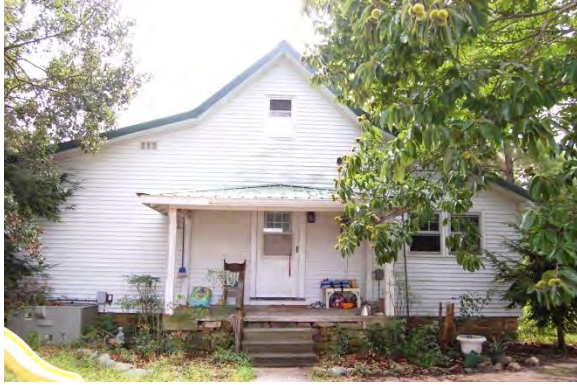
No. 67 Parrish House (PIN 1618319764), 10341 Jordan Road, Garner Vicinity, Wake County
