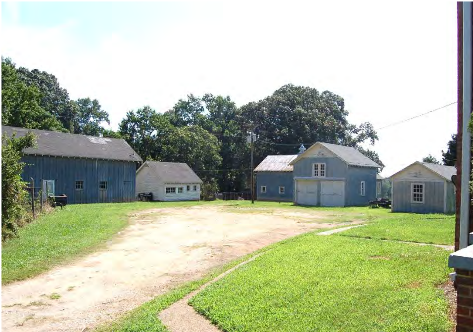
Plate 404. Dr. L. J. Faulhaber Farm, Farm Complex Northeast of House, Looking Northeast.
