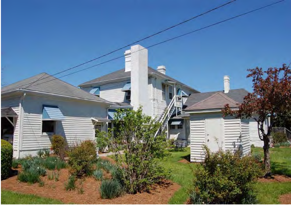
Plate 246. Richard Burnette House, Rear (East) Elevation, South Dependency (Garage), and Power Plant, Looking North.
