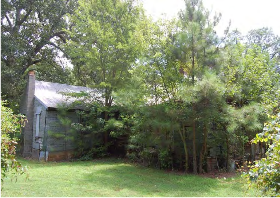
Plate 15. Wes Jones Farm, House, Rear Ell, Looking Northeast.
