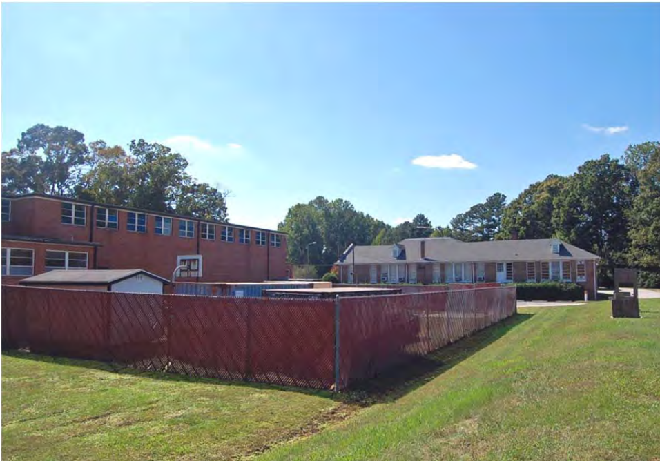
Plate 293. Mount Auburn School, Gymnasium, Rear Elevation, Looking West towards School.
