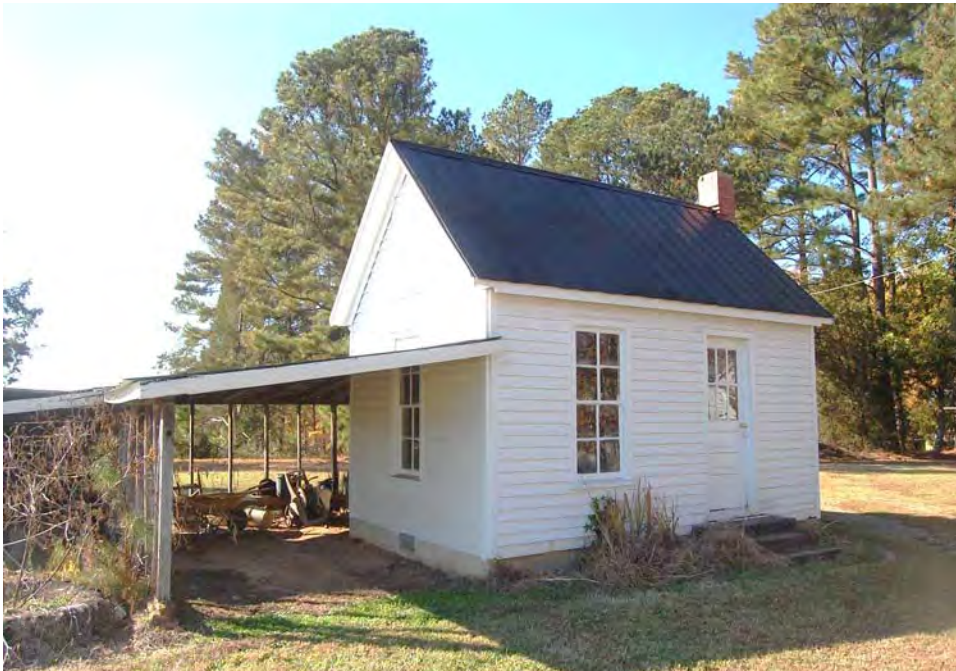
Plate 50. C. B. Sorrell House, Storage Building, Looking West.
