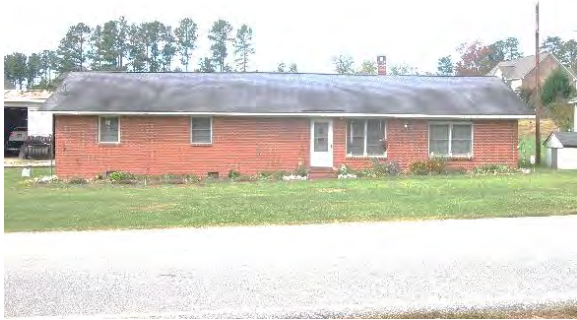
No. 245 House (PIN 1720102449), 7950 Bryan Road, Garner Vicinity, Wake County
