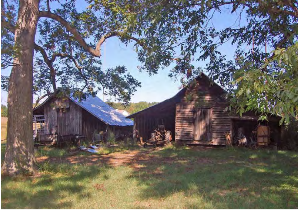
Plate 268. W. A. Gowers Farm, Fertilizer Shed and Corncrib, Looking North.
