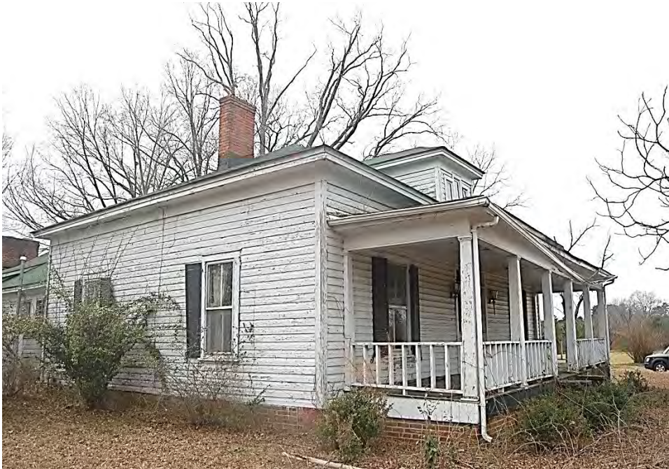
Plate 582. James Sugg House, Façade and Side (East) Elevation, Looking West.
