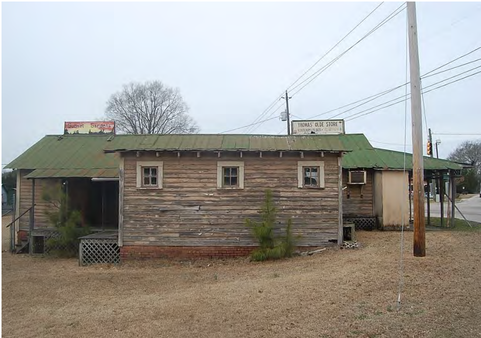
Plate 572. Thomas Store, Side (Southeast) Elevation and Rear Ell, Looking Northwest.
