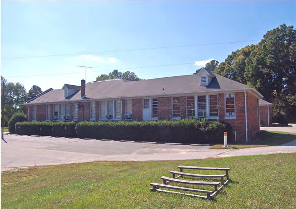
Plate 288. Mount Auburn School, East Elevation, Looking West from Gymnasium.
