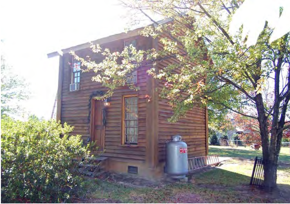
Plate 185. Juniper Level, House, 9114 Sauls Road, Modern Other House, Looking West.
