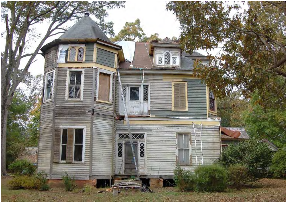
Plate 595. Atkinson-Whitted House, Front (East) Elevation, Looking West.
