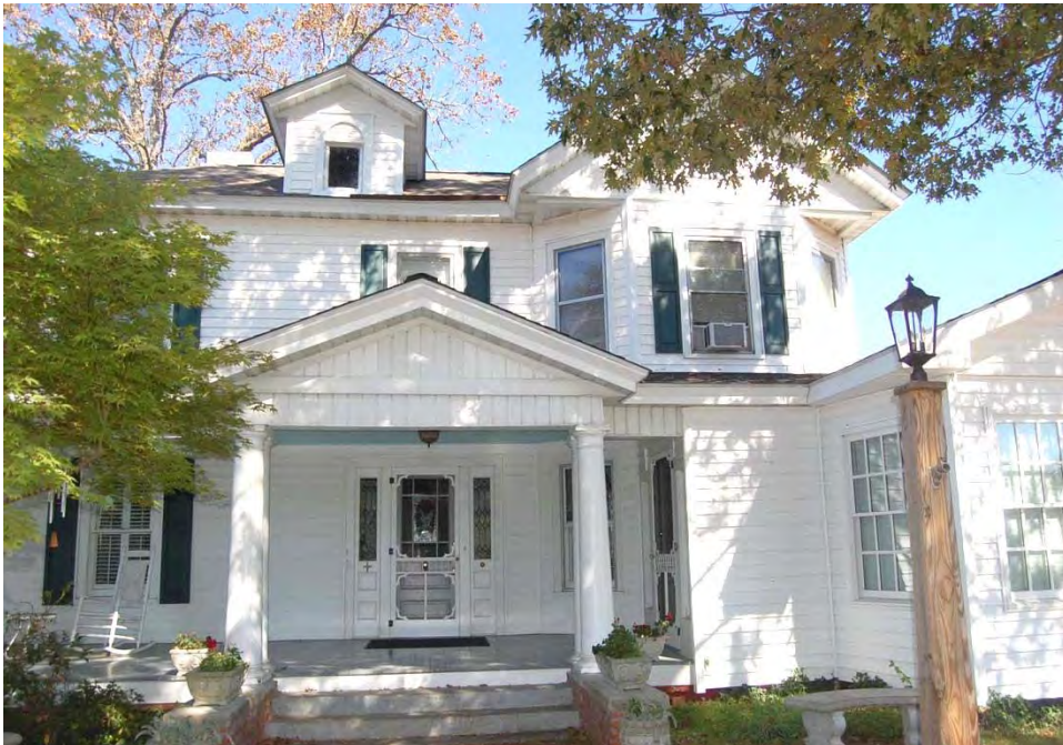
Plate 300. Icana Poole House, Entrance, Looking North.
