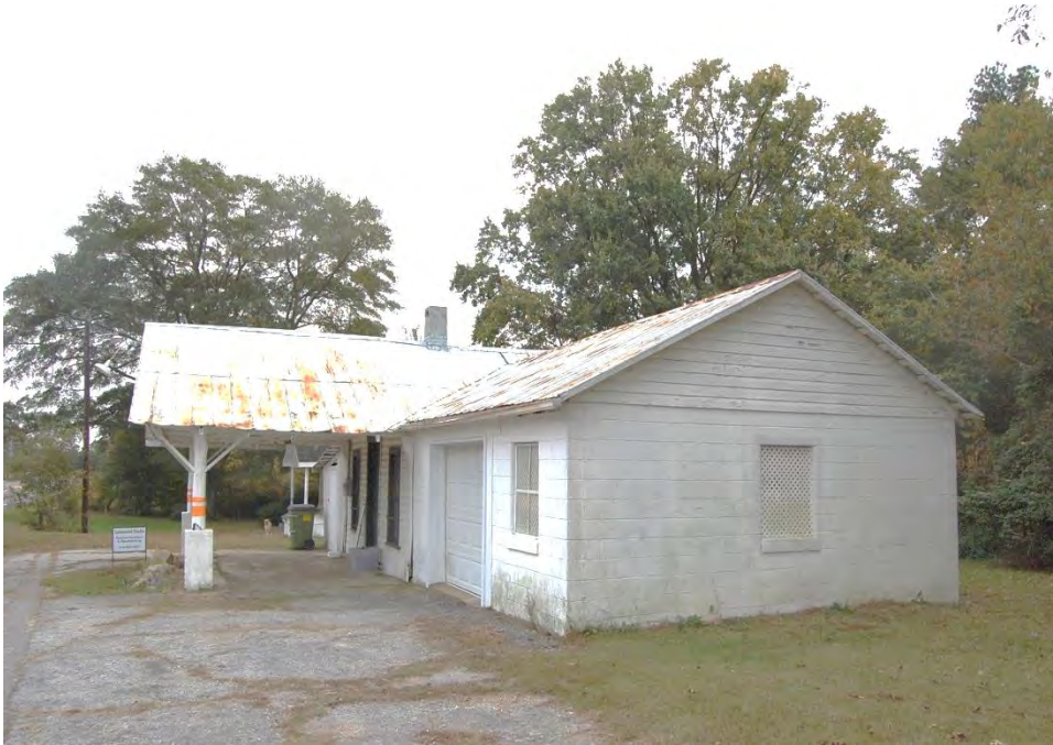
Plate 672. Weathers Store, 1950s Garage Addition, Looking South.
