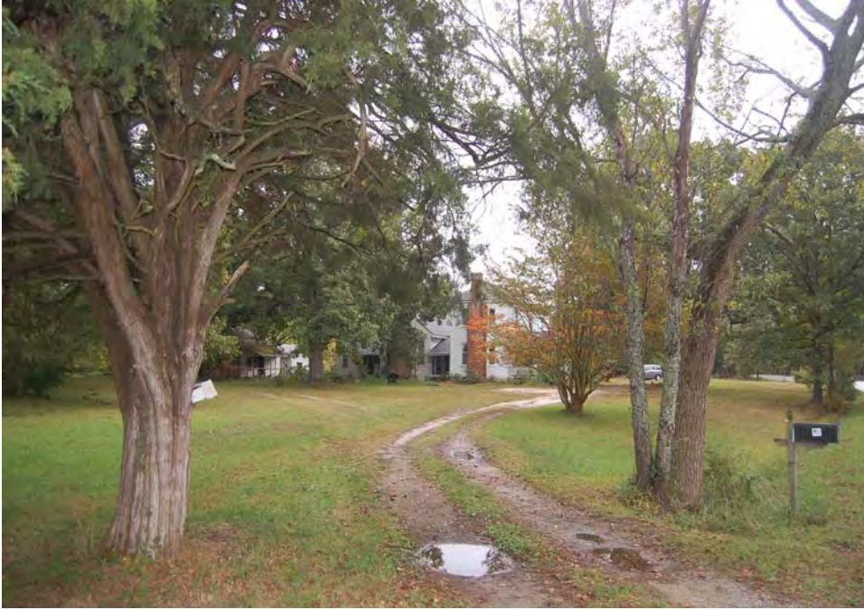
Plate 335. Baucom-Stallings House, House and Setting, Looking Northeast.
