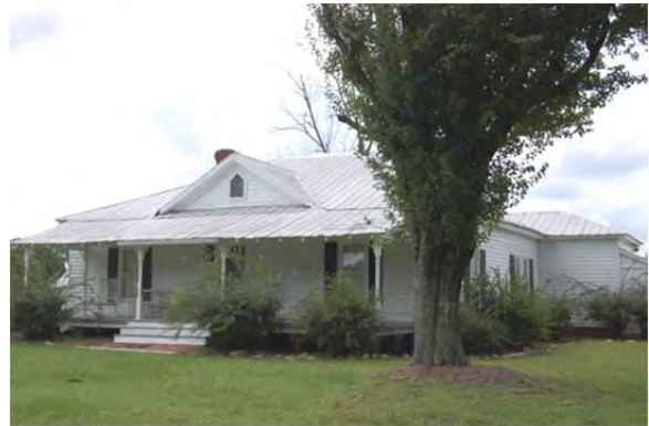
No. 60 Carroll House (WA0256) (PIN 1618113674), 10400 Jordan Road, Garner Vicinity, Wake County
