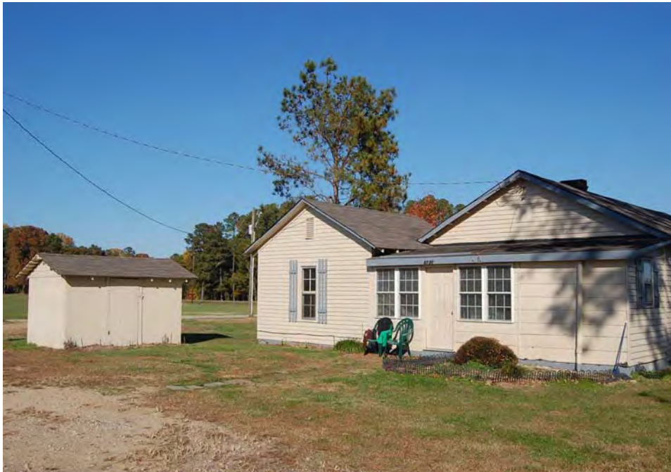
Plate 28. Pierce Farm, Pierce House, Rear Elevation and Pump House, Looking Northeast.
