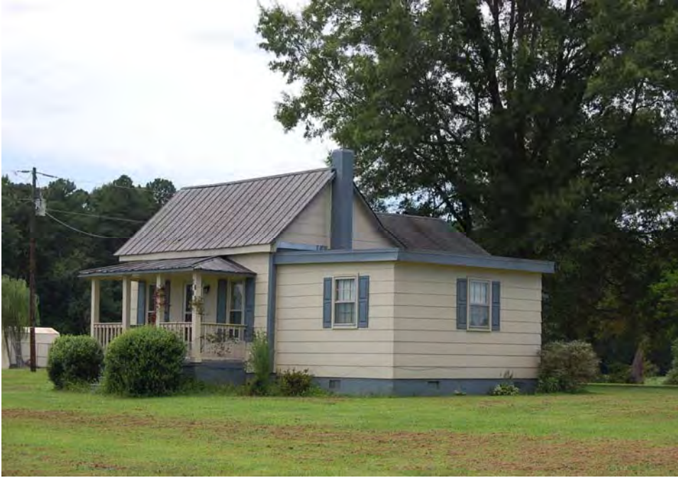
Plate 23. Pierce Farm, Relocated Nineteenth-Century House, Looking Southwest.
