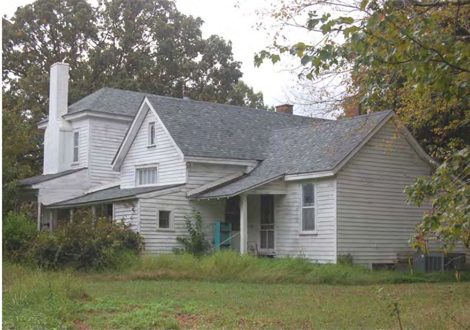
Plate 341. Baucom-Stallings House, Original House, Rear Addition, and Rear Elevation of Main House, Looking South.
