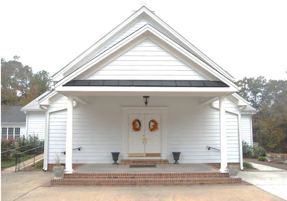
Plate 641. Plymouth Christian Church, Modern Portico and Entrance, Looking West.
