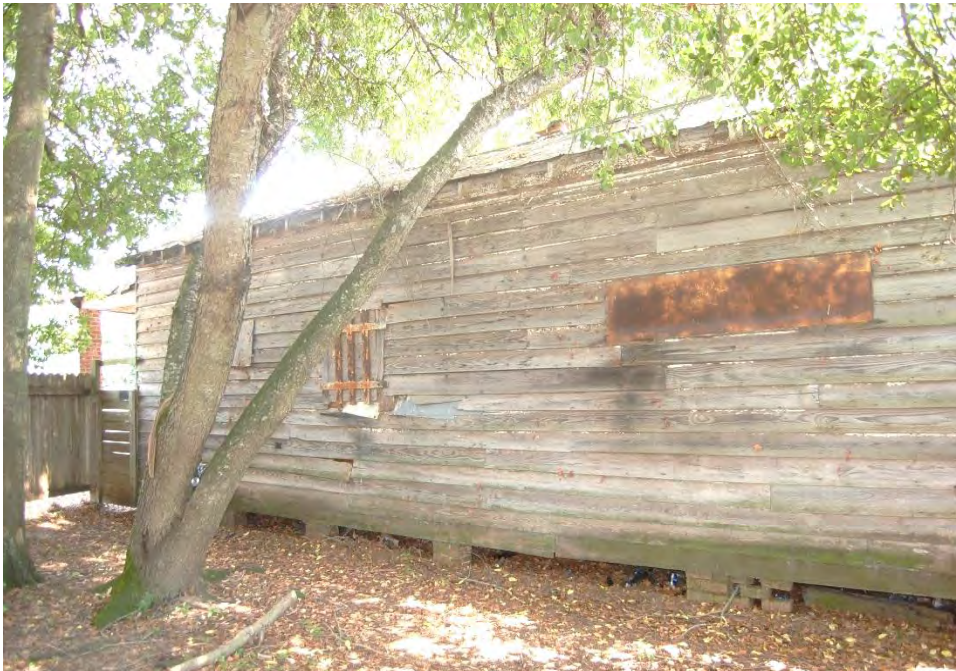
Plate 559. Britt's Store, Side (North) Elevation, Looking South.
