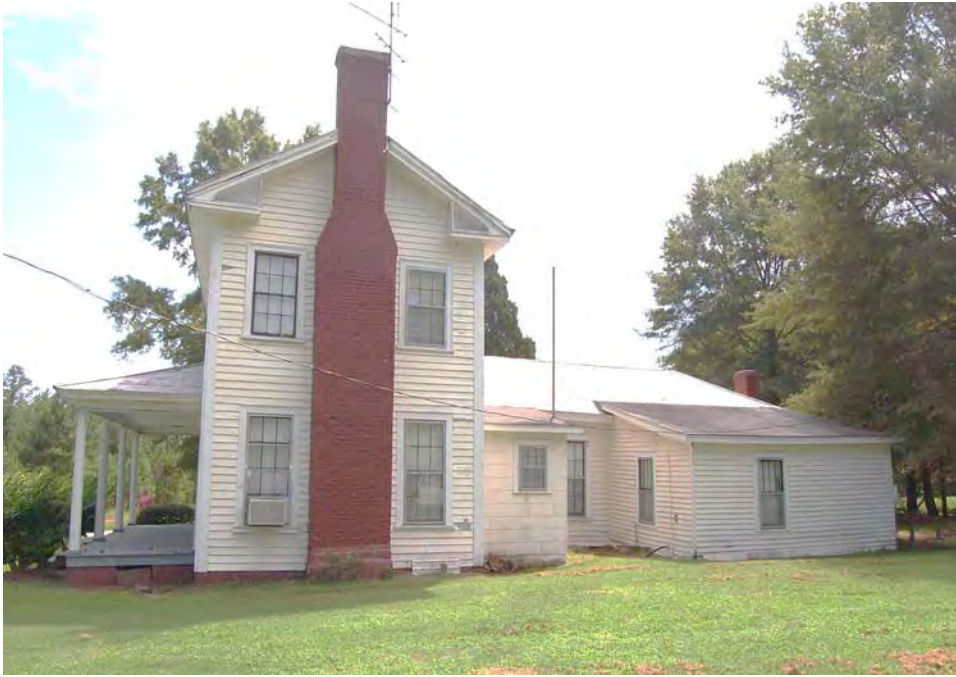
Plate 91. John B. Strain House, Side (North) Elevation, Looking South
