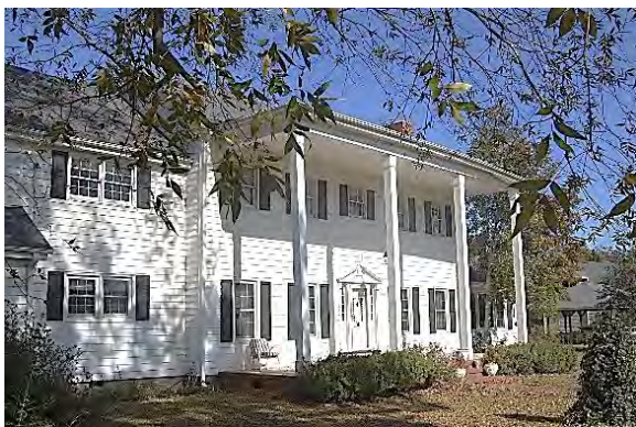
No. 309 House (PIN 162700-47-1501), 13380 Cleveland School Road, Garner Vicinity, Johnston County
