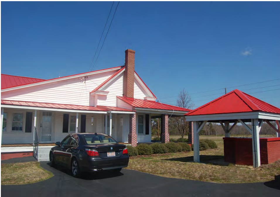
Plate 636. Joseph M. Blalock Farm, Well and House, Side (South) Elevation, Looking Northeast.
