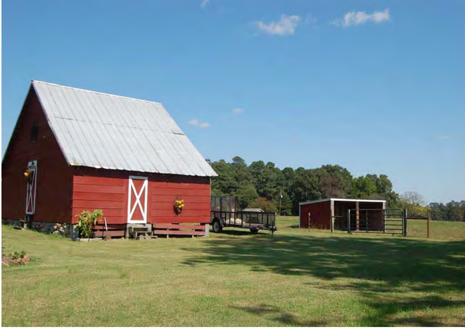
Plate 240. Umstead Farm, Penny-Alston Tract, Modern Outbuildings, Looking North.
