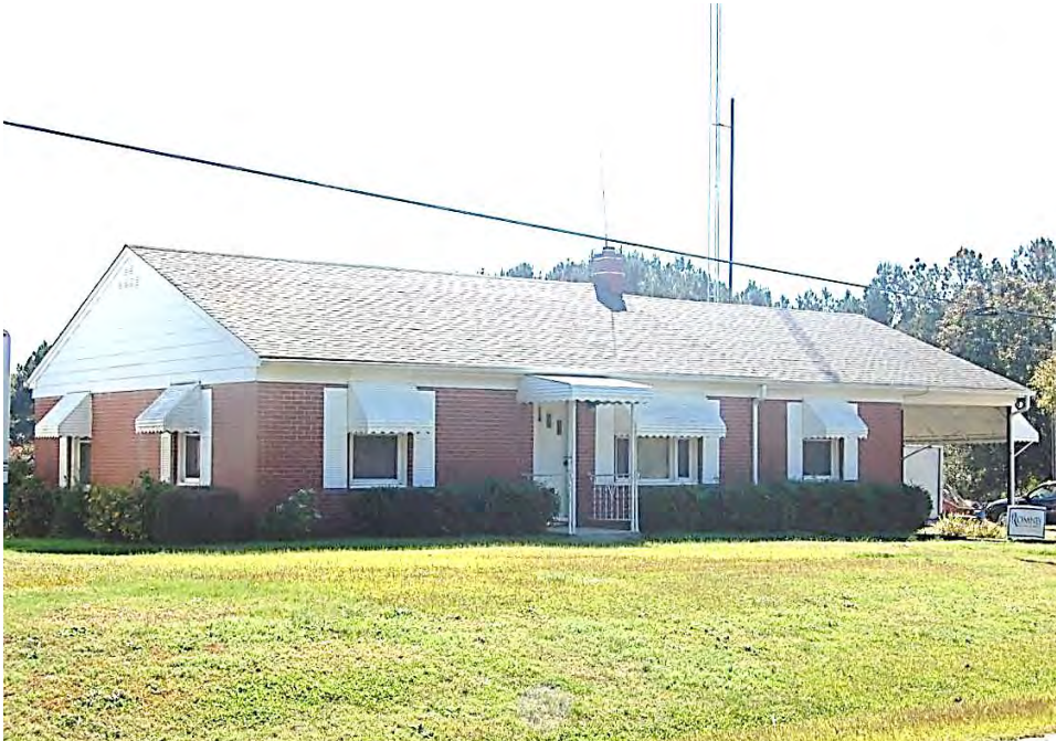
Plate 546. Auburn, House (No. 277), Looking South.
