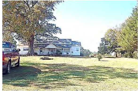
No. 295 House (PIN 0698755017), 5128 Rock Service Station Road, Garner Vicinity, Wake County
