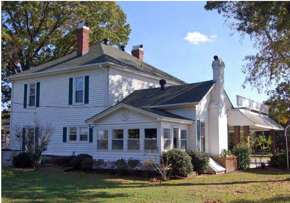
Plate 169. Samuel Jefferson Rhodes House, Side (North) Elevation, Rear Wing, and Additions, Looking Southeast.
