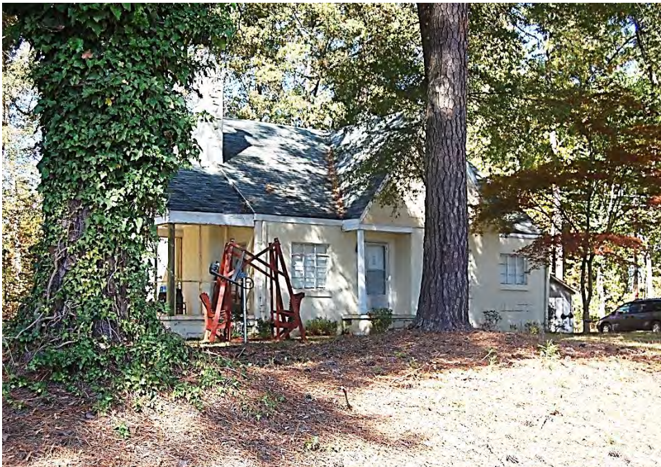
Plate 418. Willis House and Store, House, Façade, Looking West.
