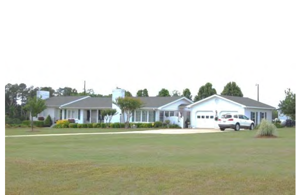
No. 179 House (PIN 1743667809), 4716 Old Faison Road, Garner Vicinity, Wake County
