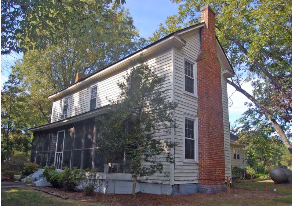
Plate 484. David Lewis House, Façade, Looking Northwest from White Oak Road.
