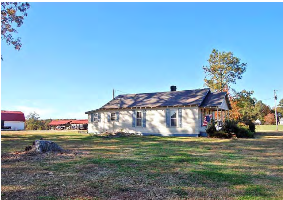
Plate 26. Pierce Farm, Pierce House, Looking North.
