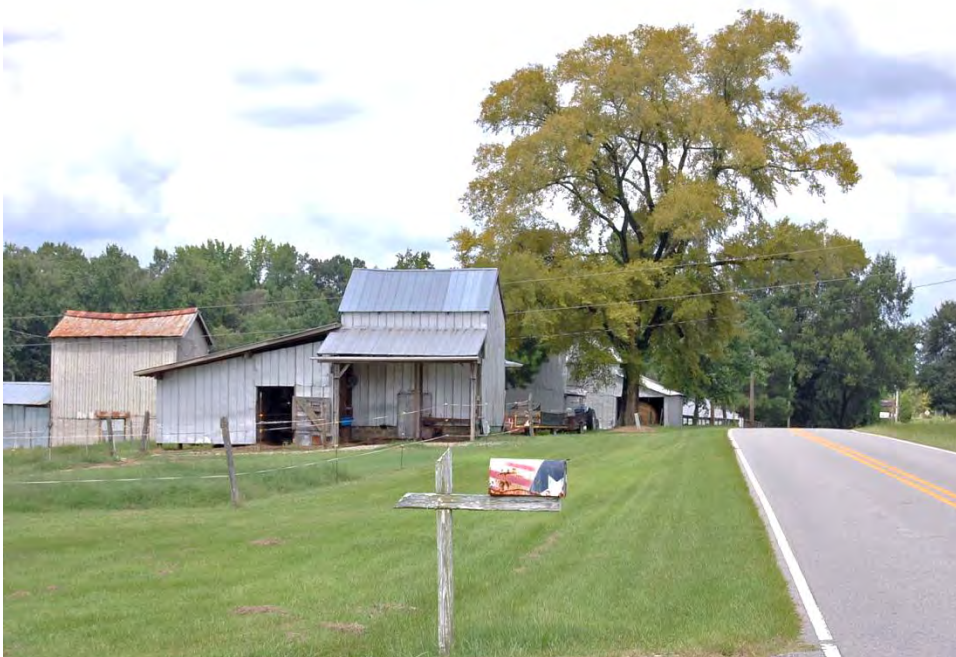
Plate 217. Jones Family Farm, Outbuildings on West Side of Jordan Road, Looking North.
