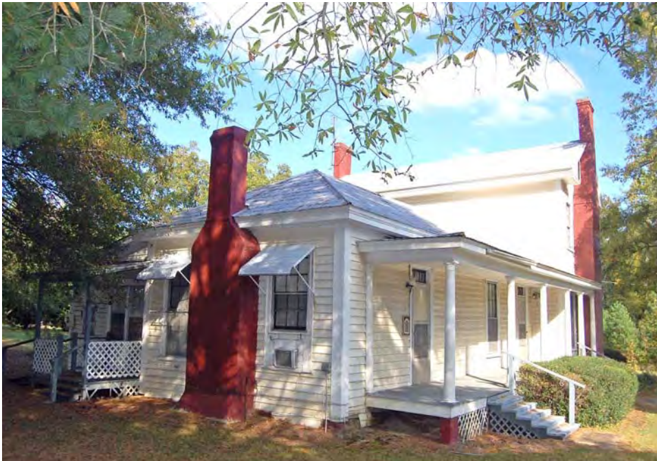
Plate 94. John B. Strain House, Rear Elevation, Looking East.
