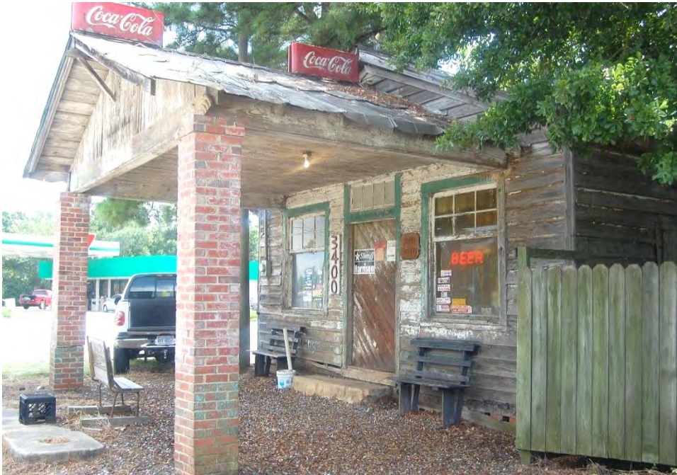
Plate 557. Britt's Store, Pump Canopy and Façade, Looking South towards Ten Ten Road.
