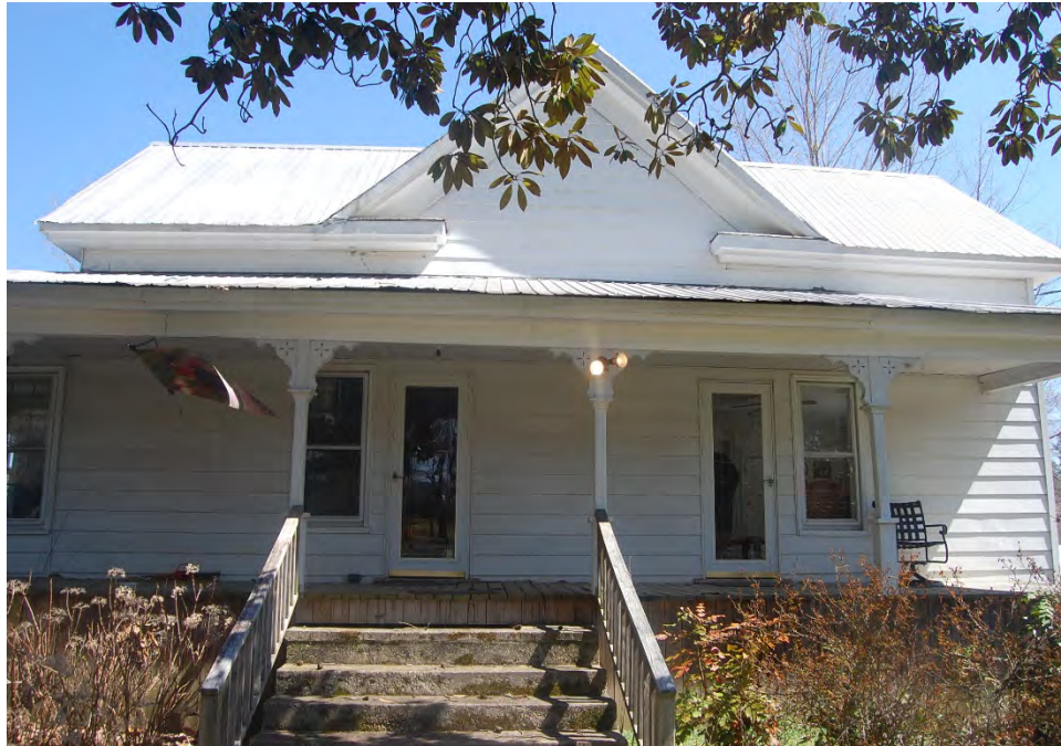
Plate 662. Jim Jordan Farm Complex, House, Façade (West Elevation), Looking Northeast.
