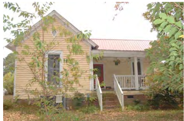
No. 322 Bennett House (WA1121) (PIN 0687010968), 6987 Kennebec Road, Willow Springs, Wake County
