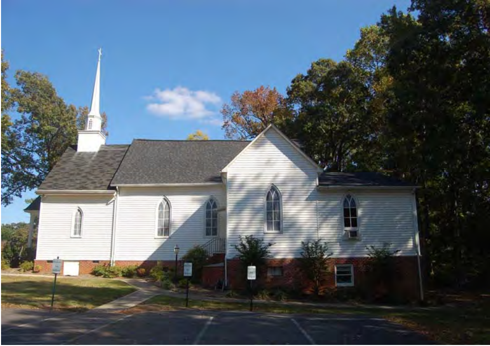
Plate 101. Wentworth Christian Church, Side (West) Elevation, Looking East.
