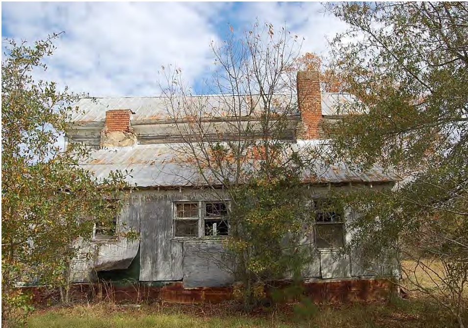
Plate 651. Jones-Ellington House, Rear Shed, Looking East.
