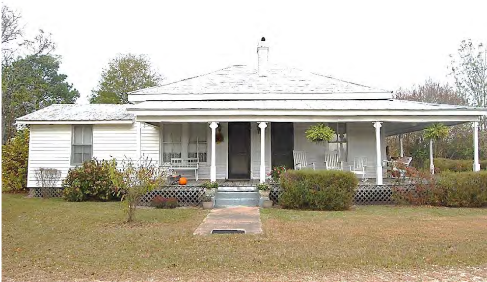
Plate 621. Grady Rowland House, Façade (South Elevation), Looking North.
