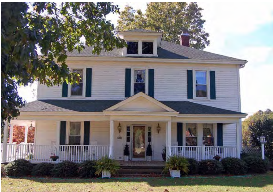
Plate 167. Samuel Jefferson Rhodes House, Façade, Looking West.
