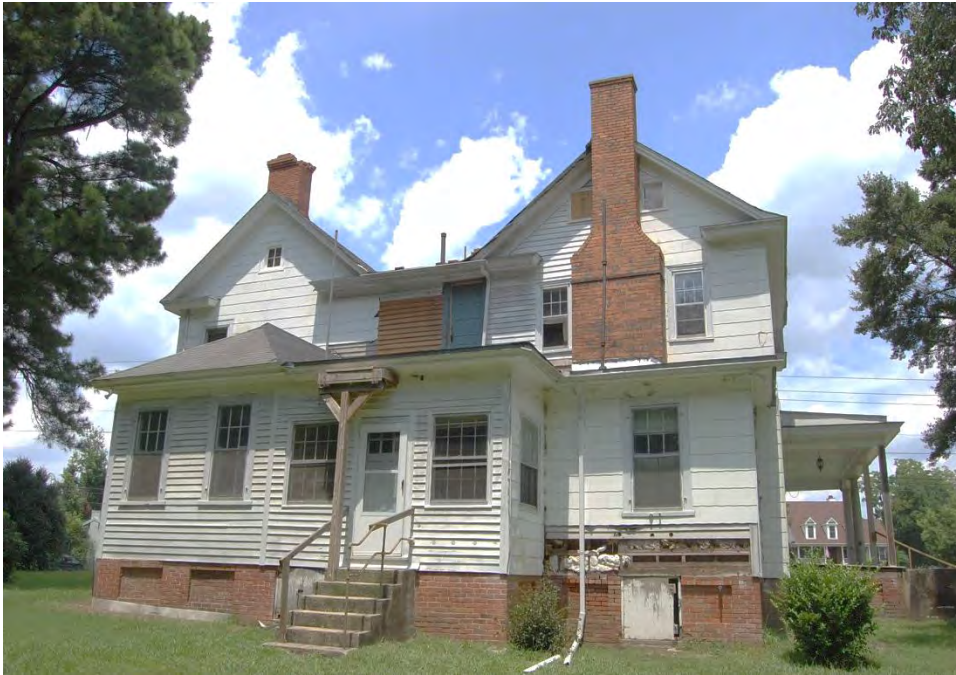
Plate 505. Johns-Lane-Poole House, Rear (South) Elevation, Looking North.
