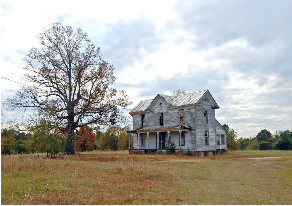
Plate 646. Jones-Ellington House, House and Setting, Looking West.
