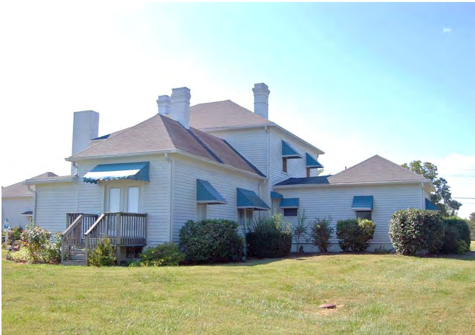
Plate 247. Richard Burnette House, Rear (East) Elevation, Rear Ell, and North Dependency, Looking West.
