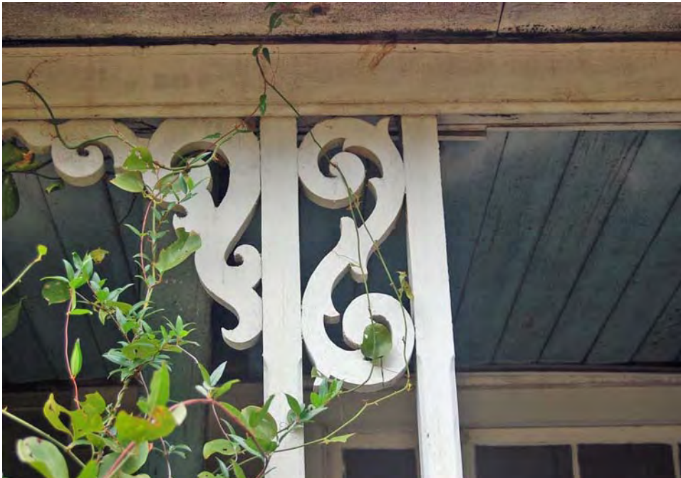
Plate 321. Penny House, Porch Detail, Looking East.
