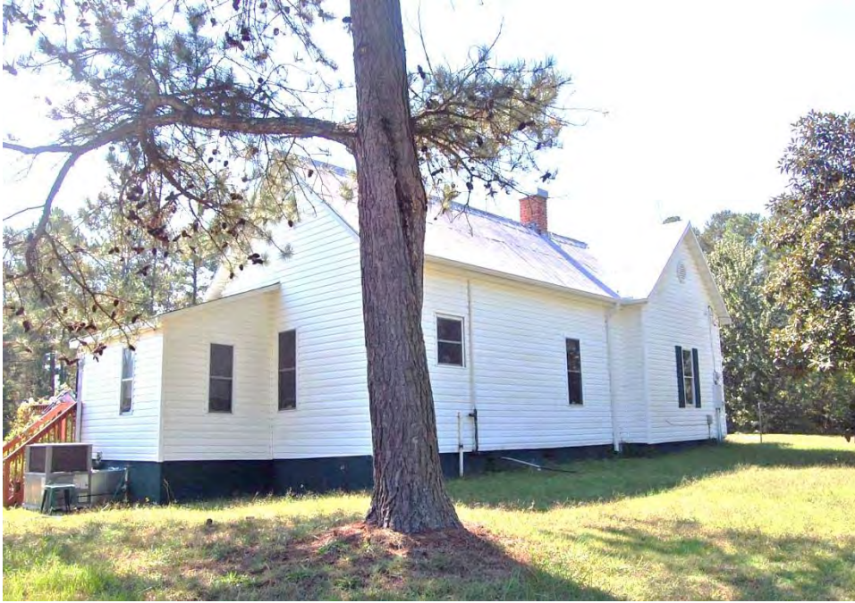
Plate 258. John Williams Farm, House, Rear and Side (North) Elevations, Looking Southwest.
