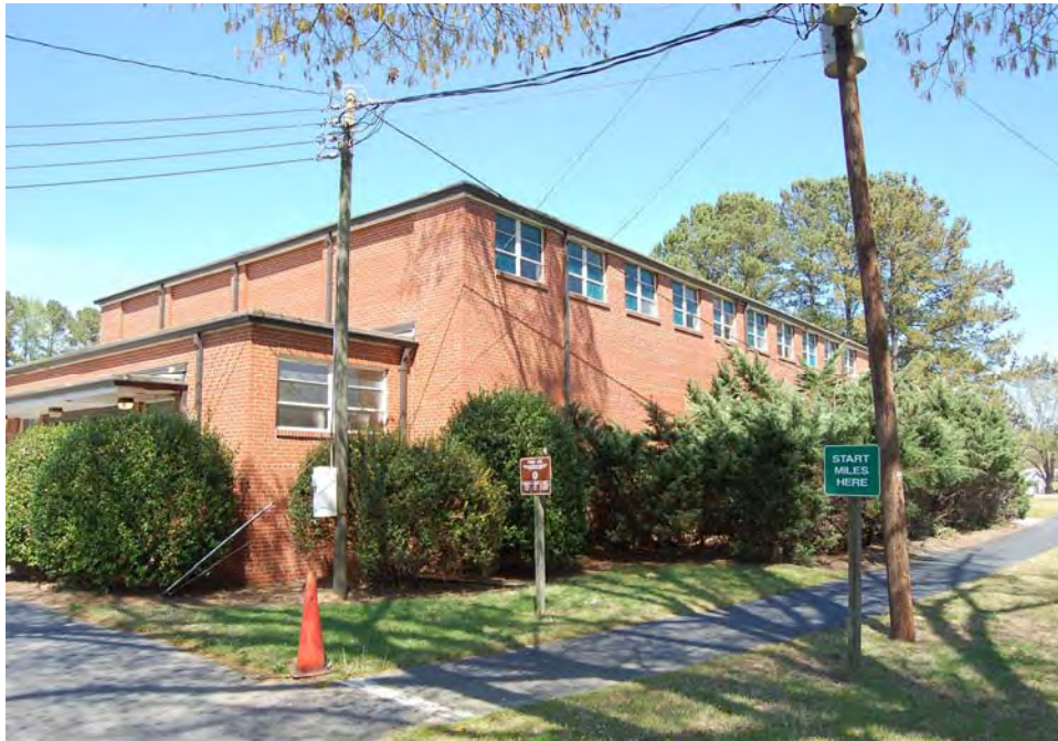
Plate 291. Mount Auburn School, Gymnasium, Looking Northeast.
