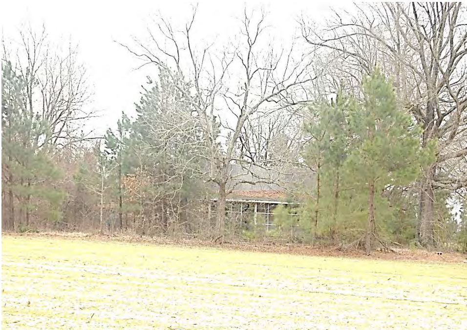
Plate 594. James Sugg House, Deteriorated Tenant House on Overgrown Site West of House, Looking South.
