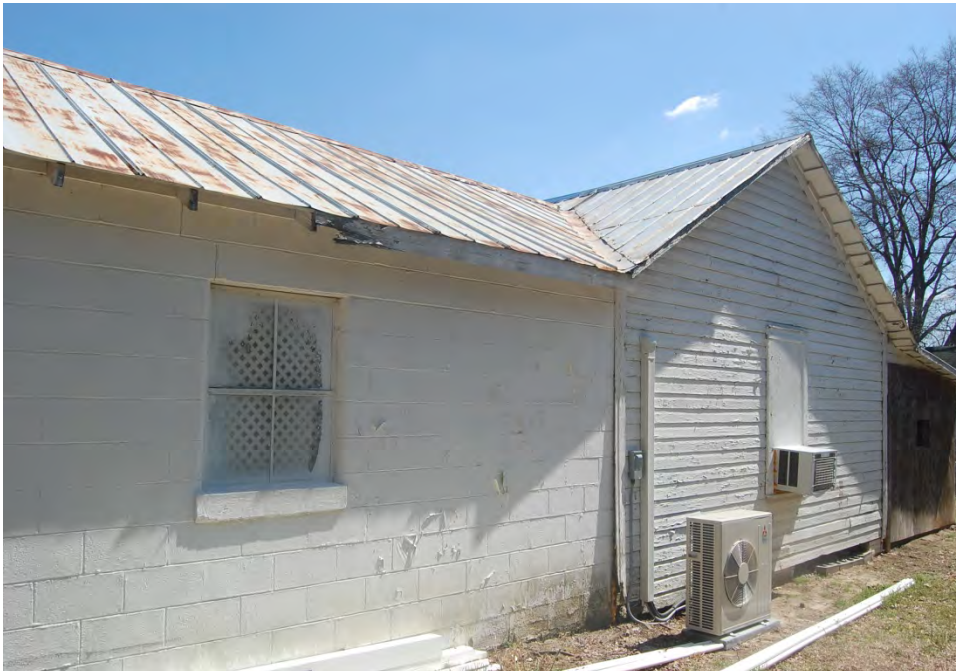
Plate 671. Weathers Store, Rear (West) Elevation, Looking South.
