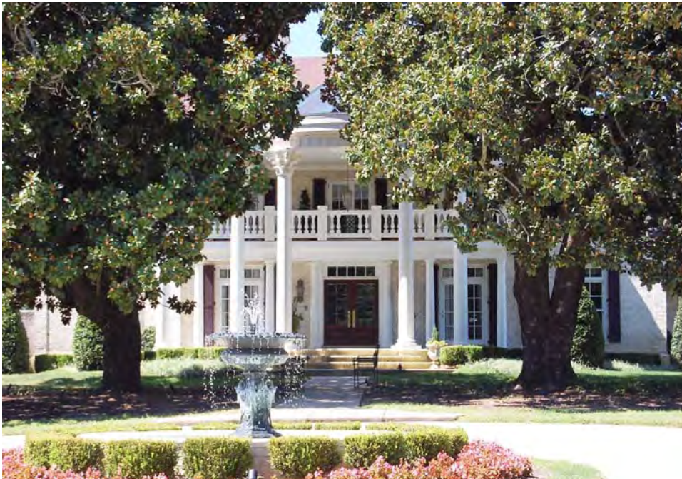
Plate 225. Ransom Penny House, Facade, Looking West.
