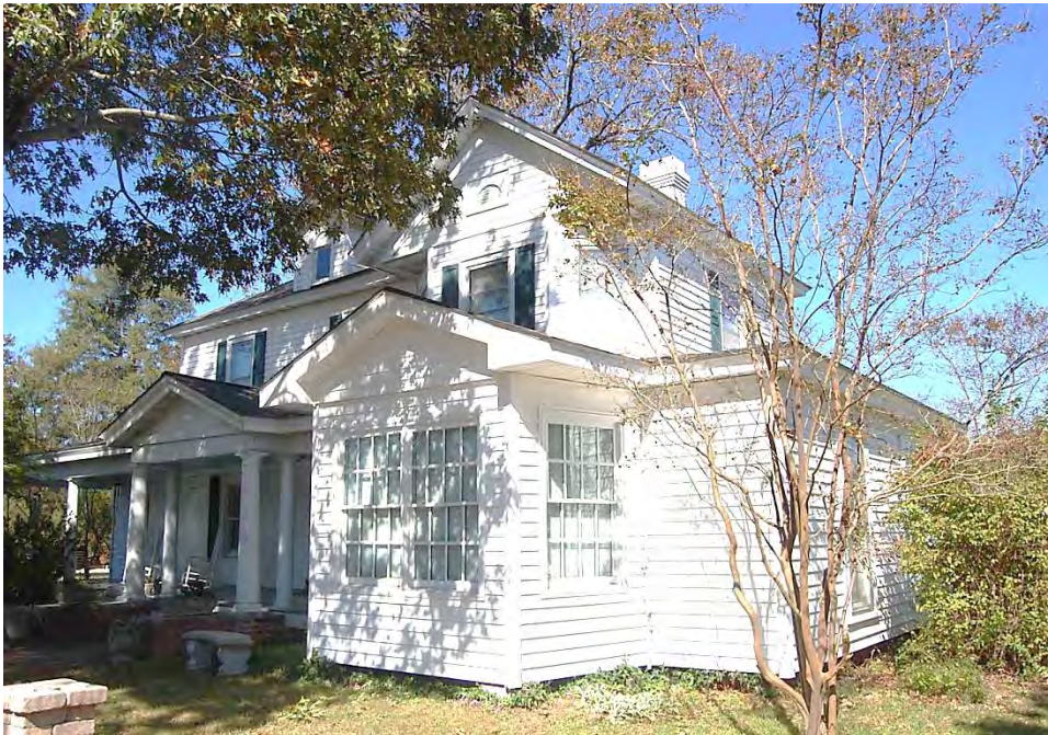
Plate 302. Icana Poole House, Enclosed Porch, East Elevation, Looking Northwest.
