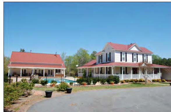
No. 98 House (PIN 1639362540), 2200 Guy Road, Garner Vicinity, Johnston County
