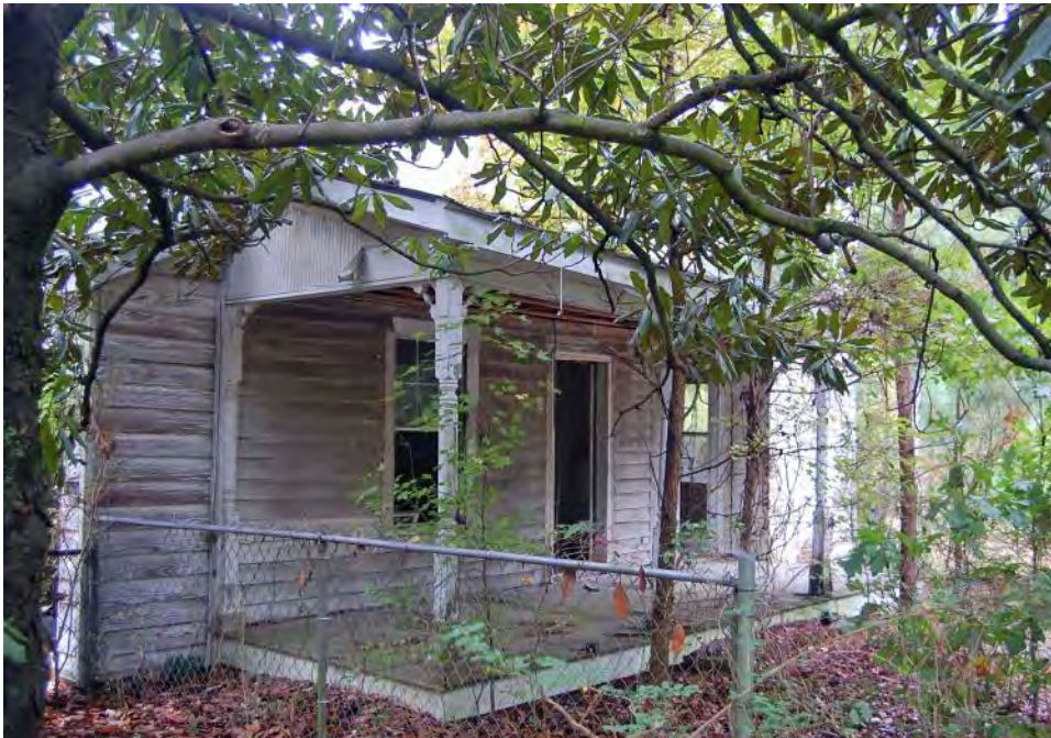
Plate 323. Penny House, Porch, North Elevation of Rear Ell, Looking Southwest.
