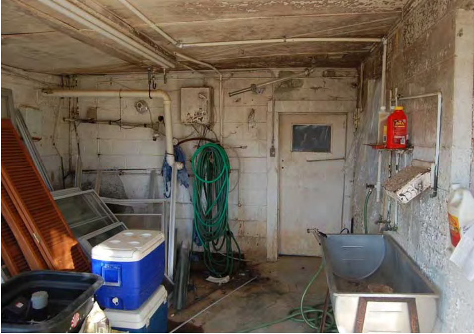
Plate 31. Pierce Farm, Dairy Barn, Equipment Room.
