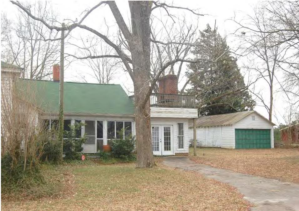
Plate 589. James Sugg House, Rear Ell and Garage, Looking Southeast.
