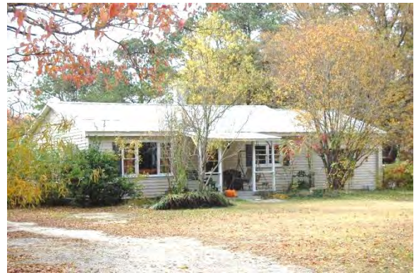
No.193 House (PIN 1629804007), 2420 New Bethel Church Road, Garner Vicinity, Wake County
