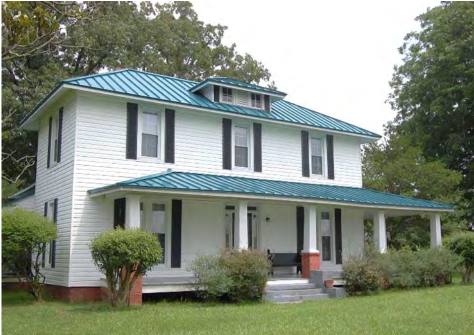
Plate 150. George Williams Farm, House, Looking Southeast.
