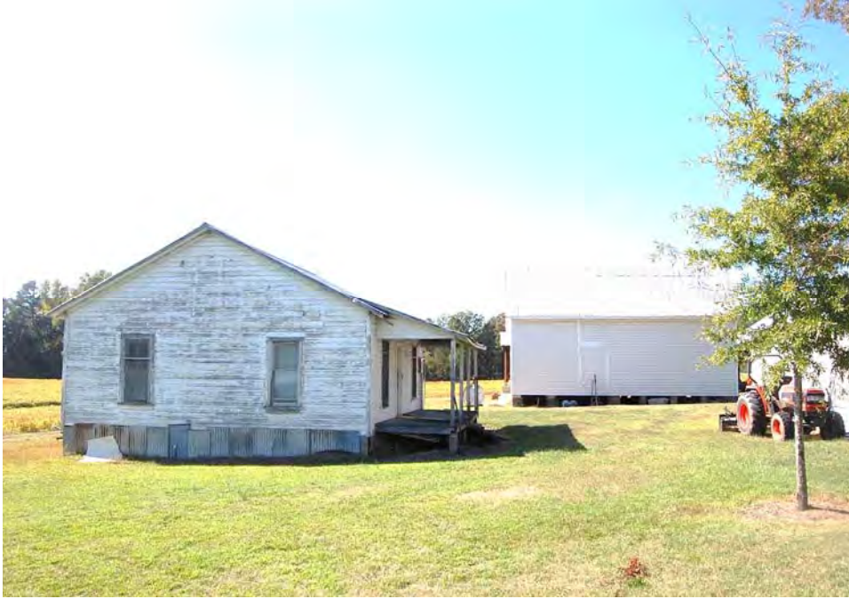
Plate 126. Percy and Mynette Strother House, Tenant House and Packhouse, Looking West.
