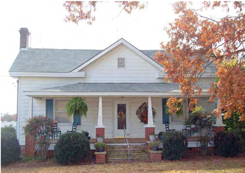
Plate 54. Bell-Pierce Farm, Eastern Tract, Bell-Pierce House, Looking South.
