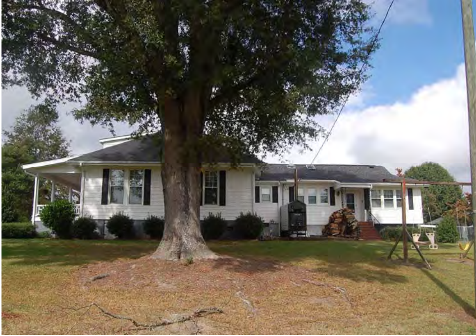
Plate 316. Mount Moriah Academy, Side (South) Elevation, Looking North.
