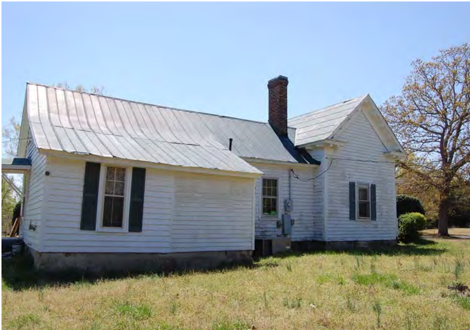
Plate 281. Gower-Johnson House, North Elevation and Rear Ell, Looking South.
