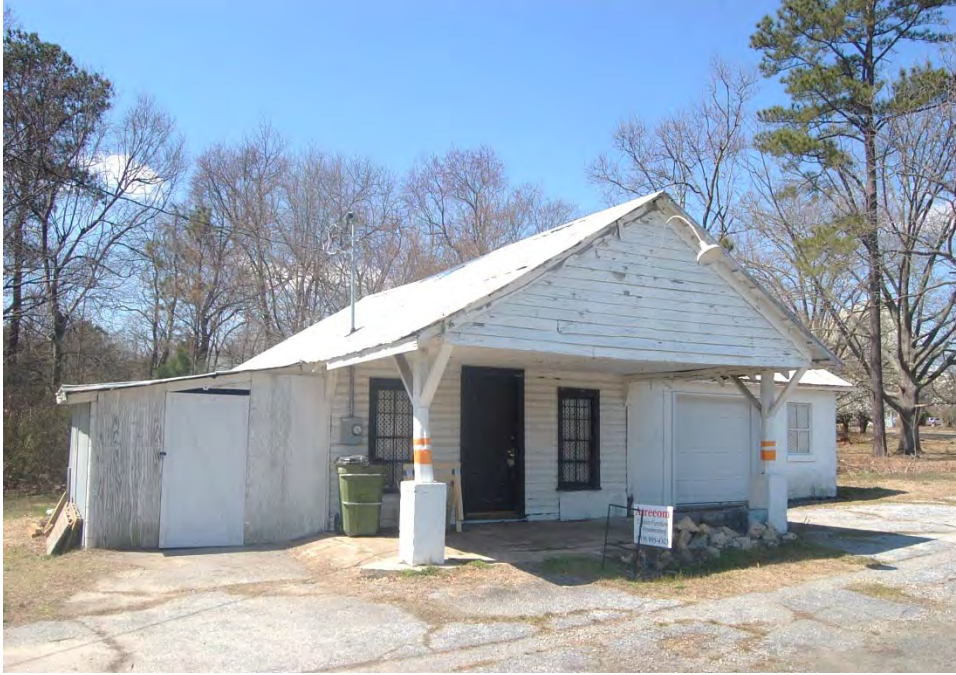
Plate 668. Weathers Store, Overall View, Looking Northwest.
