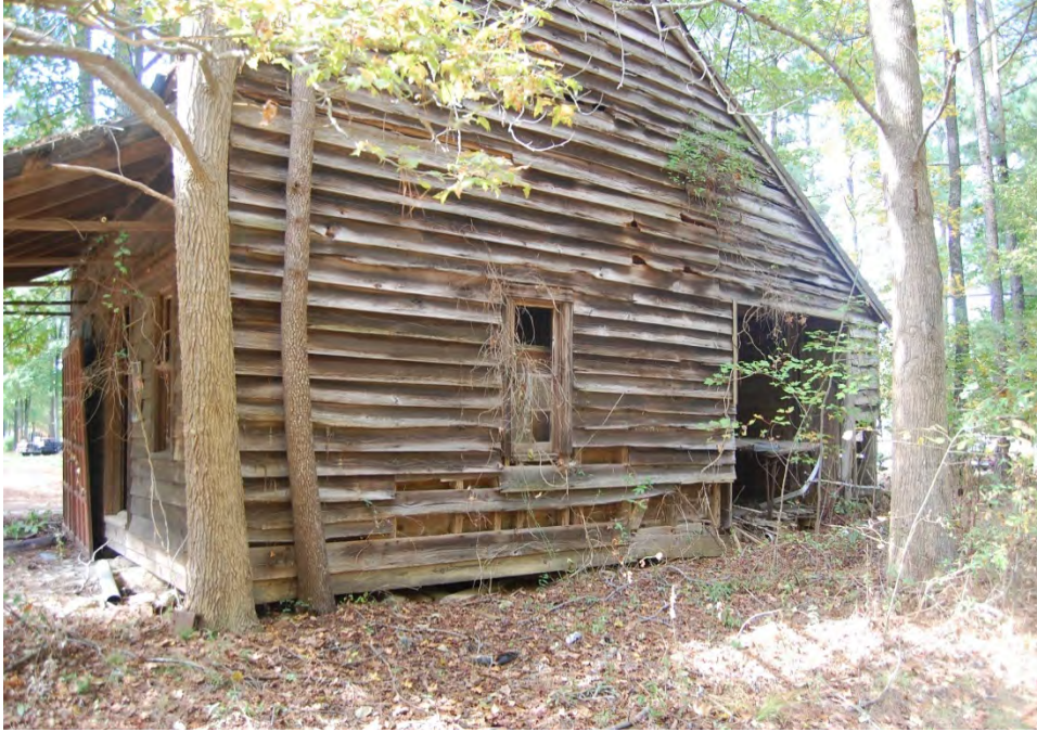
Plate 470. Lewis House, Side (East) Elevation, Looking West.
