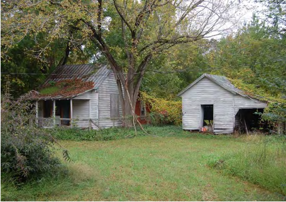
Plate 343. Baucom-Stallings House, Original Kitchen and Smokehouse, Looking North.
