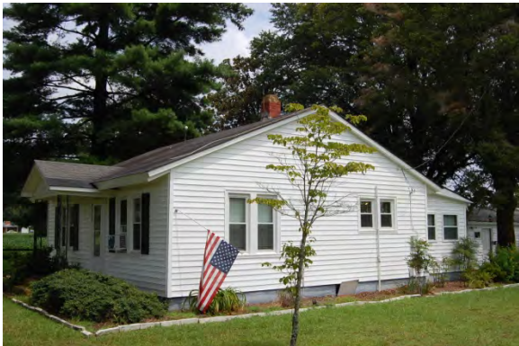
Nos. 39-40 Russell-McGee Complex (WA2450) (PINs 0699805778 and 0699804698), 9317-9321 Old Stage Road, Williams Crossroads Vicinity, Wake County
