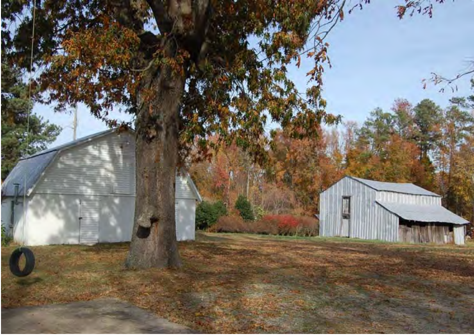
Plate 154. George Williams Farm, Gambrel-Roofed Workshop (Left) and Packhouse (Right), Looking Northeast.
