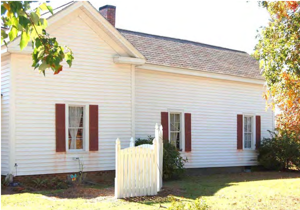
Plate 182. Juniper Level, House, 9114 Sauls Road, Side (North) Elevation, Looking Southwest.
