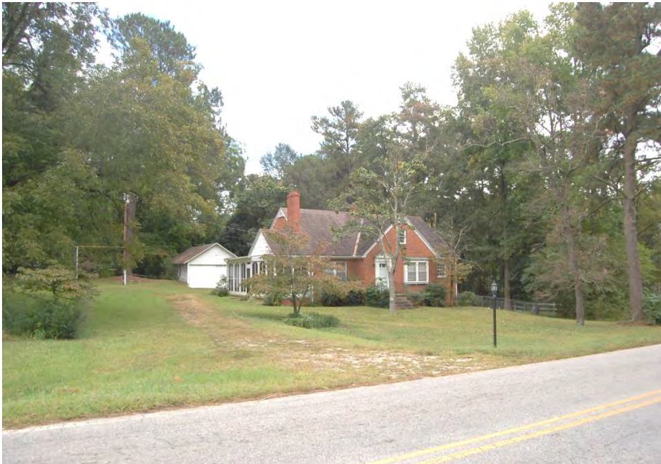
Plate 534. Leland and Addy Poole House (No. 270), Looking Southeast.
