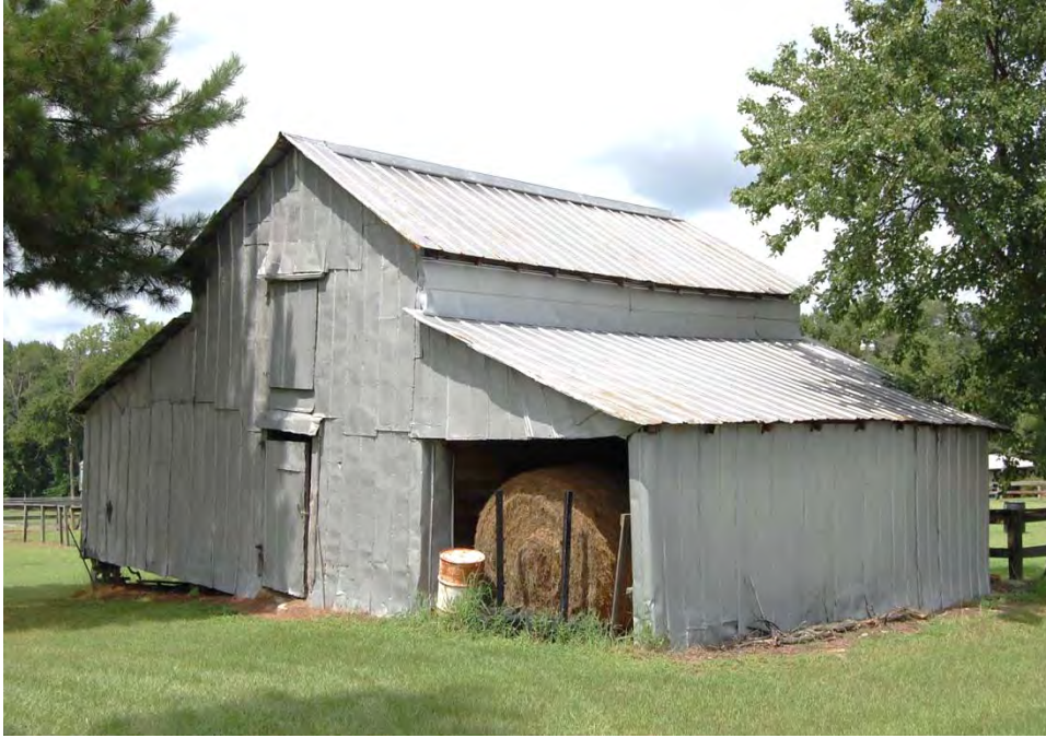
Plate 216. Jones Family Farm, Packhouse on West Side of Jordan Road, Looking Northwest.
