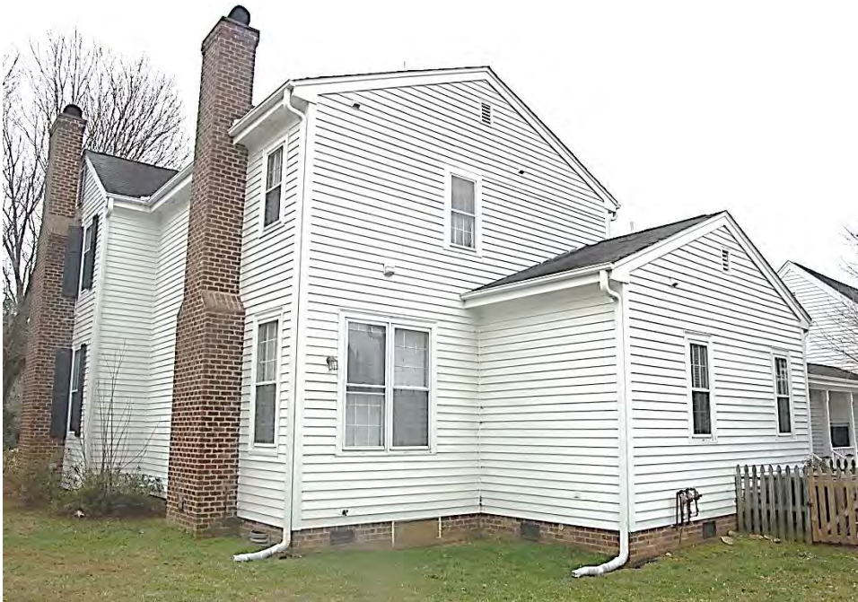
Plate 689. Burt-Utley House, Rear Ell with Additions, Looking Southwest. Looking East.
