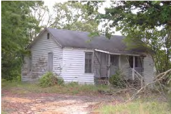
No. 159 House (PIN 1742261807), 3033 Hodge Road, Garner Vicinity, Wake County
