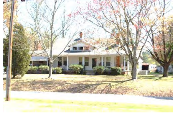
No. 114 House (WA0303) (PIN 1730660705), 2432 East Garner Road, Garner Vicinity, Wake County
