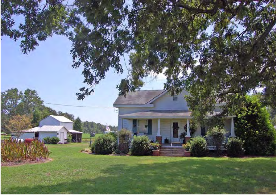
Plate 53. Bell-Pierce Farm, Eastern Tract, Bell-Pierce House and Outbuildings, Looking South.
