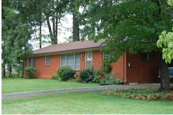
No. 27 House (PIN 0689825884), 8336 Old McCullers Road, Garner Vicinity, Wake County
