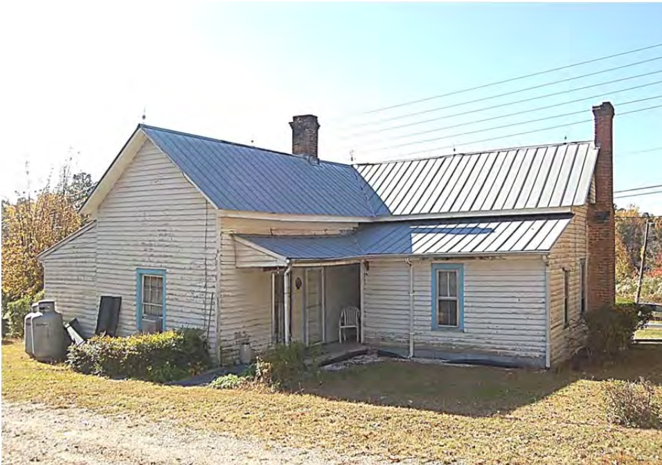
Plate 378. William Pierce House, Rear Ell, Looking West.
