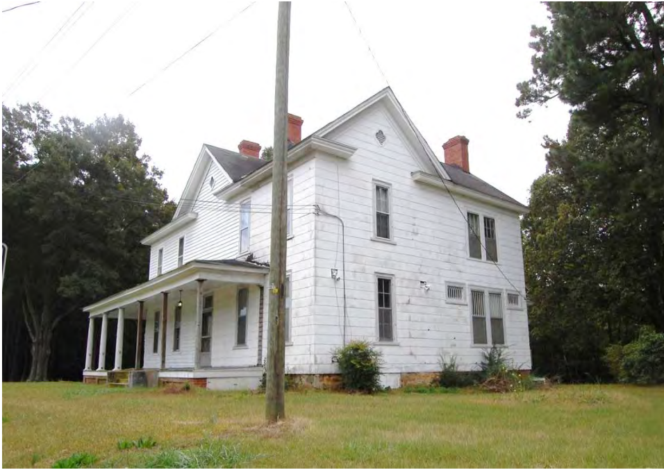
Plate 503. Johns-Lane-Poole House, Façade and Side (West) Elevation, Looking Southeast.
