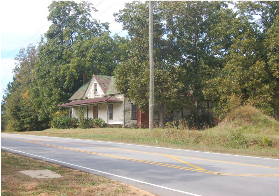
Plate 474. Yeargan House, House and Setting, Looking West along White Oak Road.
