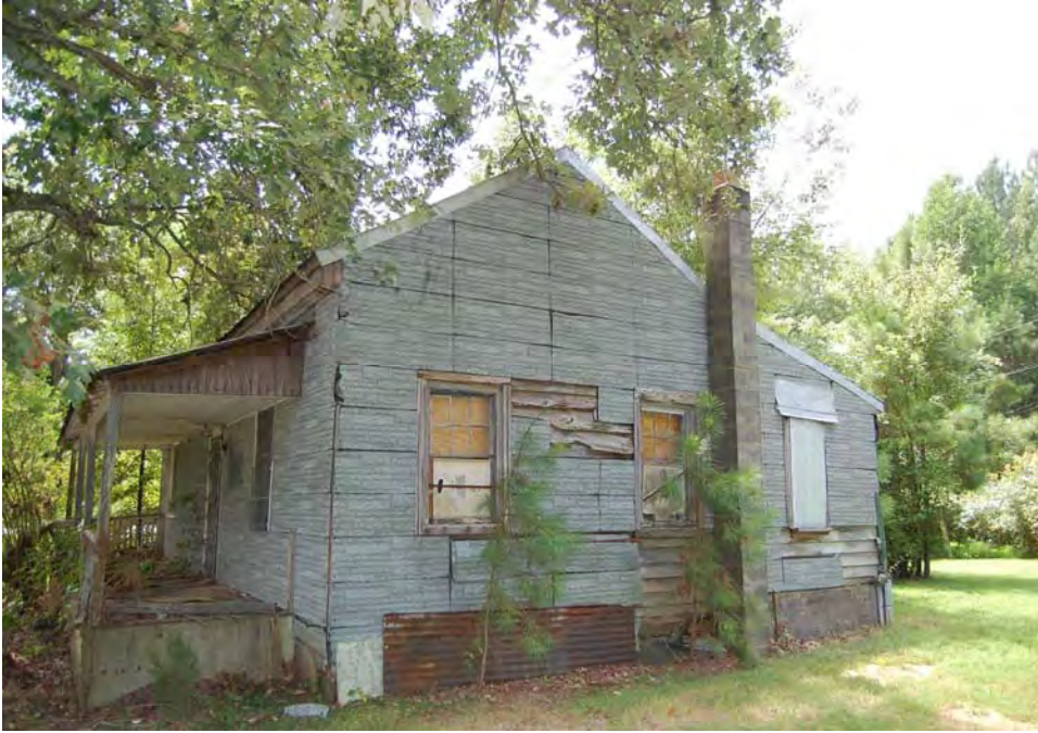
Plate 9. Wes Jones Farm, House, Side (North) Elevation, Looking South.
