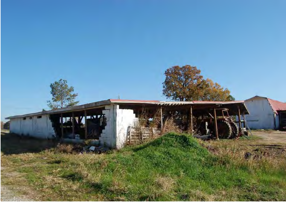
Plate 33. Pierce Farm, Former Chicken House/Equipment Storage Shed, Looking Southeast.
