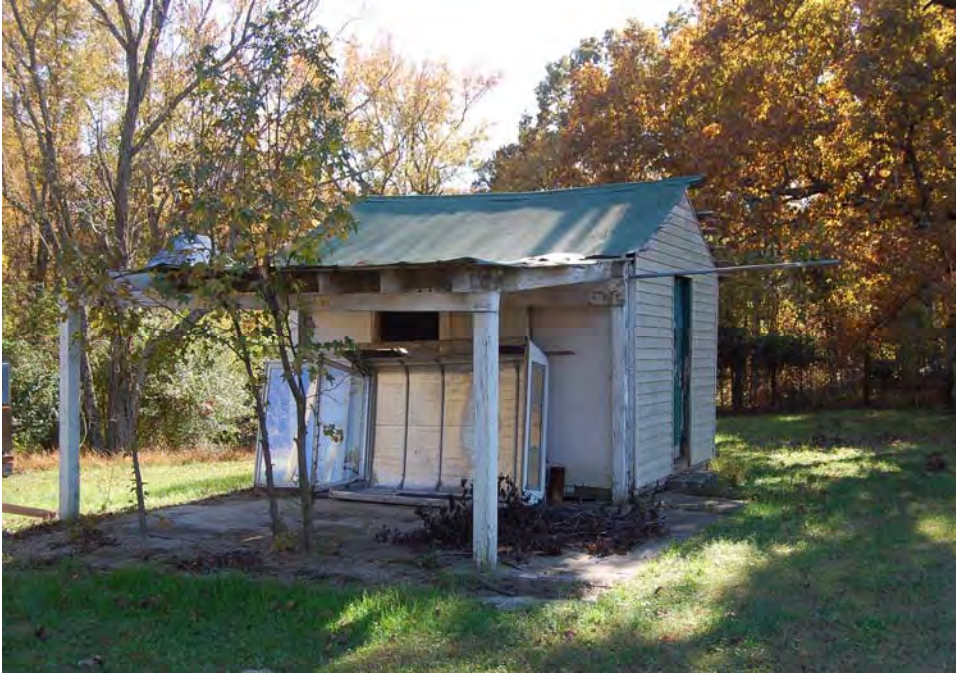
Plate 7. G. L. Pierce House, Storage Shed West of House, Looking South.
