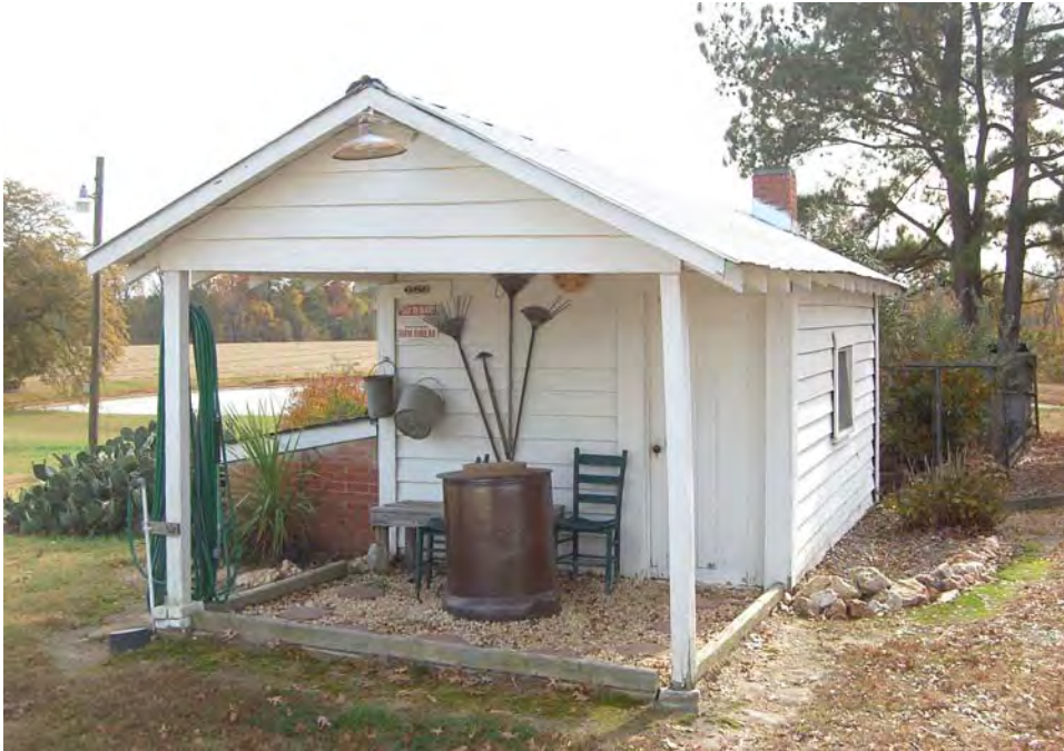
Plate 61. Bell-Pierce Farm, Eastern Tract, Washhouse (Chicken Sheds to the Rear), Looking South.
