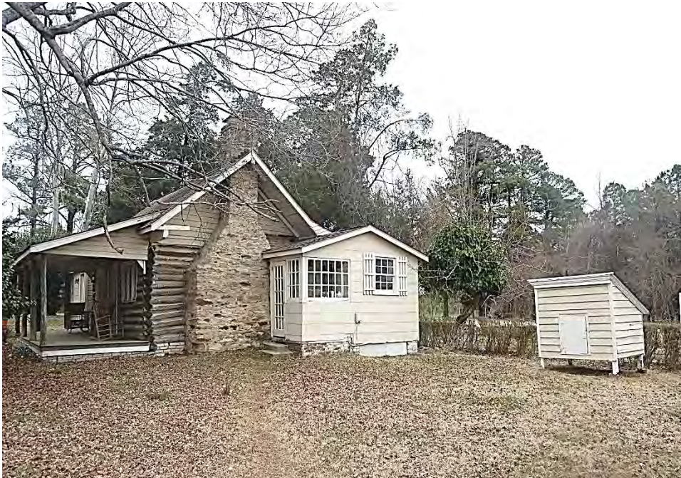
Plate 609. Jones-Johnson Farm, Log House and Ice House, Looking Northeast.
