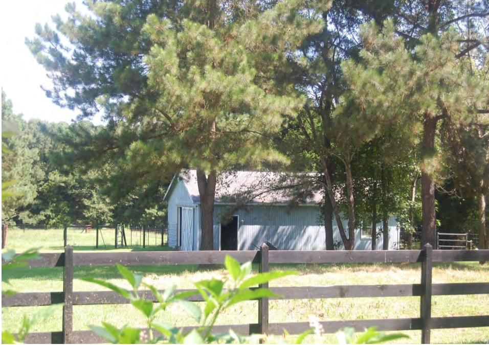
Plate 490. David Lewis House, Modern Horse Barn, Looking North.
