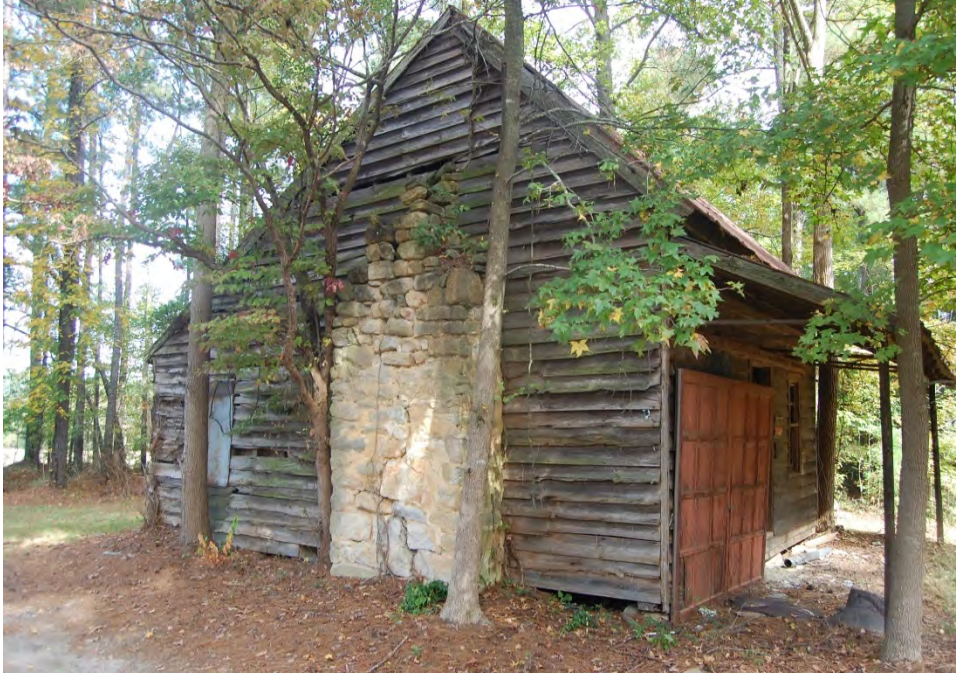
Plate 468. Lewis House, Side (West) Elevation and Façade, Looking East.
