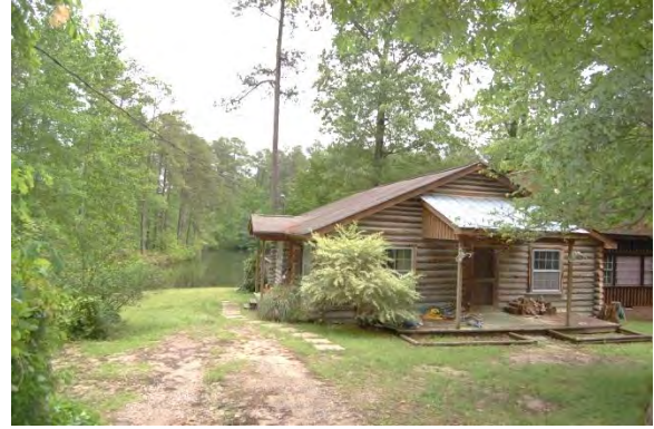
No. 158 House (PIN 1742651371), 3061 Hodge Road, Garner Vicinity, Wake County
