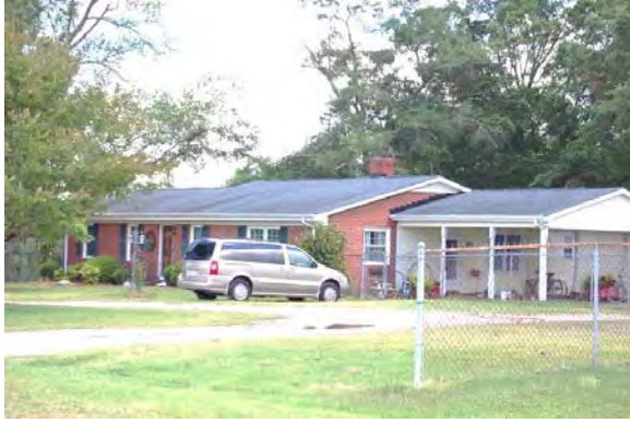
No. 175 House (PIN 1743342545), 5101 Faison Ridge Lane, Garner Vicinity, Wake County
