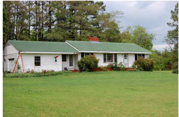
No. 143 House (PIN 1740495885), 7629 Old Baucom Road, Garner Vicinity, Wake County
