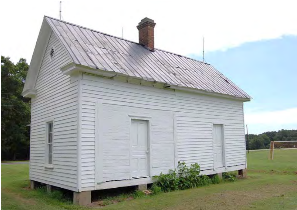
Plate 45. C. B. Sorrell House, Rear Elevation, Looking Southeast.
