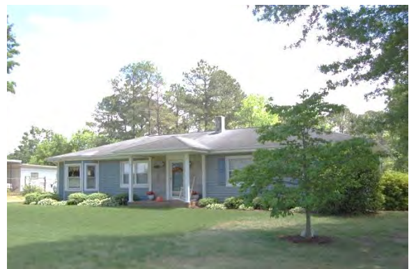
No. 174 House (PIN 1743249441), 5113 Faison Ridge Lane, Garner Vicinity, Wake County
