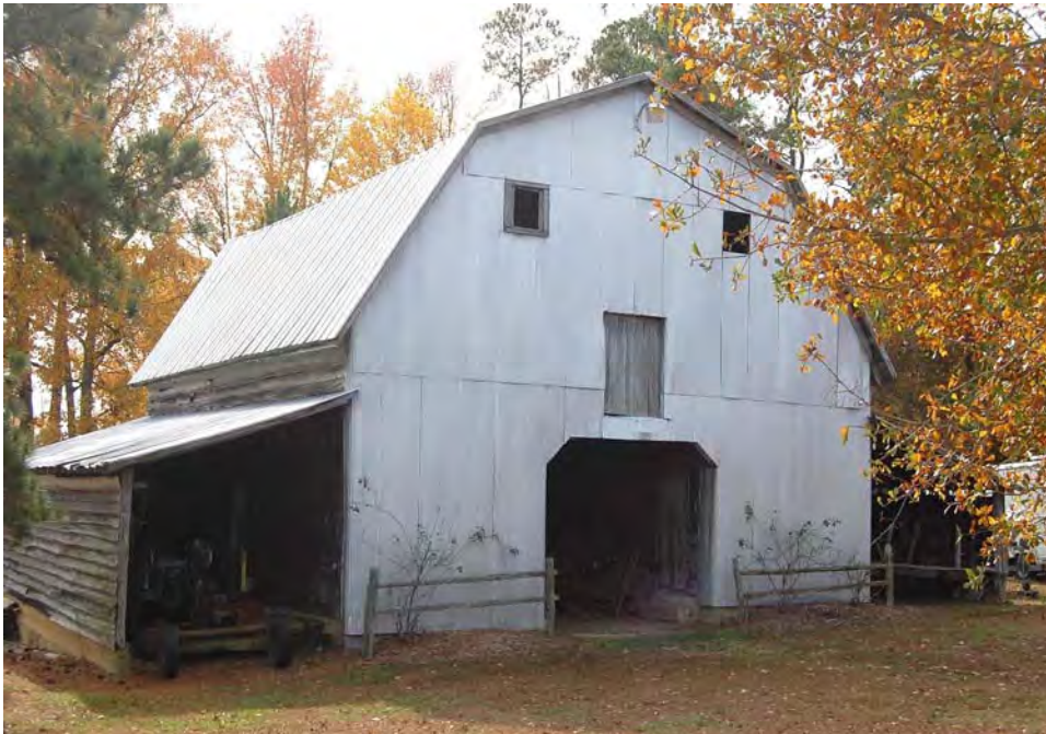
Plate 60. Bell-Pierce Farm, Eastern Tract, Barn, Looking South.
