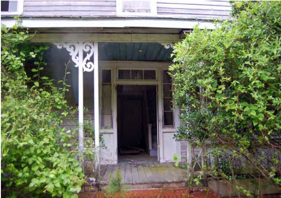
Plate 320. Penny House, Entrance and Porch Details, Looking East.
