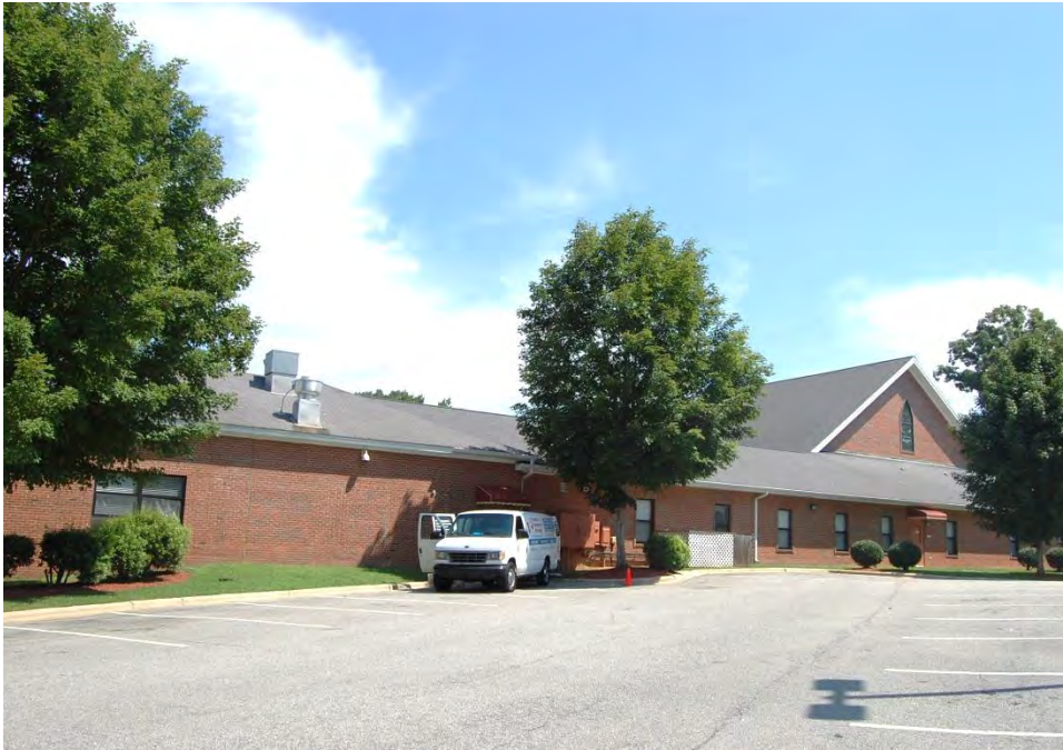
Plate 432. Popular Springs Christian Church, 1996 Addition, Rear (South) Elevation, Looking North.
