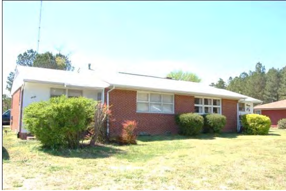
No. 106 Duplex (PIN 1740118968), 4929 Guy Road, Garner Vicinity, Wake County
