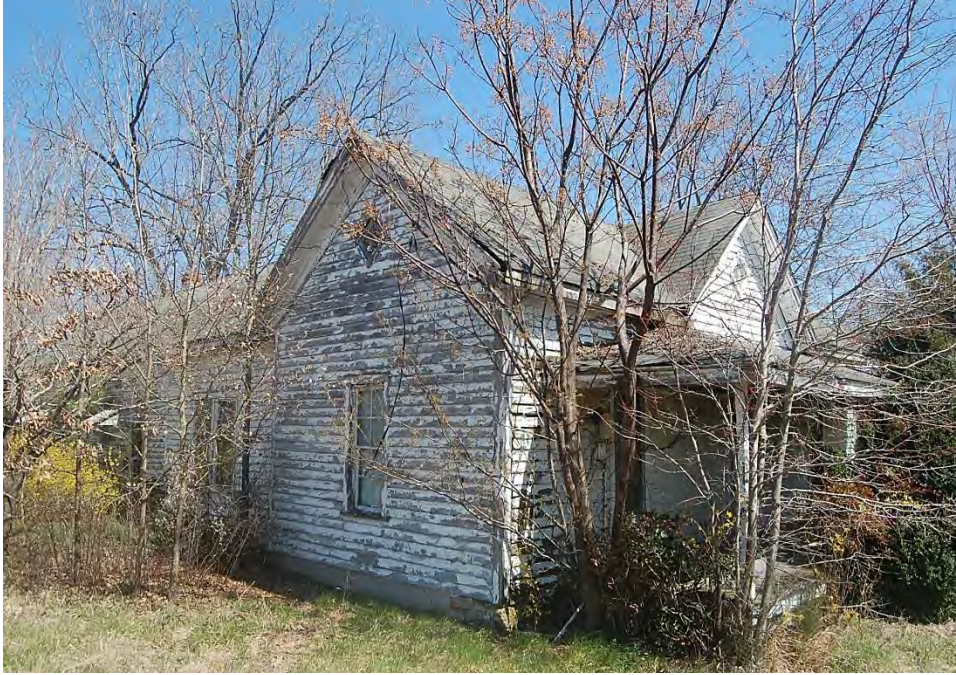
Plate 676. Thomas Woolard Farm, House, Side (West) Elevation and Facade, Looking Northeast.
