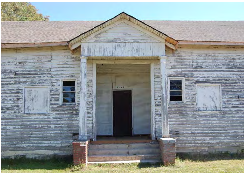
Plate 203. Panther Branch School, Main Entrance, Looking East.
