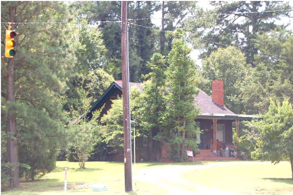
Plate 532. Auburn, James G. Lane House (No. 269), Looking Southwest.
