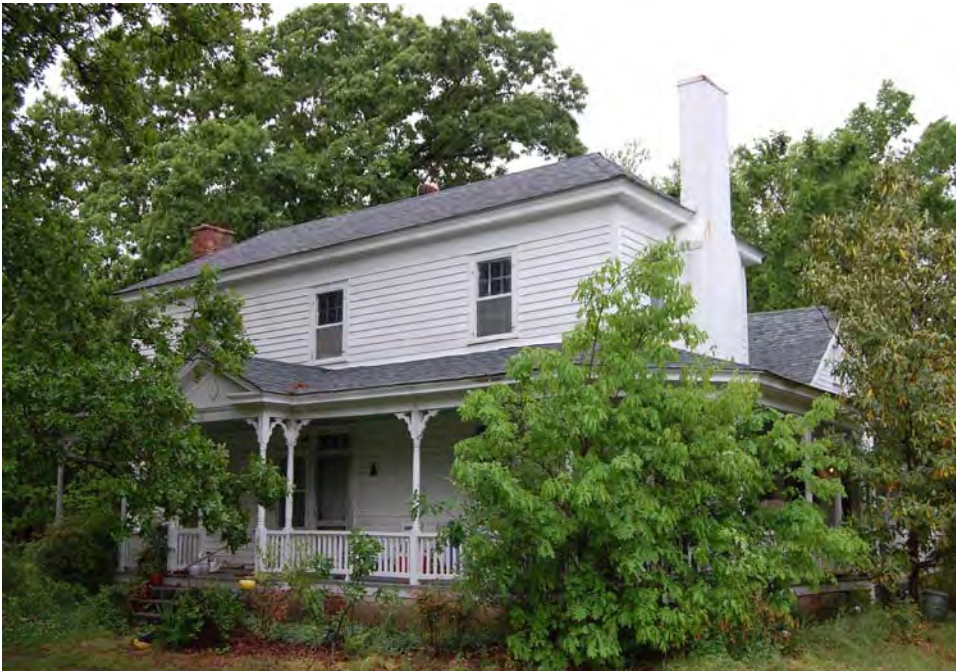
Plate 336. Baucom-Stallings House, Façade (South Elevation), Looking North.
