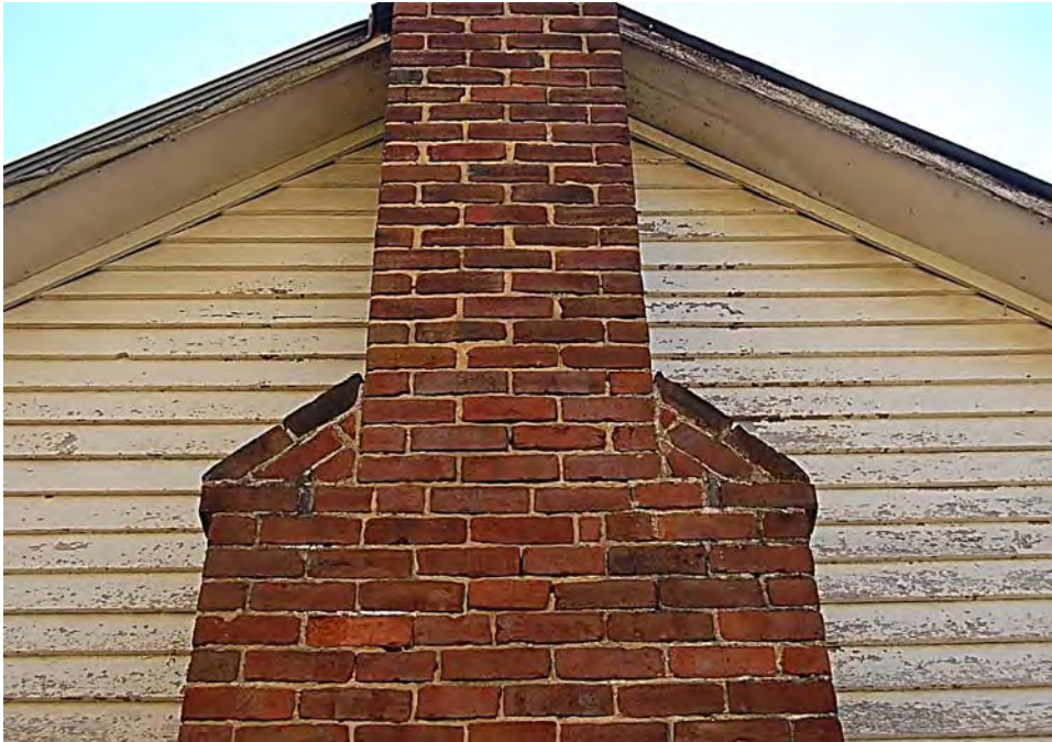
Plate 377. William Pierce House, Chimney, North Elevation, Looking South.
