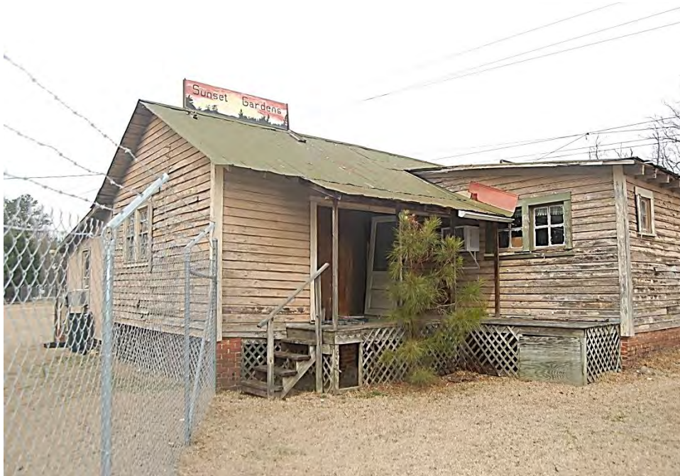
Plate 576. Thomas Store, Rear Ell, Looking North.
