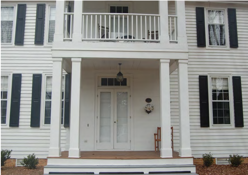
Plate 686. Burt-Utley House, Façade (South Elevation), Looking North.
