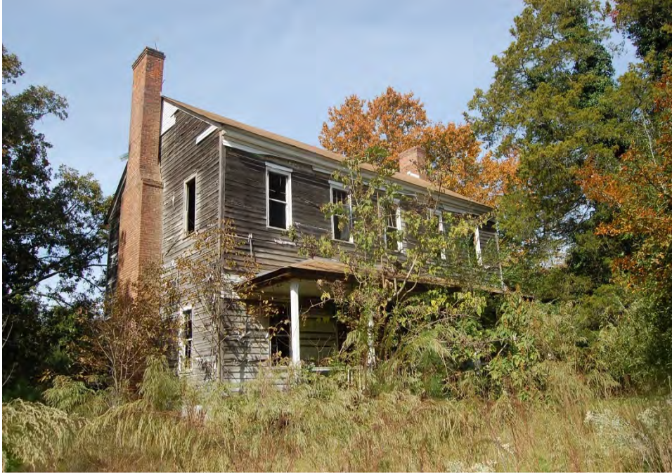
Plate 412. David and Sarah Stephenson House, Rear (East) Elevation, Looking Northwest.
