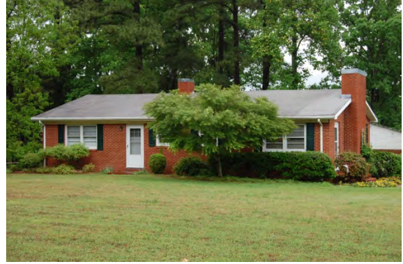
No. 141 House (PIN 1741300225), 7509 Old Baucom Road, Garner Vicinity, Wake County
