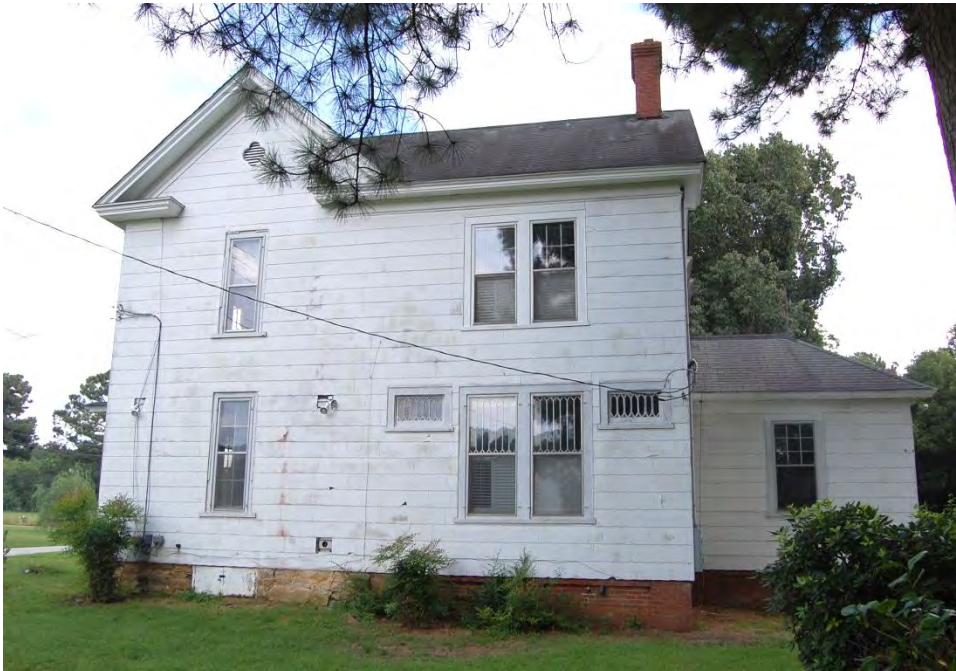
Plate 506. Johns-Lane-Poole House, Side (West) Elevation, Looking East.
