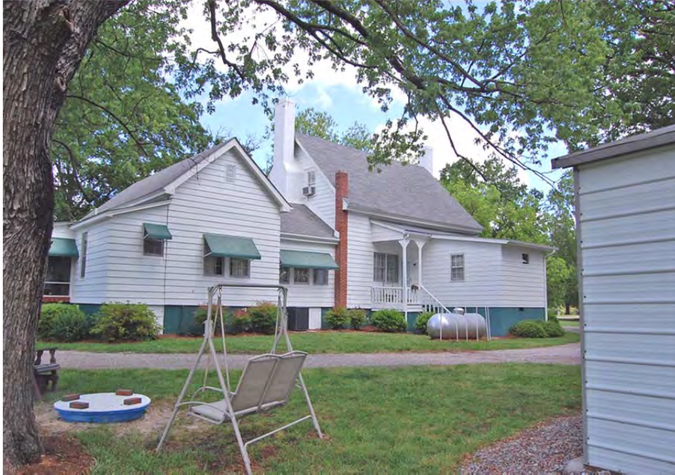
Plate 348. The Oaks, House, Rear (West) Elevation, (Original Front Elevation), Looking East.
