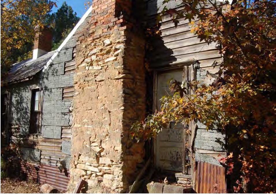
Plate 13. Wes Jones Farm, House, Chimney, South Elevation, Looking Northwest.
