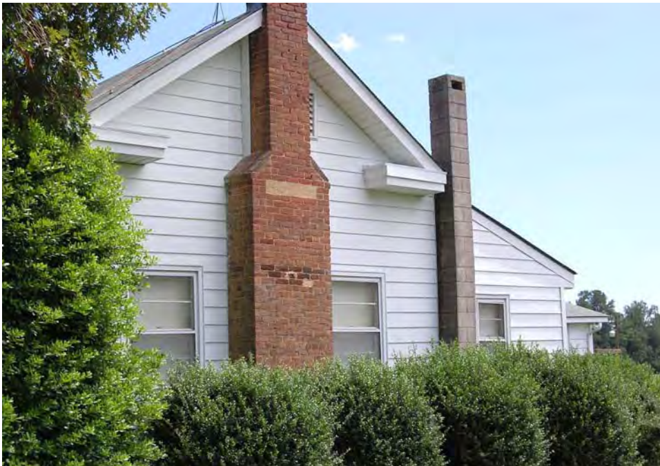
Plate 58. Bell-Pierce Farm, Eastern Tract, Bell-Pierce House, Side (West) Elevation, Looking East.
