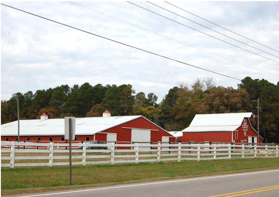
Plate 606. Jones-Johnson-Ballentine Farms Historic District, Modern Horse Training Facility on the Ballentine Farm, Looking North along Sunset Lake Road.
