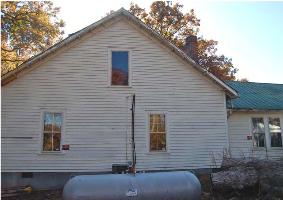
Plate 4. G. L. Pierce House, Side (North) Elevation, Looking South.
