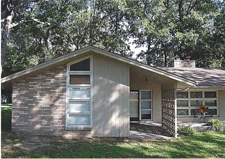
Plate 365. Gerald Cochran House, Façade, Looking East.
