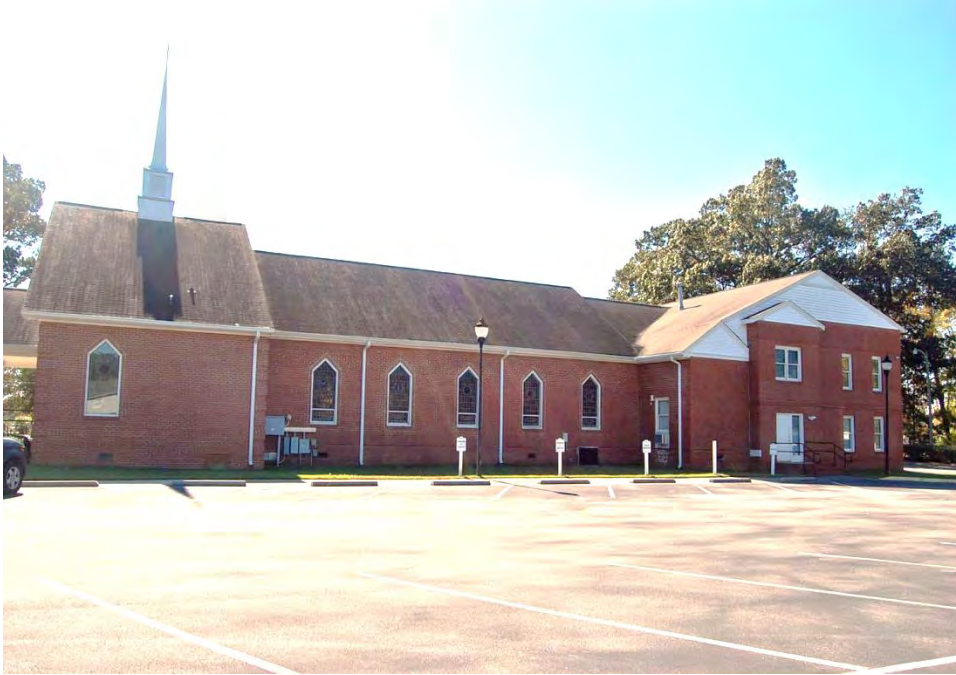
Plate 193. Juniper Level Baptist Church, Side (North) Elevation, Looking South.
