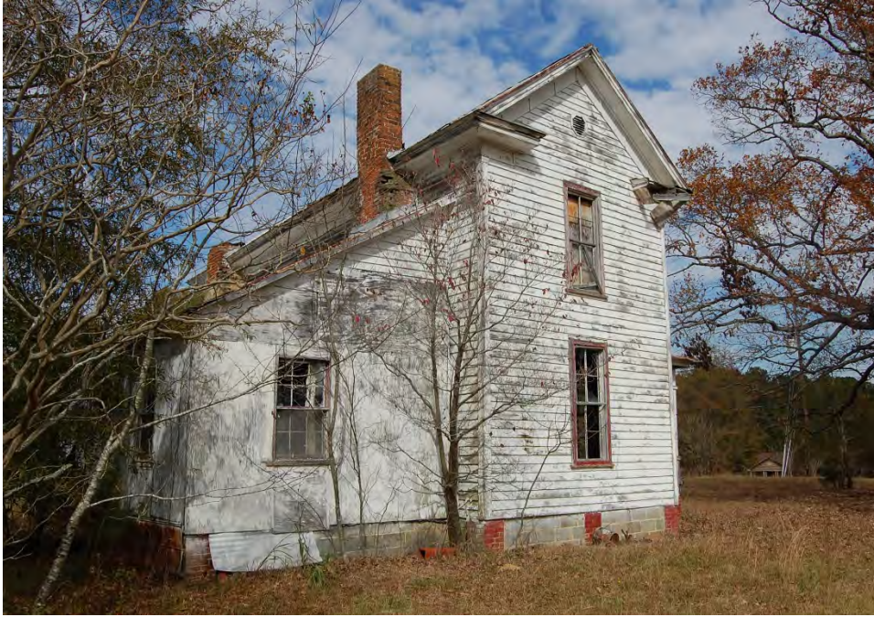
Plate 650. Jones-Ellington House, Side (South) Elevation and Rear Shed, Looking North.
