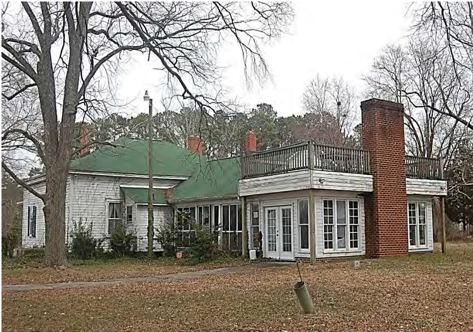
Plate 584. James Sugg House, Rear (South) Elevation and Rear Ell, Looking Northeast.
