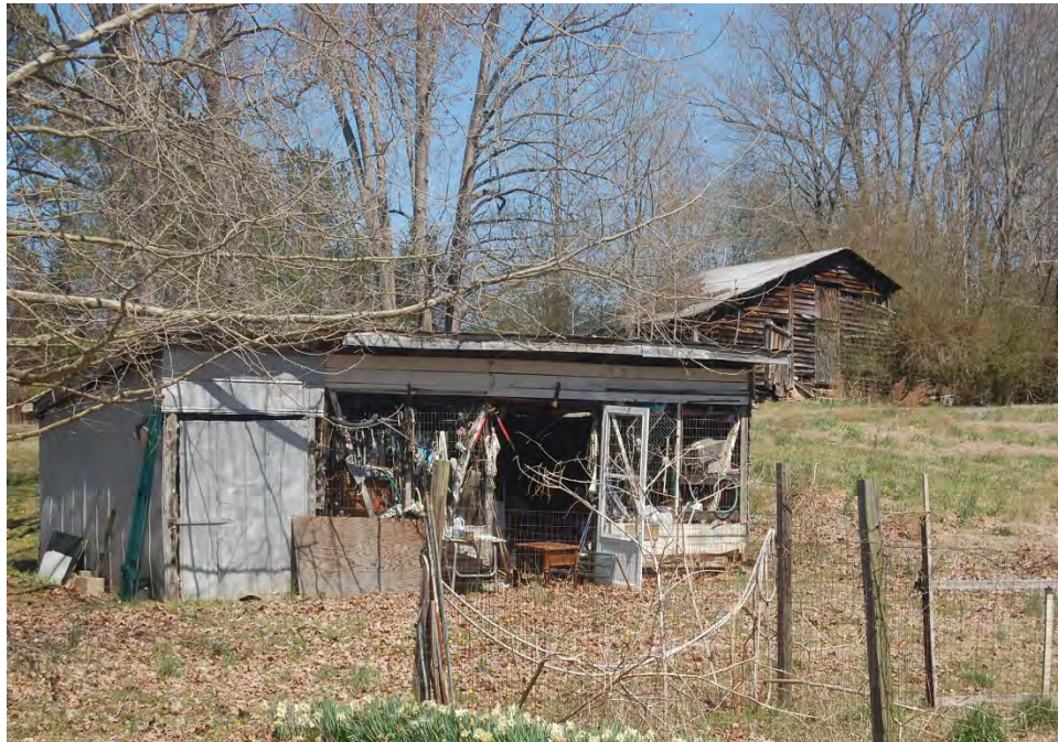
Plate 667. Jim Jordan Farm Complex, Chicken House and Packhouse (Background), Looking North.
