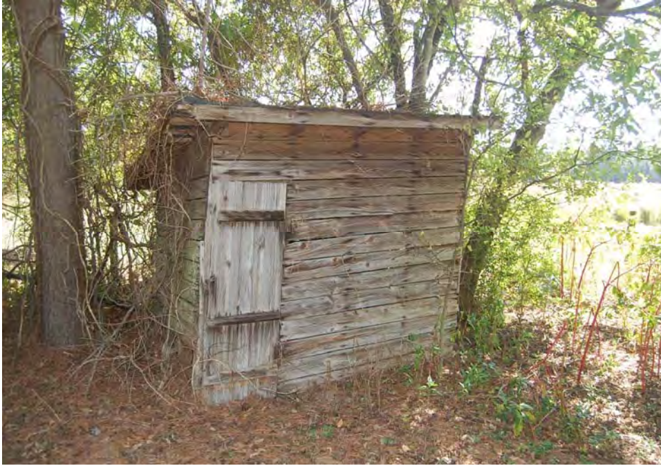
Plate 274. W. A. Gowers Farm, Tenant House Complex, Shed, Looking Southeast.
