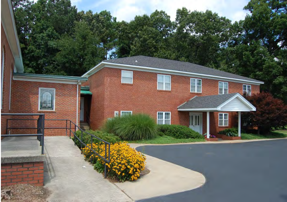
Plate 438. New Bethel Baptist Church, 1954 Classroom and Fellowship Hall Building, Looking West.
