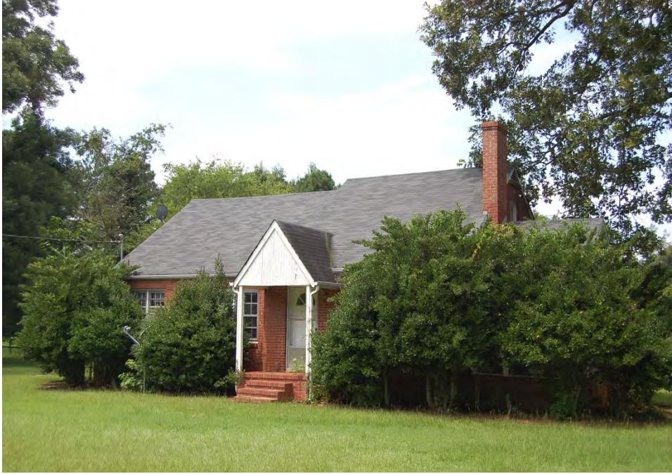
Plate 444. New Bethel Baptist Church, Parsonage, Looking Southwest.
