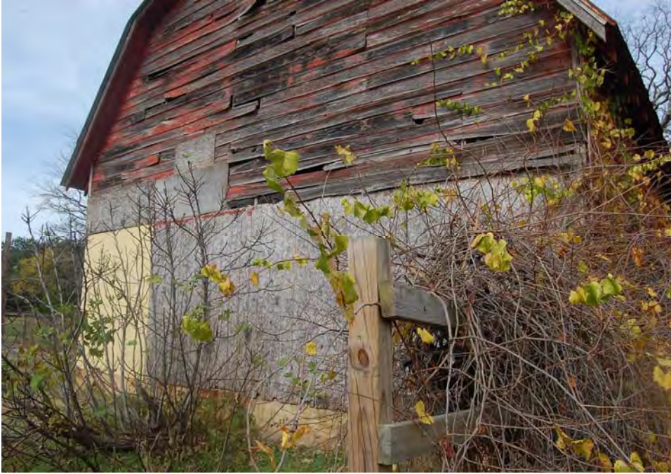
Plate 390. Arthur Atkins House, Barn, Rear (South) Elevation, Looking North.
