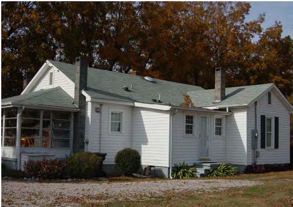
Plate 76. Bell-Pierce Farm, Western Tract, House, Side (East) and Rear (South) Elevations, Looking North.
