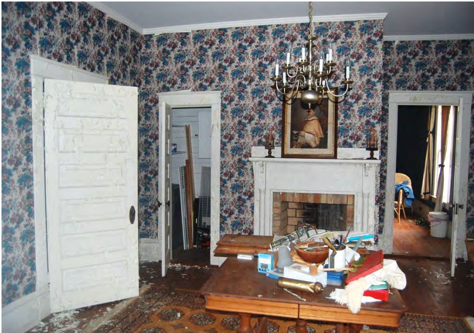
Plate 586. James Sugg House, Interior, East Rear Room.
