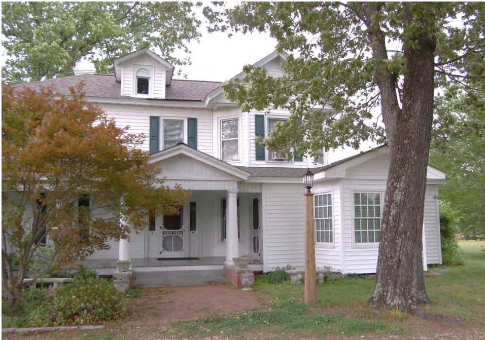
Plate 298. Icana Poole House, Façade (South Elevation), Looking North.
