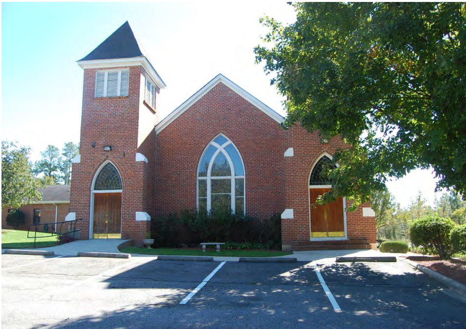
Plate 427. Poplar Springs Christian Church, 1932 Church, Front (North) Elevation, Looking South
