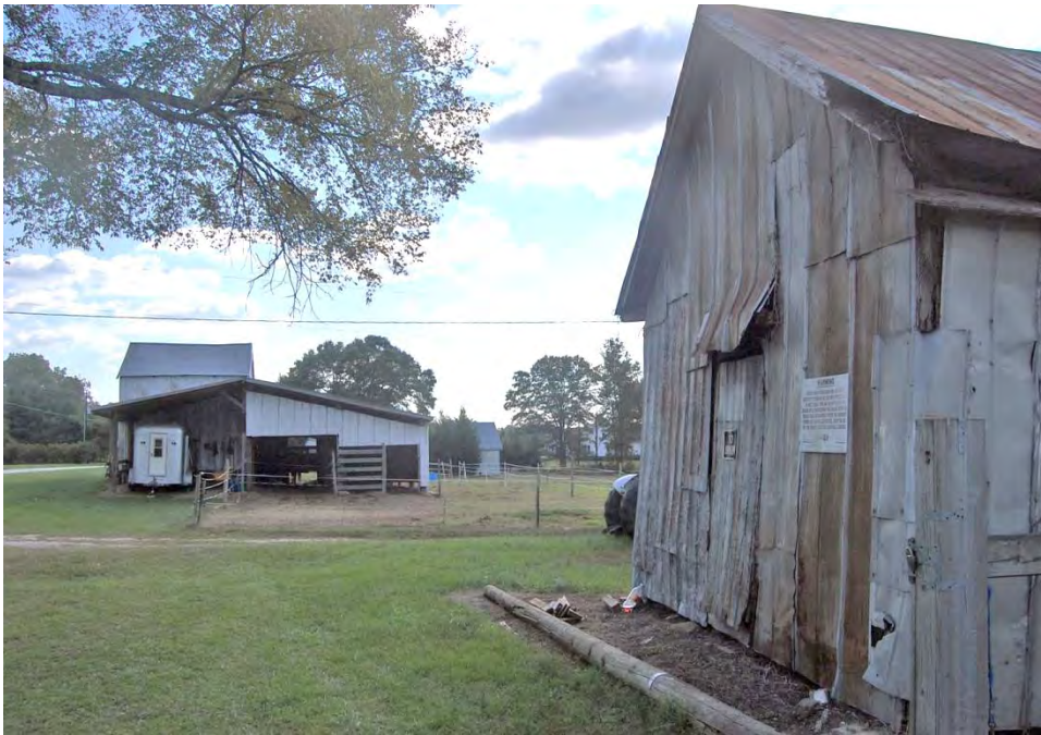
Plate 215. Jones Family Farm, Shed and Tobacco Barn, Looking South.
