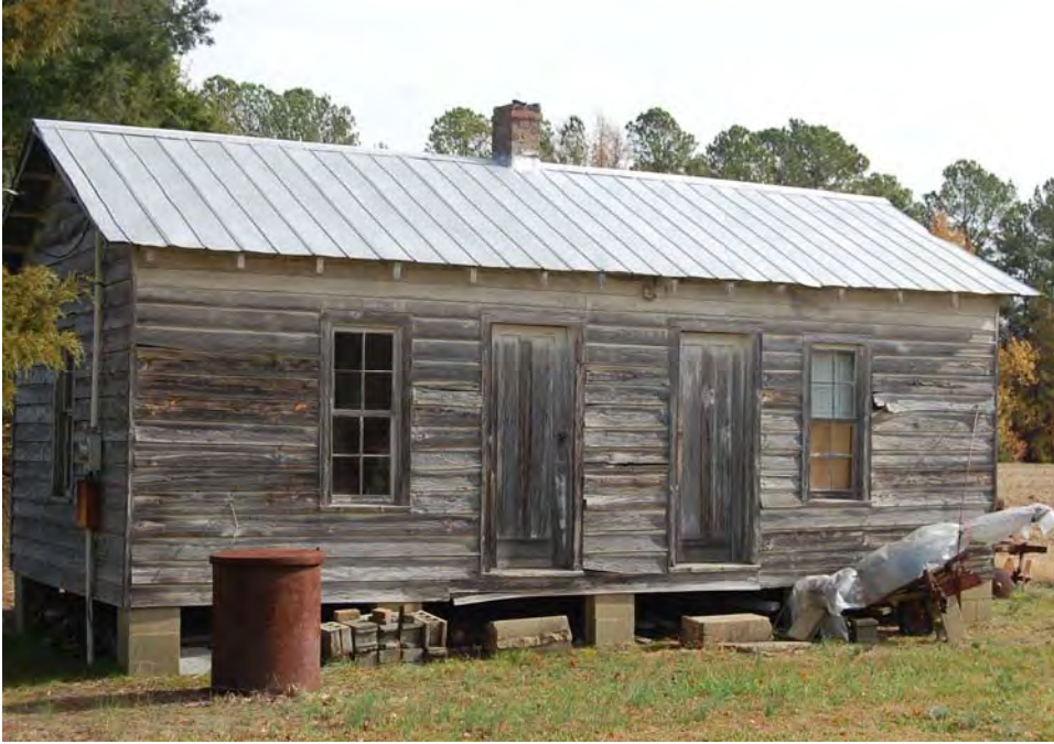
Plate 69. Bell-Pierce Farm, Eastern Tract, Tenant House, Looking East.
