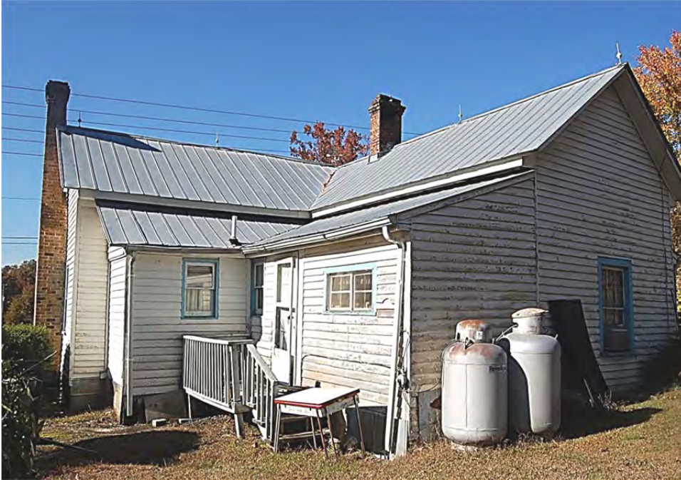
Plate 379. William Pierce House, Rear Ell, Looking West.
