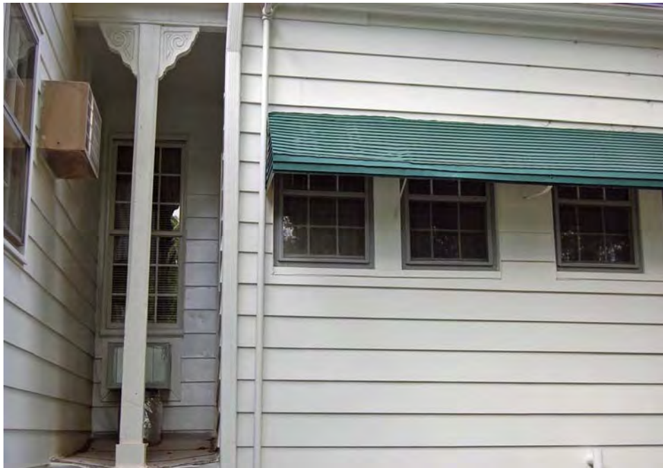
Plate 349. The Oaks, House, Porch Post, Rear (West) Elevation, Looking East.
