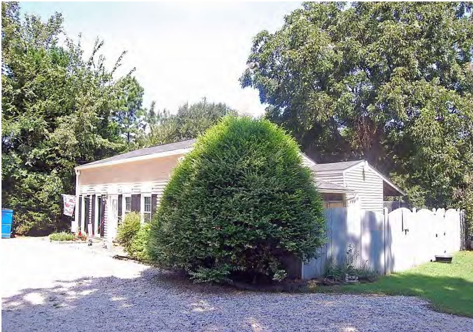
Plate 491. David Lewis House, Modern Kennel, Looking West.
