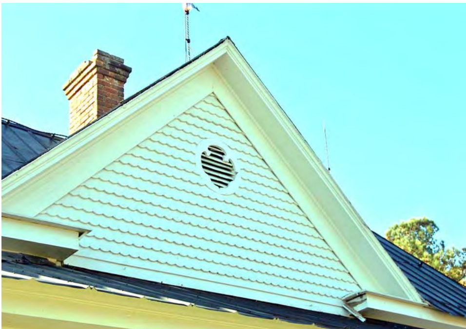
Plate 44. C. B. Sorrell House, Detail of Front Gable.
