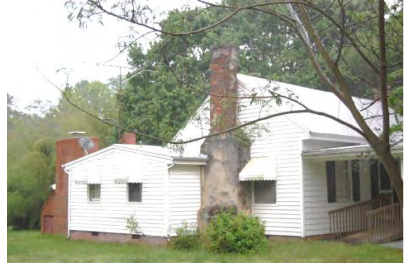
No. 134 House (PIN 1730882081), 7201 Hollybrook Farm Road, Garner Vicinity, Wake County
