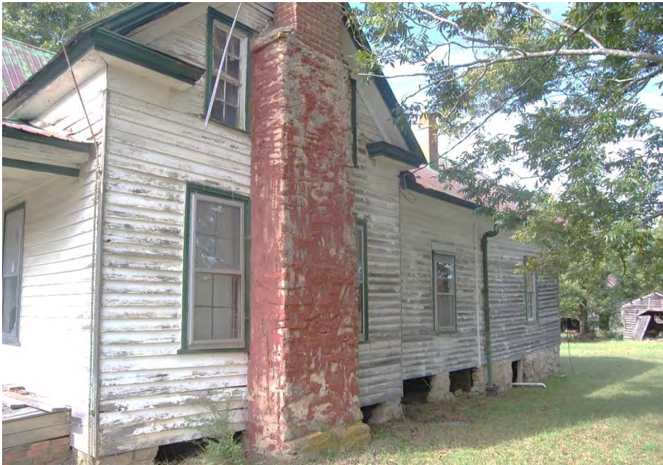
Plate 478. Yeargan House, Side (East) Elevation and Outbuildings (Background), Looking Northwest.
