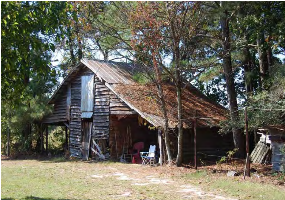
Plate 273. W. A. Gowers Farm, Tenant House Complex, Packhouse, Looking Southwest.
