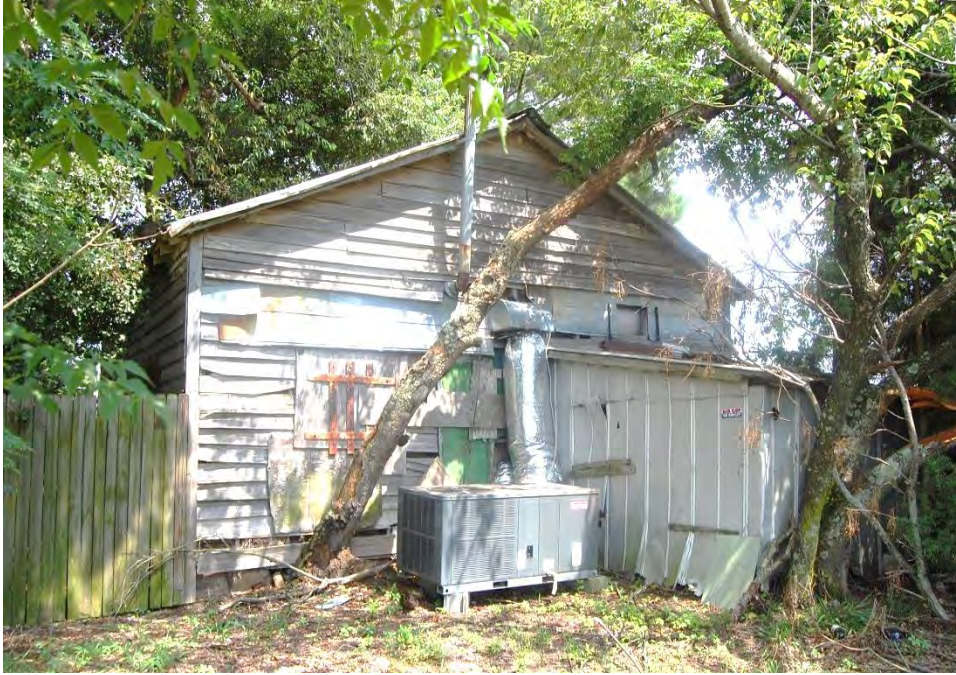
Plate 560. Britt's Store, Rear (West) Elevation, Looking East.
