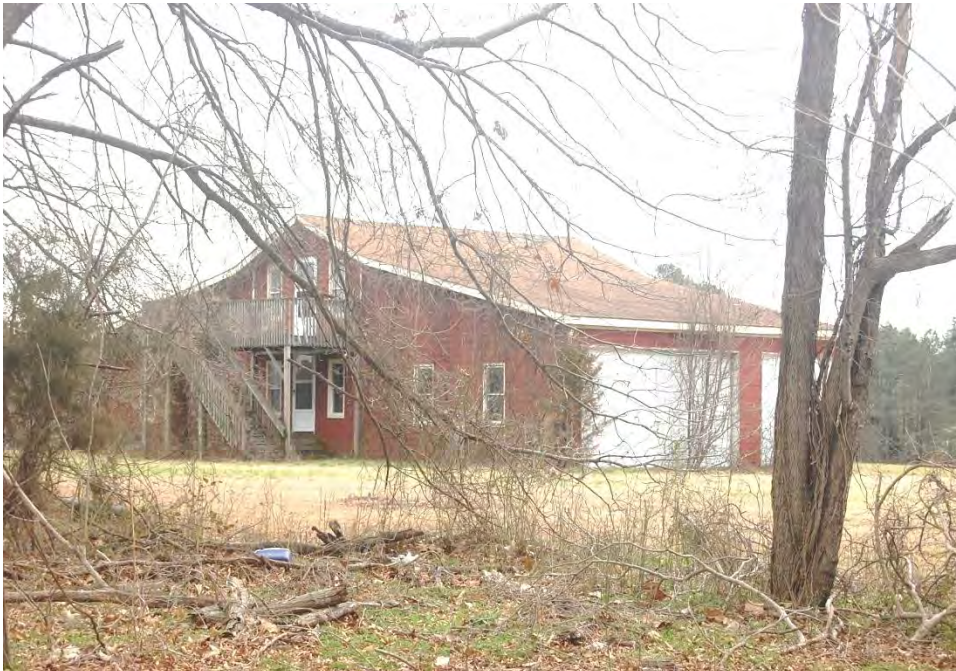
Plate 592. James Sugg House, Former Packhouse, Looking Southeast.
