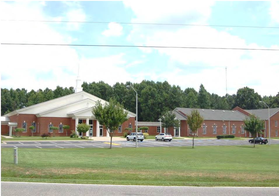
Plate 527. Springfield Baptist Church, Modern Church Complex.
