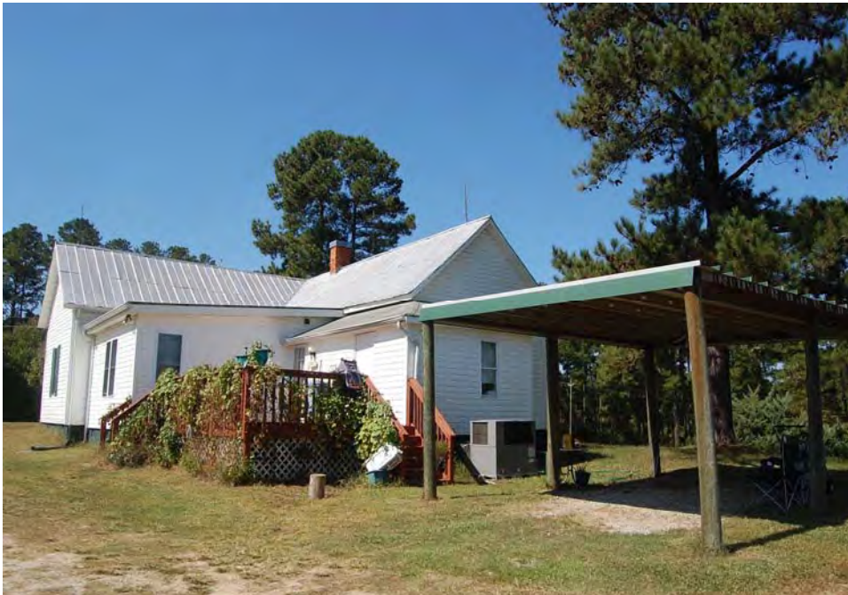
Plate 257. John Williams Farm, House, Rear (East) Elevation, Looking West.
