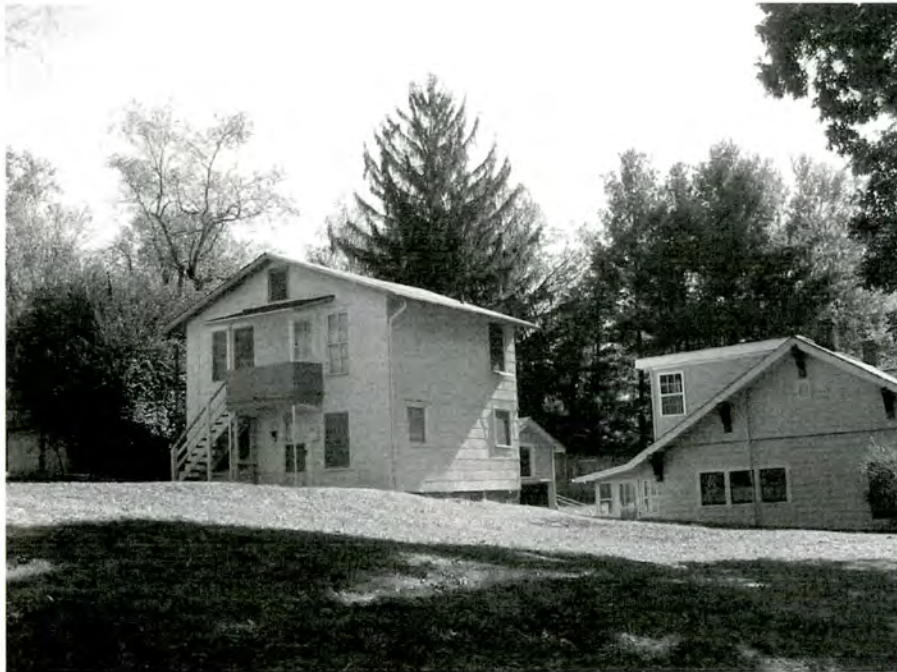
House and Guest House (No. 39), Side Elevation of Main House and Guest House.
