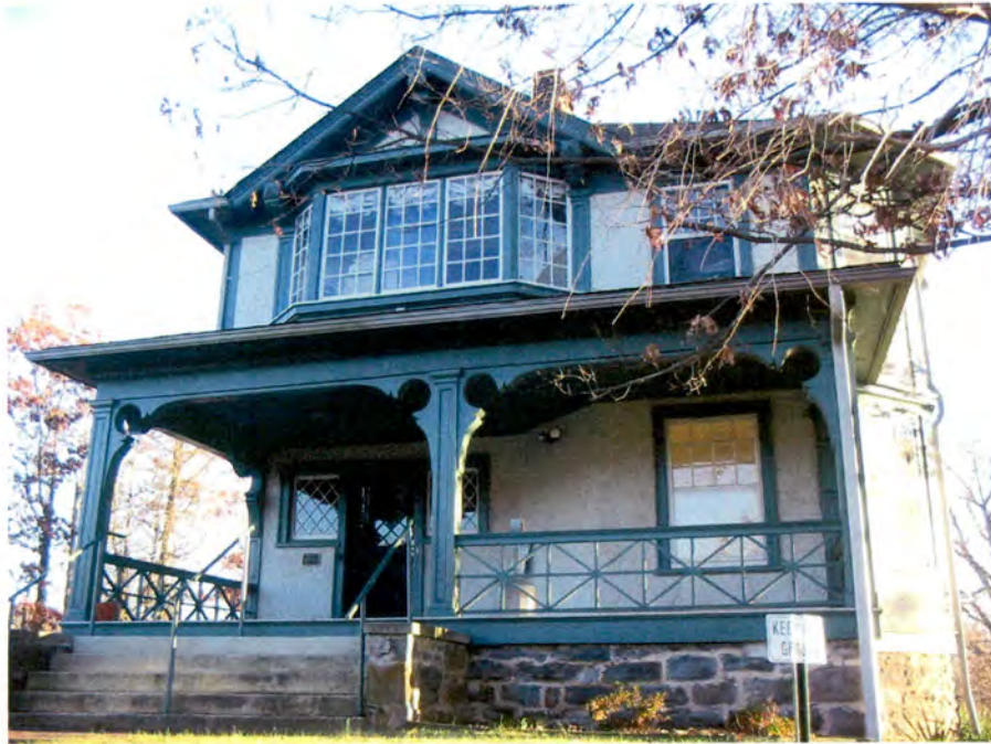
Plate 11. Mrs. Minnie Alexander Cottage (No. 134), Façade, Looking South.
