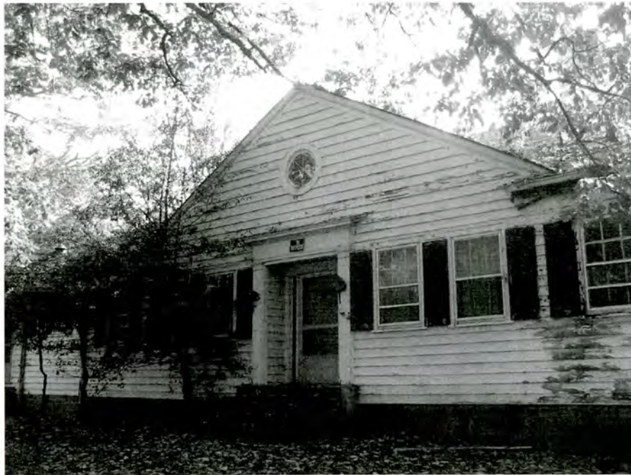
Ingle House (No. 2), Rear Elevation and Entrance.
