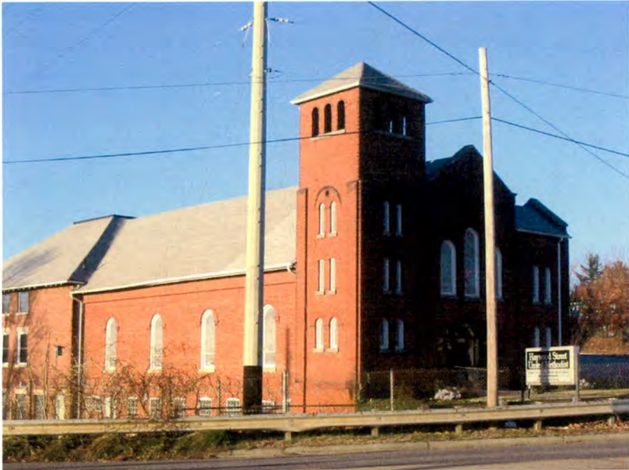
Plate 27. Haywood Street United Methodist Church (No. 136), Looking North.
