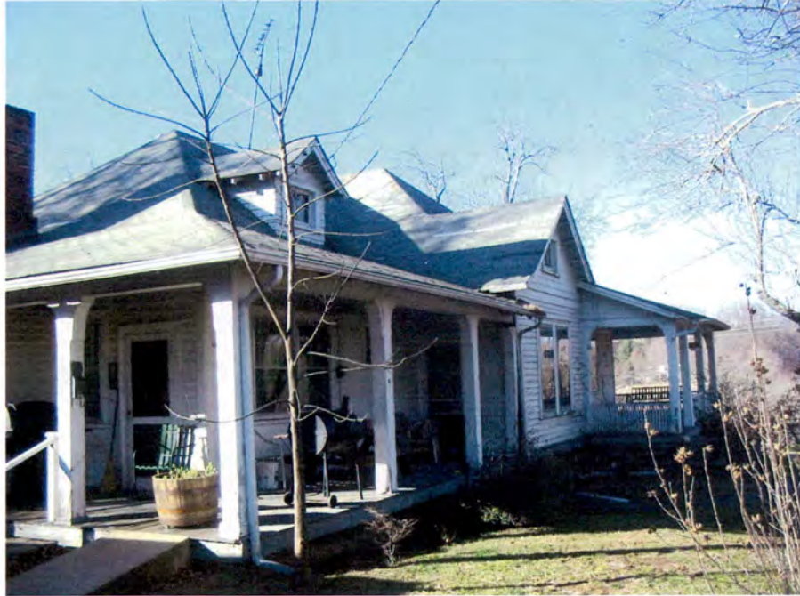
Plate 33. Freeman House (No. 147), Rear Porch and Side (East) Elevation, Looking North.
