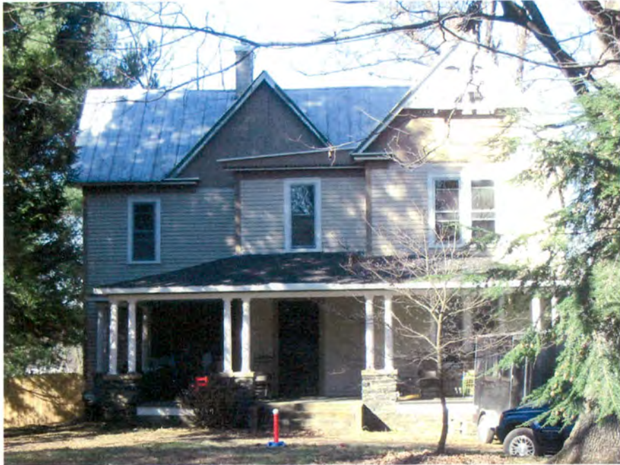
Plate 8. C.G. Worley House (No. 128), House and Setting, Looking North.
