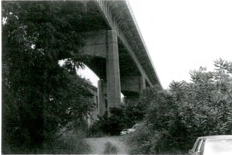
Plate 21. Great Smoky Mountain Park Bridge (No. 151), Looking West.
