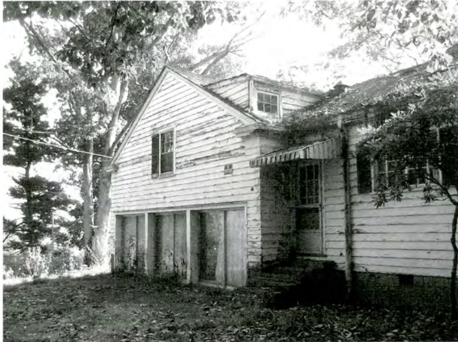
Ingle House (No. 2), Rear Elevation.
