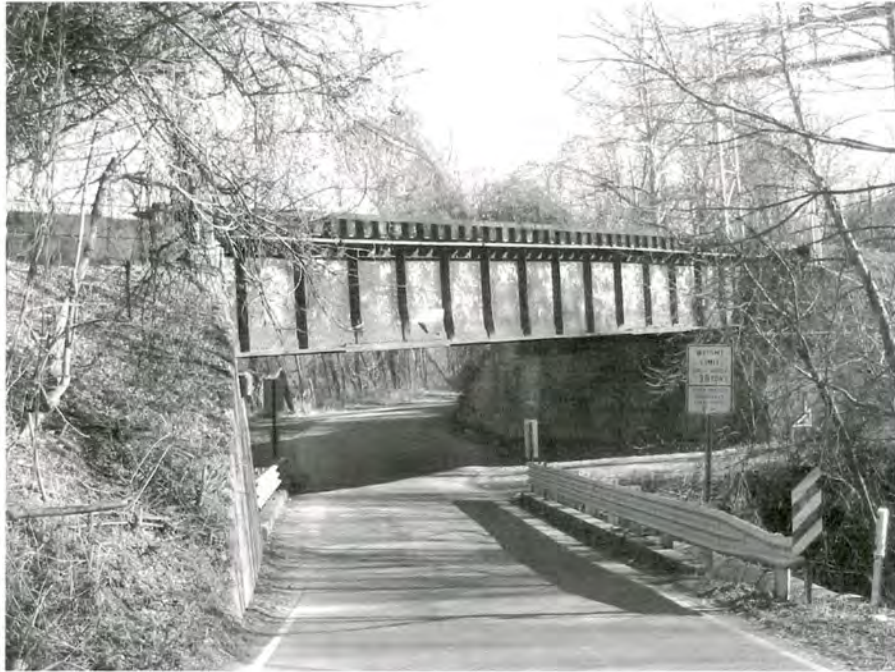
Norfolk and Southern Railway Bridge (No. 144).
