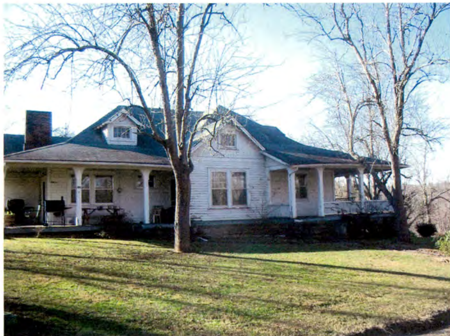
Plate 34. Freeman House (No. 147), East Elevation, Looking West.
