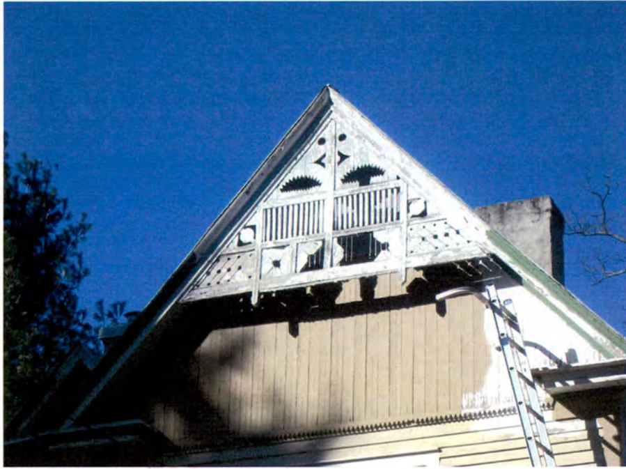
Plate 10. C.G. Worley House (No. 128), Gable Detail.
