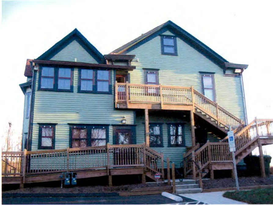
Plate 15. Whiteford G. Smith House (No. 135), Rear (North) Elevation, Looking South.
