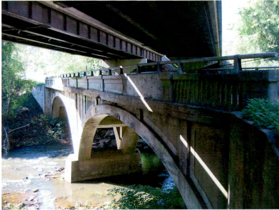
Plate 3. Buncombe County Bridge No. 216 (No. 8), Looking South.
