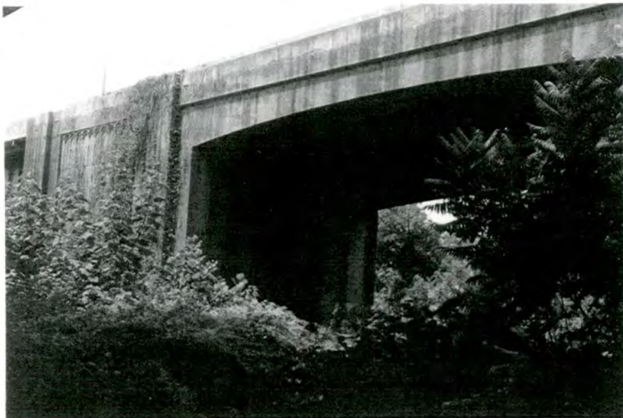
Plate 22. Great Smoky Mountain Park Bridge (No. 151), North Elevation Showing Architectural Details.
