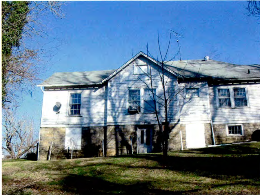
Plate 31. Freeman House (No. 147), Side (West) Elevation, Looking East.
