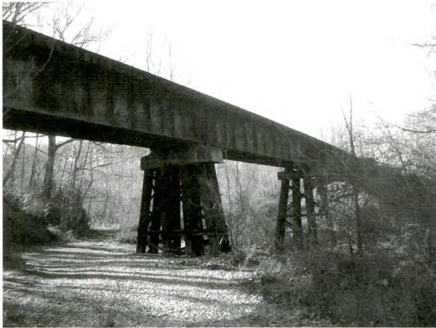
Norfolk and Southern Railway Bridge (No. 145).
