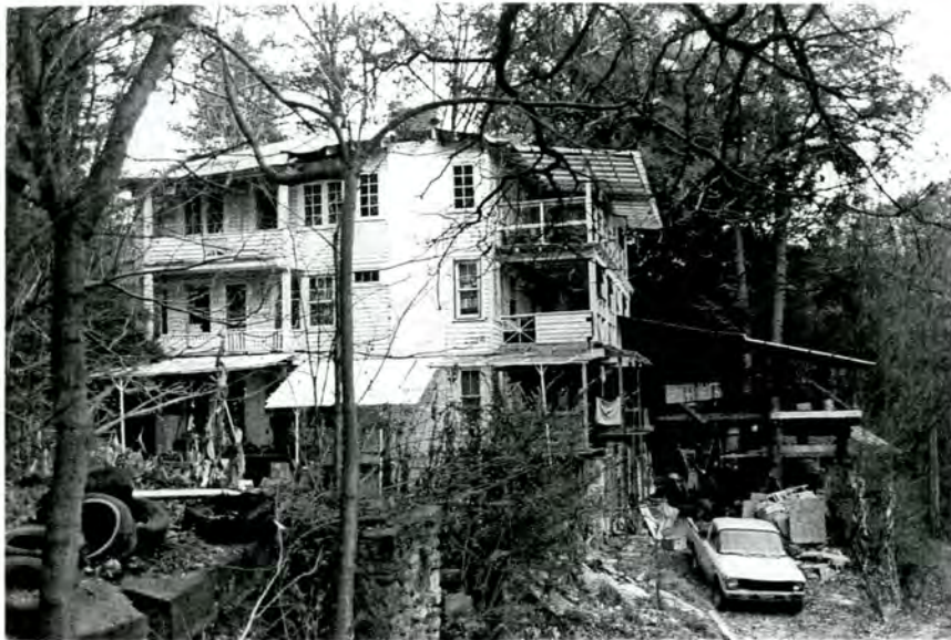
Plate 15. House, West End Pearson Drive, West of Proposed Boundary Expansion, Looking East.
