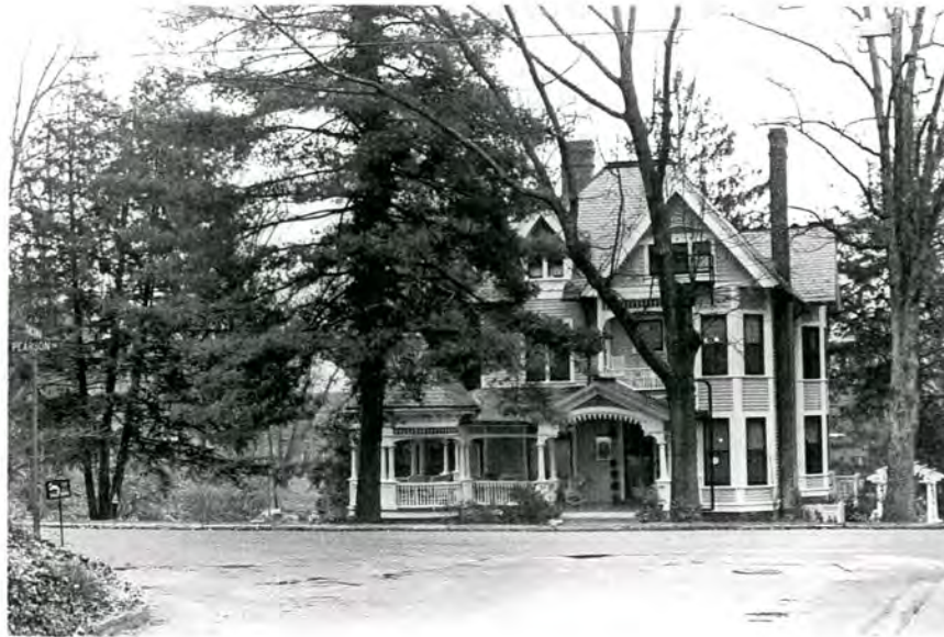
Plate 2. Montford Area Historic District, Pearson Drive at Tacoma Street, Looking East.
