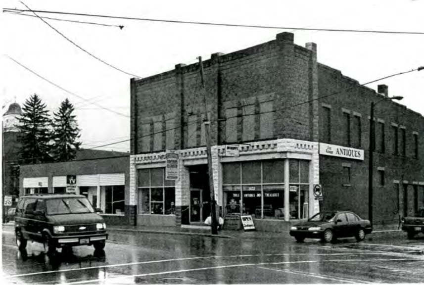
Plate 22. (Former) Friendly Grocery Store Building and Setting, Looking North
