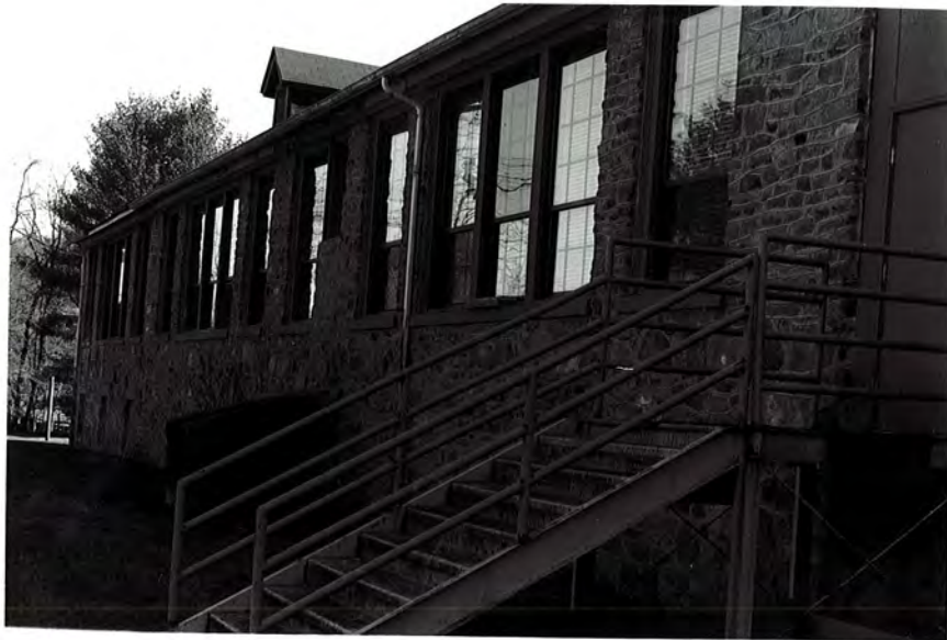
Plate 10. Stecoah School, North Elevation, Looking Southeast.
