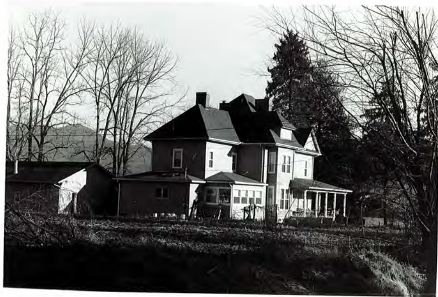
Plate 4. George B. Walker House, Rear Elevation, Looking South.
