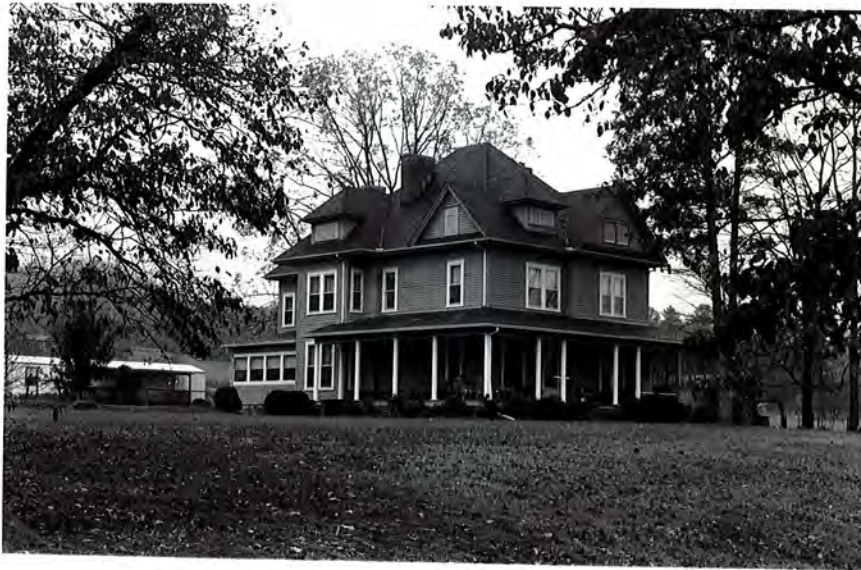
Plate 2. George B. Walker House, Looking North.
