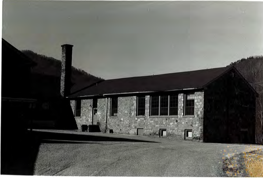
Plate 9. Stecoah School, Rear Elevation, Looking West.
