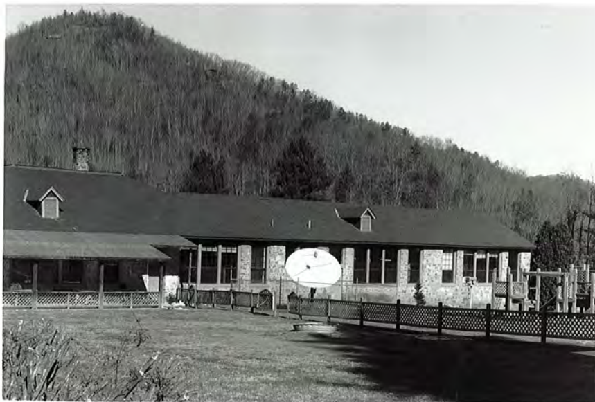
Plate 8. Stecoah School, South Elevation, Looking North.
