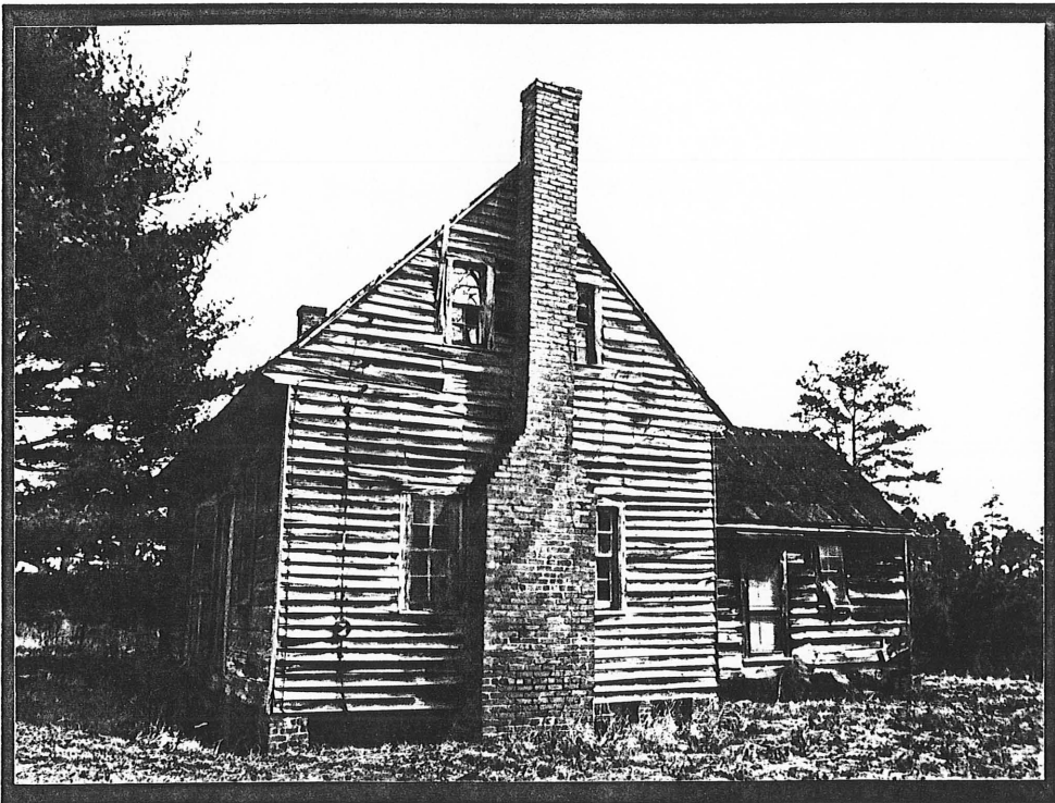
PROPERTY #65 Miller Family House— Up 0.1 Mile Dirt Lane, S Side of NC 11, 0.4 Miles W of SR 1300
