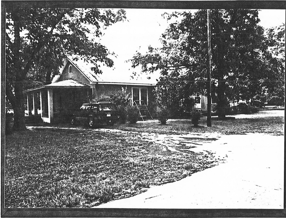
PROPERTY #23 Pink Hill Historic District—SW Corner of Broadway and Lee Street
