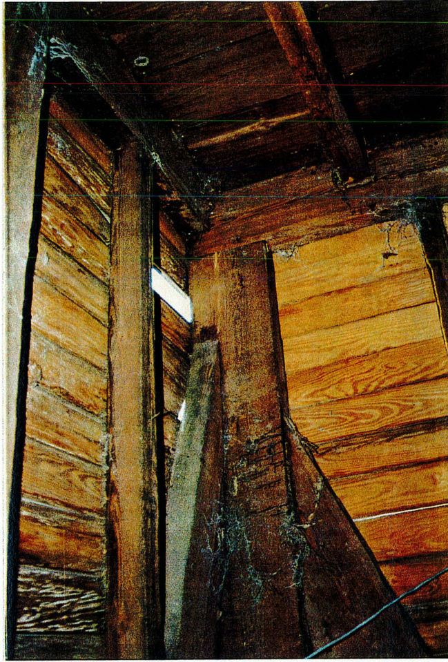
Figure 25: Warehouse (property 61), room 3, down brace detail
