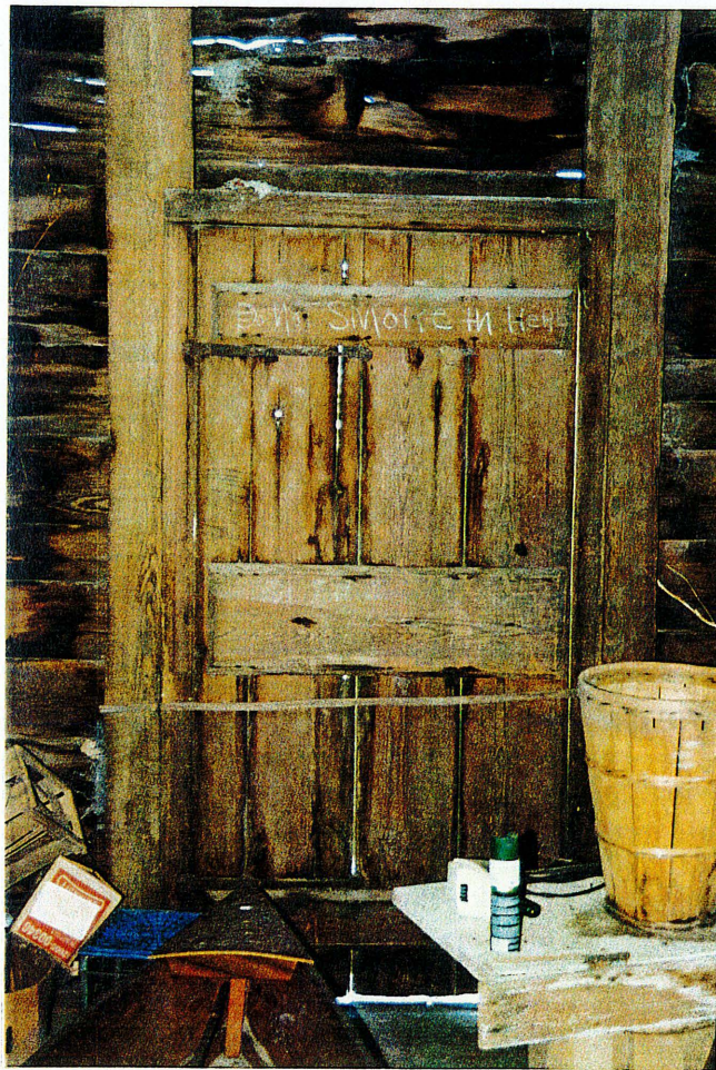
Figure 20: Warehouse (property 61), room 3, northeast door detail
