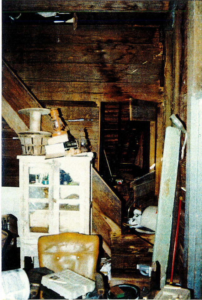
Figure 18: Warehouse (property 61), room 3, stair
