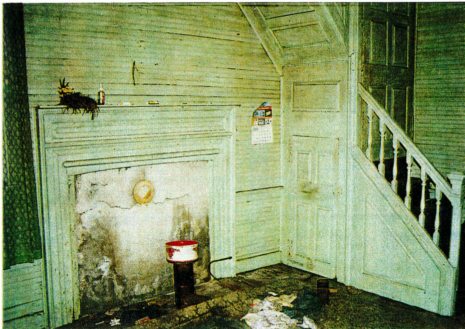
Figure 6: Colonel Stephen Miller House, interior, hall
