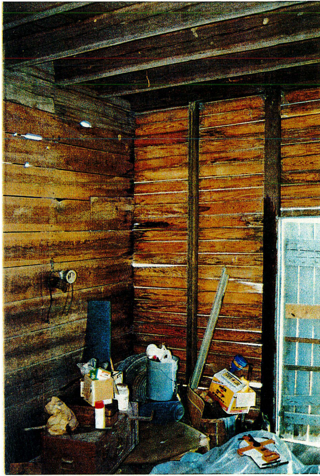
Figure 14: Warehouse (property 61), room 1, east corner
