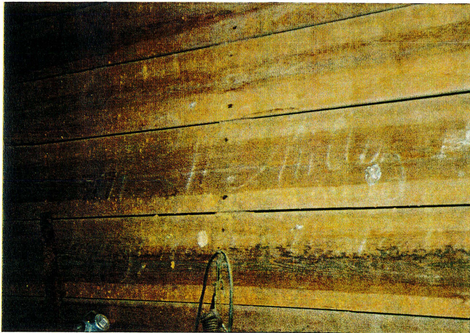
Figure 15: Warehouse (property 61), room 1, partition wall detail
