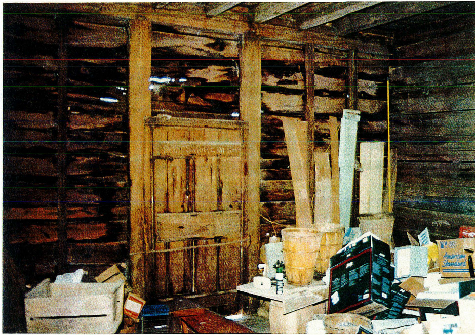
Figure 19: Warehouse (property 61), room 3, northeast door
