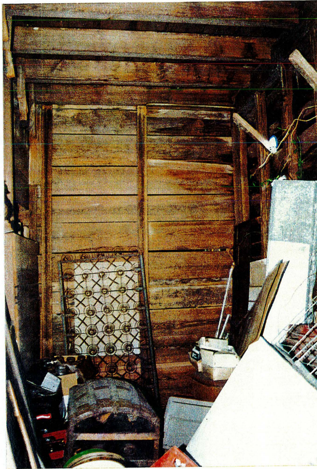
Figure 21: Warehouse (property 61), room 2, west wall
