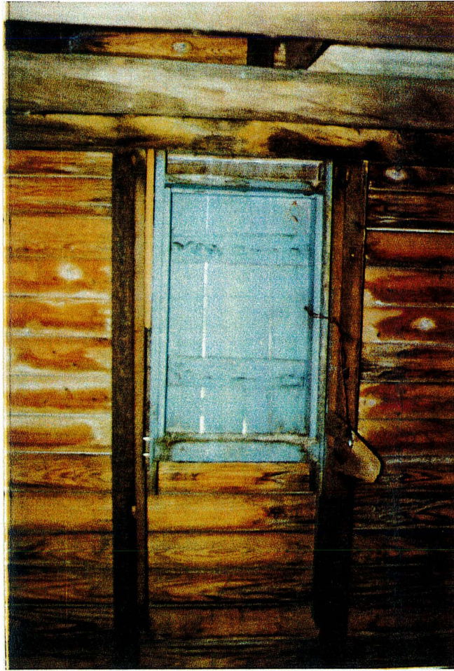
Figure 31: Warehouse (property 61), attic, window
