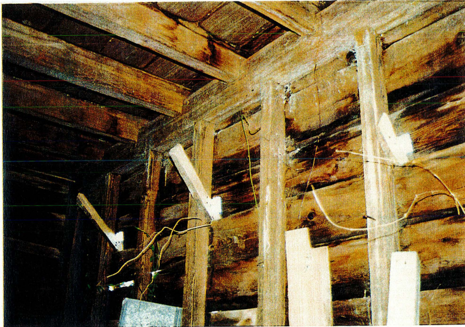
Figure 23: Warehouse (property 61), room 2, northeast wall detail
