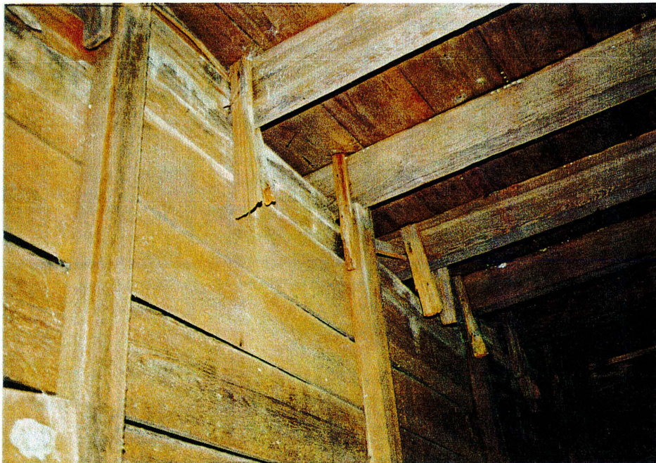
Figure 22: Warehouse (property 61), room 2, partition wall detail
