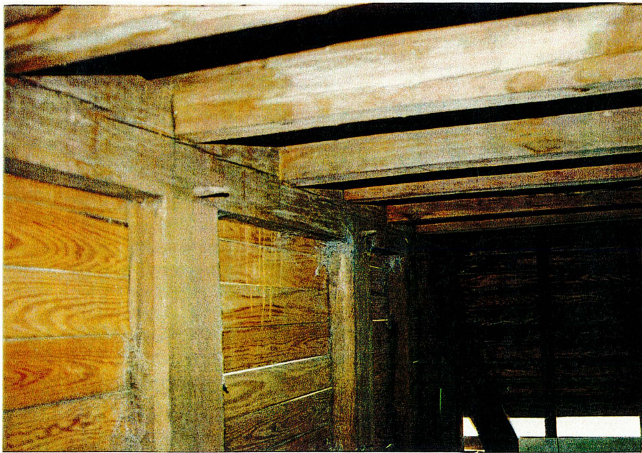
Figure 26: Warehouse (property 61), mortise and tenon detail
