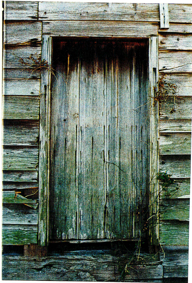
Figure 13: Warehouse (property 61), northeast door
