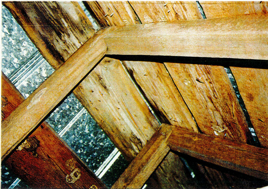
Figure 30: Warehouse (property 61), attic, pegged rafters detail
