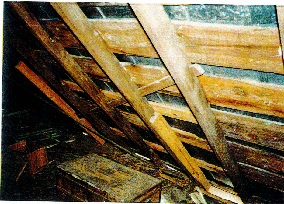
Figure 28: Warehouse (property 61), attic, cross brace detail
