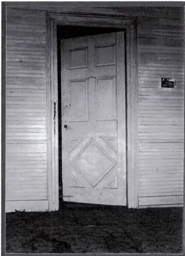
Plate IX.17 Miller Family House Door Between Hall and Parlor (Property #65)
