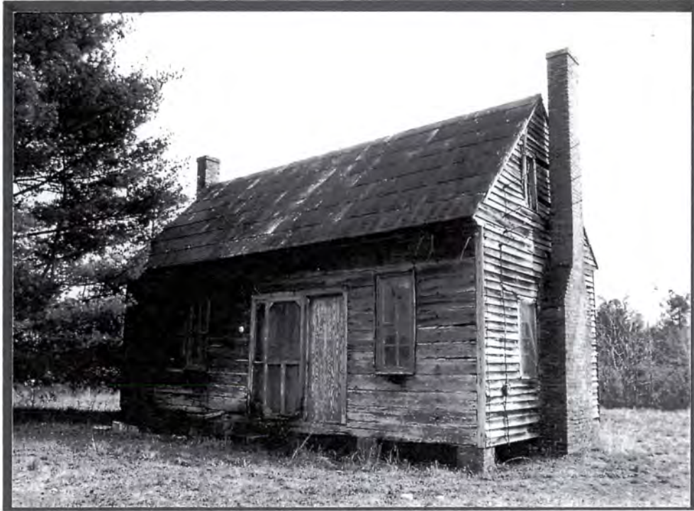
Plate IX.13 Miller Family House (Property #65)
