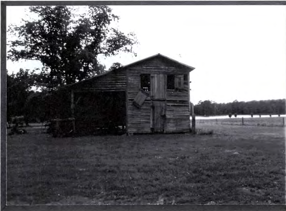
Plate IX.79 Grady House, Packhouse (Property #56)
