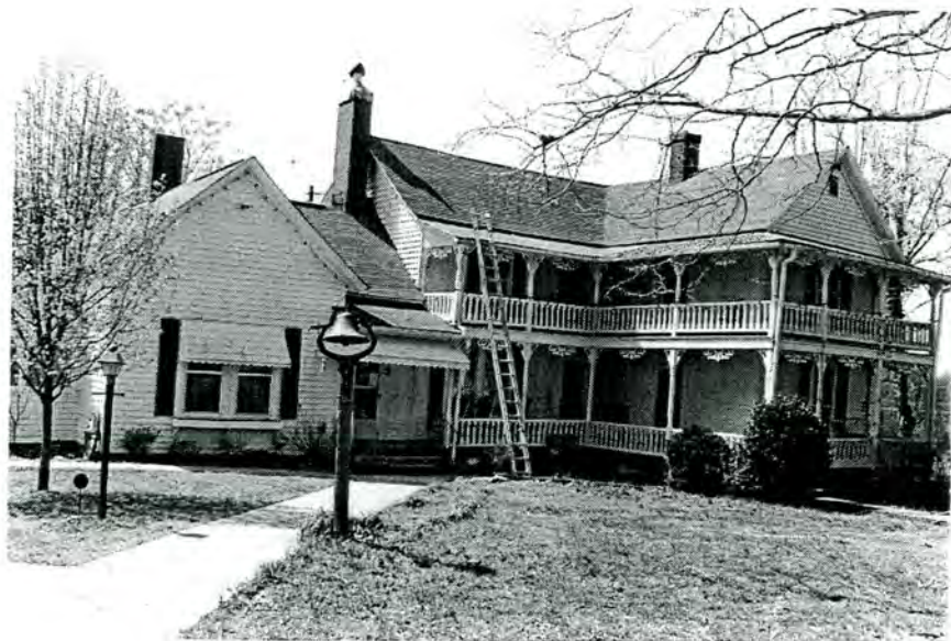
Plate 3. Hamilton-McBrayer House, Looking West.
