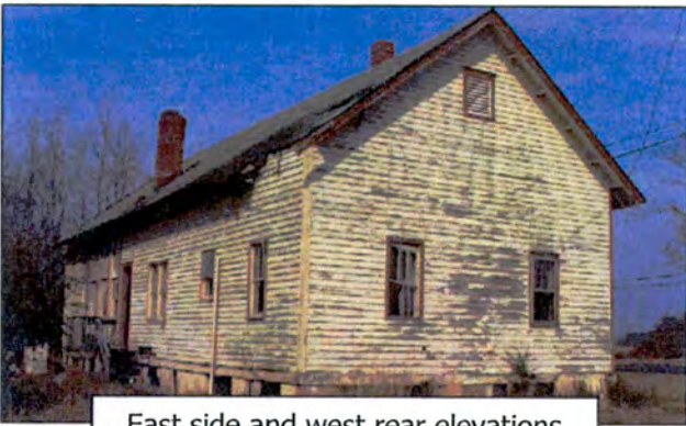
East side and west rear elevations
