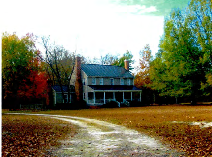
Buena Vista, House and Setting, Looking West.
