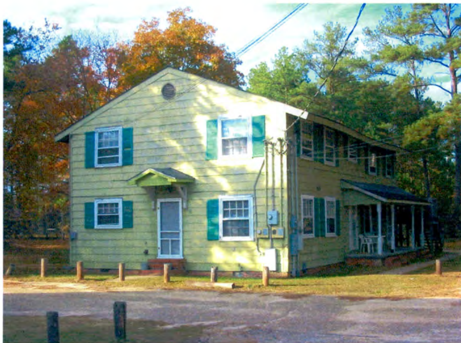
Military Houses, 700 Block, Looking North.
