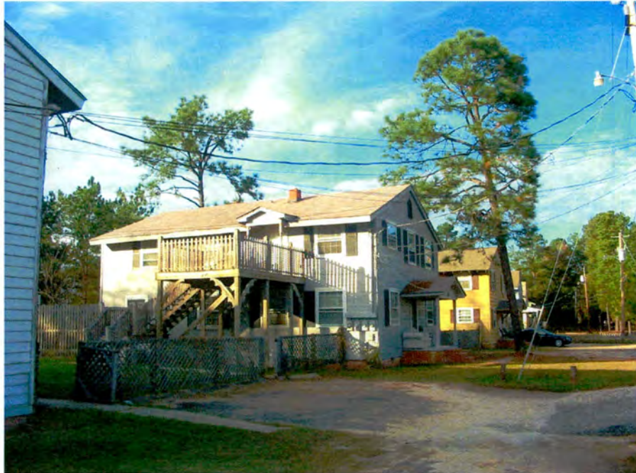
Military Houses, 700 Block, Looking North.
