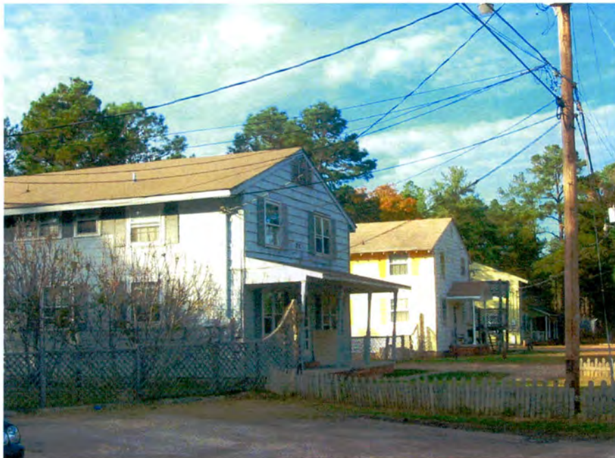
Military Houses, 700 Block, Looking North.
