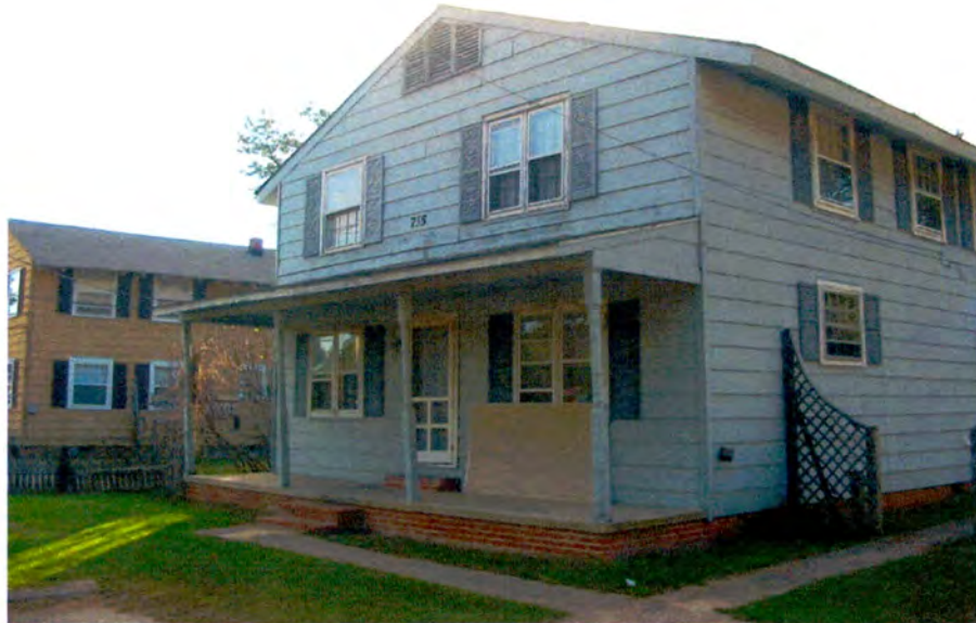
Military Houses, 700 Block, Looking West.
