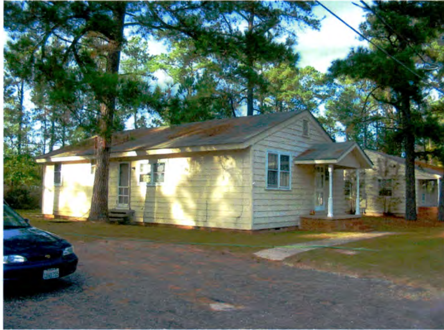
Military Houses, 800 Block, Looking North.
