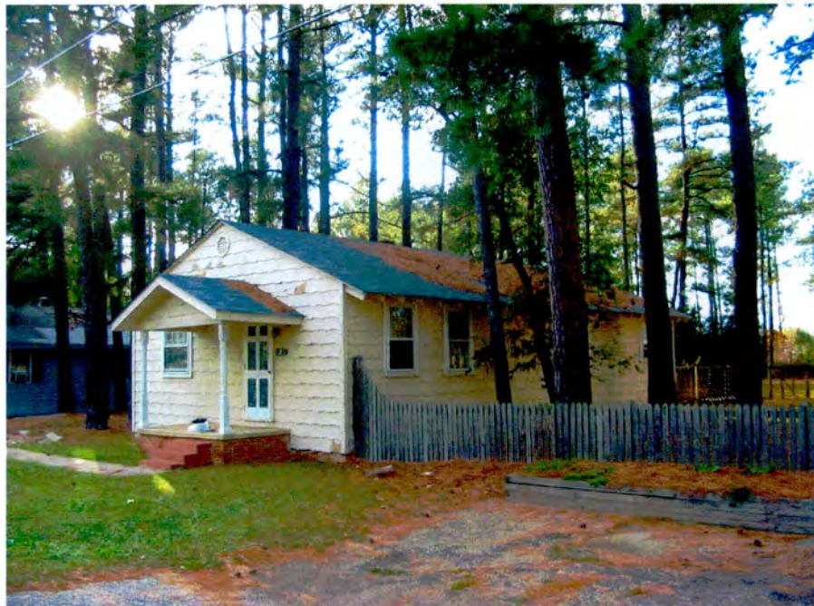
Military Houses, 839 Reilly Road, Looking West.
