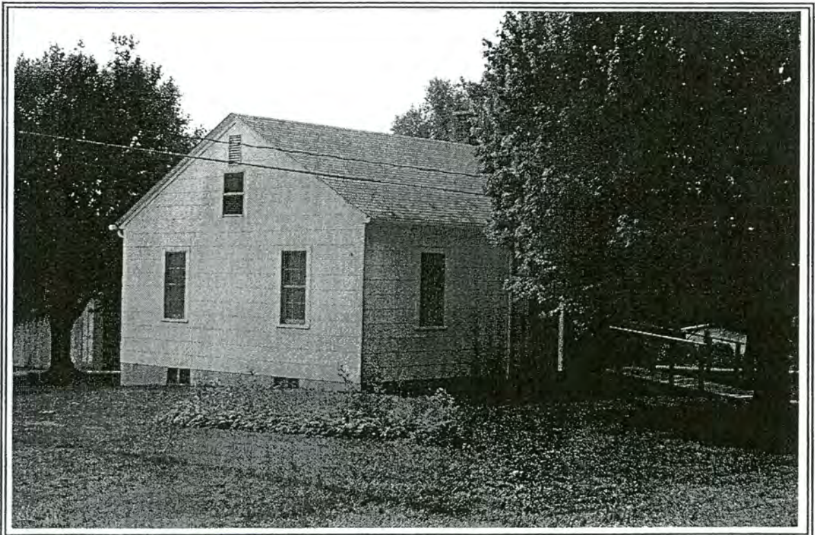
80. House, 5685 Luperville Drive
