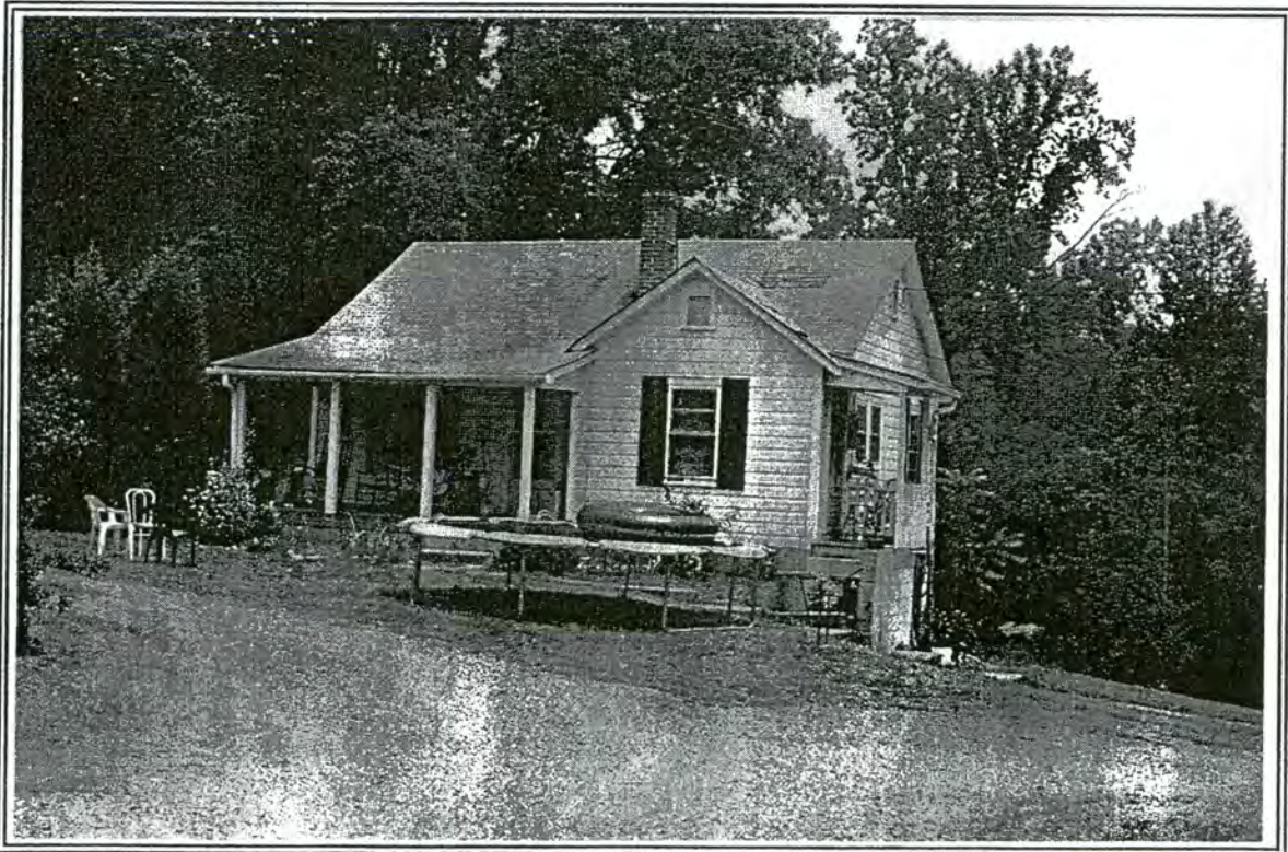
142. House, SE corner Robinhood Road and Lyndale Road
