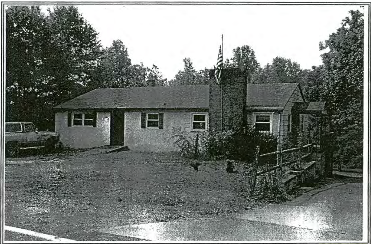
92. House, 5940 Kinney Road
