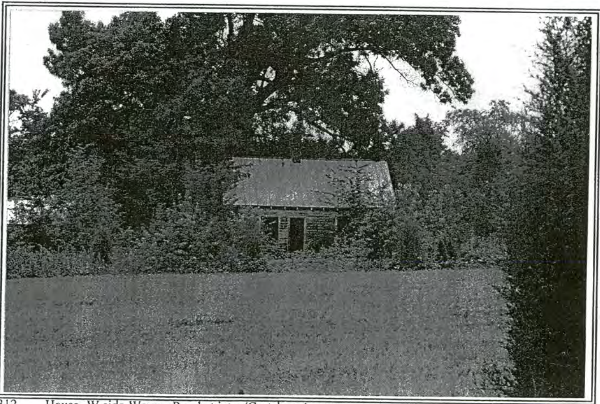
312. House, W side Warner Road at jct w/Gretchen Avenue
