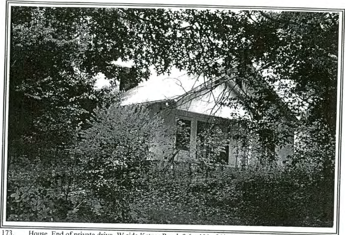
173. House, End of private drive, W side Ketner Road, 0.6 mi N of Shallowford Road
