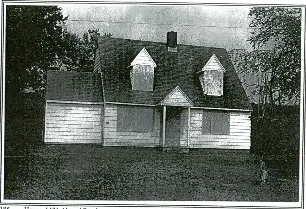
185. House, 1481 Algood Road
