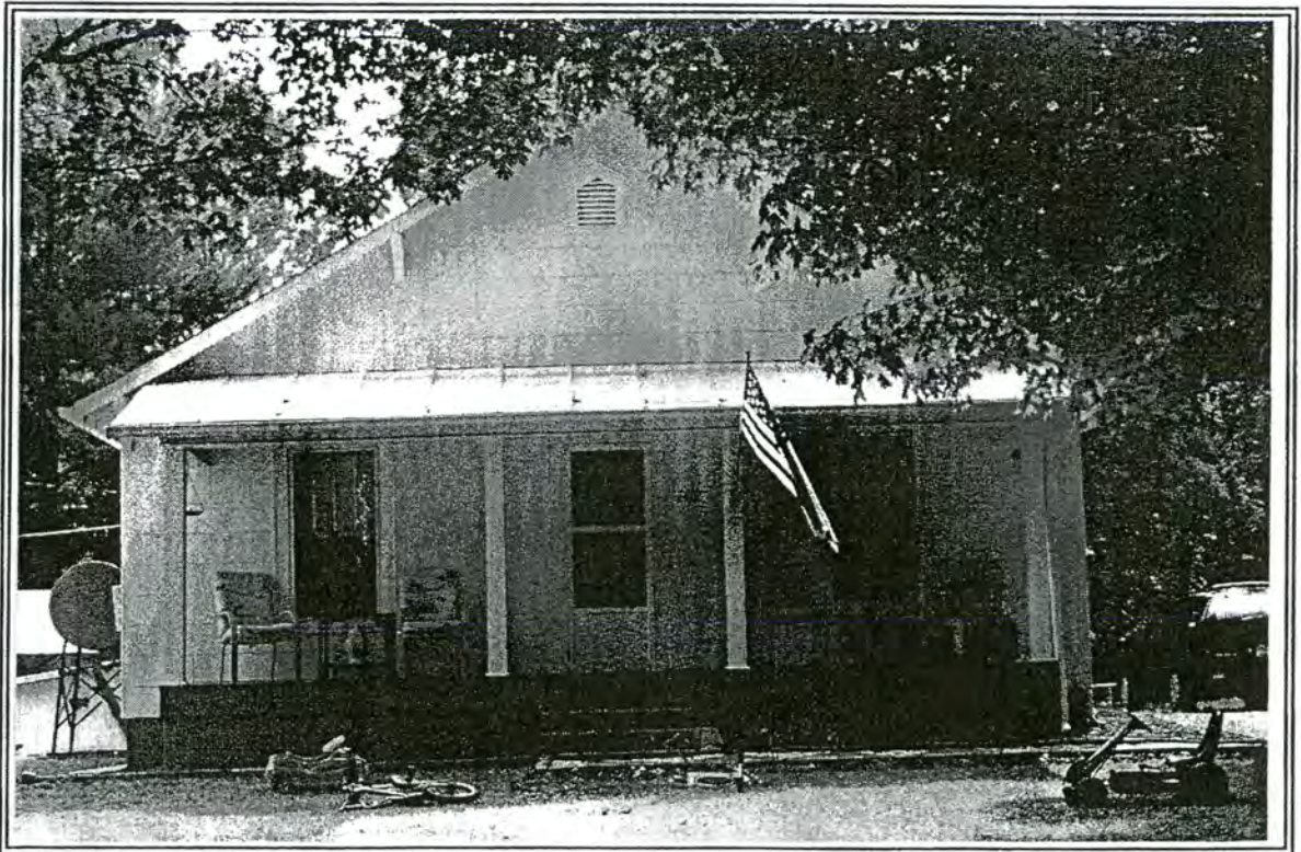
219. House, 2801 Kecoughtan Road
