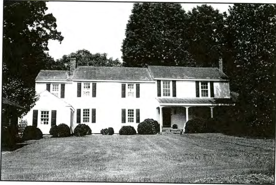
Clayton House, South Elevation
