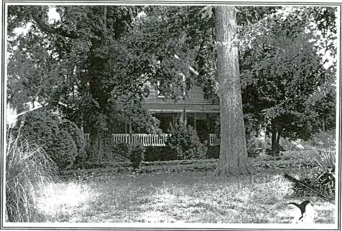
289. House, 1615 Mizpah Church Road
