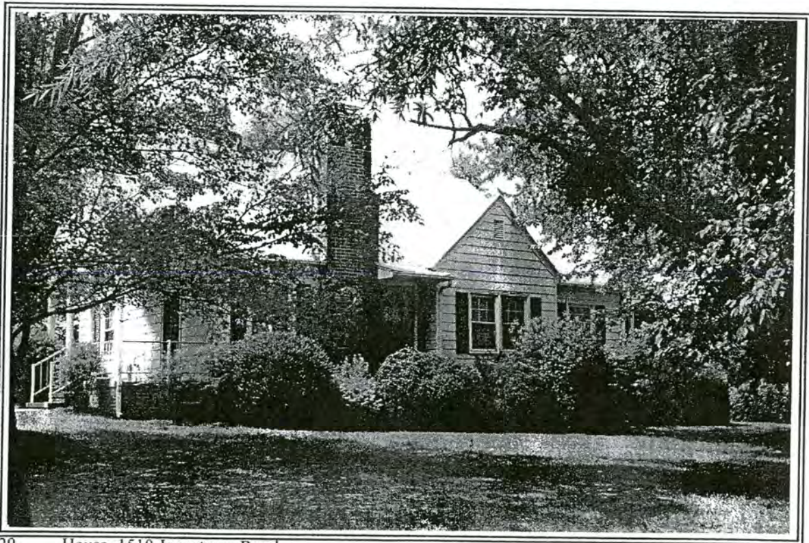
29. House, 1510 Jonestown Road
