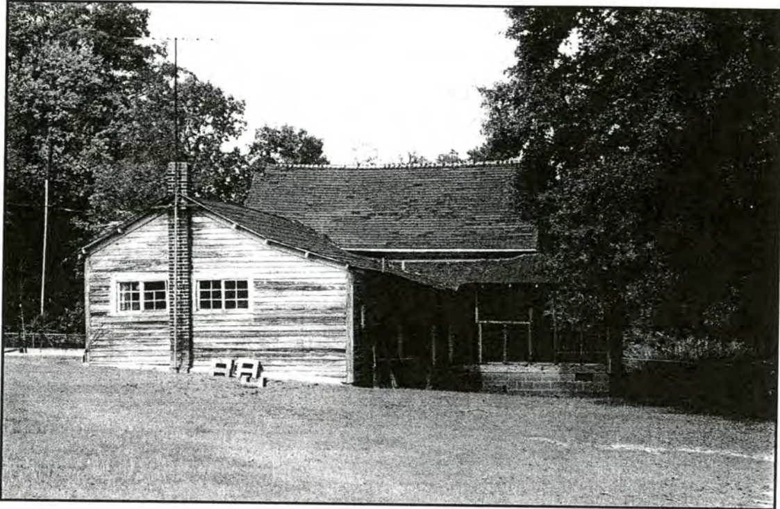
Todd House, south elevation
