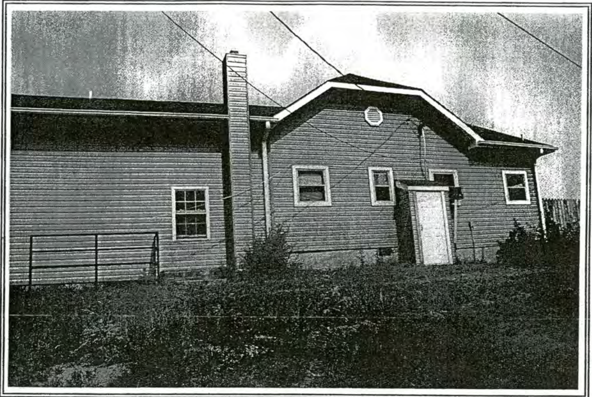
232. Store, SW corner Skylark Road and Transou Road
