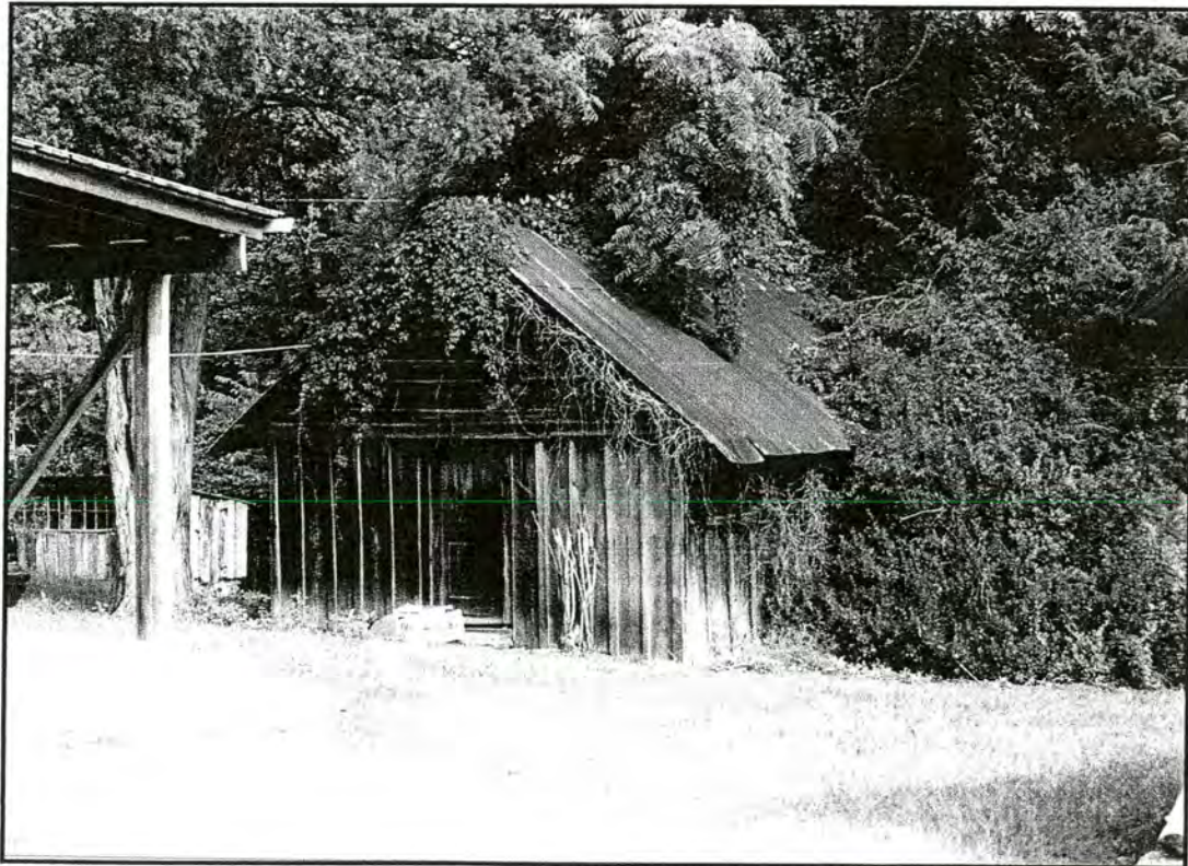
John William Kapp Farm, outbuilding, south elevation
