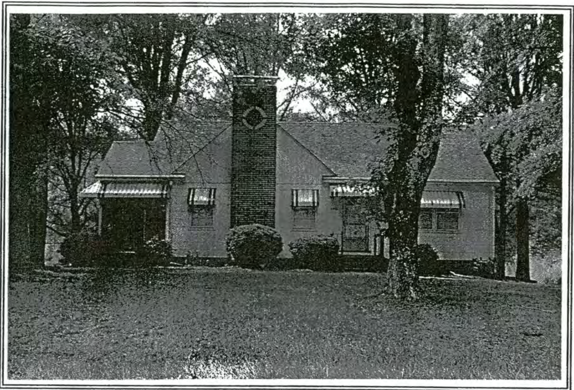
200. House, 5995 Yadkinville Road (On the edge of the APE)
