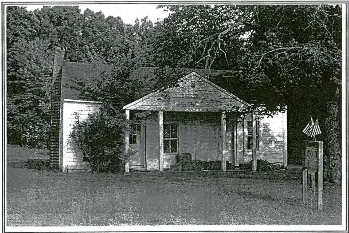
206. House, 5365 Yadkinville Road
