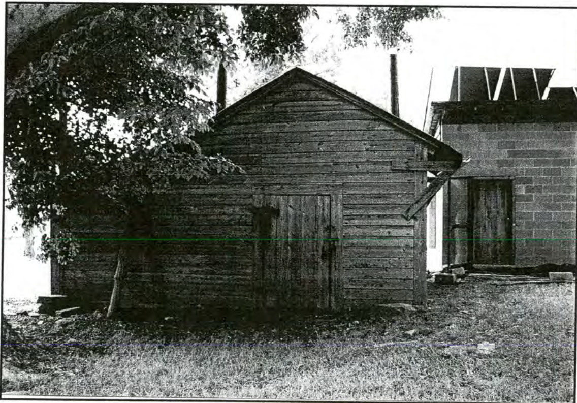
John William Kapp Farm, storage building, north elevation
