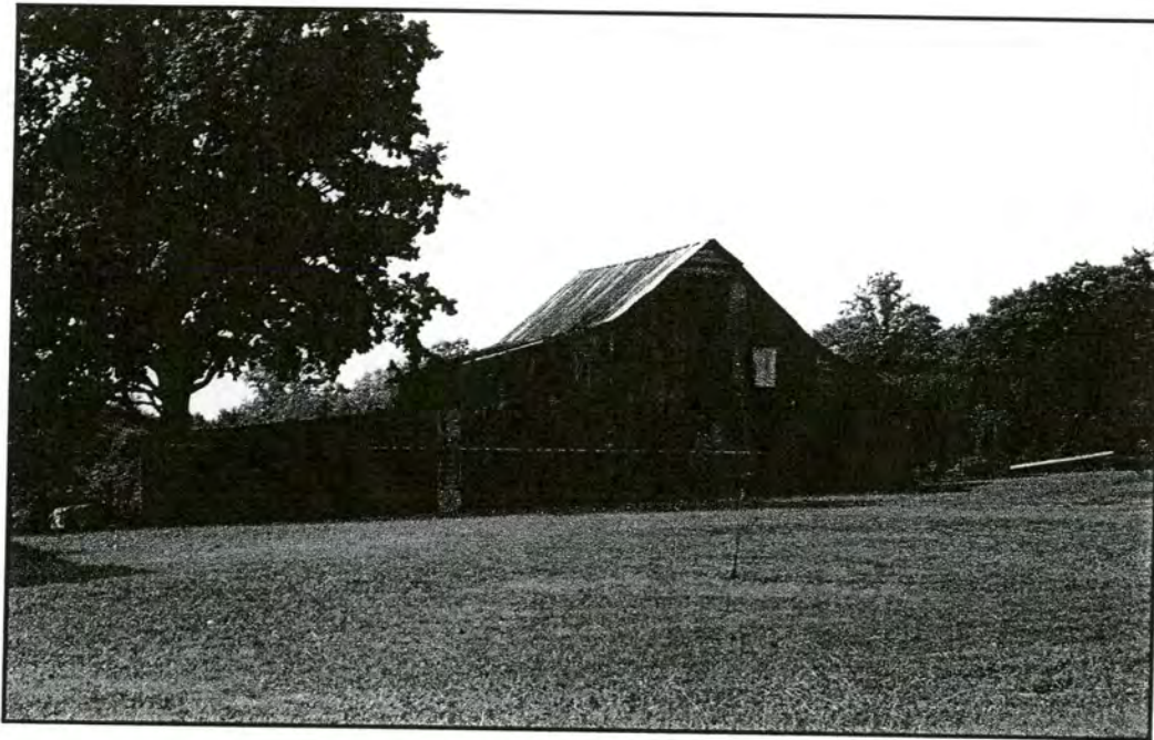
John S. Shore Farm, barn/granary
