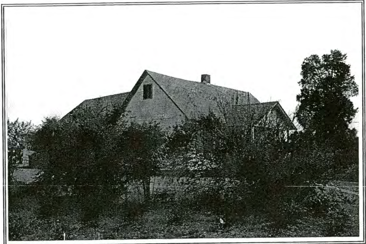
109. House, Behind 4801 Lewisville Clemmons Road
