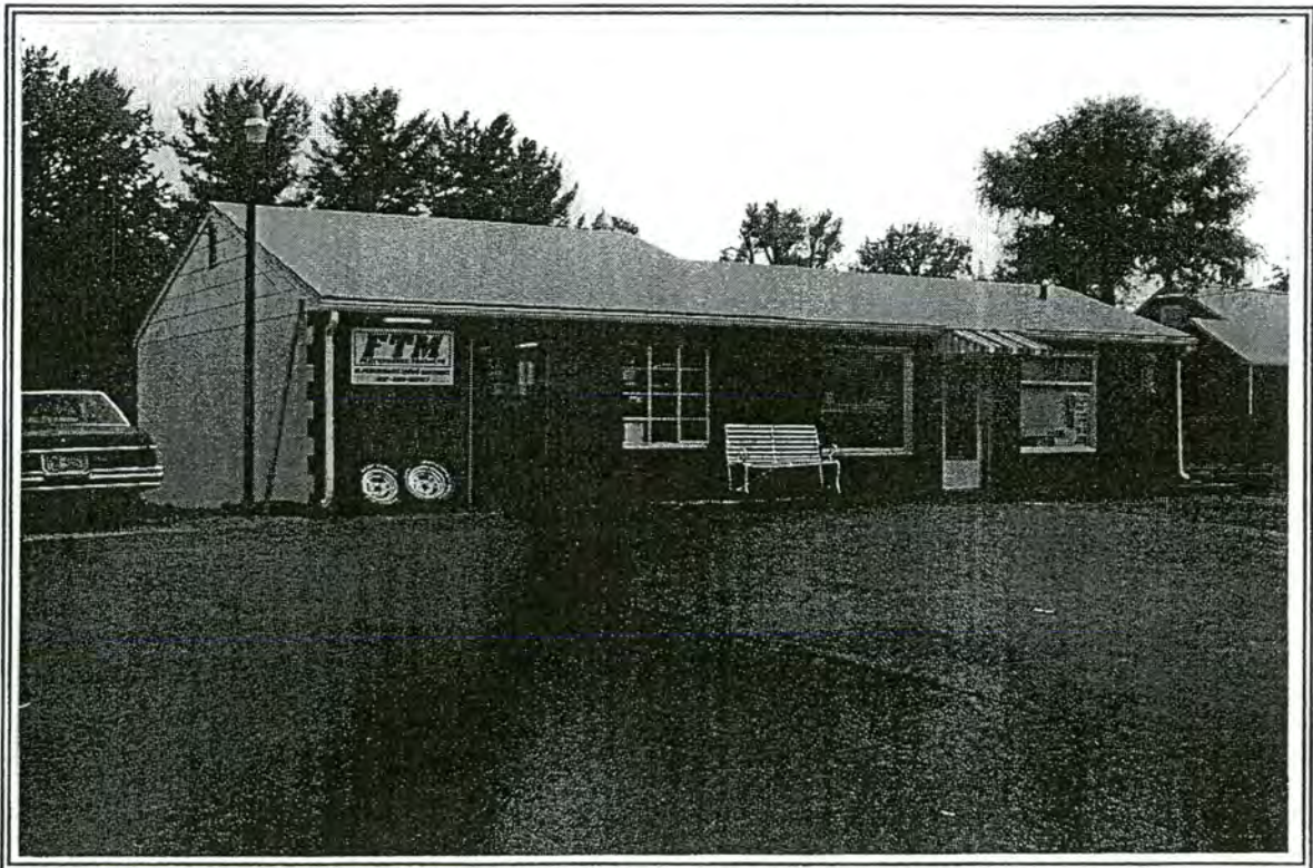
203. Commercial Building, 5800 Yadkinville Road
