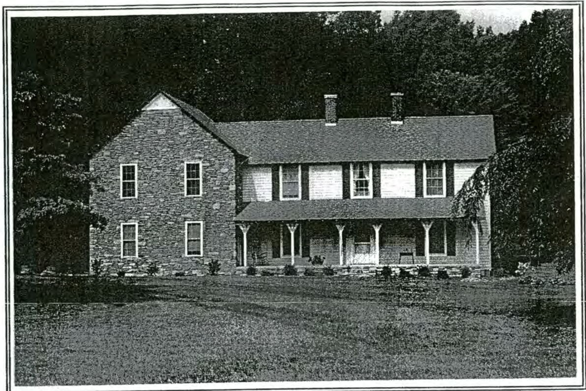
220. House, 2812 Kecoughtan Road
