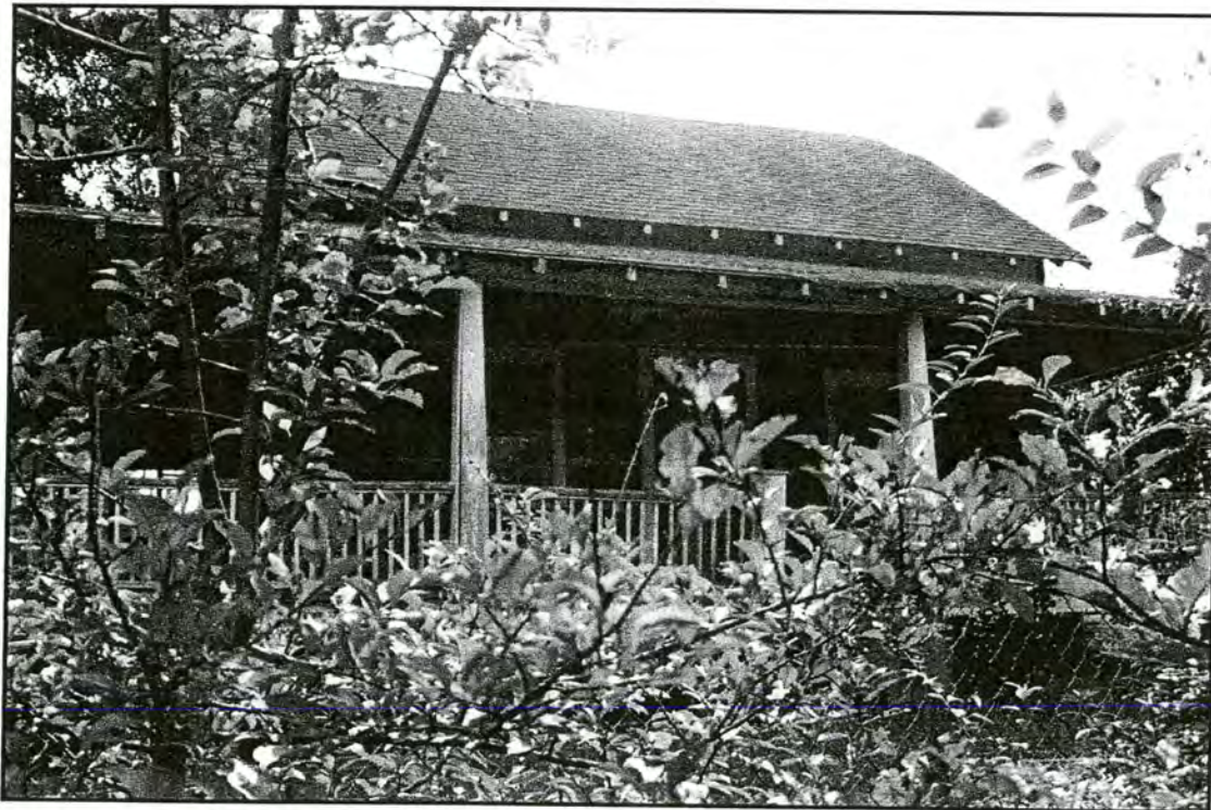
Todd House, north elevation
