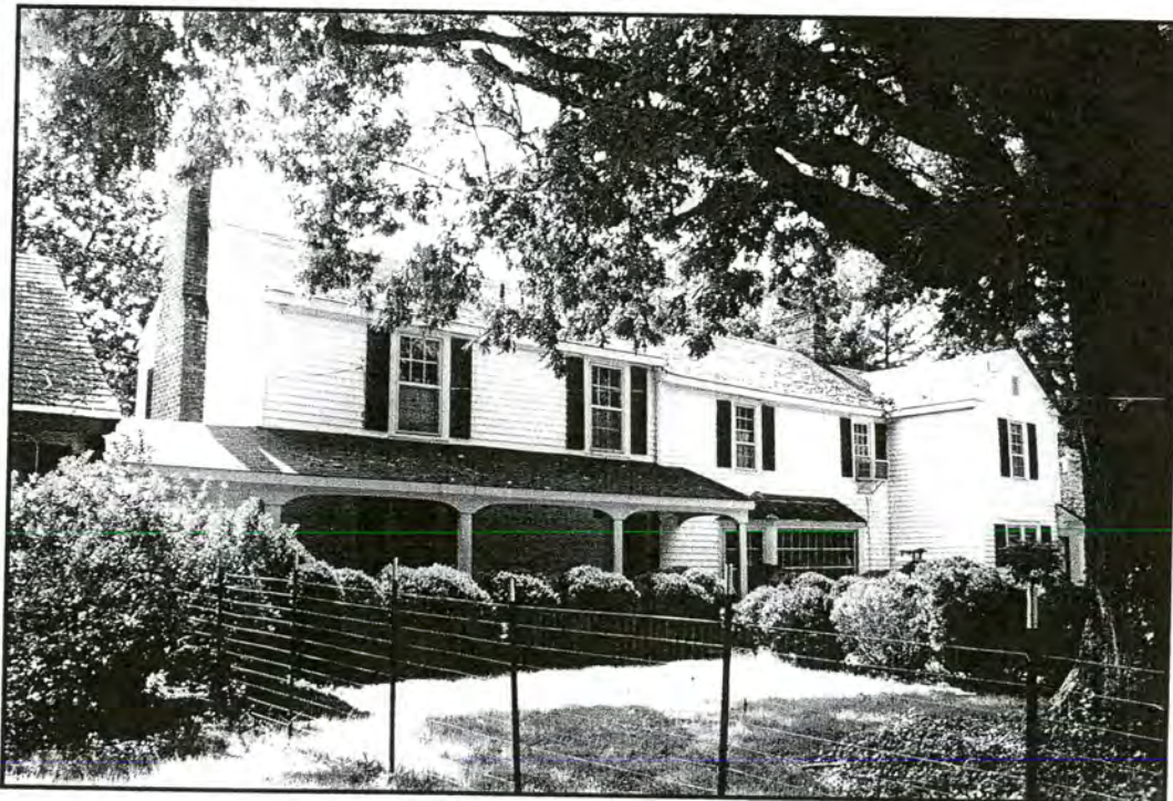
Clayton House, North Elevation
