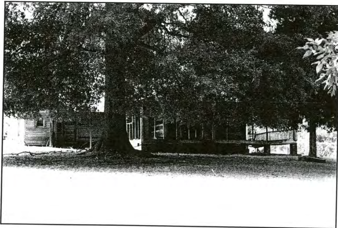
Todd House, east elevation
