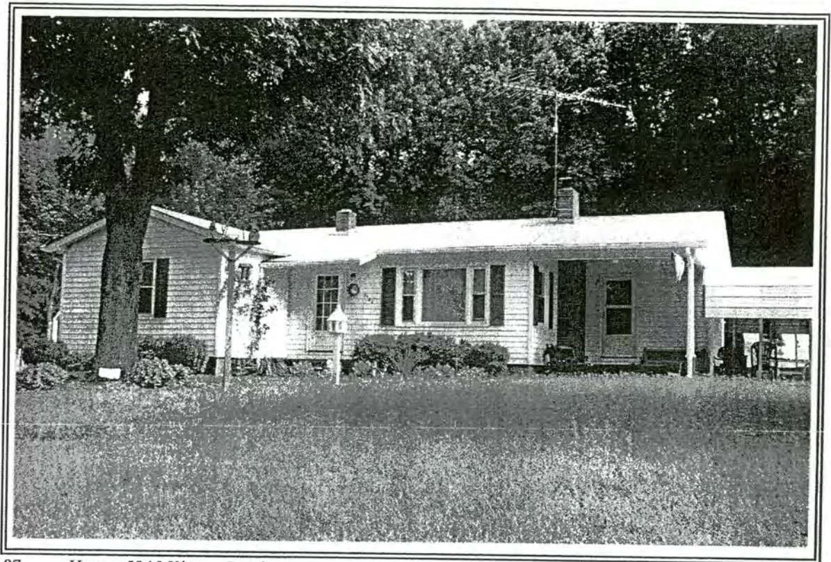
87. House, 5845 Kinney Road
