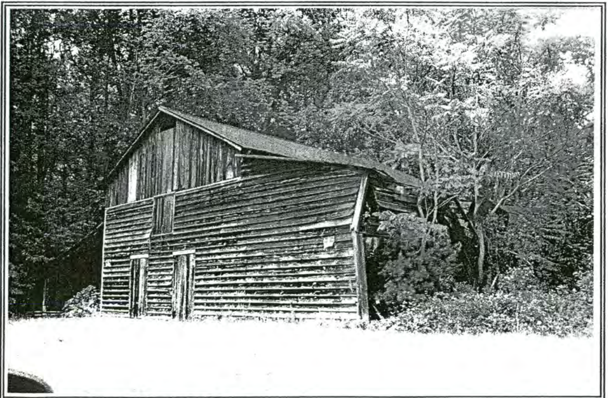
189. House (barn), 1660 Chickasha Road
