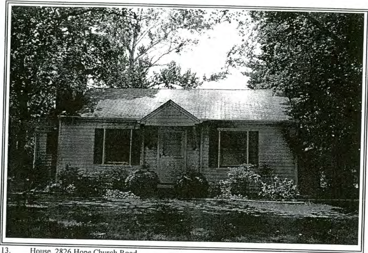
13. House, 2826 Hope Church Road
