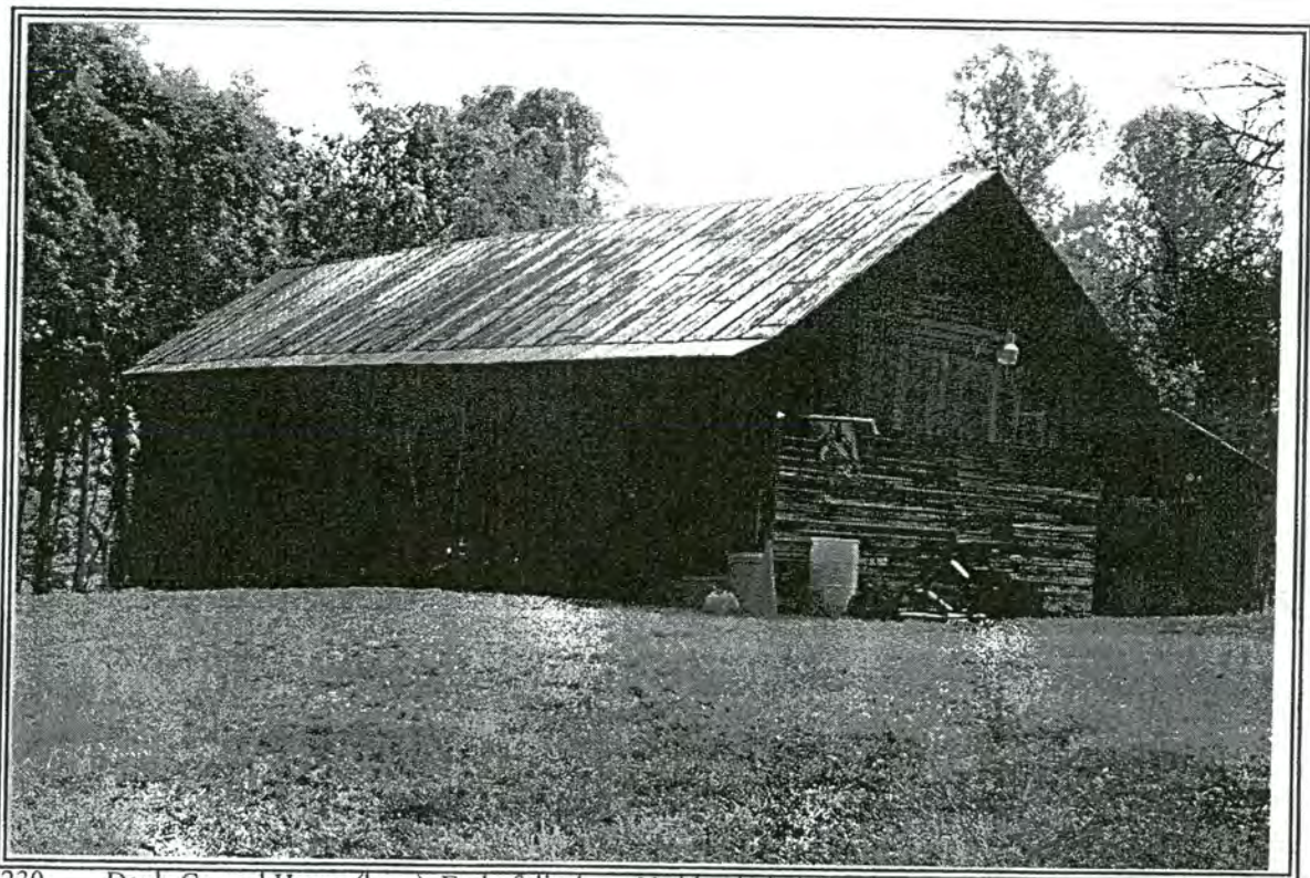
230. Daub-Conrad House (barn), End of dirt lane, N side Skylark Road, 0.2 mi W of jct w/Transou Rd
