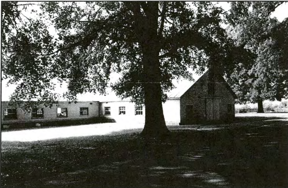
Brookberry Farm, milking parlor, north elevation
