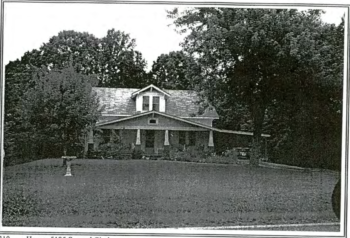
310. House, 5195 Seward Circle
