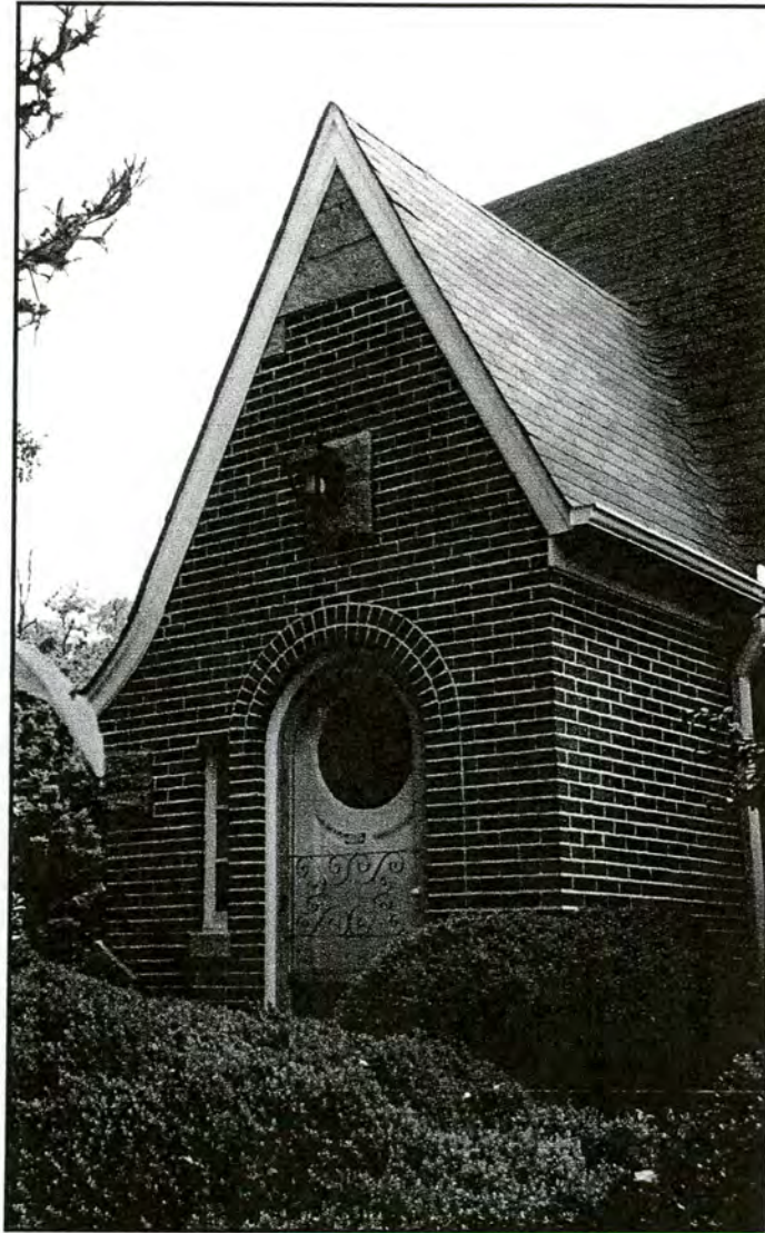
Thomas House, north elevation detail
