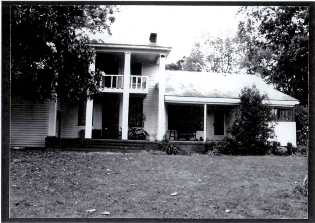
PLATE VII.4 Goodman House and Doctor's Office (#57), 1890s Block at Left, 1830s Block at Right, North Front Elevation
