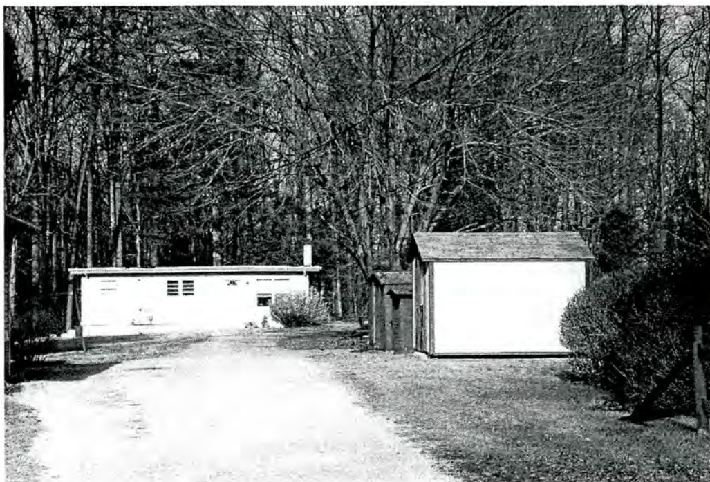
Property 43. House, circa 1960, 5504 Keren Drive, and Property 42 Outbuildings
