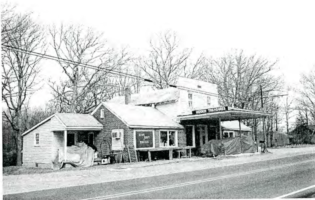
Property 87. Commercial Building, circa 1922, 5103 Summit Avenue
