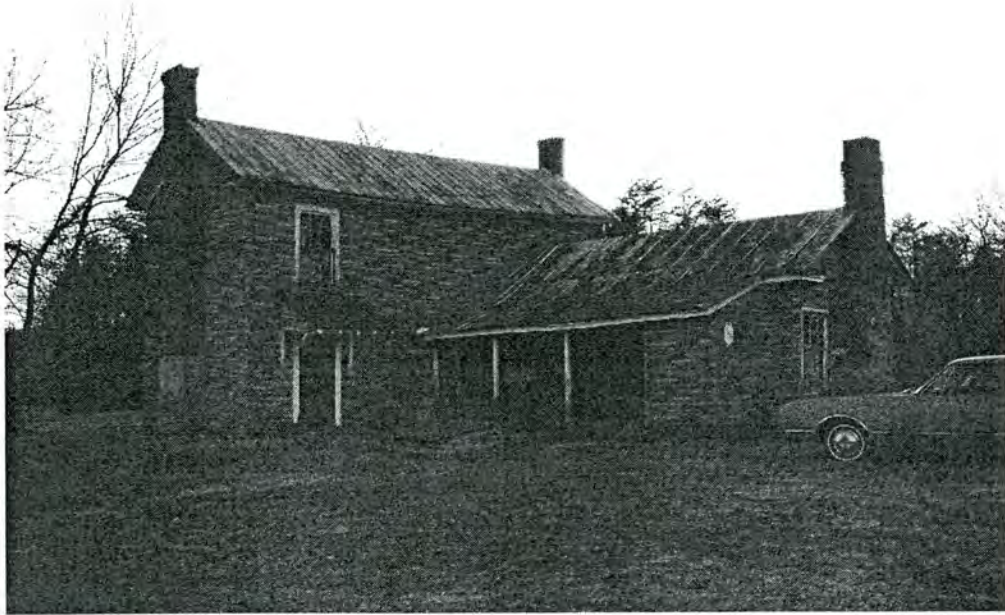
Schoolfield-Hatcher House, East Elevation
