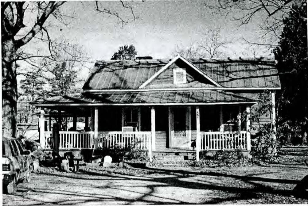
Holt-Baldwin House, South Elevation
