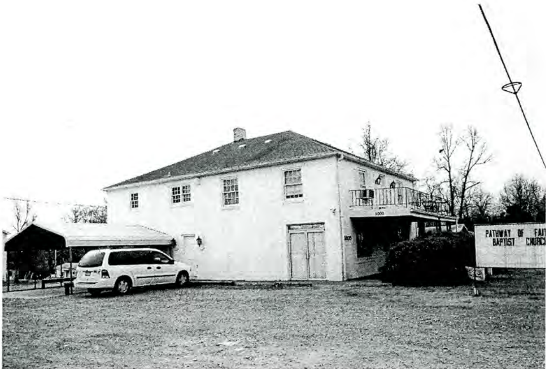
Property 89. Commercial Building, circa 1949, 5000 Summit Avenue
