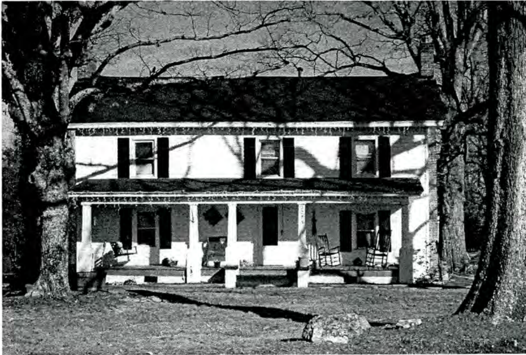
Property 3. Rierson House (GF 1833), circa 1881, 2223 Huffine Mill Road
