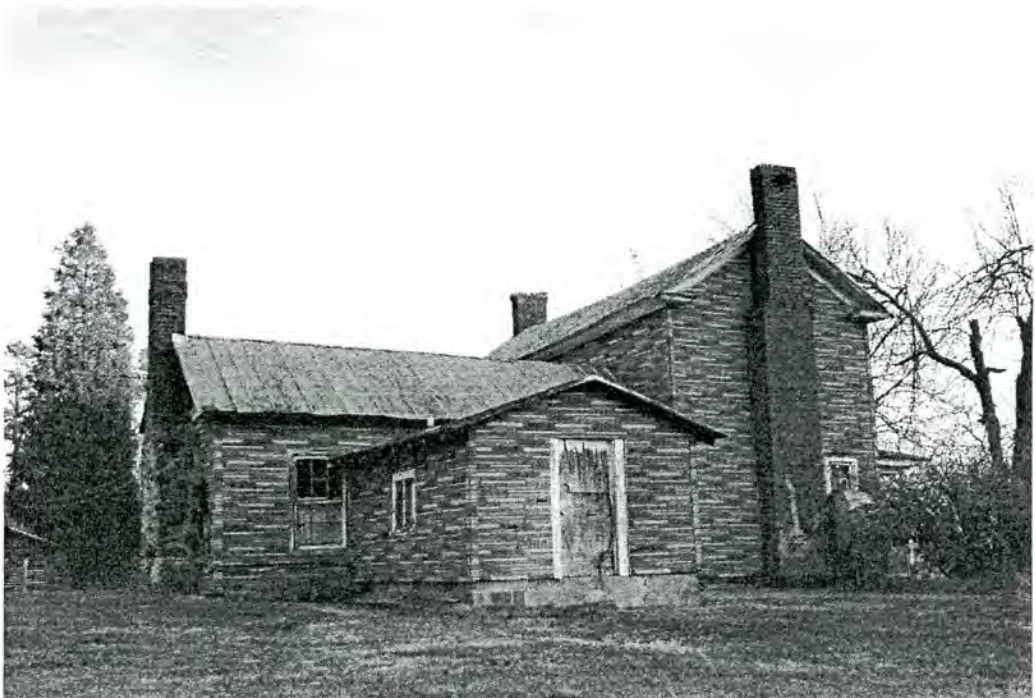
Schoolfield-Hatcher House, West Elevation
