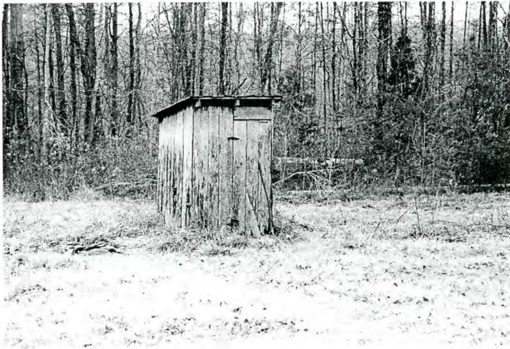
Property 56. William Clymer Privy, circa 1917, 4623 US Highway 29 North
