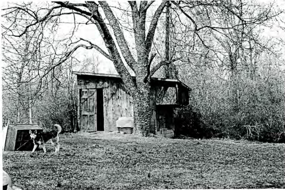
Modern Shed North of Dr. C. I. Carlson Cabin
