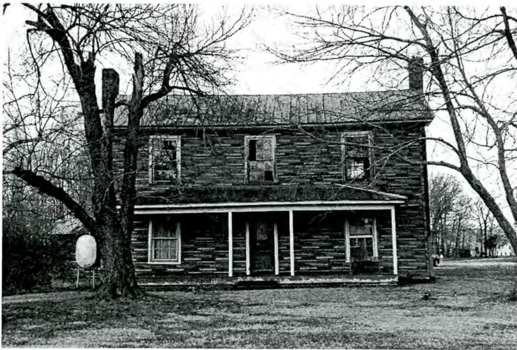
Schoolfield-Hatcher House, Façade (South Elevation)
