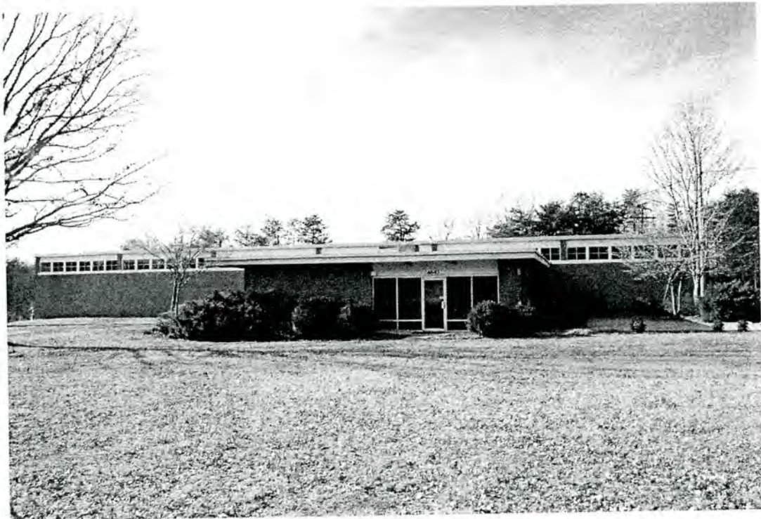
Property 36. Industrial Building, circa 1956, 4643 US Highway 29 North
