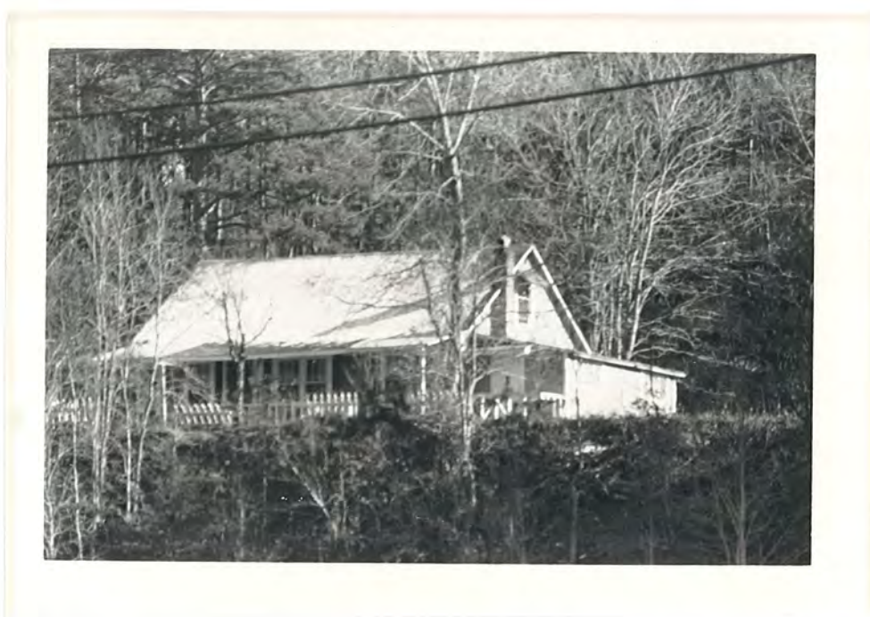
Plate 5. House No. 5, Looking South.
