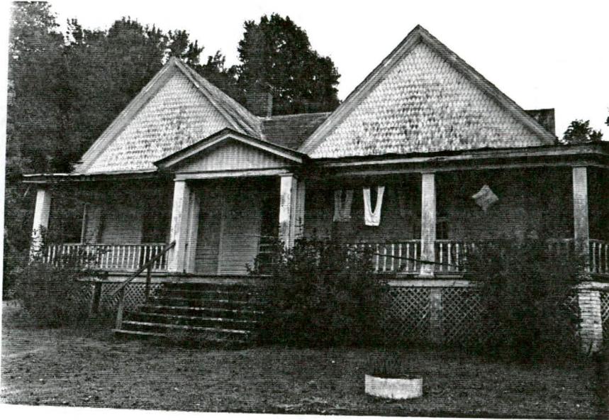
Plate 6. George Fleming House, Facade, Looking South.
