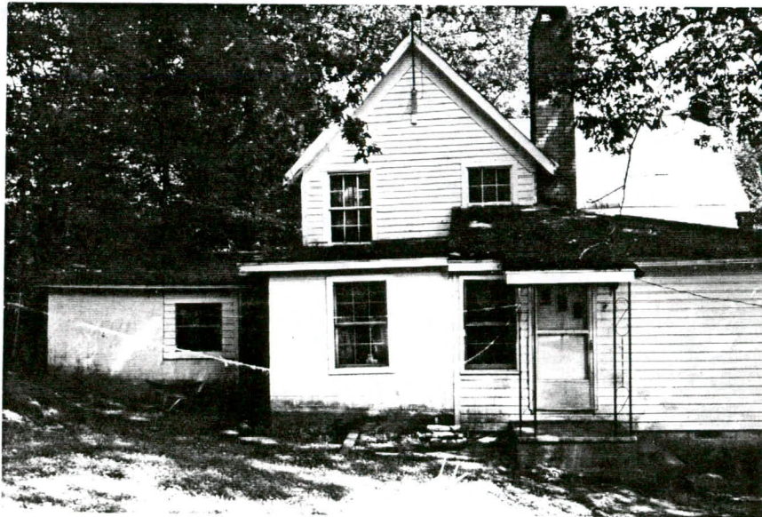
Plate 25. Alfred Morgan House, Rear Elevation, Looking North.
