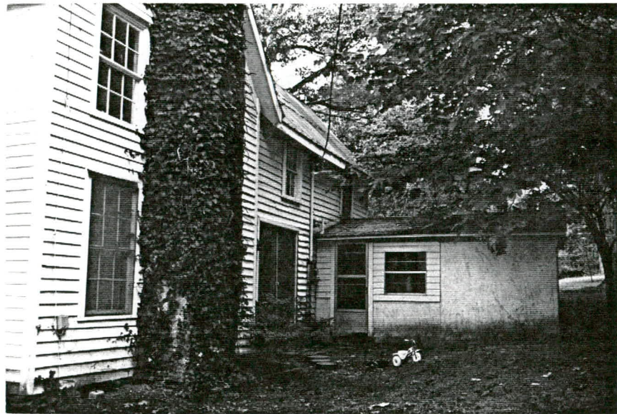
Plate 22. Alfred Morgan House, West Elevation and Rear Wings, Looking Southeast.
