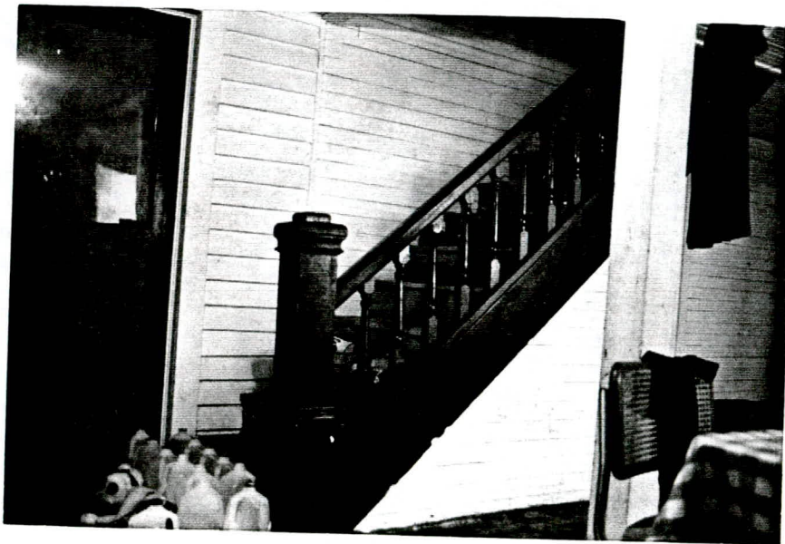
Plate 13. George Fleming House, Rear Staircase.
