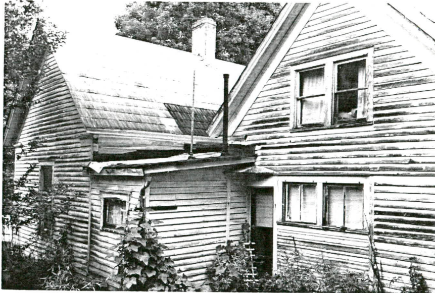
Plate 10. George Fleming House, Rear Elevation, Looking North.
