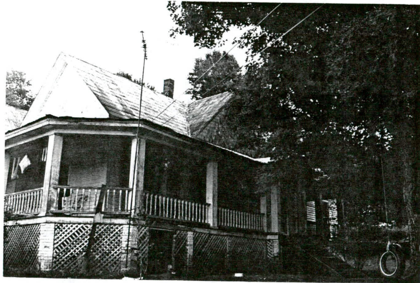
Plate 8. George Fleming House, West Elevation, Looking Southeast.
