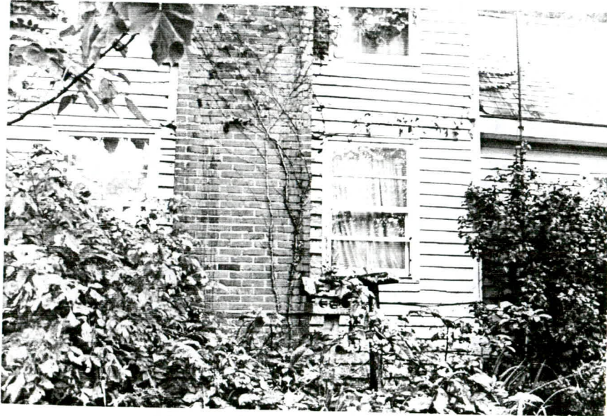
Plate 15. McCombs House, North Elevation, Looking South.
