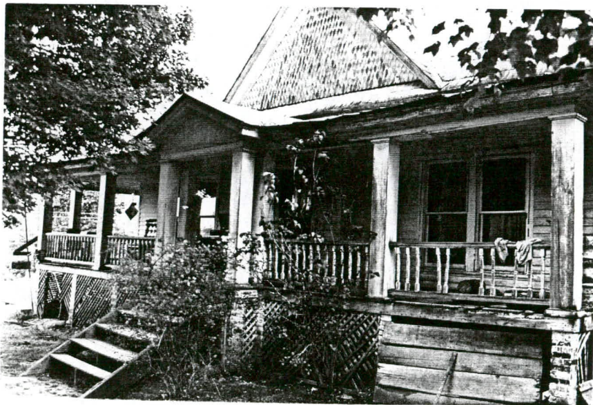
Plate 7. George Fleming House, Facade, Looking Southeast.
