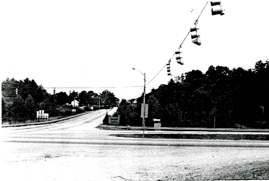
Plate 4. Western Terminus of Project, Looking West Towards Murphy.
