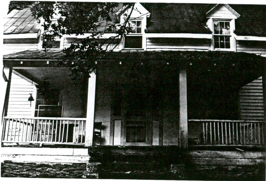
Plate 21. Alfred Morgan House, Facade, Looking South.
