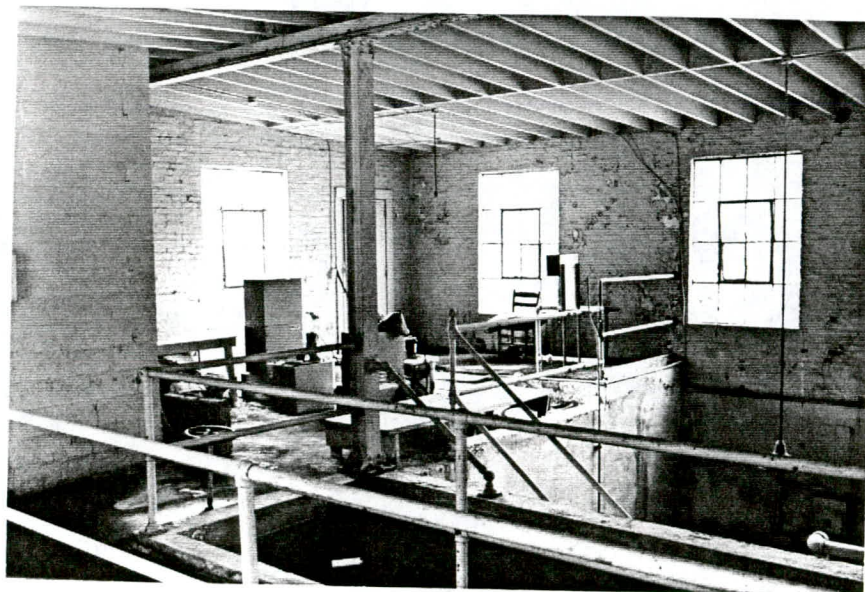
Plate 31. Water Treatment Plant, Interior of 1925-1926 Section.
