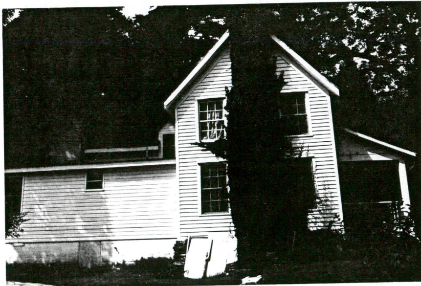
Plate 23. Alfred Morgan House, East Elevation, Looking West.
