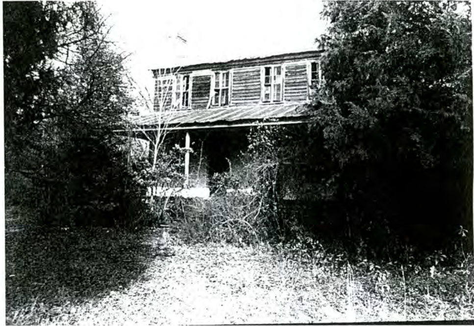
55-C. Eli Gibson House, facade, view to N
