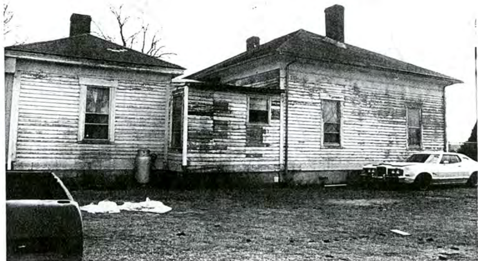
53-C. Bullard Family House, NW elevation, view to S
