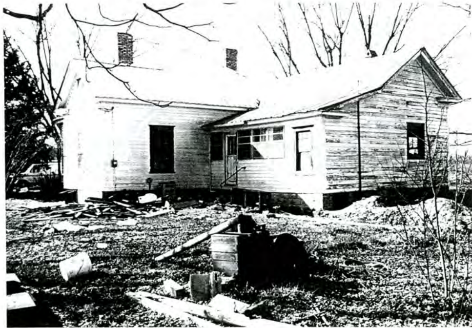
54-C. H. L. Rush House, rear view to W
