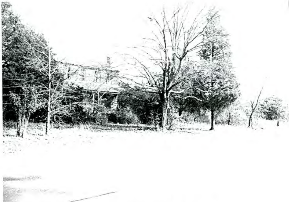
55-B. Eli Gibson House, context view to E
