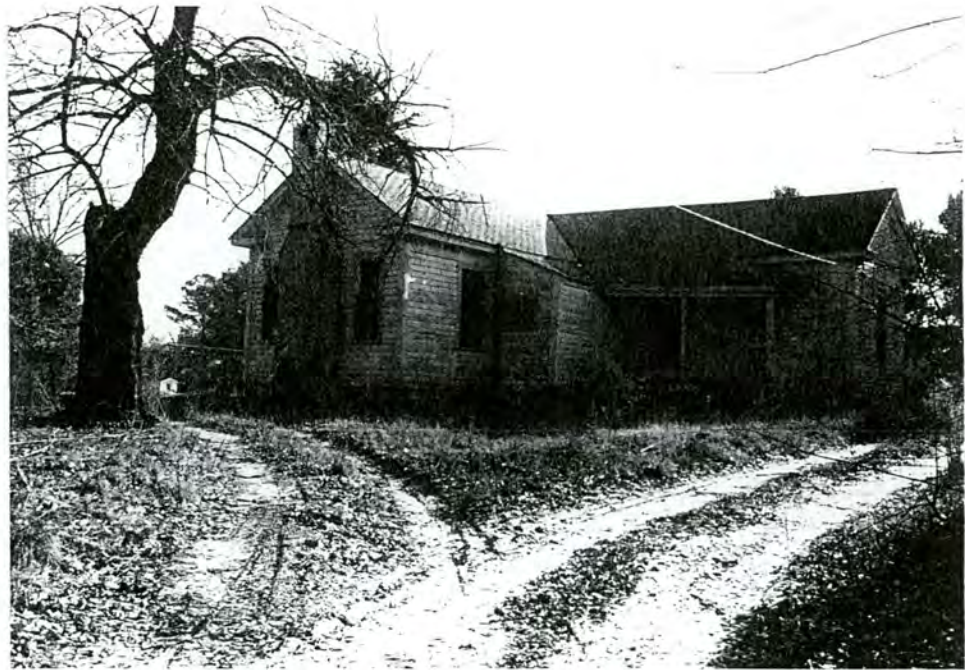
127-B. Thomas Franklin Boyd House, overall rear view to E
