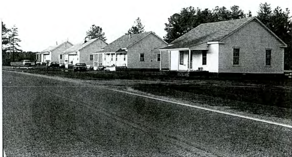
73-A. Morgan Mill Houses, overall view to N
