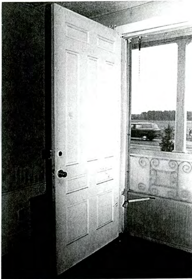
53-F. Bullard Family House, front door, view to S
