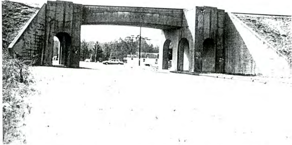
82-A. Seaboard Air Line Railway Overpass, overall view to SW
