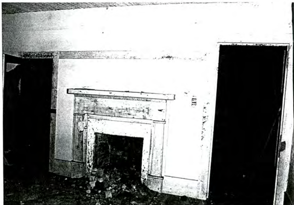
55-I. Eli Gibson House, dining room mantel, view to NE
