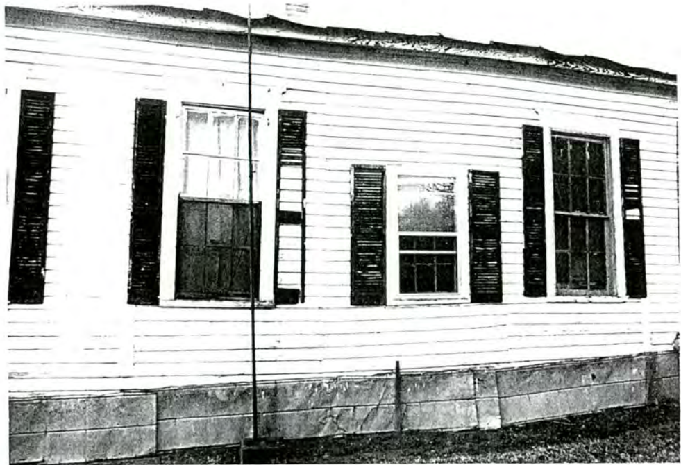
63-B. House, detail of SE elevation
