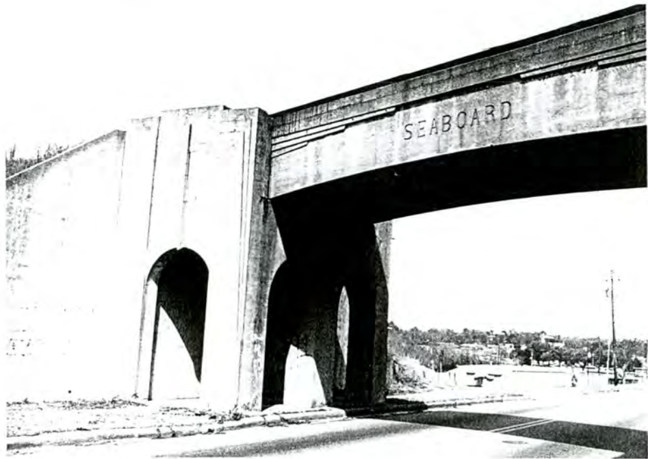
82-B. Seaboard Air Line Railway Overpass, detail, view to N
