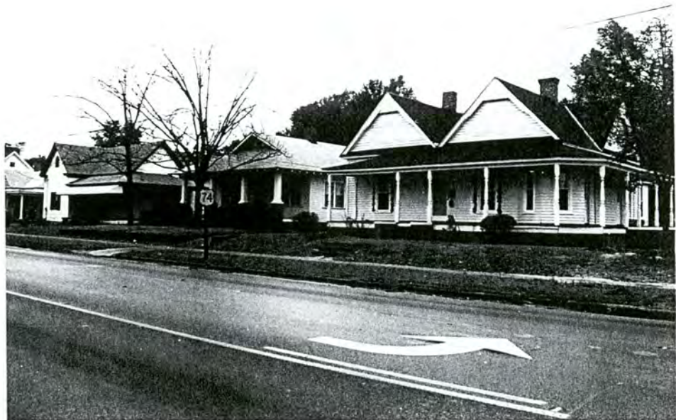
93-112-C. W. Hamlet Ave. Residential Area, 300 block, view to NE
