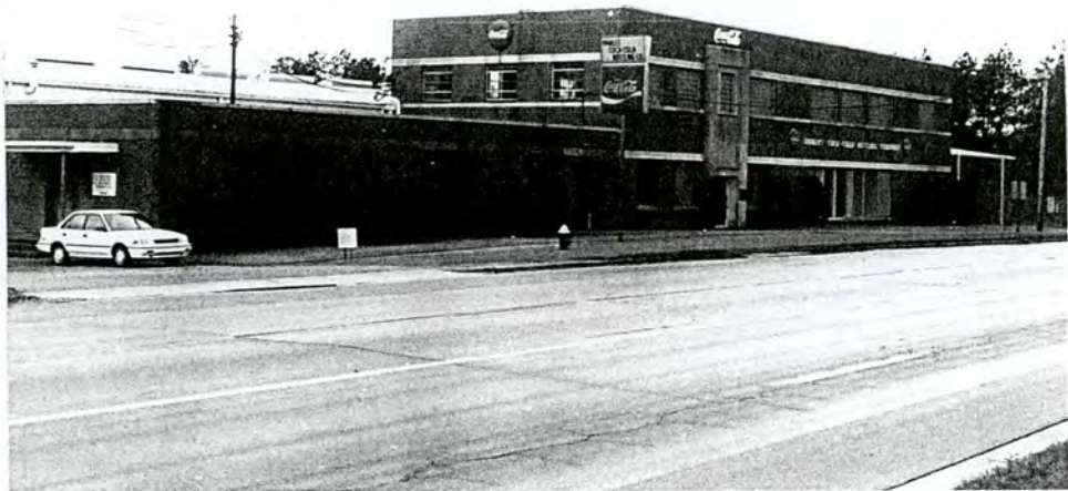
84-A. Hamlet Coca Cola Bottling Company Plant, overall view to SW
