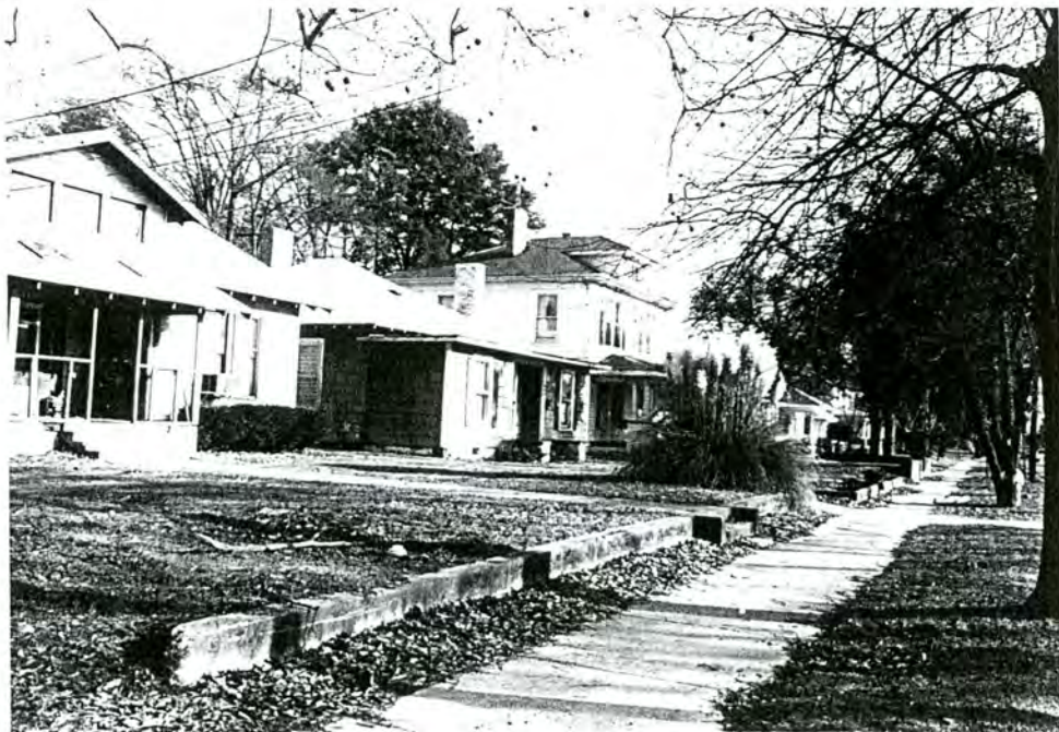
93-112-E. W. Hamlet Ave. Residential Area, 500 block, view to SE
