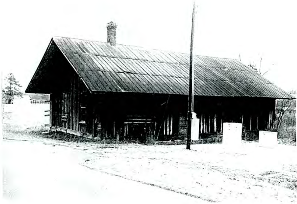
41-B. Ghio Depot, overall view to E
