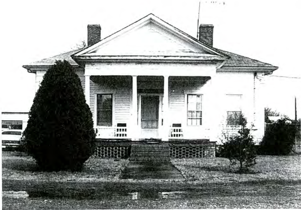
53-B. Bullard Family House, facade, view to NE
