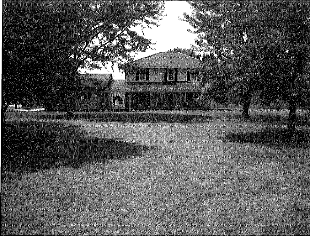
Figure 7. Structure LC-1, facing southwest.
