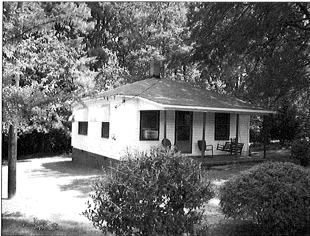
Figure 9. Structure LC-3, facing east.
