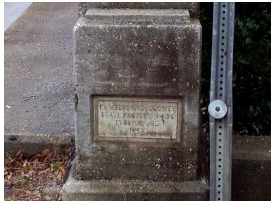
Property No. 49 – Bridge No. 116
