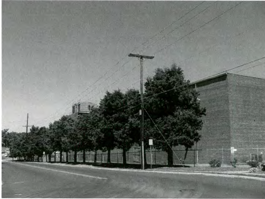
Plate 5. Voorhees Manufacturing Company, Modern Building, Looking Northwest Along Parker Street.
