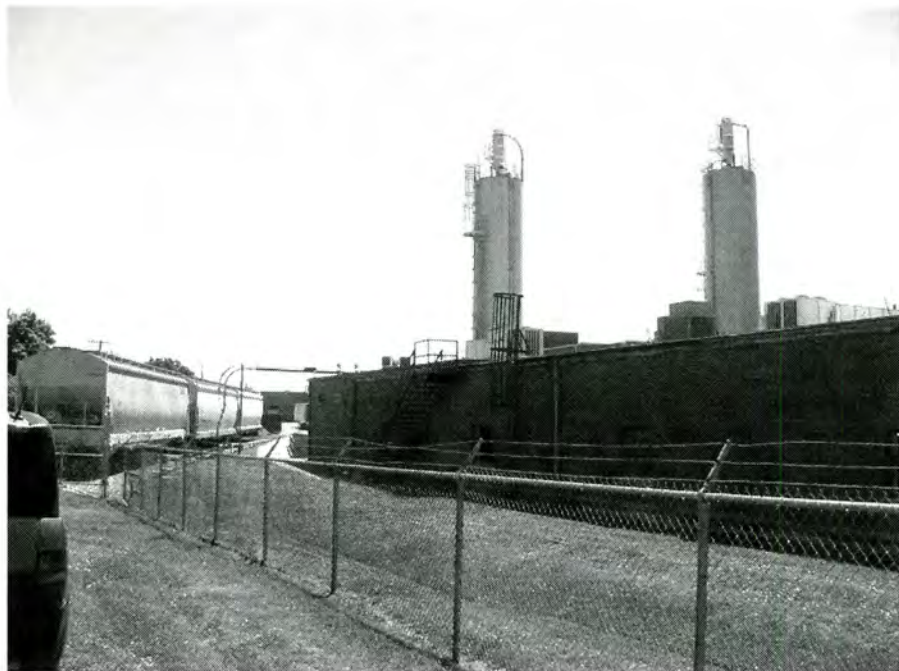
Plate 2. Voorhees Manufacturing Company, Modern Additions, Looking Southeast.
