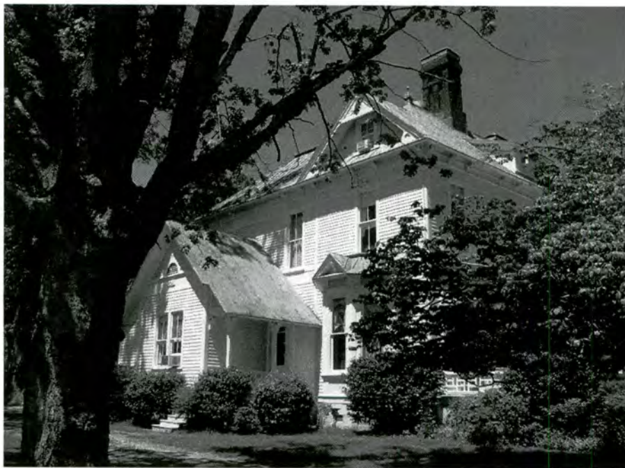
Plate 8. Dr. Edward C. Laird House, Side (South) Elevation, Looking Northwest.
