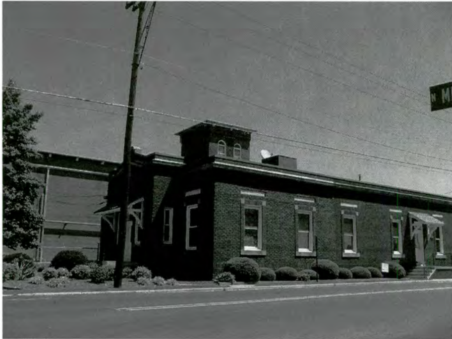
Plate 3. Voorhees Manufacturing Company, Office, Looking North.
