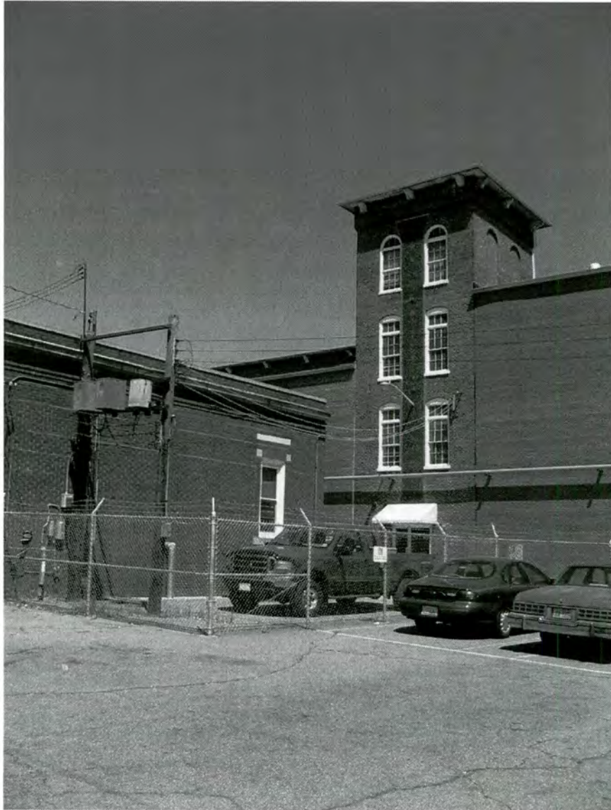
Plate 6. Voorhees Manufacturing Company, Office and Stair Tower Surrounded by Modern Additions, Looking North.
