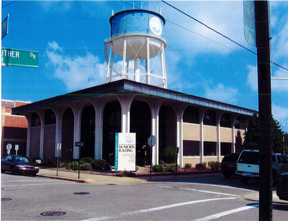
Property No. 31 – Albemarle Savings and Loan Building. Northwest corner of E. Colonial Avenue and N. Martin Luther King Street.
