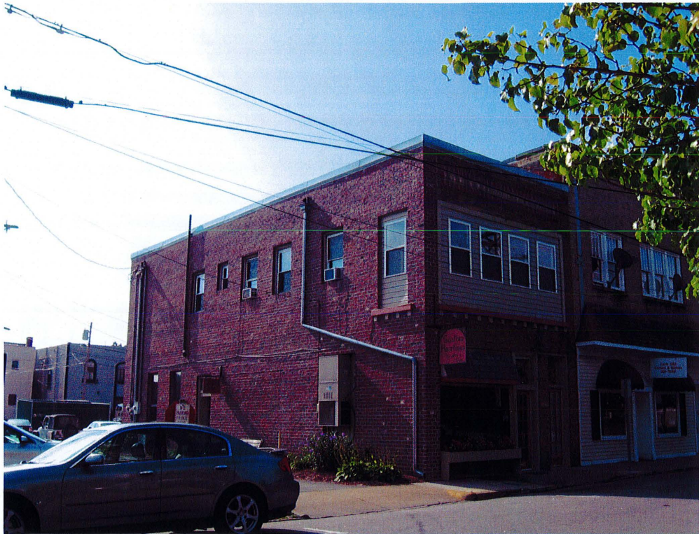
Property No. 33 – Davis Building. West (main) and north elevations.
