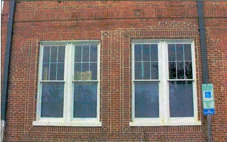
Detail of brickwork around windows
