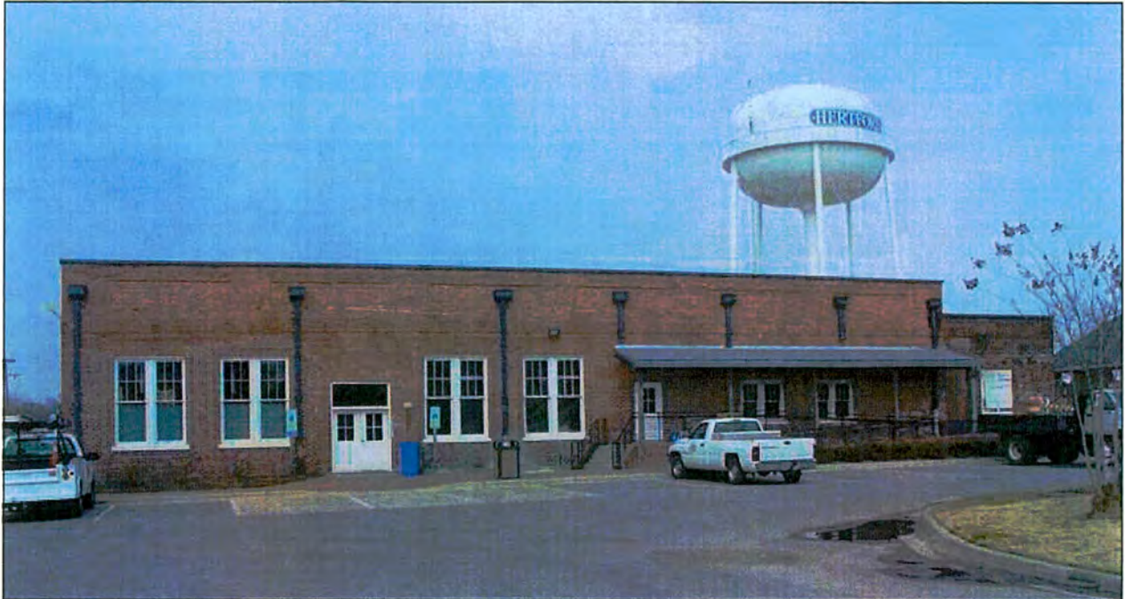
South facade of the former Hertford Water Works and Ice Plant
