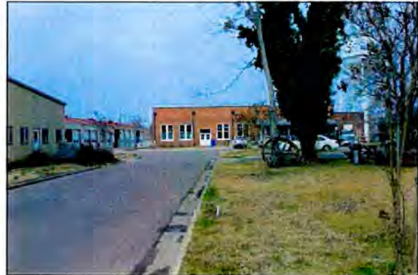
View of the former Hertford Water Works and Ice Plant from West Grubb Street
