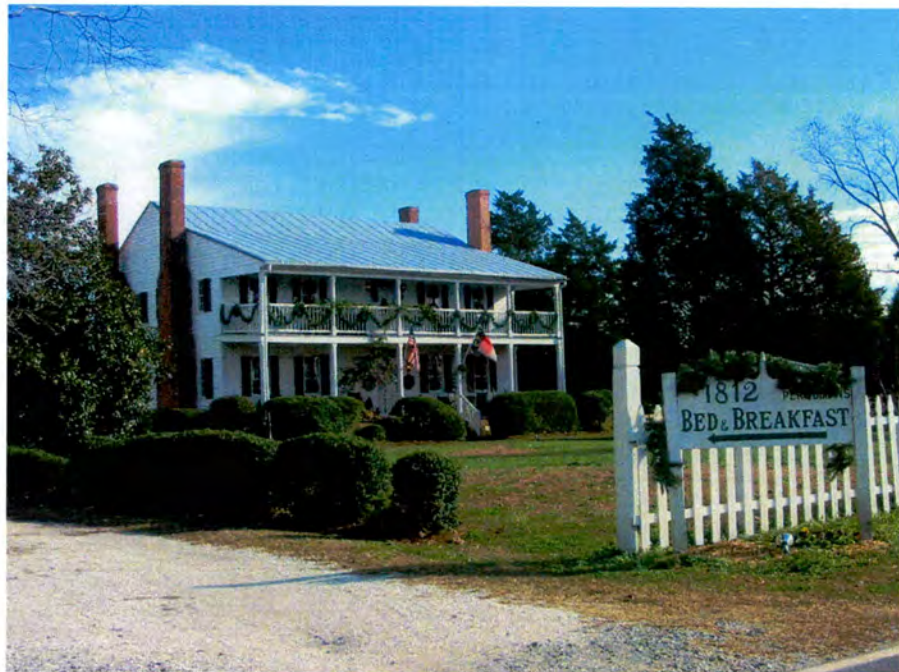
Plate 2. Old Neck Historic District, Fletcher-Skinner-Nixon House, Looking North.
