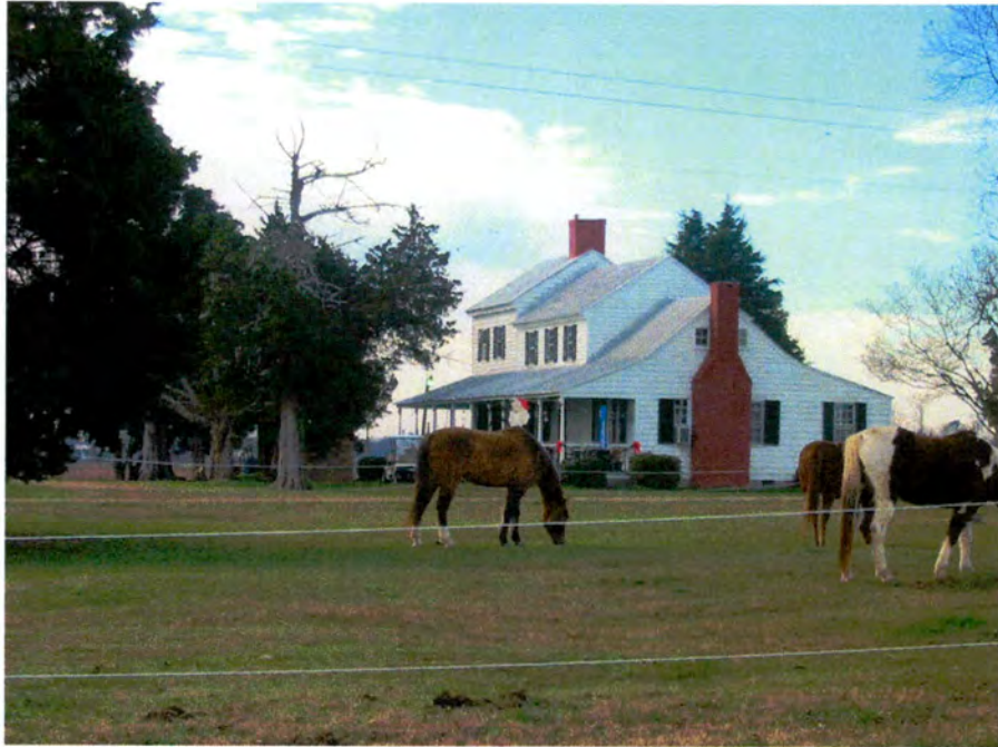
No. 3. Old Neck Historic District, Francis Nixon Plantation, House, Looking South.
