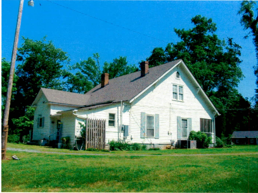
Plate 3. Rogers House, Side (West) and Rear (North) Elevations, Looking Southeast.
