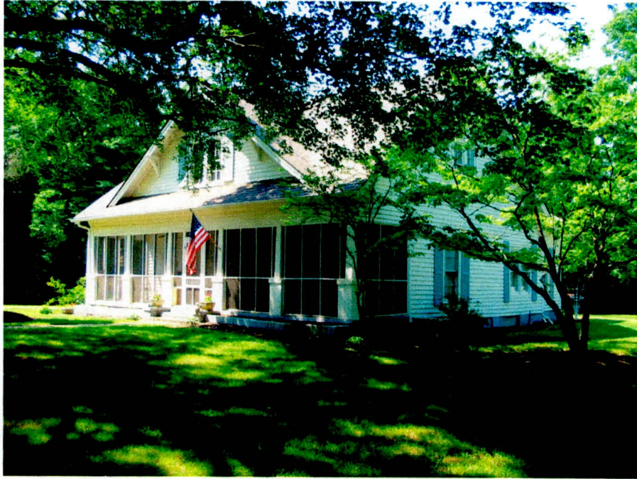
Plate 5. Rogers House, Facade and Side (East) Elevation, Looking Northwest.
