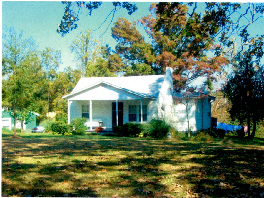
Plate 9. House No. 4, House and Setting, Looking East.
