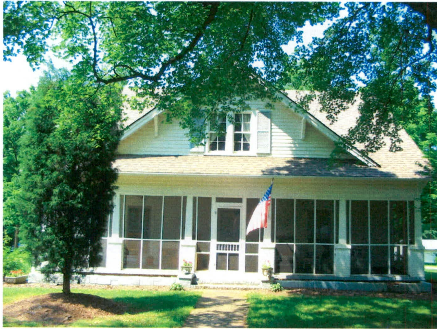
Plate 1. Rogers House, Facade, Looking North.
