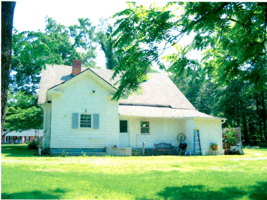
Plate 4. Rogers House, Rear (North) Elevation, Looking South.
