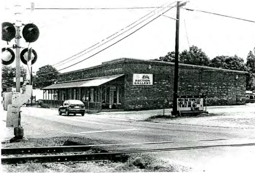
Plate 1. James Orr Stores, Facade and South Elevation, Looking Northeast Across Railroad Tracks.
