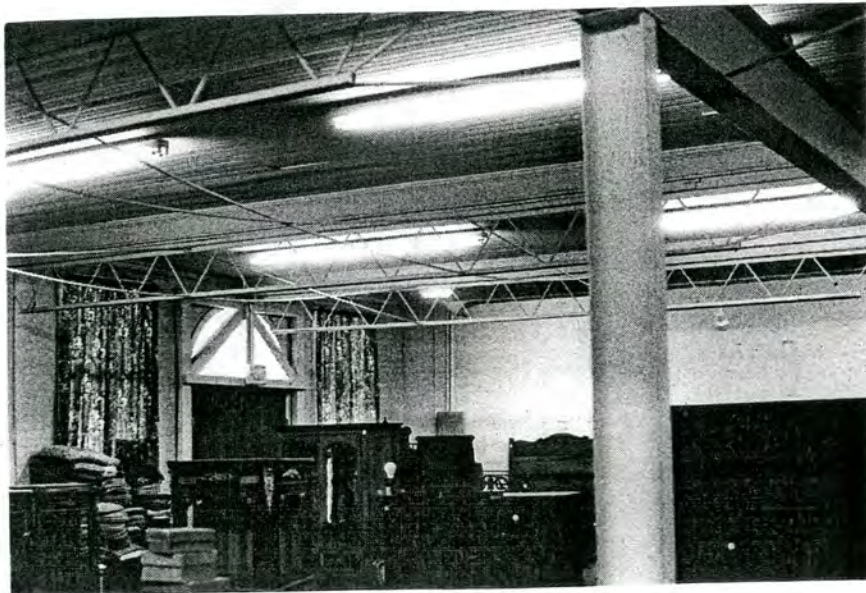
Plate 8. James Orr Stores, Interior, Northern Unit, Showing Roof Trusses.
