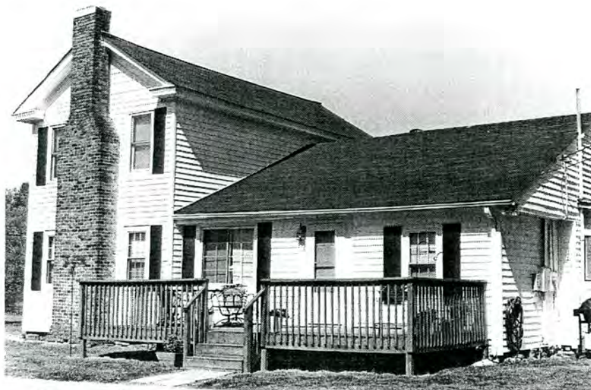
Plate 40. Stinson House, East Elevations, Looking West.
