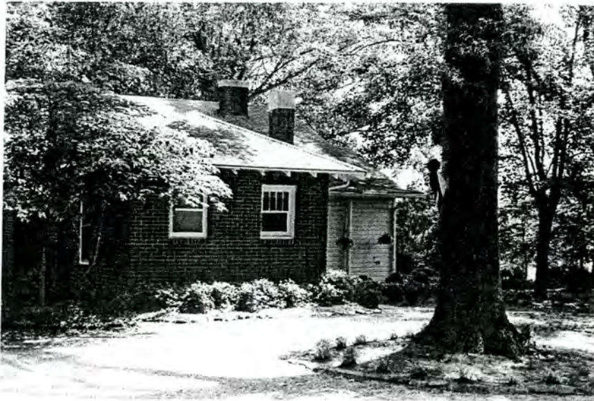
Plate 12. Secret Farmhouse, Rear Ell and Enclosed Porch, Looking Northeast.
