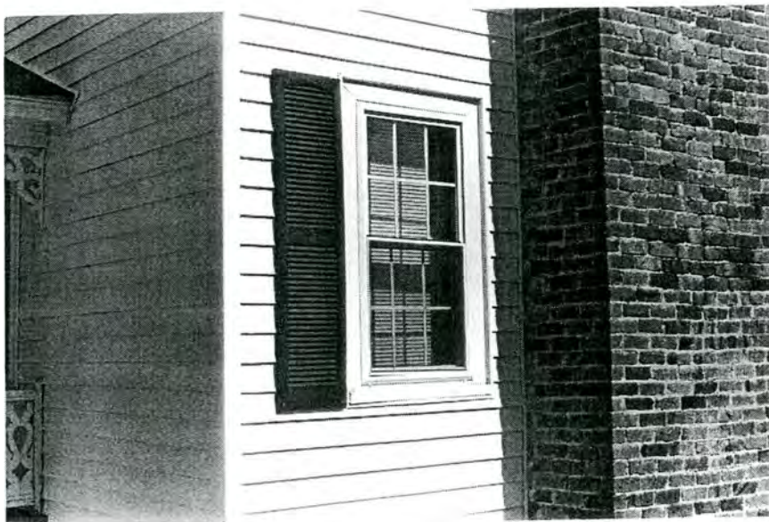
Plate 41. Stinson House, Modern Window Sash, East Elevation.
