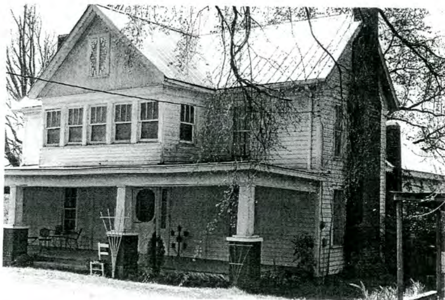
Plate 24. Secret House, Front and West Elevations, Looking Southeast.
