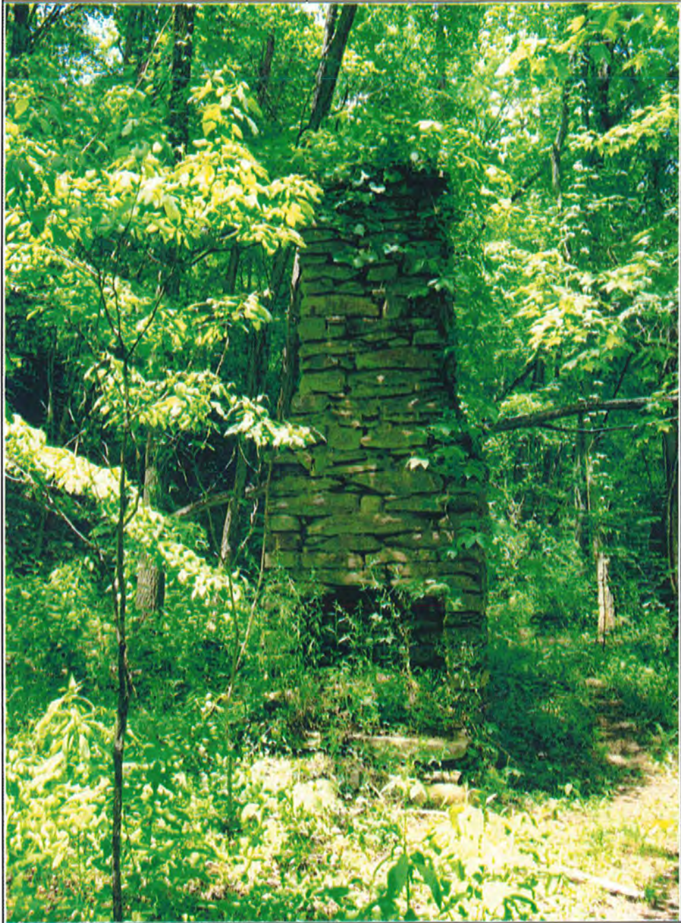
Figure 5.2. Standing chimney at Chambers Creek campsite.
