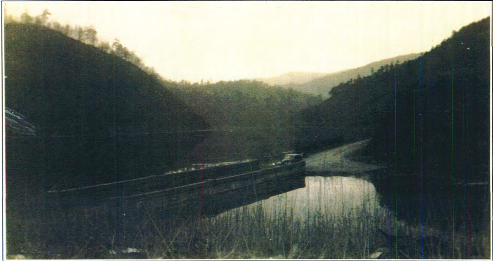
Figure 4.56. Water rising at Forney Creek Bridge.
