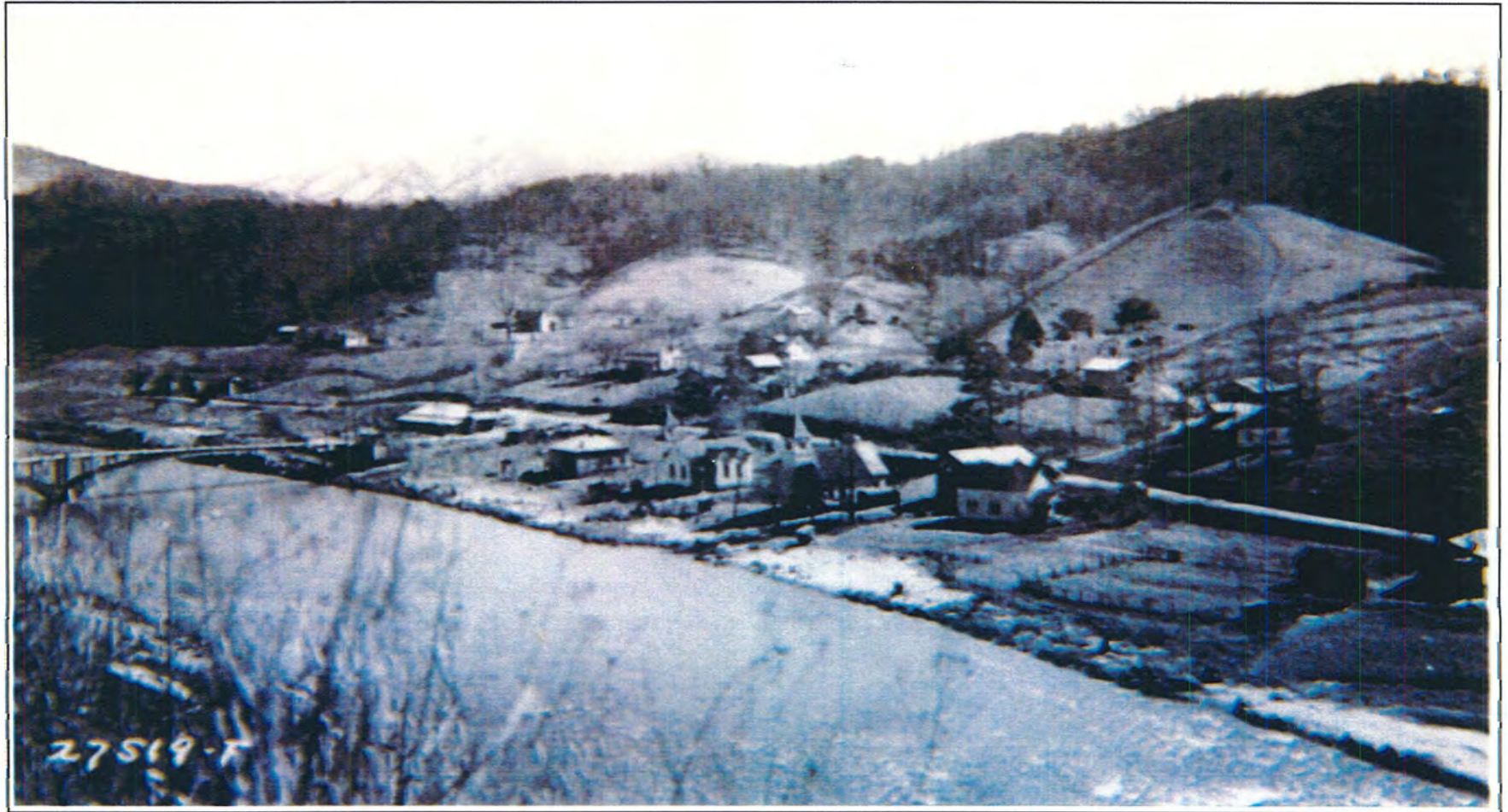
Figure 4.41. Judson (view to northeast).
