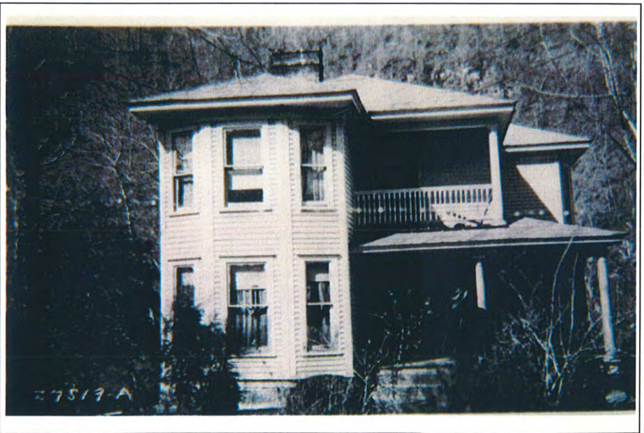
Figure 4.51. Frame house in Fontana acquisition area.
