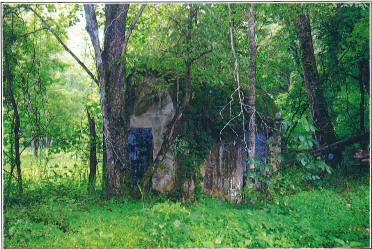
Figure 5.14. Pump or valve house at Proctor.
