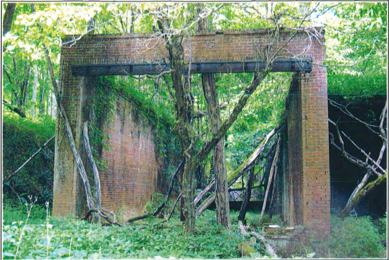
Figure 5.13. W.M. Ritter Lumber Company dry kilns at Proctor.
