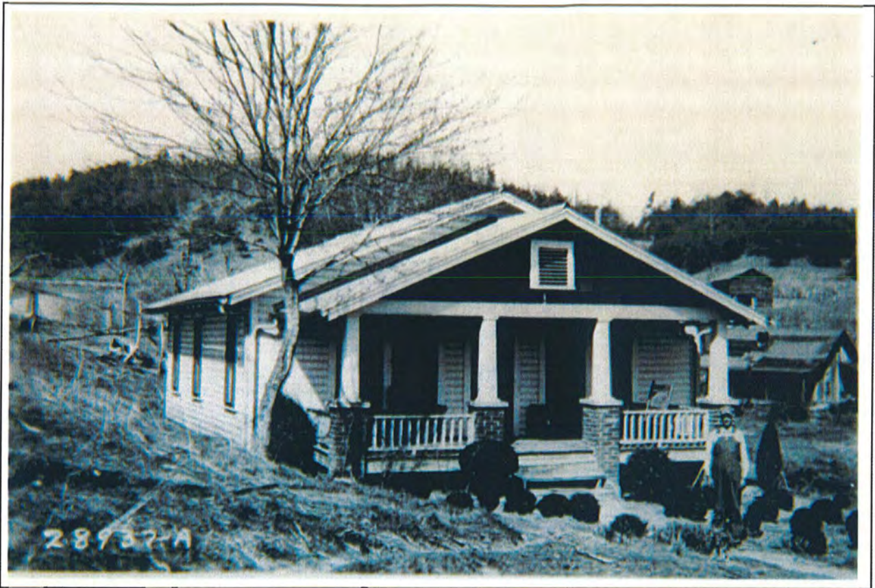
Figure 4.50. Frame house in Fontana acquisition area.
