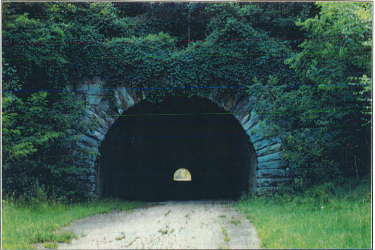
Figure 1.2. Lake View Drive tunnel through Forney Ridge.
