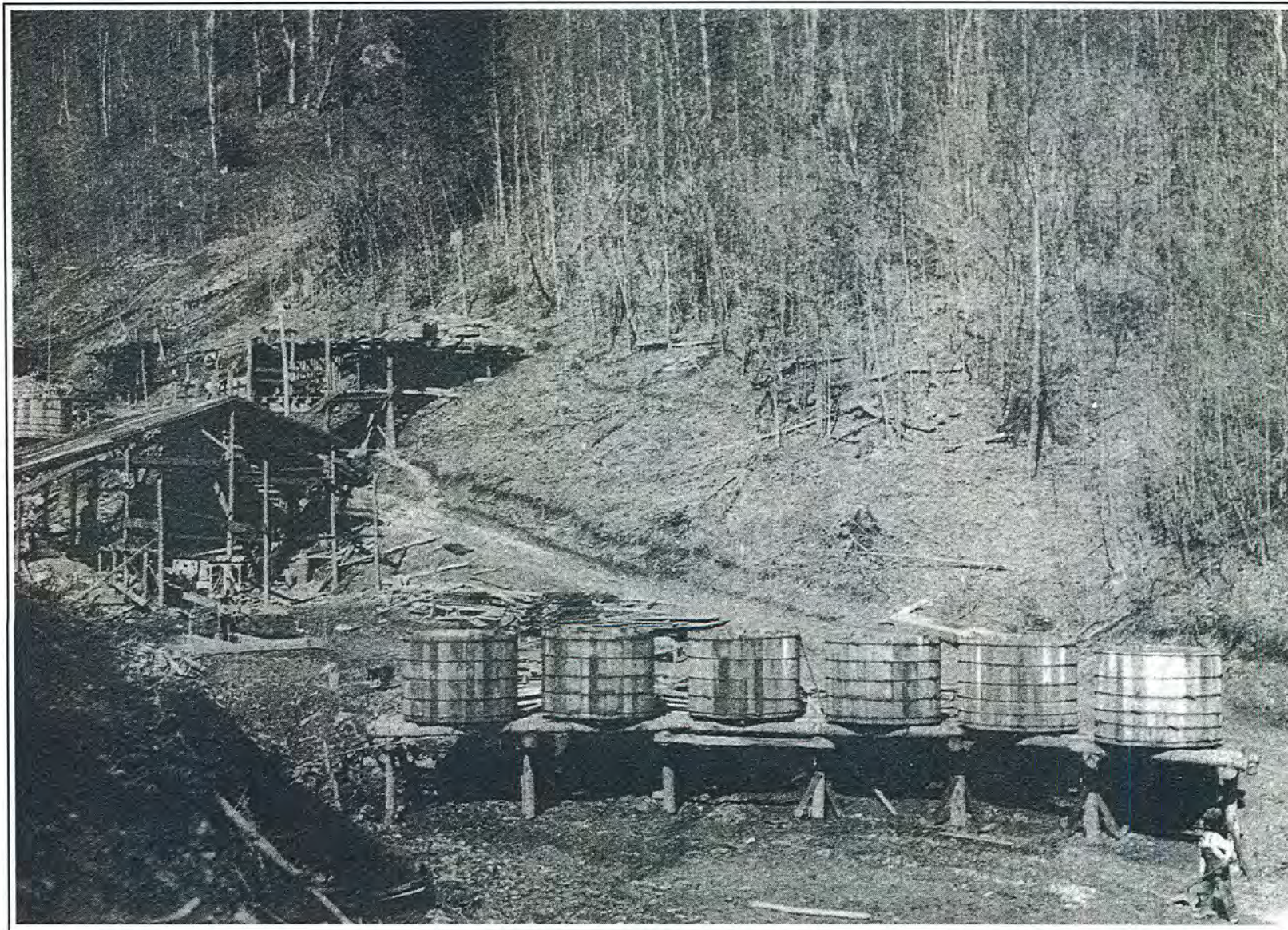
Figure 4.20. Structures and settling tanks at Adams Mine.
