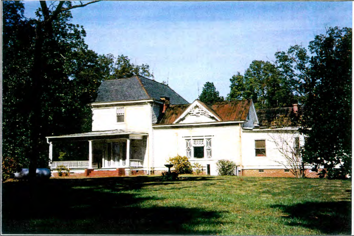
The Howard Family House--South Face
