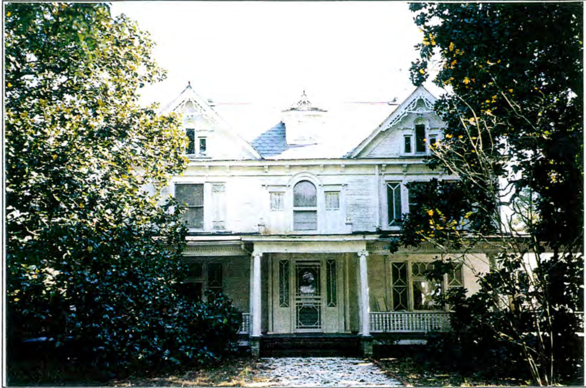
The Howard Family House--Facade
