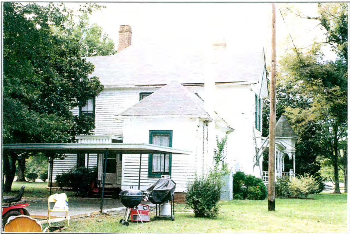
The John Walker Matthews House--rear face
