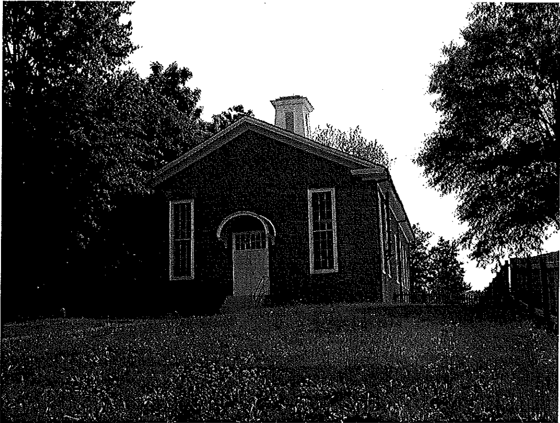
St. Philips Moravian Church, West and South Elevations
