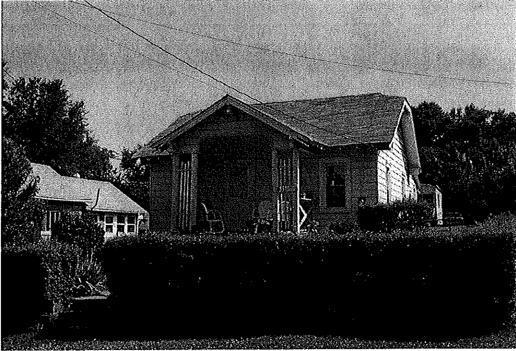
Property 20. House, circa 1920s, 511 Alexander Street
