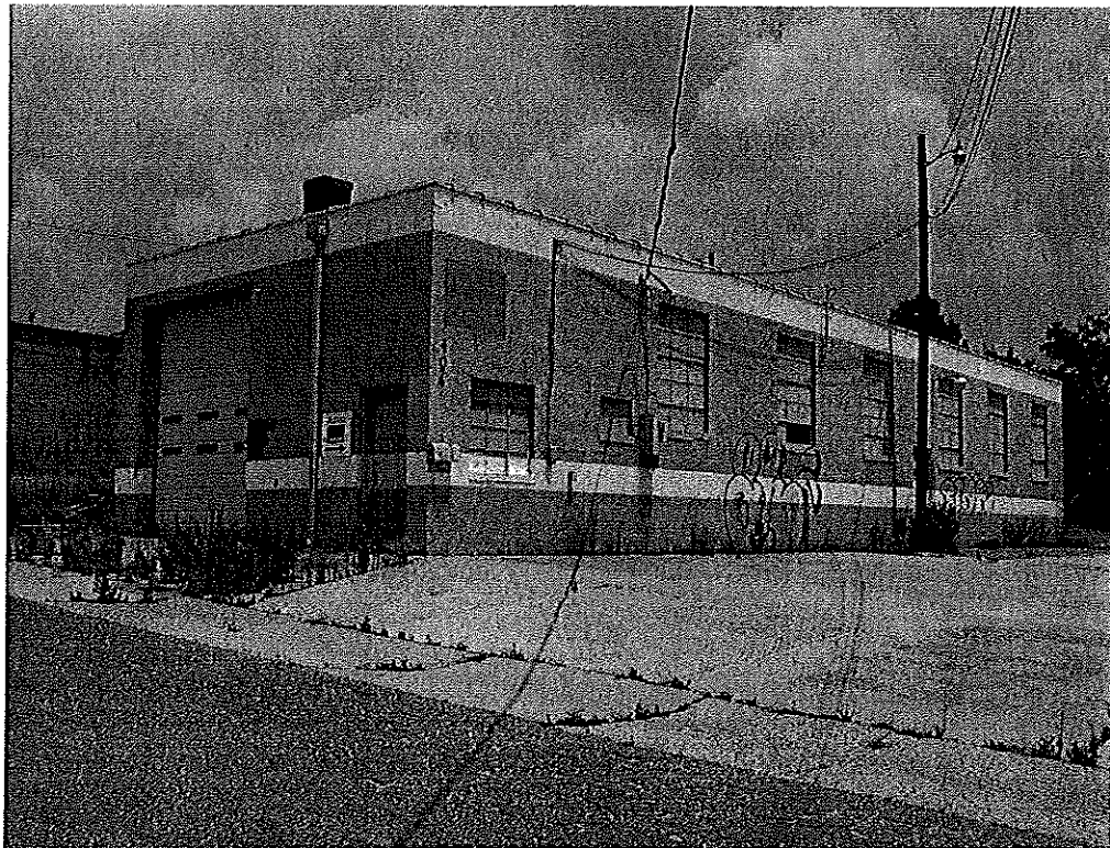
Property 195. Warehouse, 1952, 404 Dean Street
