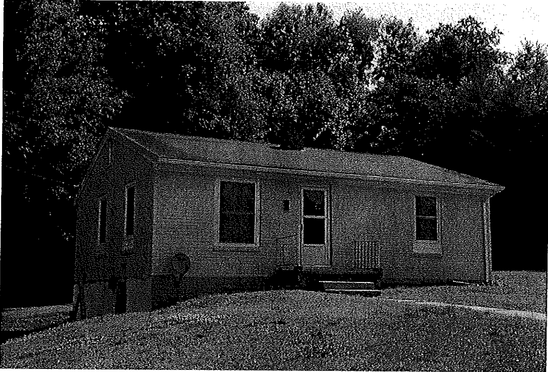
Property 7. House, circa 1950, 501 Humphrey Street
