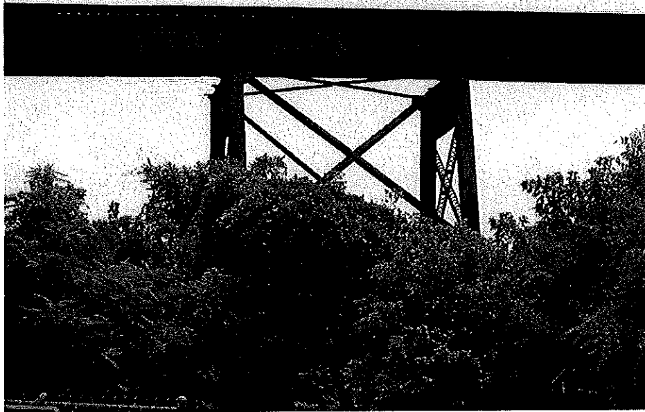
Property 190. Winston-Salem Southbound Railroad Trestle over Salem Creek, 1910
