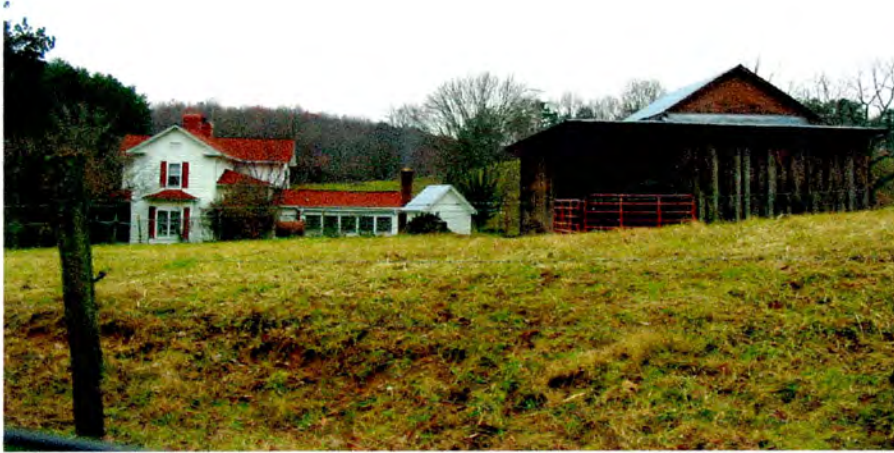
Plate 10. Albert Weaver Farm, Side (North) Elevation of House, Rear Elevation of Antebellum Smokehouse, and Rear Elevation of Milk House, Looking South.
