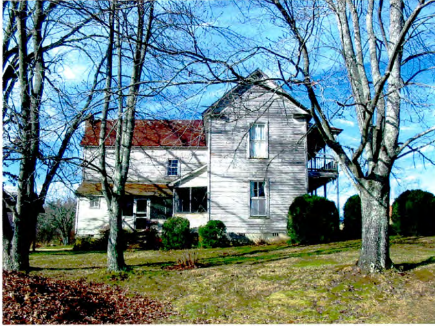
Plate 22. B.G. Hensley House, Side (East) Elevation, Looking West.
