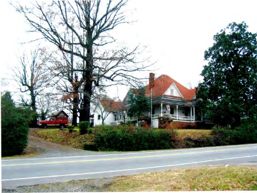
Plate 1. William Monteith House, Facade and Side (South) Elevation, Looking Northwest.
