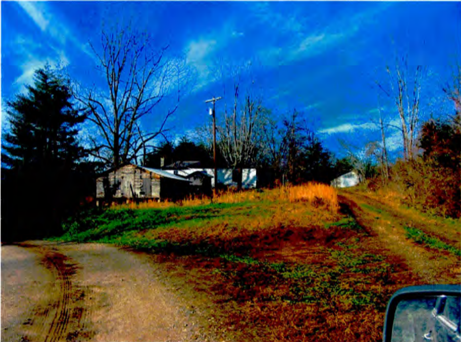
No. 29 House - Outbuildings
