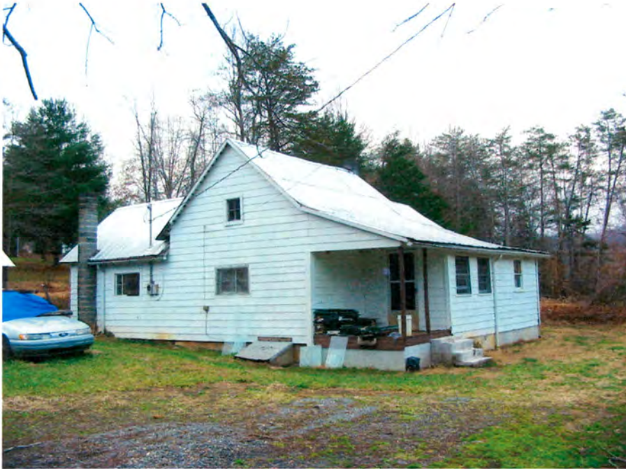
No. 25 Log House
