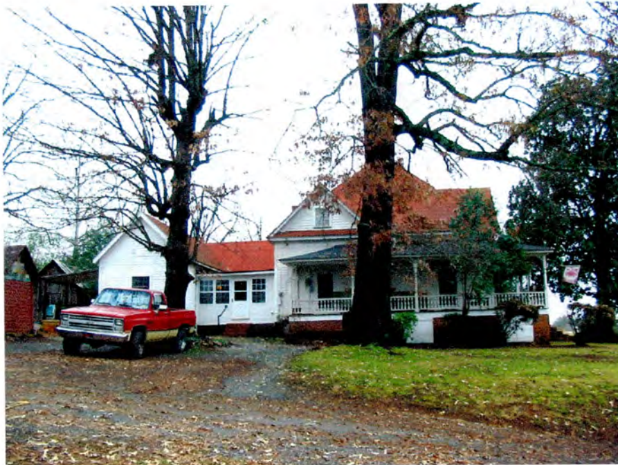
Plate 2. William Monteith House, Side (South) Elevation, Looking North.
