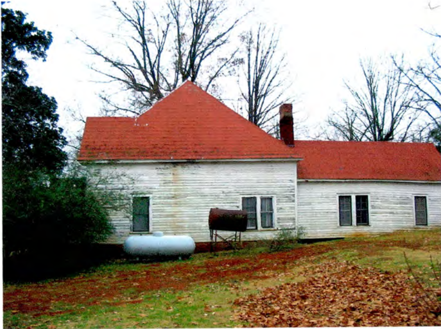
Plate 3. William Monteith House, Side (North) Elevation, Looking South.
