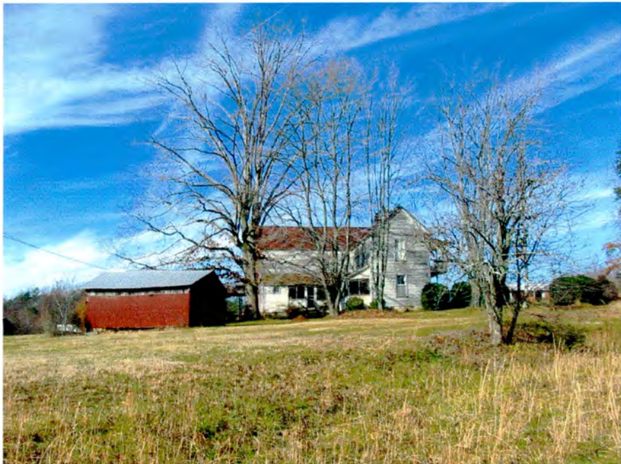
Plate 21. B.G. Hensley House, Overall View of House and Equipment Shed, Looking West.
