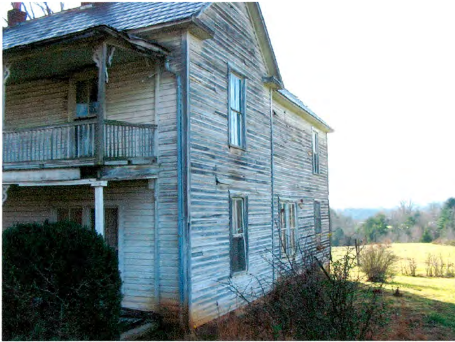
Plate 24. B.G. Hensley House, Side (West) Elevation, Looking South.
