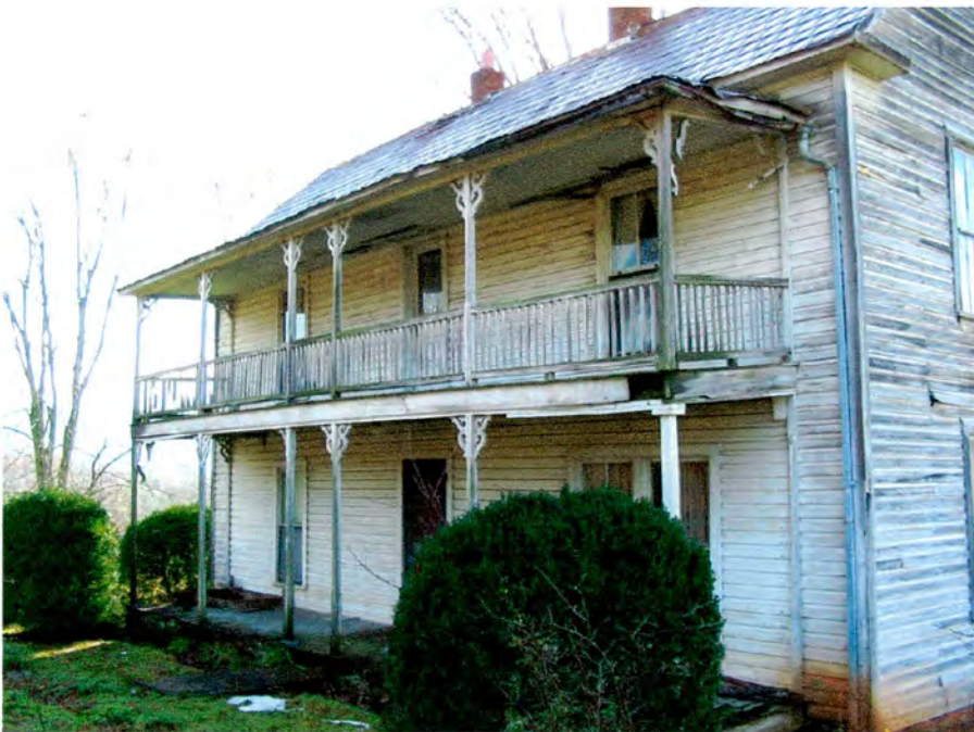
Plate 25. B.G. Hensley House, Facade, Looking Southeast.
